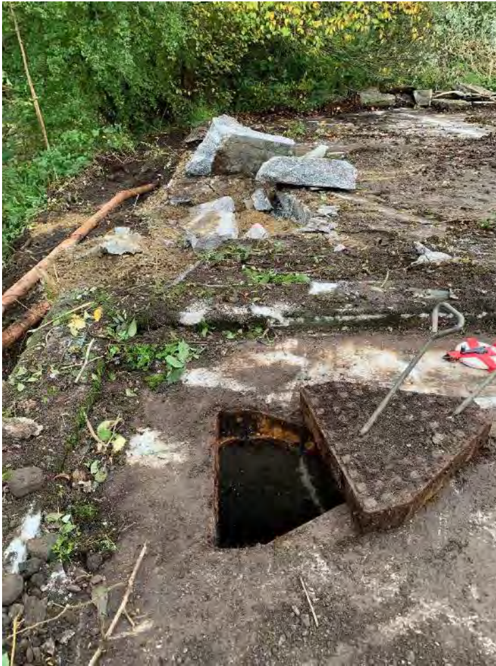
Photo of MH 4702 with evidence of 150mm dia plastic pipe former site connection on far side of channel. Flow going right to left.
