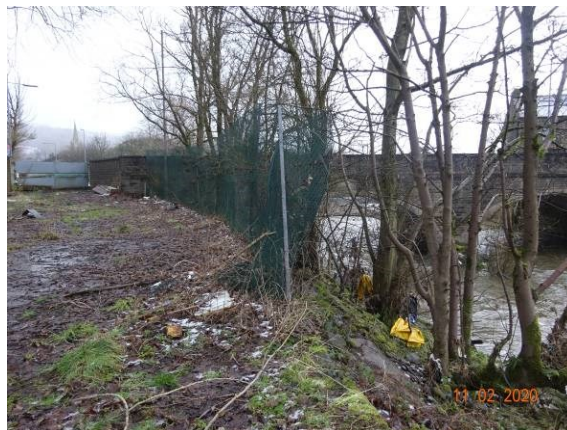
Pic 5 shows the view looking north west along the eastern perimeter towards its north eastern corner. The bank down to the River Irwell can also be seen on the right of the picture.
