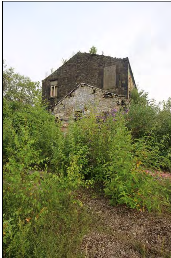
Photograph 27: View of the outline of a former structure which adjoined the southern elevation of building B
