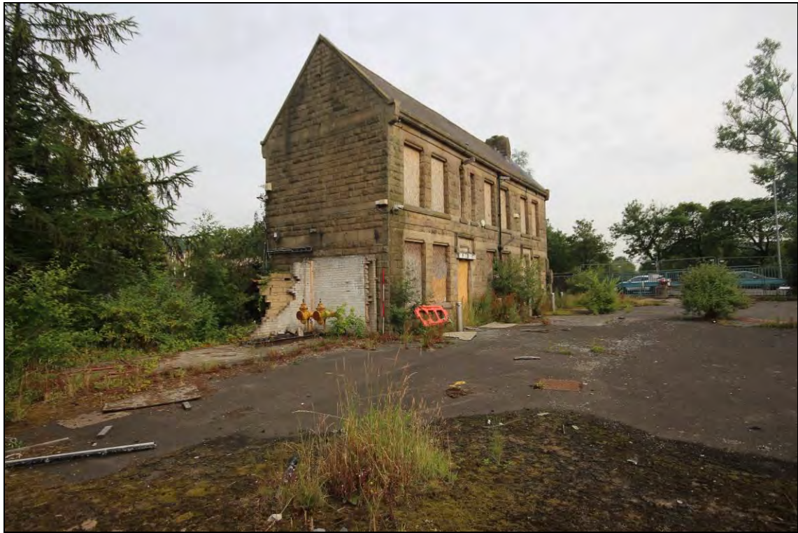
Photograph 21: View of building A facing north-west, 2m scale
