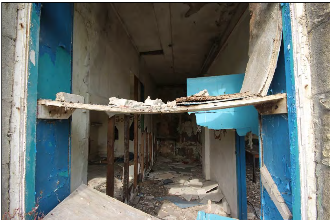
Photograph 32: View of one section of the interior of building C, facing west
