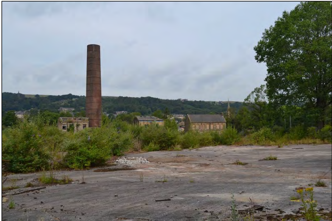
Photograph 7: General view north-west across the site
