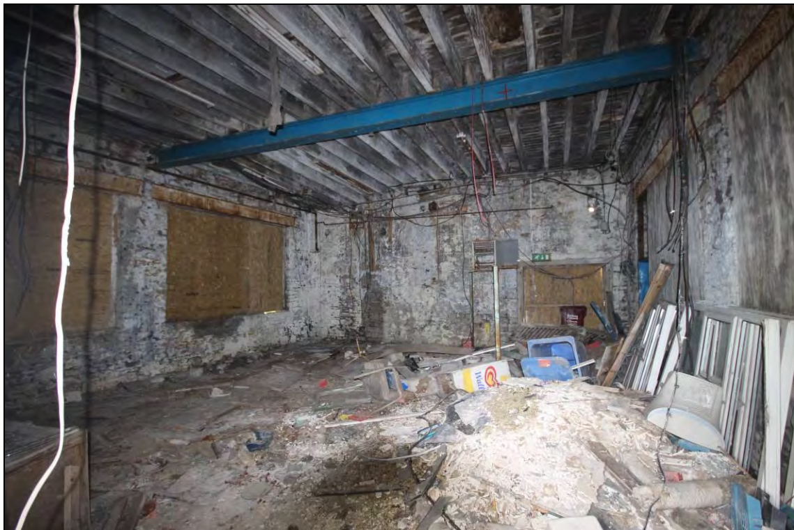
Photograph 28: General view of the ground floor space in building B, facing north-west
