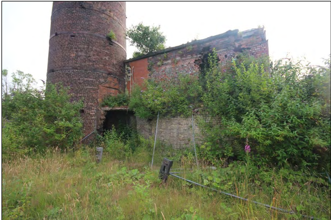
Photograph 31: View of the western elevation of building C adjoining the chimney
