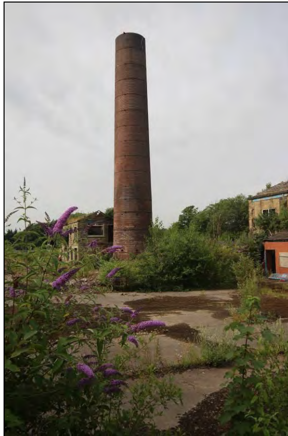
Photograph 33: General view of the reduced chimney, facing south-west
