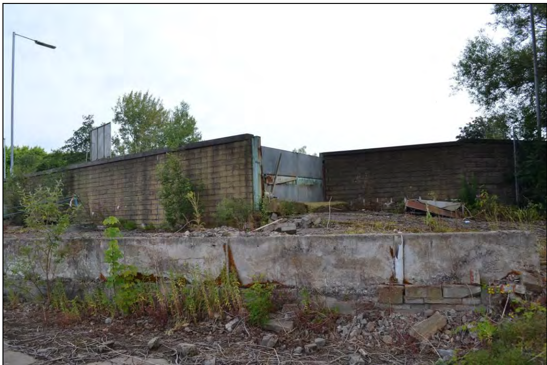
Photograph 2: View north-west of the second site entrance, adjacent Peel Bridge
