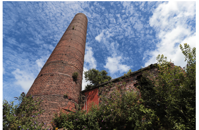
Image 14 – Existing Building C (West Elevation) Plus Chimney
