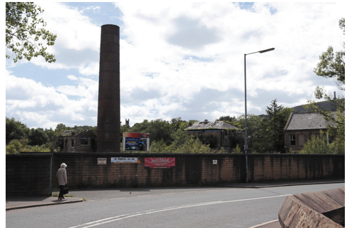
Image 22 – South West Facing View of Application Site from Bridge
