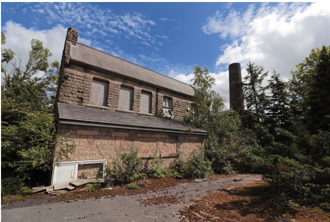
Image 5 – Existing Building A, West Elevation
