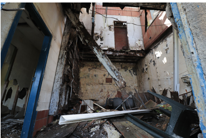
Image 15 – Existing Building C Interior
