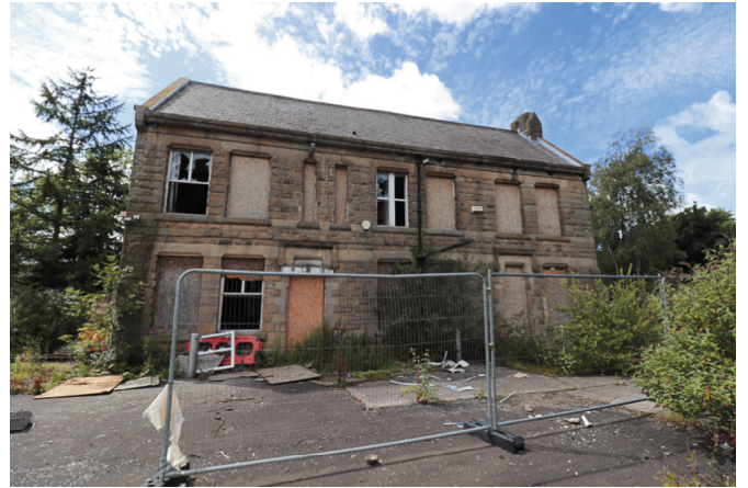
Image 2 – Existing Building A, East Elevation
