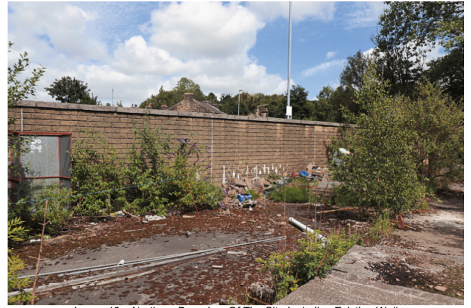
Image 18 – Northern Boundary Of The Site Including Existing Wall
