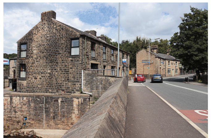
Image 24 – North-West Facing Views from Bridge
