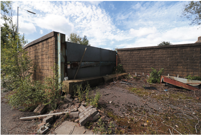
Image 19 – Gate on Northern Boundary Wall at Curve of Bridge Street
