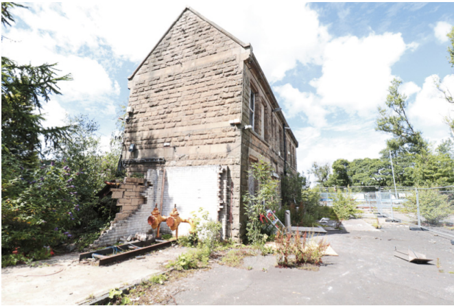
Image 3 – Existing Building A, South Elevation
