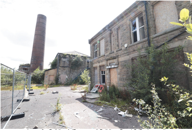
Image 9 – Building A (Foreground) Buildings B and C (Background)
