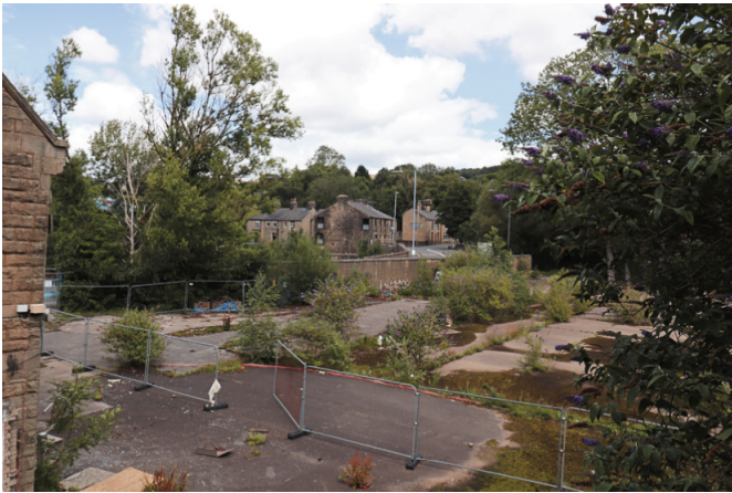
Image 11 – Elevated 1st Floor View from Existing Building B Towards Bridge Street (Facing North-East)
