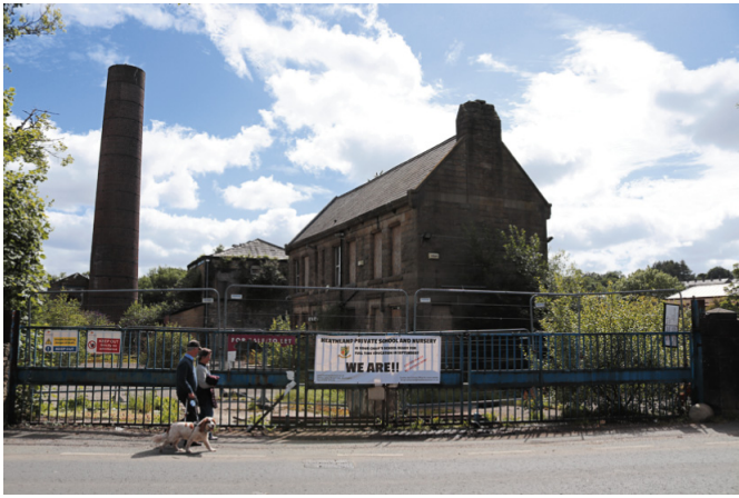
Image 36 – South Facing View of Application Site from Bridge Street
