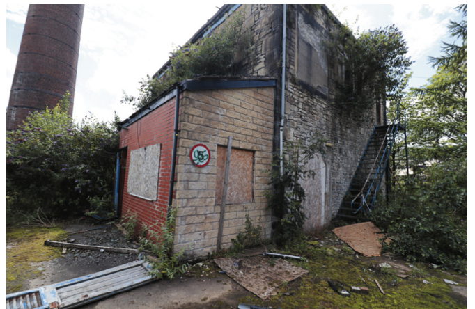
Image 8 – Existing Building B, North and East Elevations
