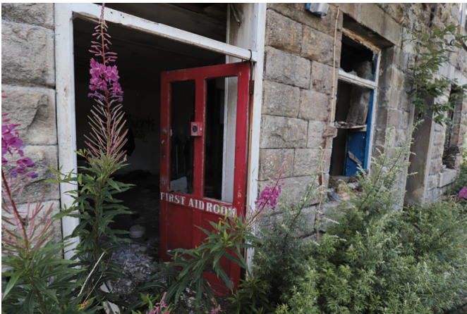
Image 13 – Existing Building B, East Elevation
