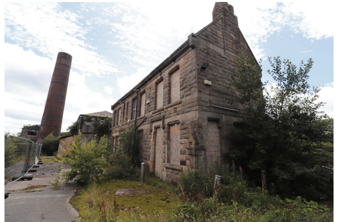
Image 6 – Existing Building A, North and East Elevations
