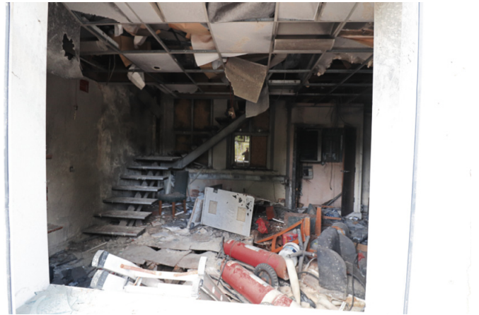
Image 4 – Existing Building A, Interior
