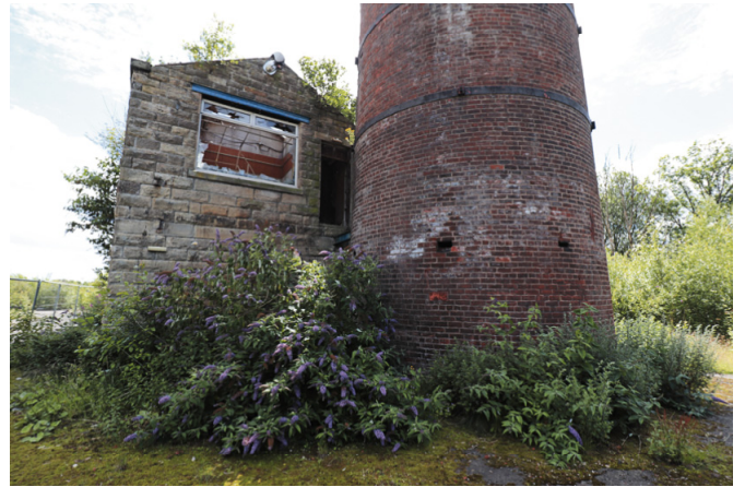
Image 12 – Existing Building C North Elevation (And Chimney)
