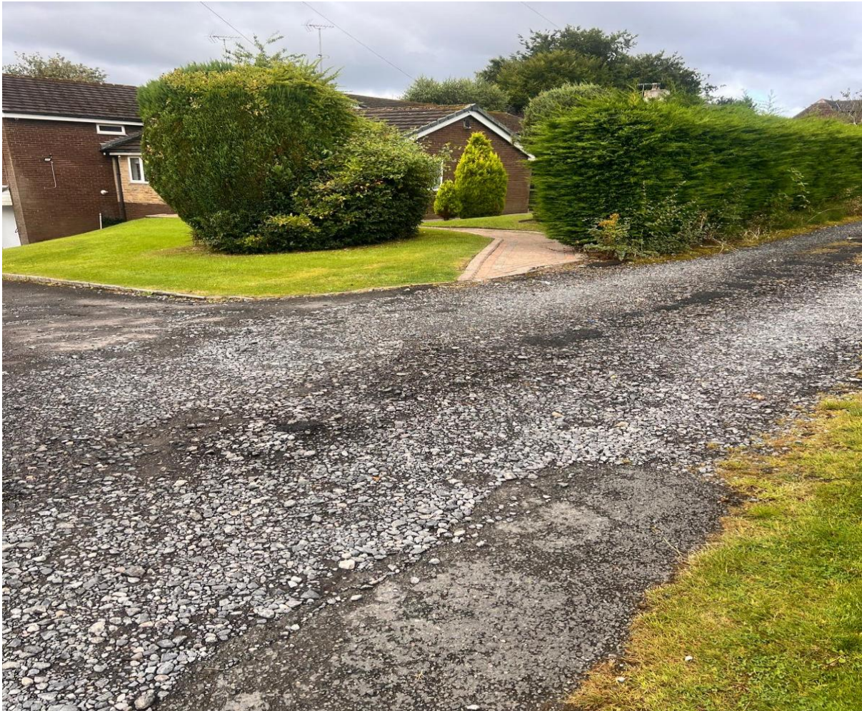
The above Photo illustrates the existing hedge row which will be partly removed to accommodate amended access and visibility .
