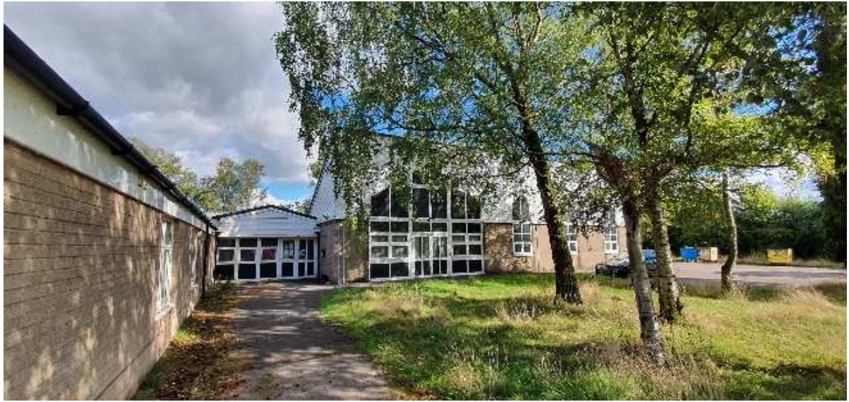
Fig.3 – Front Aspect, view from Pole Lane
