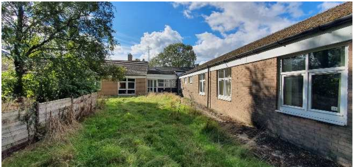
Fig.4 – Rear/side aspect, view from South elevation
