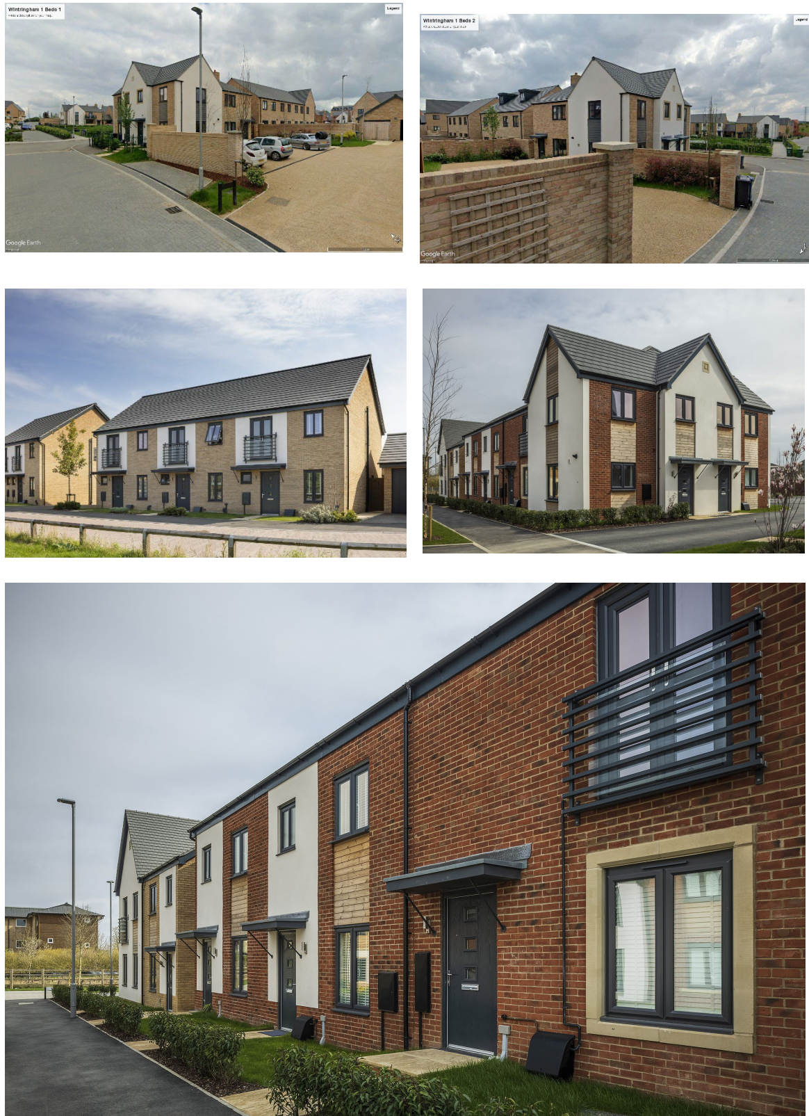
Fig 5. Further typical contemporary modern affordable housing scheme completed by Morris Homes utilising similar dwellings to those proposed at the former East Lancs Paper Mill.
