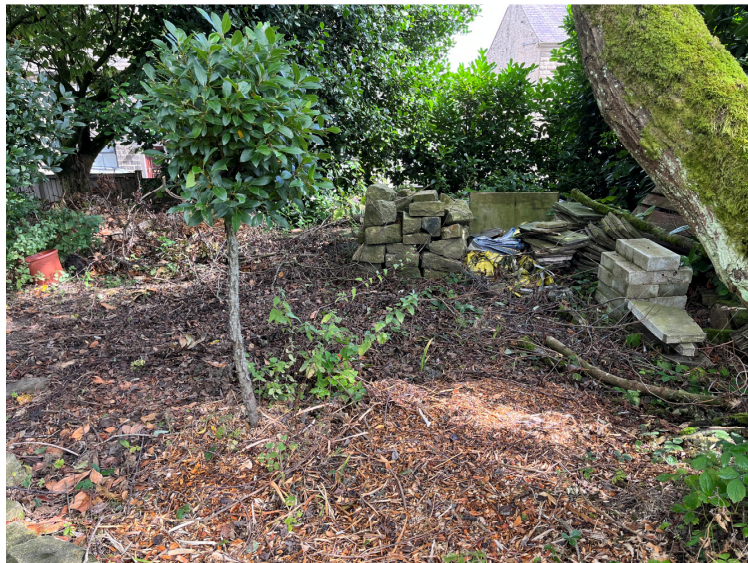
Clearing intended for the new out-building
