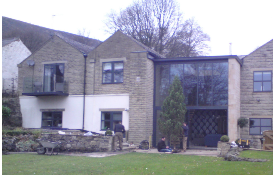
Recent infill between the wings of Tower View
