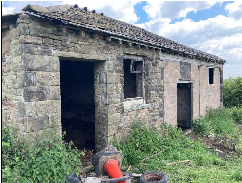
Photograph 1 showing the front elevation of the building
