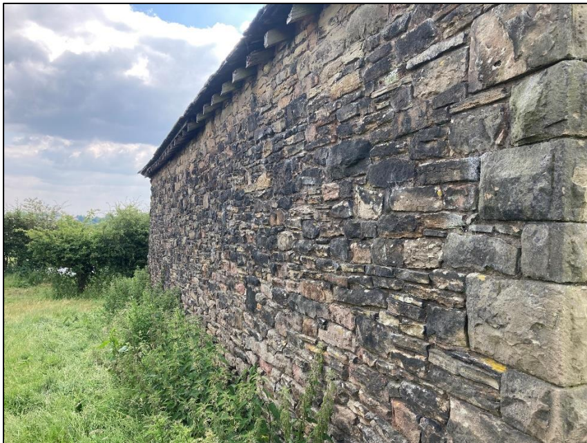
Photograph 2 showing the rear elevation of the building
