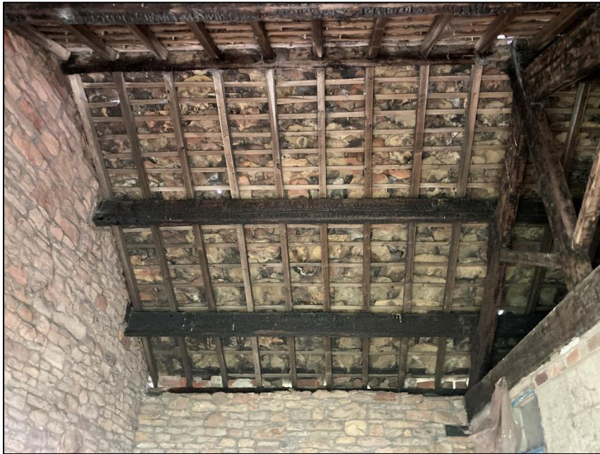
Photograph 7 showing the roof structure
