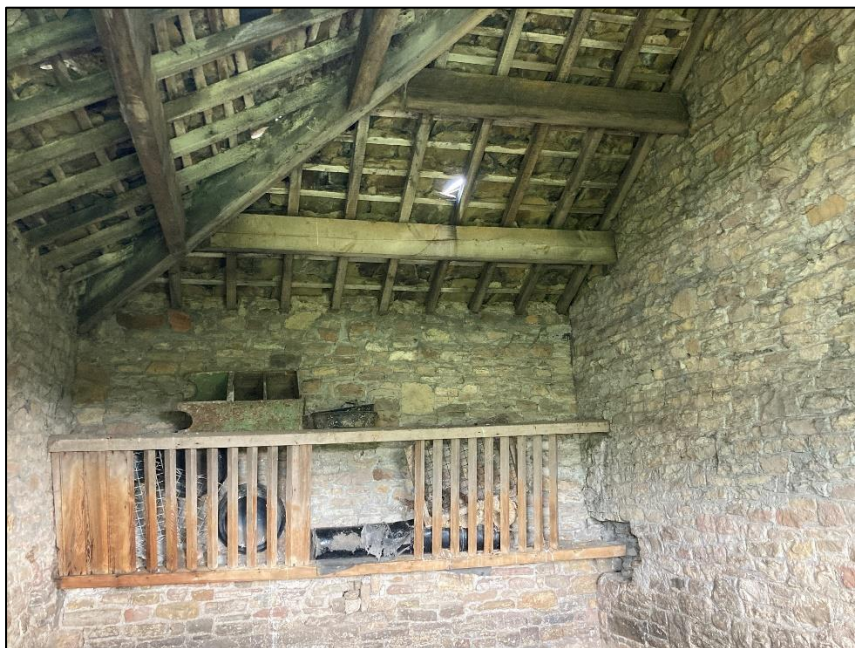
Photograph 5 showing the interior walls and roof structure of one half
