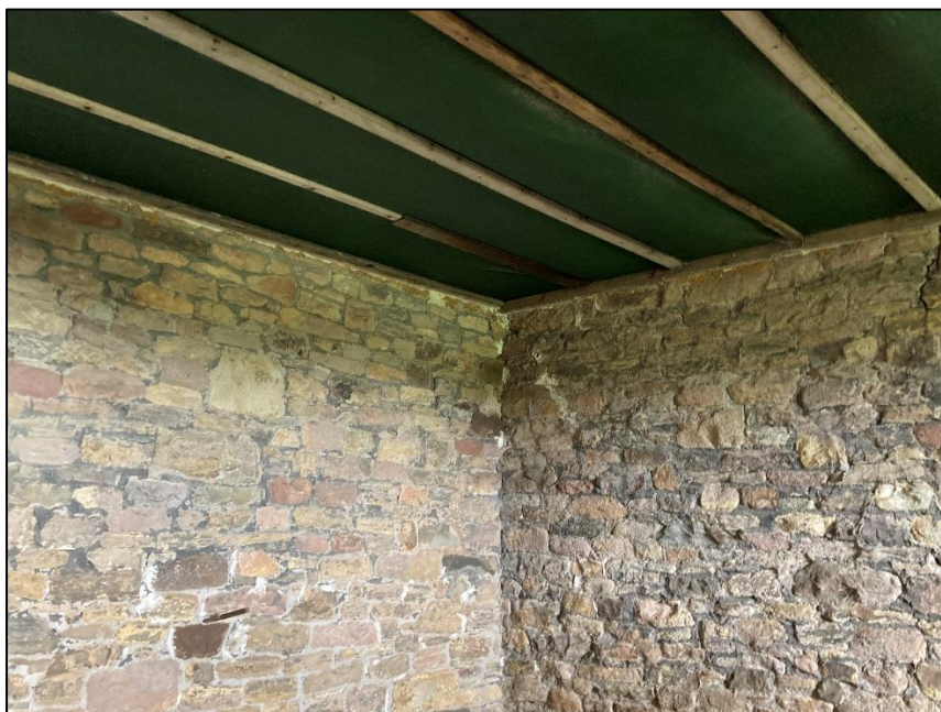
Photograph 6 showing the interior walls and roof structure of the other half
