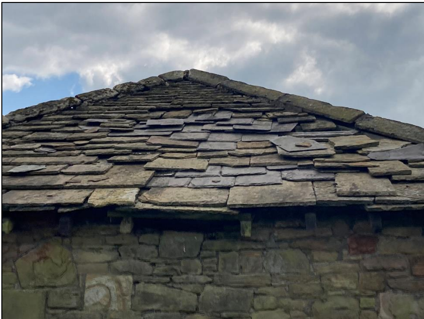
Photograph 4 showing the roof tiles on one elevation
