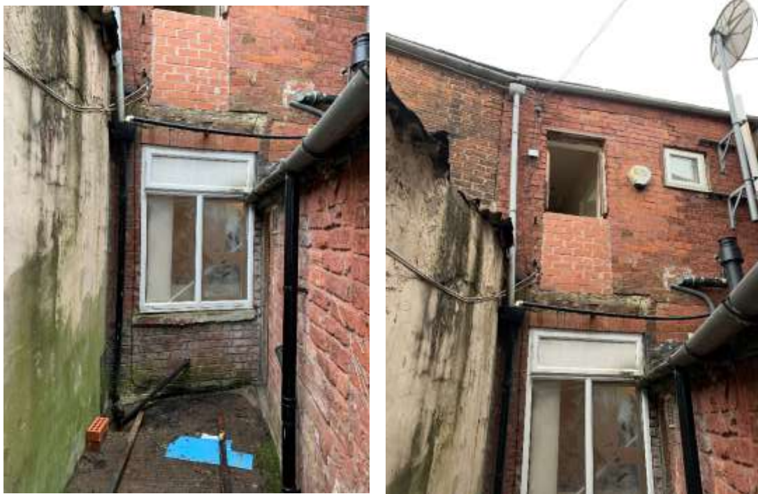
Fig 2. Rear of main property and single-storey extension
