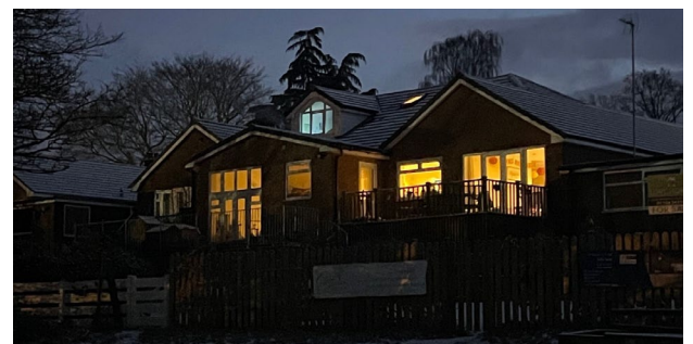
Image A - 14 Ashborne Drive with similar roof form on extension
