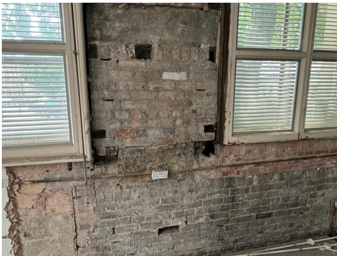
Photo 34: Ground floor main hall, exposed brickwork with missing bricks
