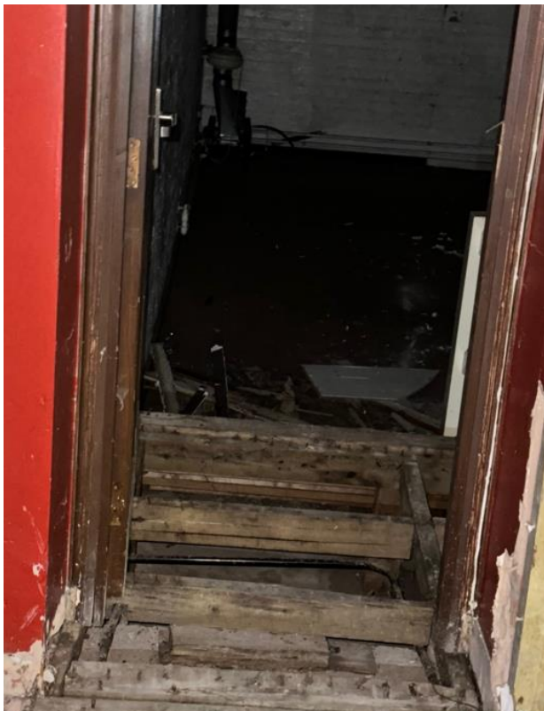
Photo 19: First floor rear room, rotten floor joists
