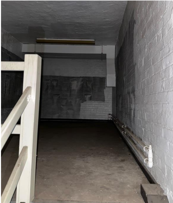
Photo 20: First floor mezzanine floor
