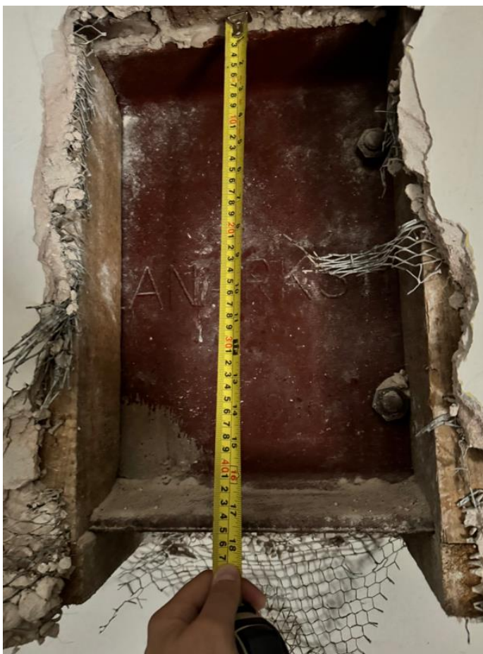
Photo 23: Ground floor mezzanine, room 1 exposed steelwork
