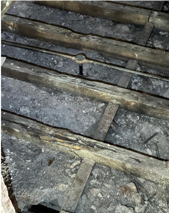
Photo 19: First floor rear room, rotten floor joists
