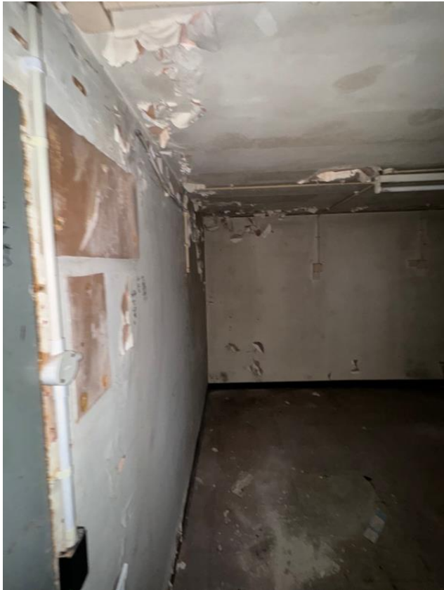
Photo 49: Ground floor rear, ext vault
