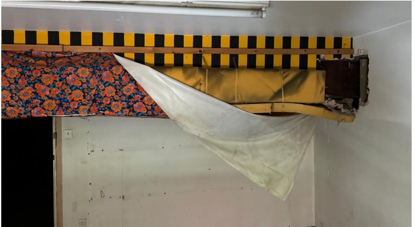
Photo 23: Ground floor mezzanine, room 1 exposed steelwork
