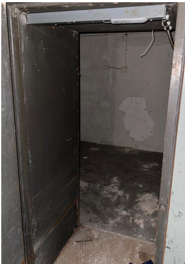
Photo 44: Ground floor rear, ext bank vault
