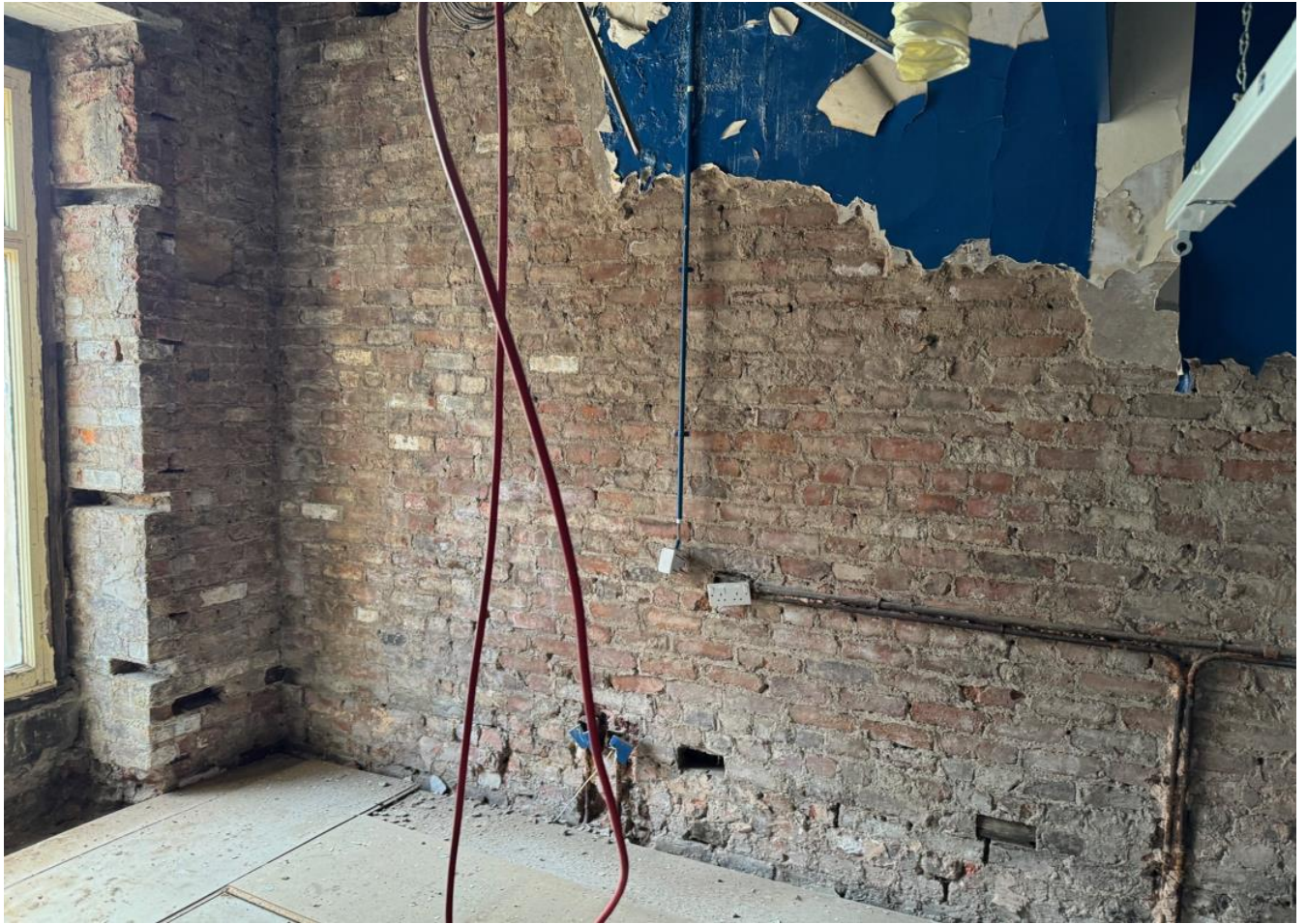
Photo 11: First floor room 1, moderate exposed brickwork
