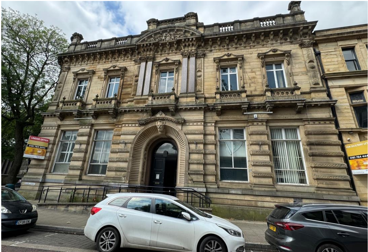
Photo 1: External Front Elevation
