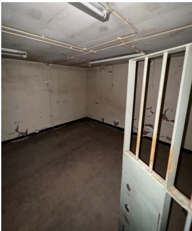
Photo 50: Ground floor rear, ext vault
