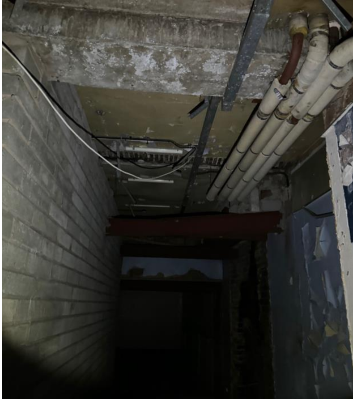
Photo 40: Ground floor rear, exposed steels
