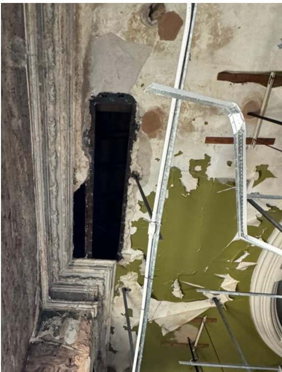
Photo 10: First floor room 1 damaged ceiling and coving
