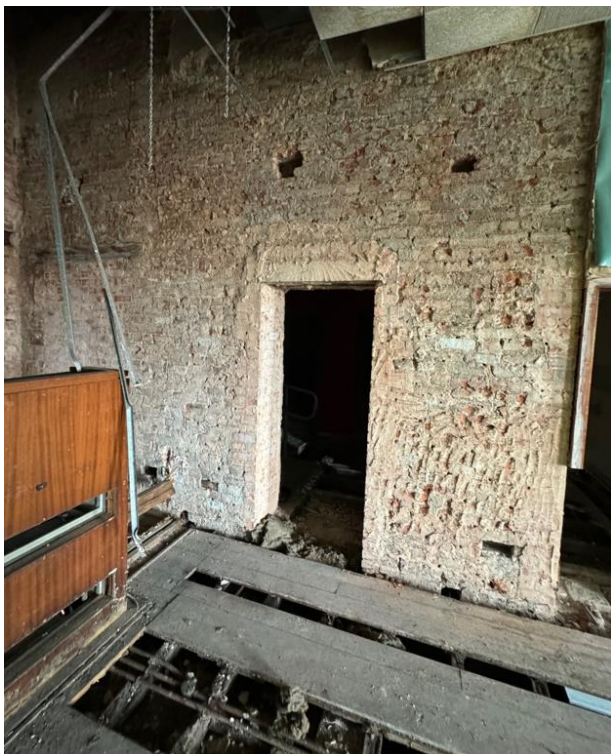
Photo 15: First floor rear of the hall, Exposed damage brickwork
