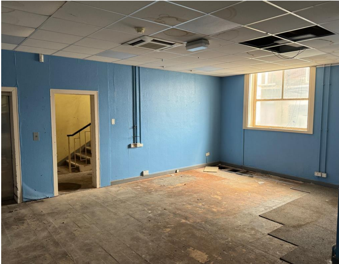
Photo 30: Ground floor main hall, Damage floor
