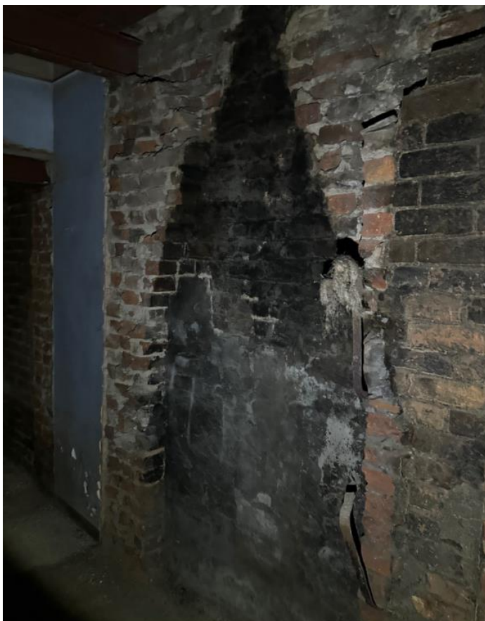
Photo 42: Ground floor rear, removed chimney
