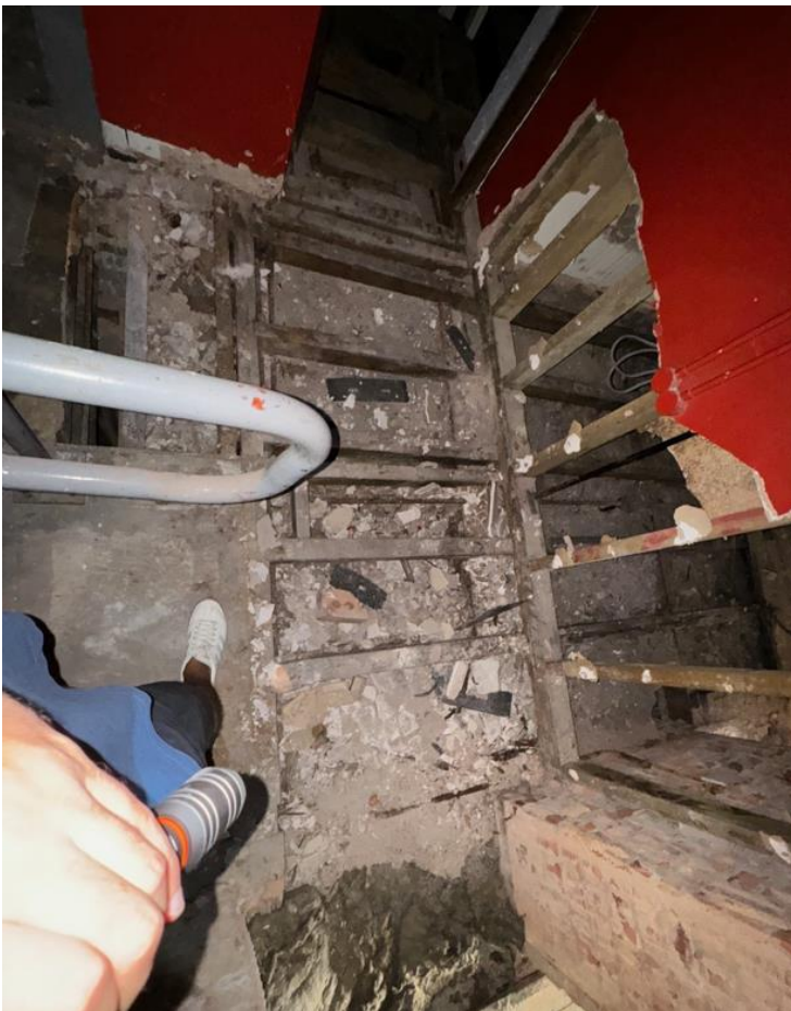
Photo 17: First floor rear room, rotten floor joists
