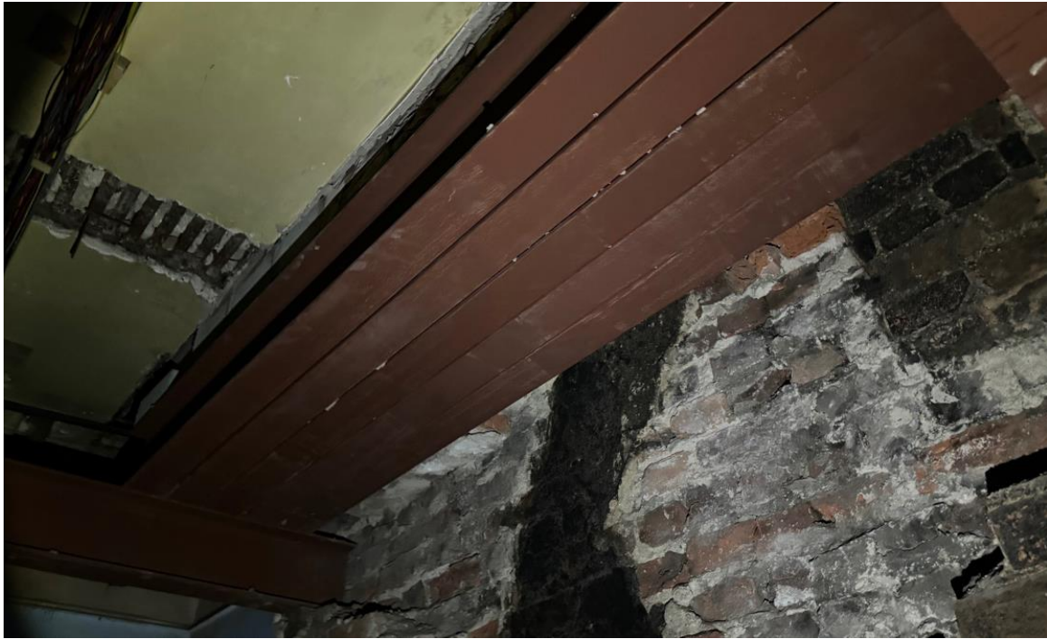
Photo 42: Ground floor rear, removed chimney
