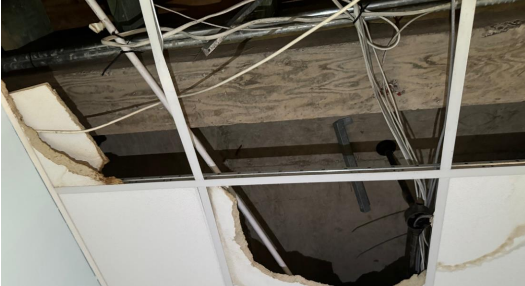
Photo 37: Ground floor rear of main hall, exposed beam
