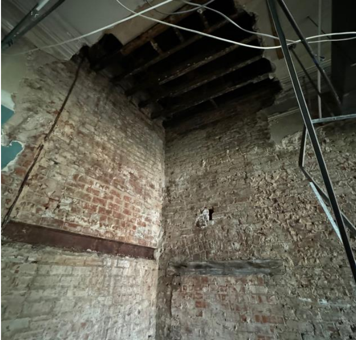
Photo 17: First floor rear room, rotten floor joists
