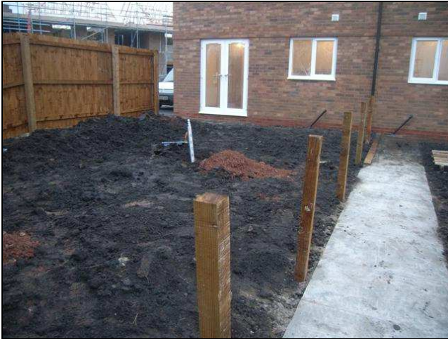
Photographs 1 and 2: Examples of validation photographs demonstrating validation hole location and soils forming inert cover.
