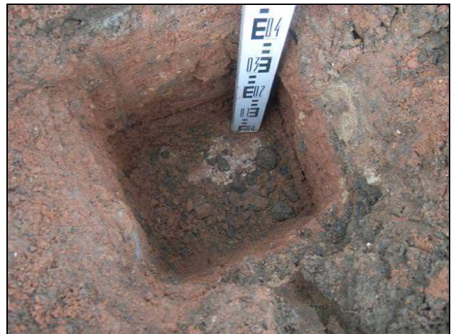
Photographs 3 and 4: Examples of validation photographs demonstrating inert cover depth and geotextile.
