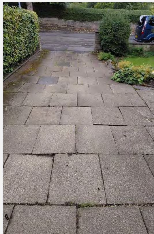
Plate 4: Facing northwest to Delamere Road (driveway)
