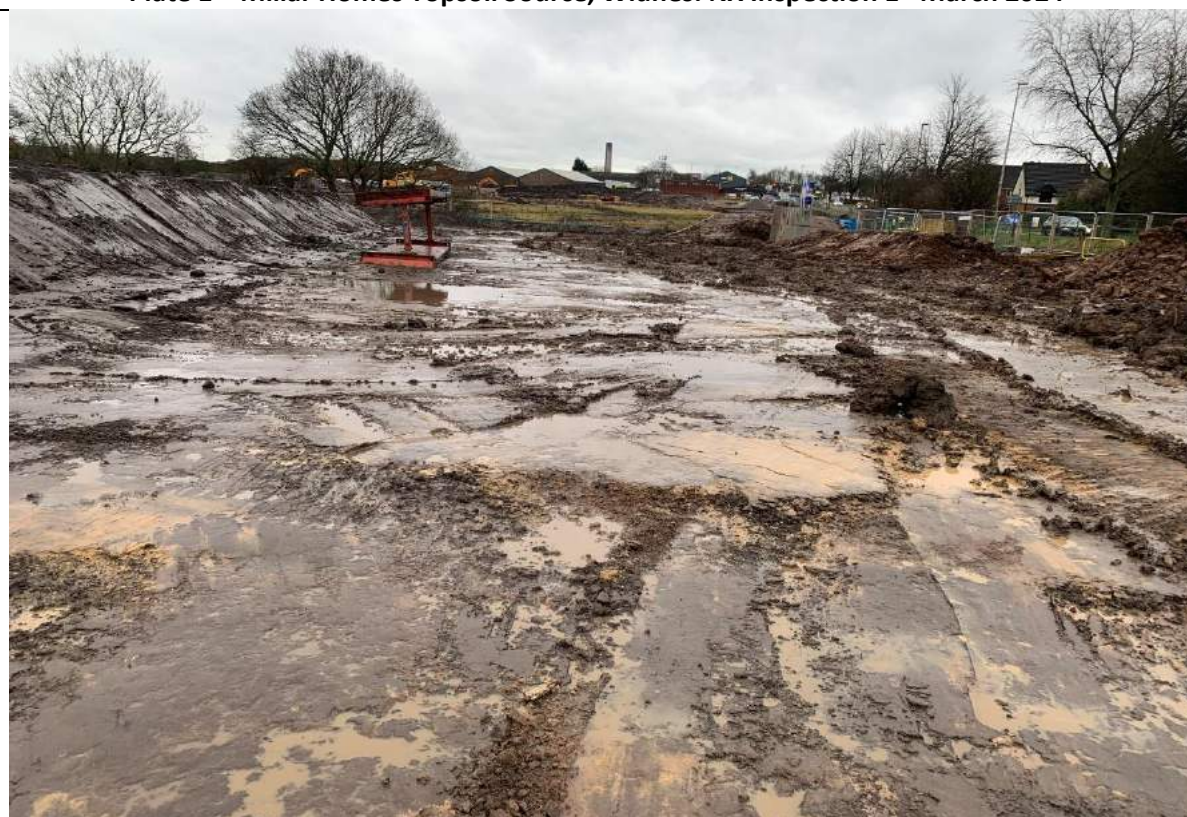
Plate 2 – Millar Homes Topsoil Source, Widnes. NX Inspection 1 st March 2024
