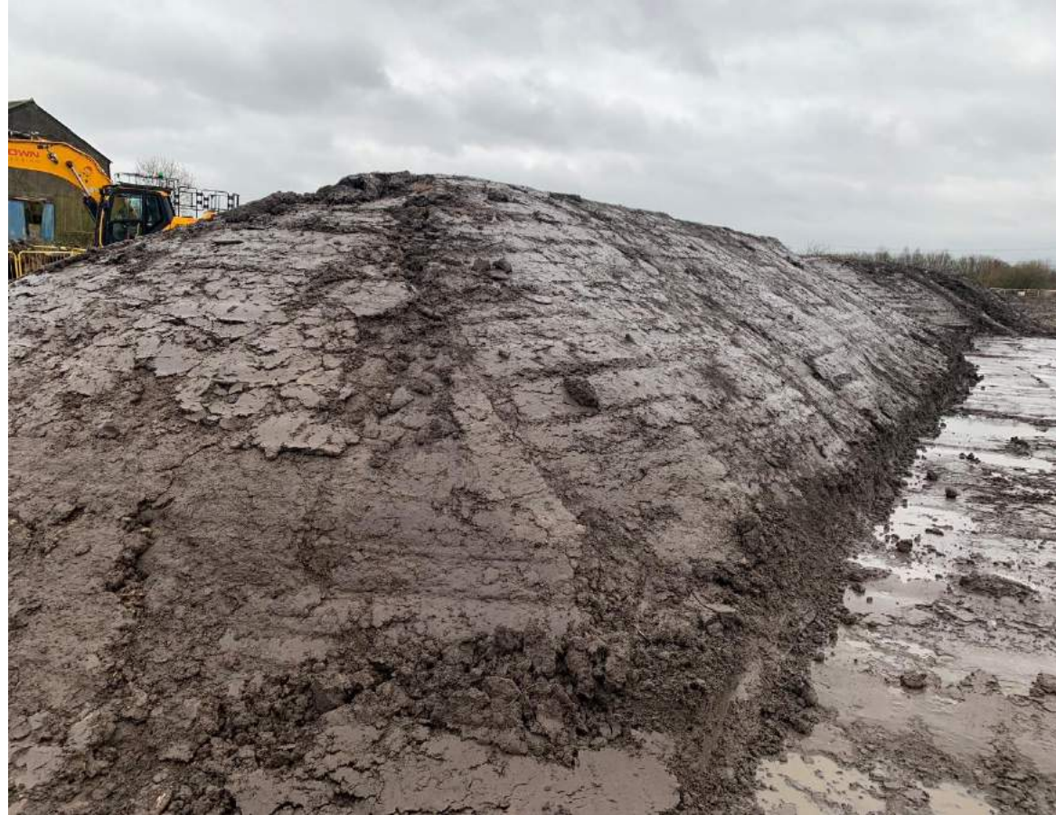
Plate 3 – Millar Homes Topsoil Source, Widnes. NX Inspection 1 st March 2024
