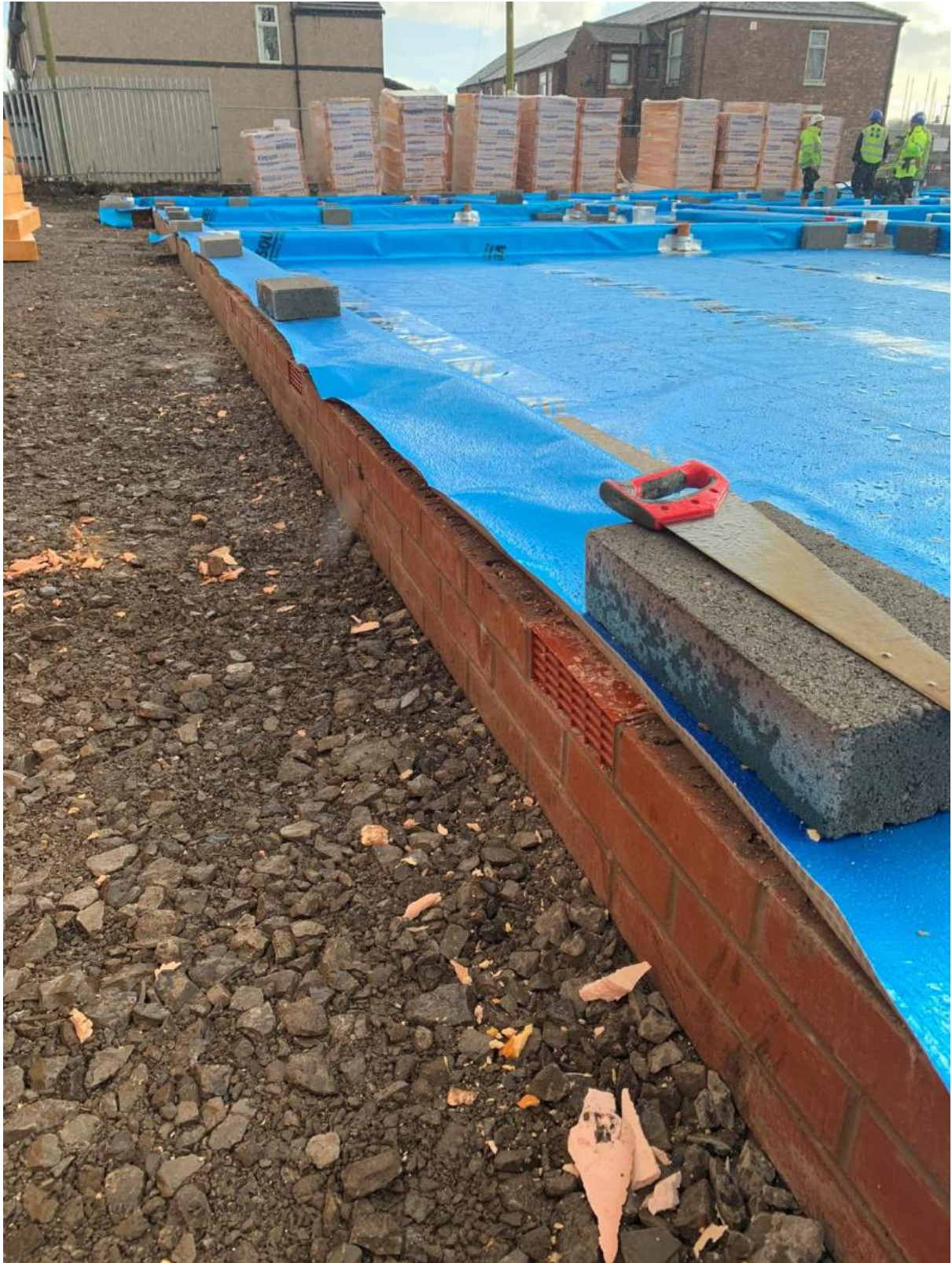
PLATE 8: Subfloor Venting on 2m to 3m centres
