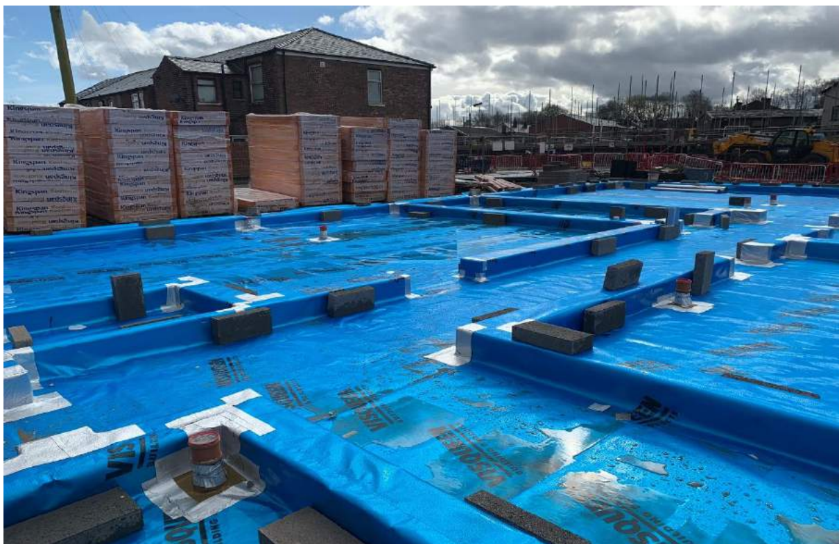
PLATE 5: Membrane Coverage and internal Wall lapping
