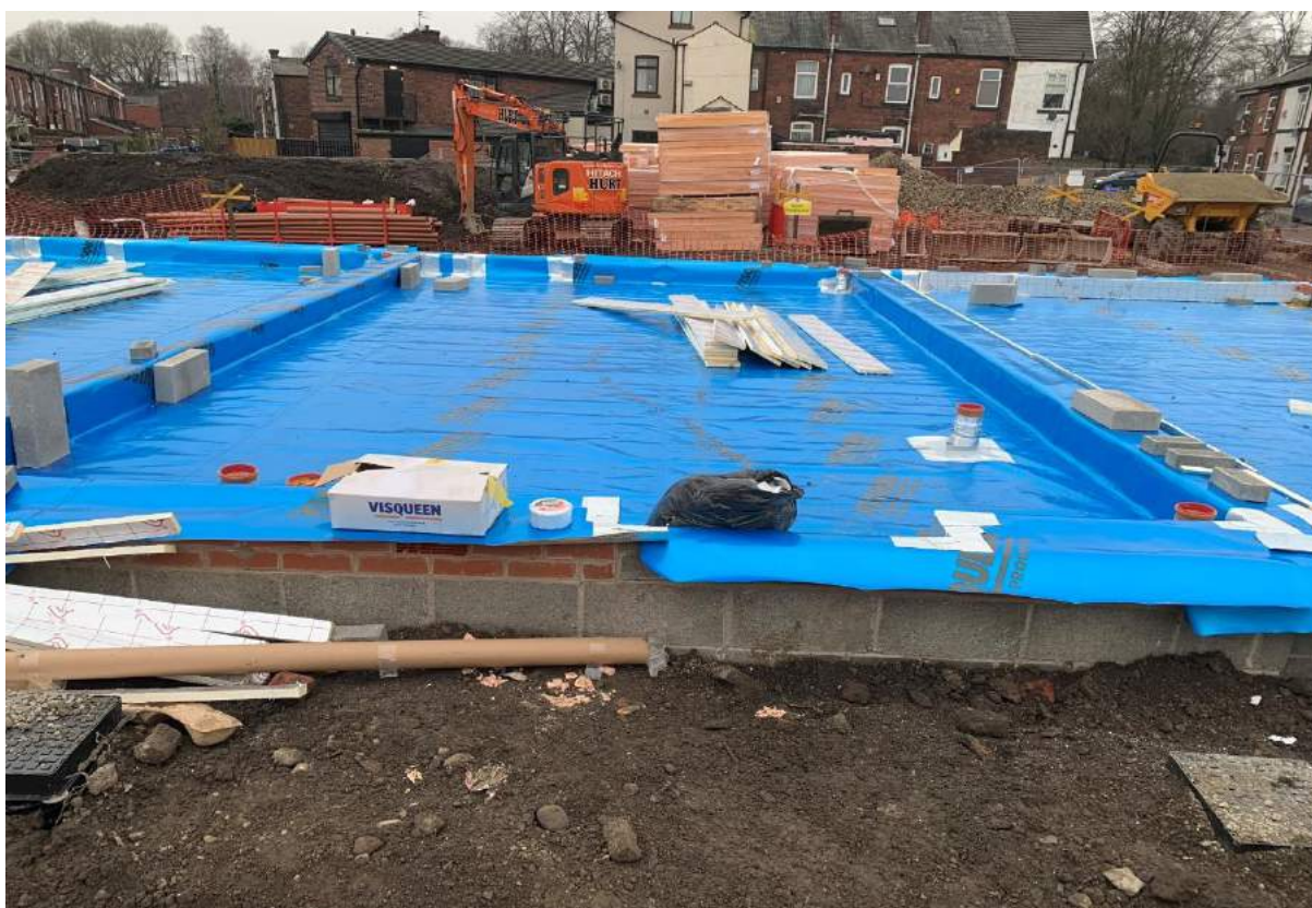
PLATE 2: Plots 2, 3, 4 with Full Visqueen Barrier Coverage
