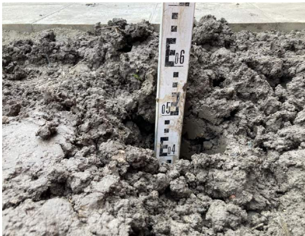
Plate 8 – Plot 2 front garden cover system GL to 0.60mbgl with 0.15m of topsoil.
