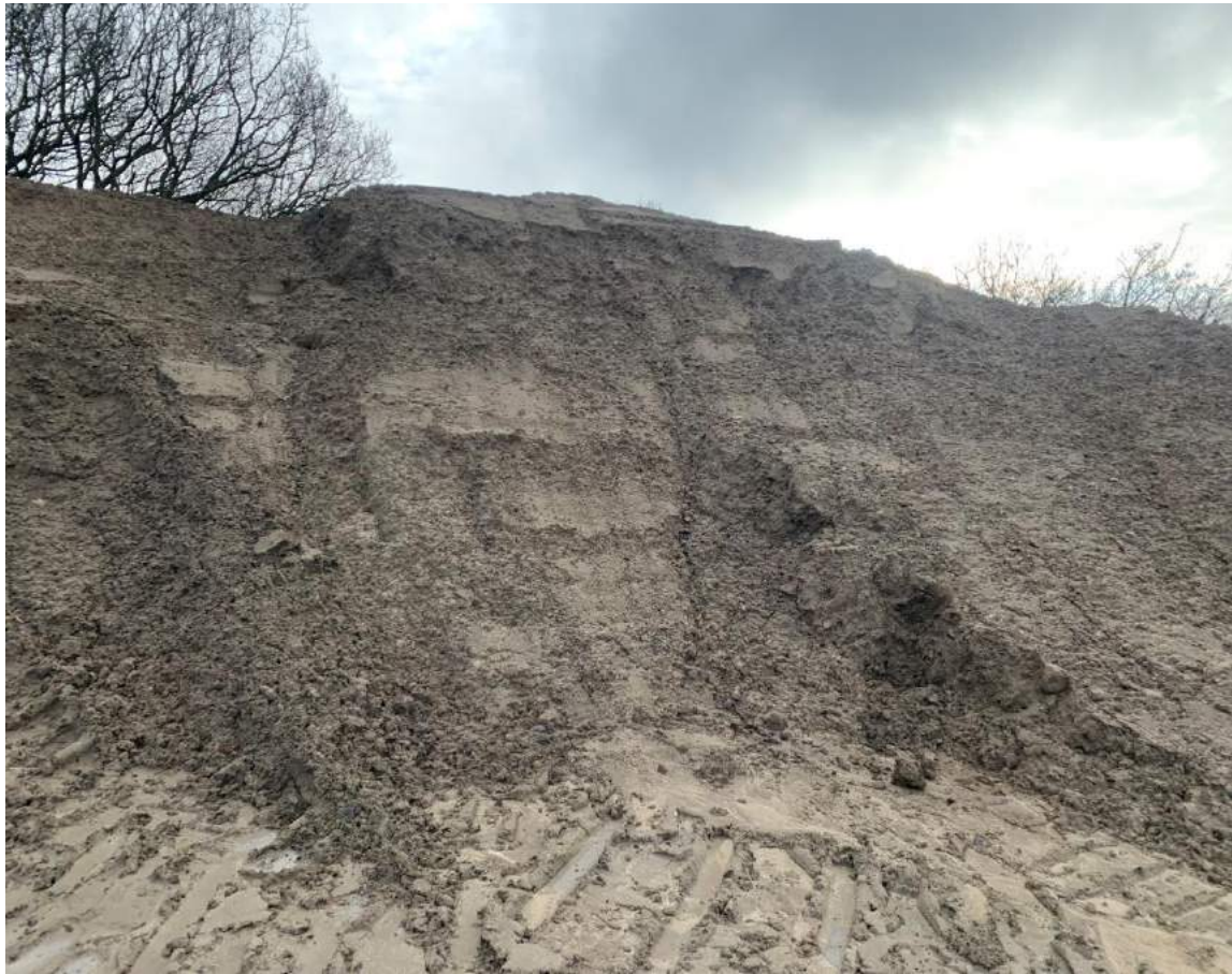
Plate 3 – Marchington Quarry, Glossop. NX Inspection 20 th March 2024
