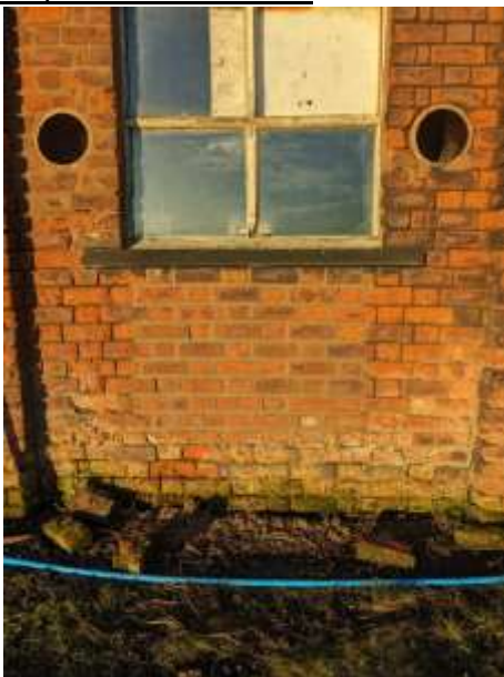
Image 03 – sample of facing brick/pointing
