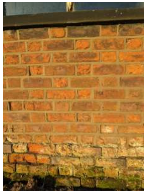
Image 04 – sample of facing brick/pointing
