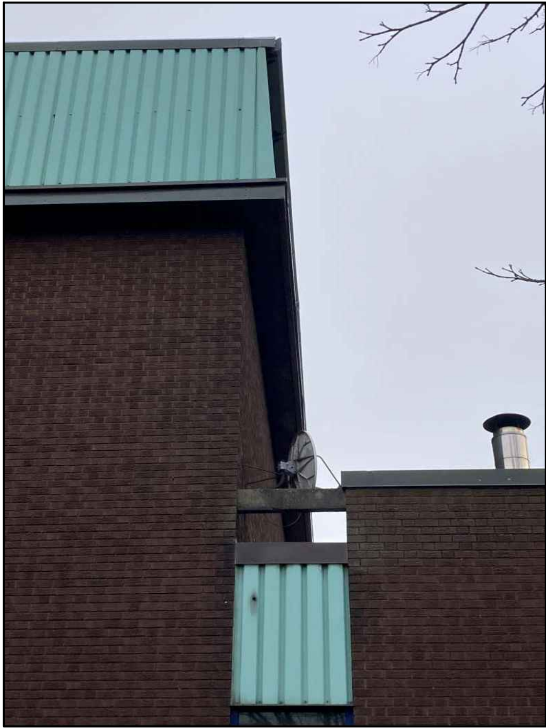
Photograph of Existing East Facing Elevation
