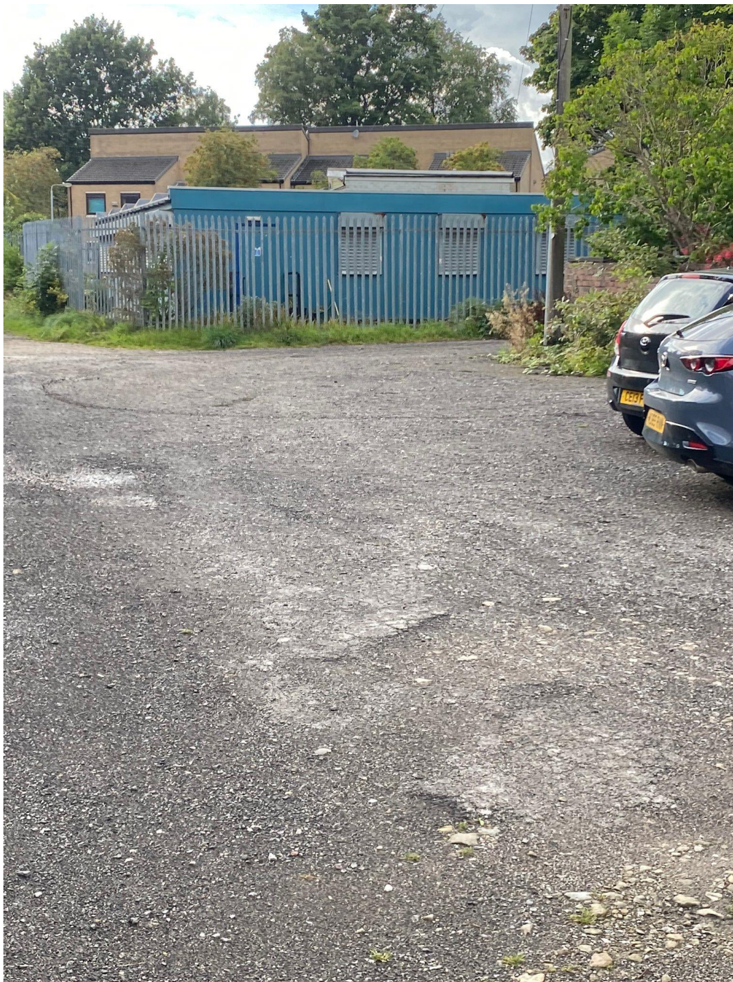
Figure 14: Spare parking capacity and turning space at the south end of Robin Lane (photo taken 4.30pm -5.30pm on 07.09.2022).
