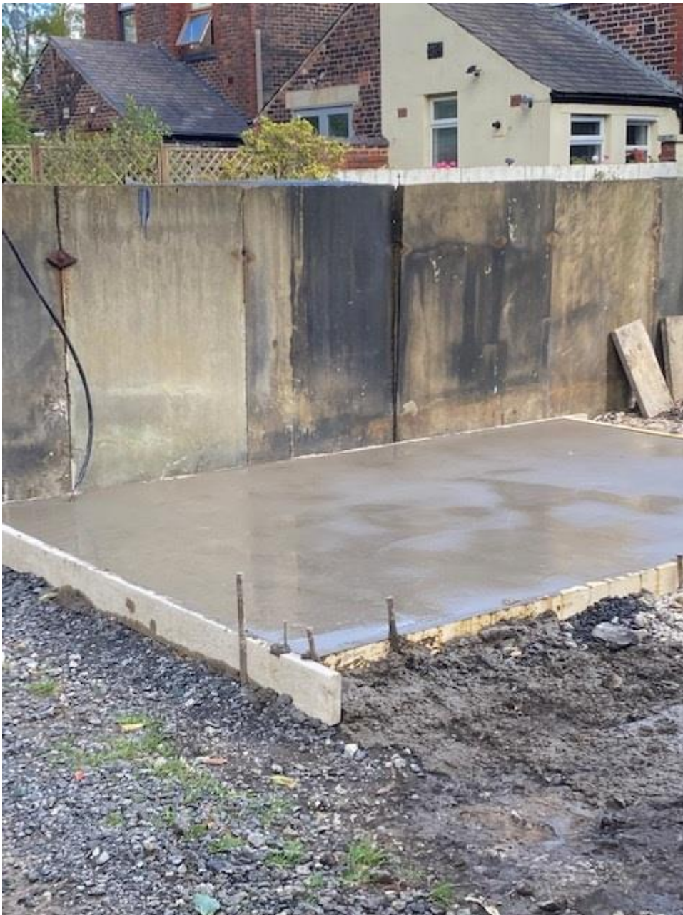
Figure 11: Concrete delivered by a 30tonne wagon which was able to access Robin Lane (photo taken 11.30am on 31.08.22).
