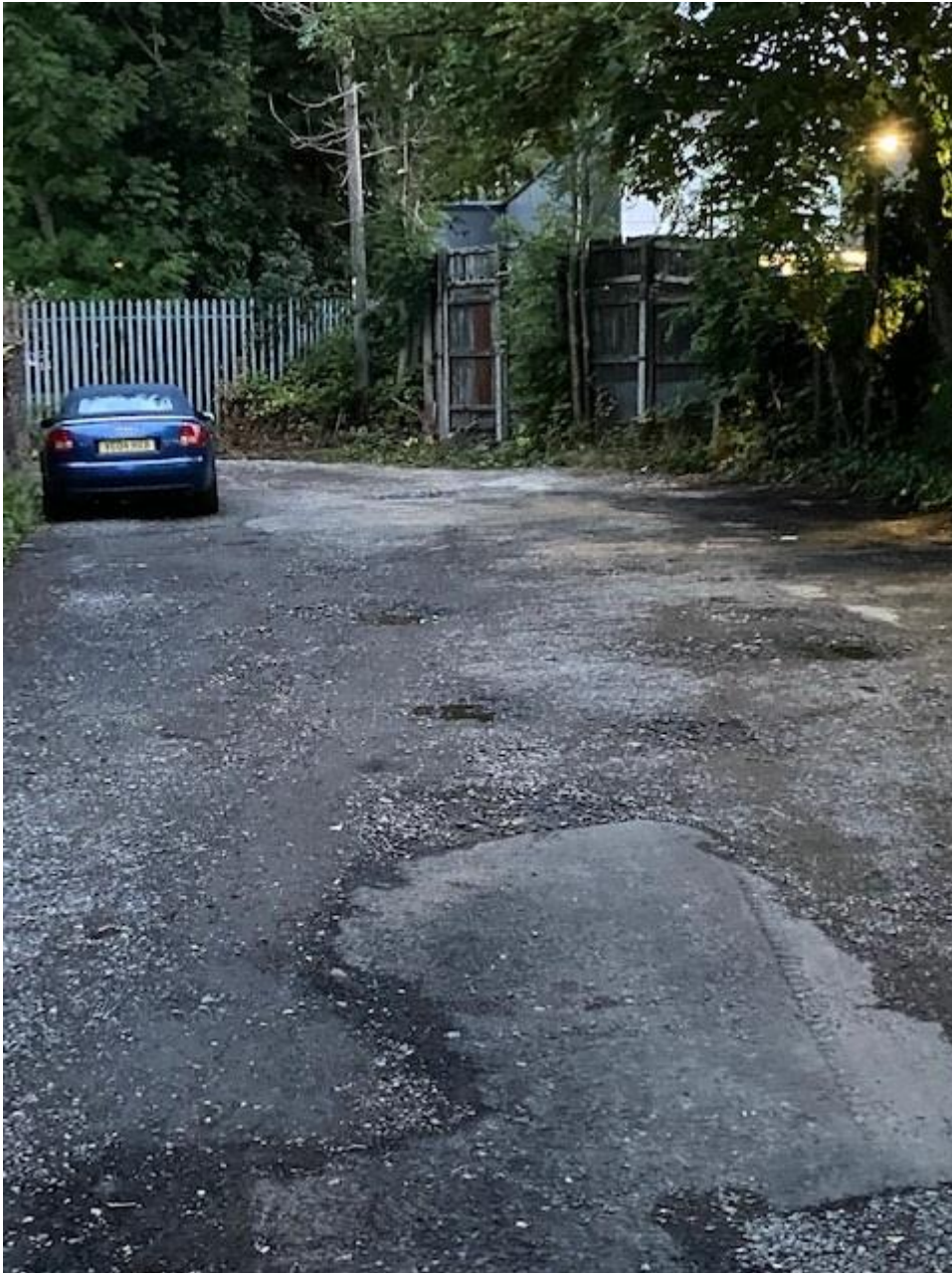
Figure 6: view showing the condition of the access road (photo 8.30pm on 23.08.22).
