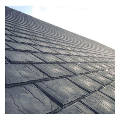
Roof - Slate Tiles
