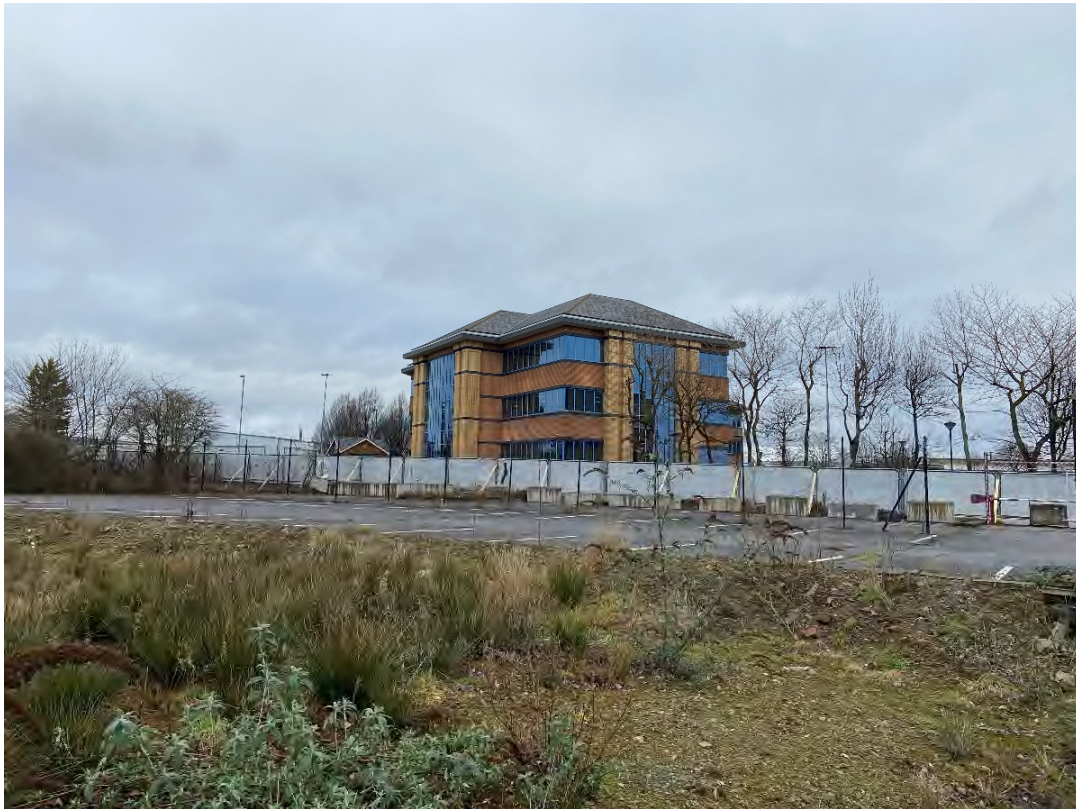
Photograph 3 – Tarmac area to the east of the site along with adjacent office block.
