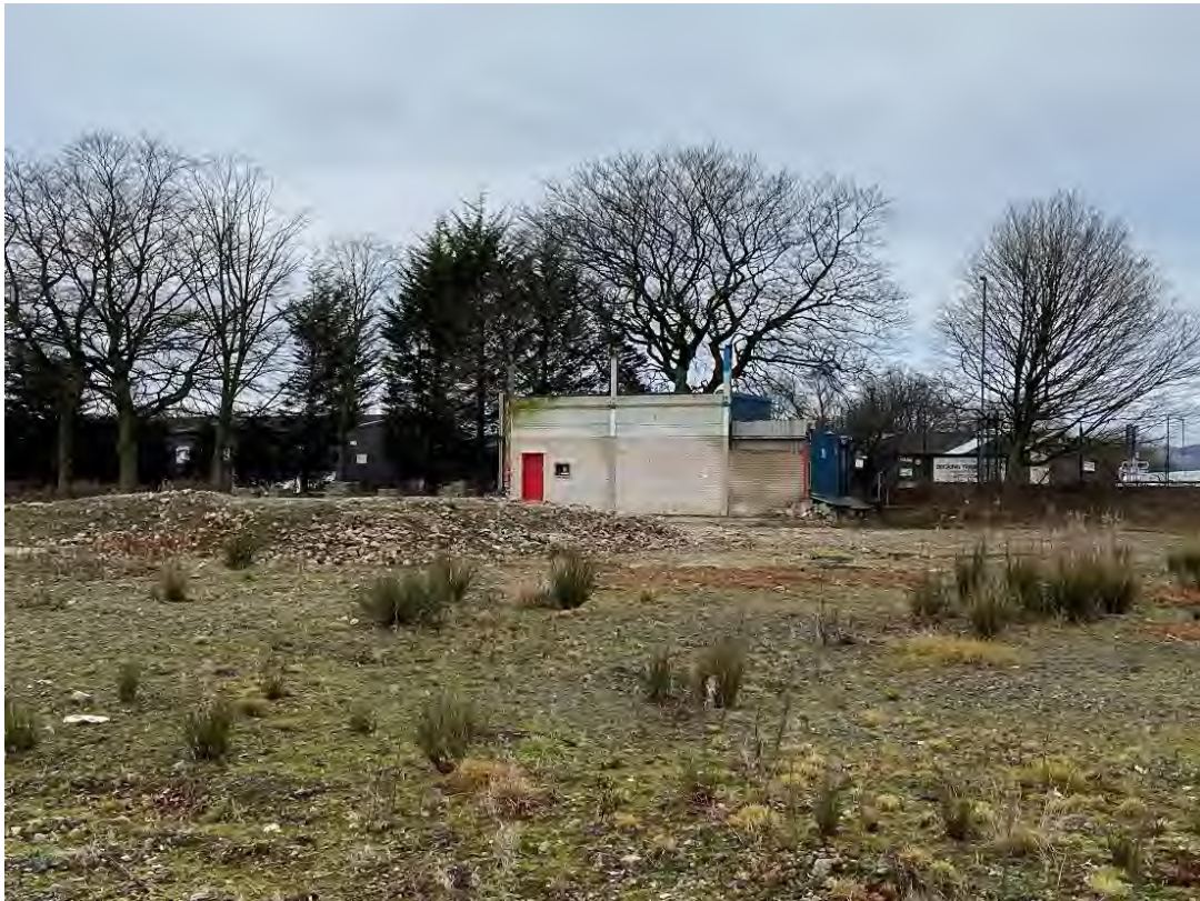
Photograph 5 – Existing building on site.
