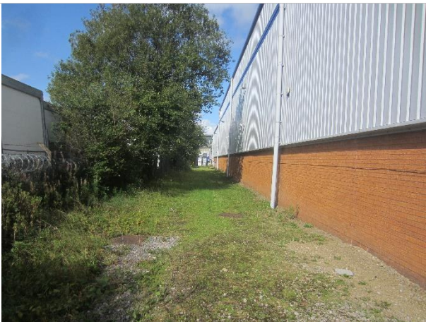
Photo 17: Western elevation of Gateway House
