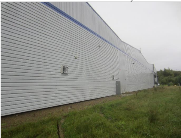
Photo 15: Southern elevation of Gateway House
