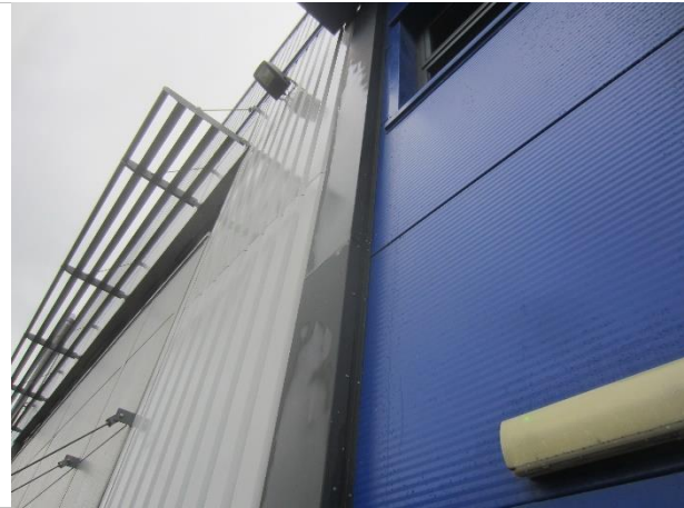
Photo 14: Southern elevation of Gateway House
