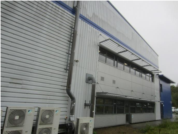
Photo 13: Southern elevation of Gateway House
