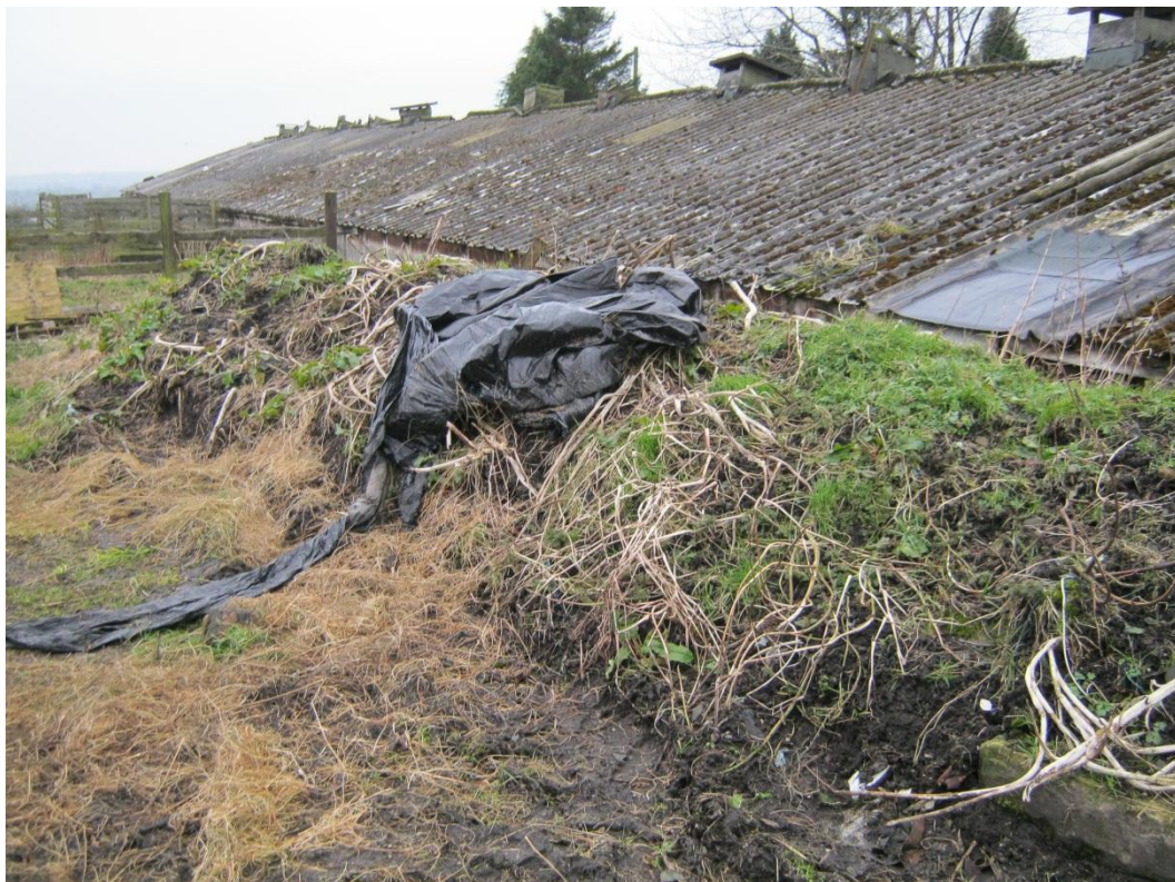
Photo 4: Stockpile of soil at the eastern edge of the barn.
