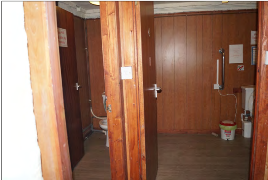
Plate 9. The modern WCs.
