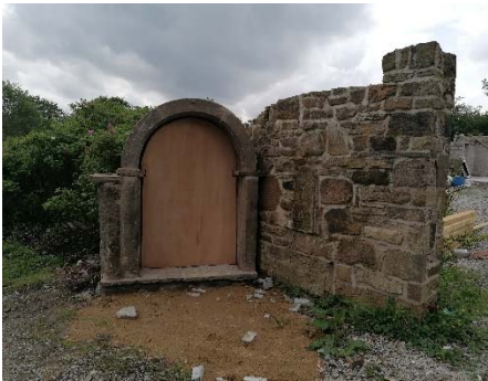
5. Pet Memorial under construction at the side of the main access track, next to the secondary entrance to Abbots Hall
