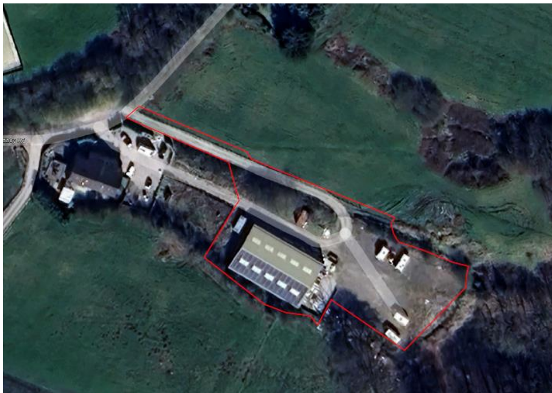
Figure 1.1: Abbots Hall, Woodhey Road, Holcombe Brook.
