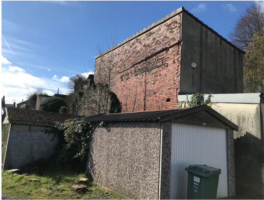
View to Rear of Existing Buildings from Existing Garage parking area
