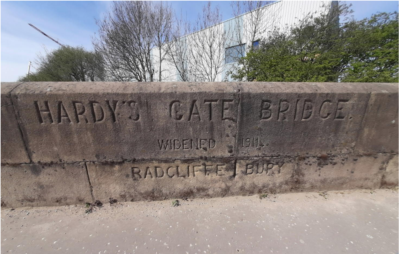
Photo 4.2: Inscription on the Bridge, commemorating the widening in 1911
