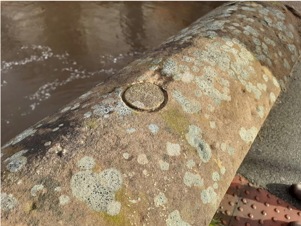
Photo 1.1: Example of reinstatement of historic fabric after insertion of steel dowels into the Bridge.
