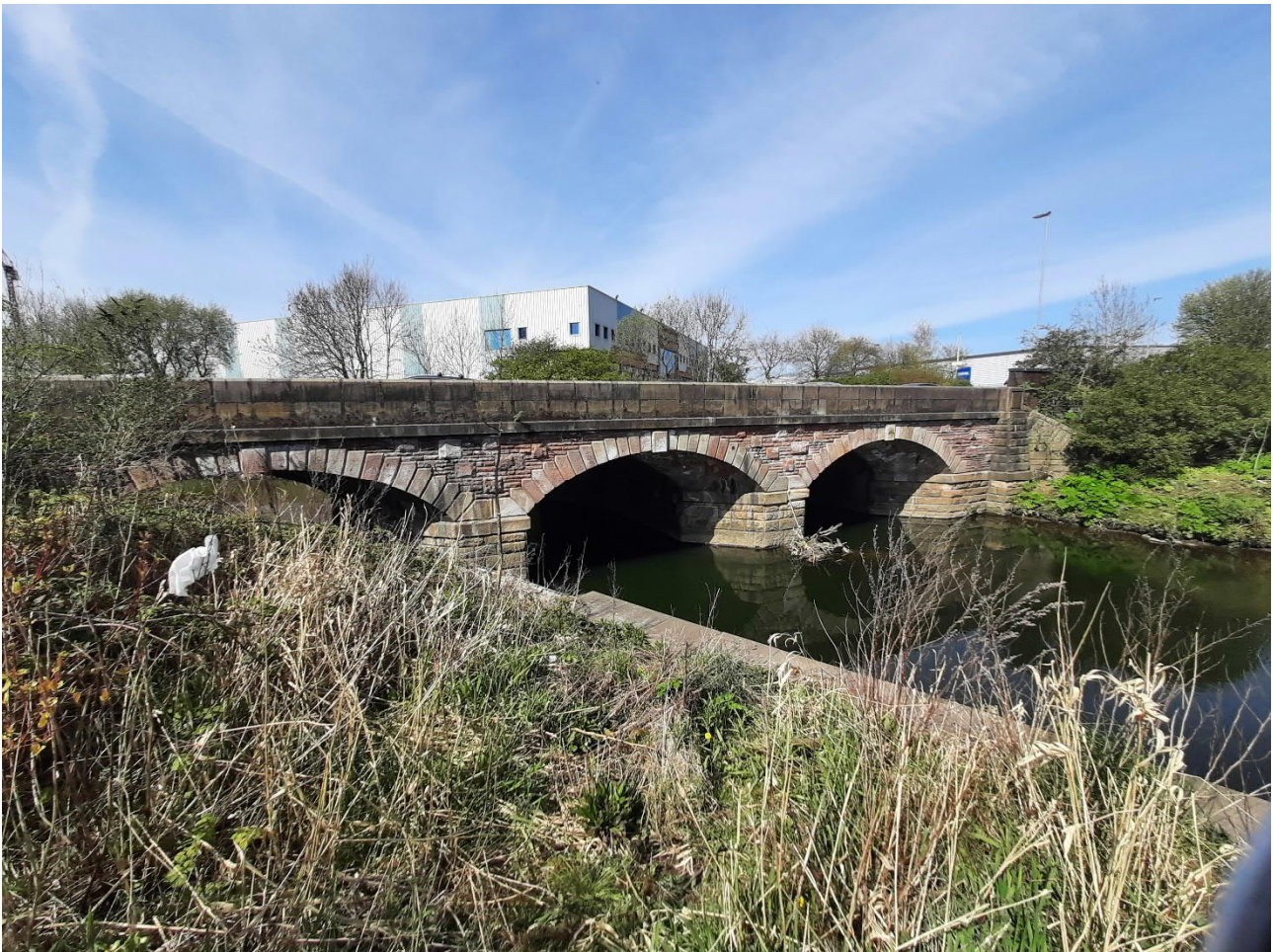
Photo 4.1: The Bridge - South, downstream, face built in 1911
