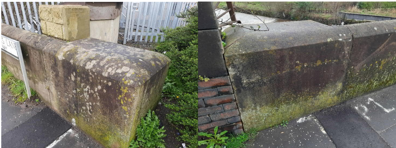
Photo 5.1: The western (left) and eastern (right) abutments which will be raised to install the swing gate fittings on new concrete tops
