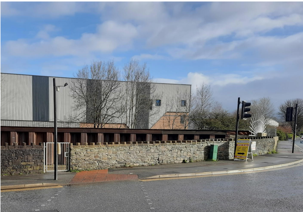
Photo 5.2: Existing masonry wall at the southern end of the bridge
