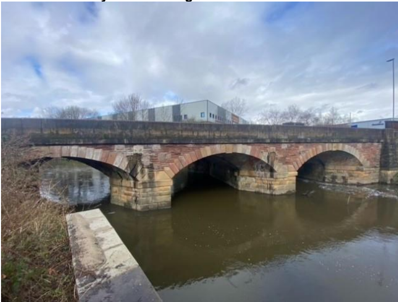
Photo 1.2: Hardy's Gate Bridge – Eastern Elevation
