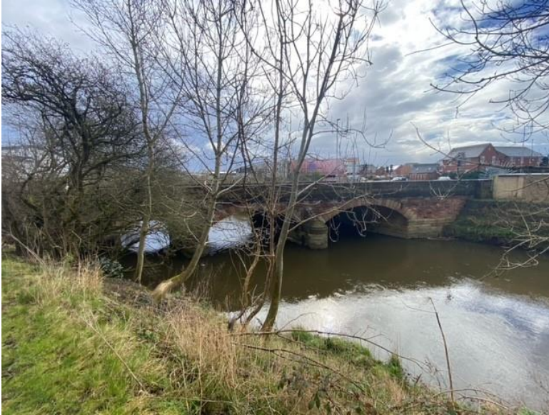
Photo 3.2: Hardy's Gate Bridge – Western Elevation
