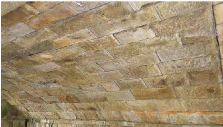
Photo 3.4: Underside of Hardy's Gate Bridge
