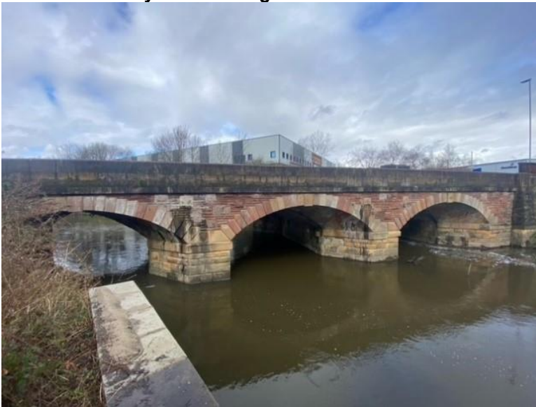
Photo 3.1: Hardy's Gate Bridge – Eastern Elevation
