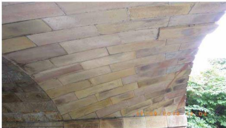
Phot 3.5: Underside of Hardy's Gate Bridge
