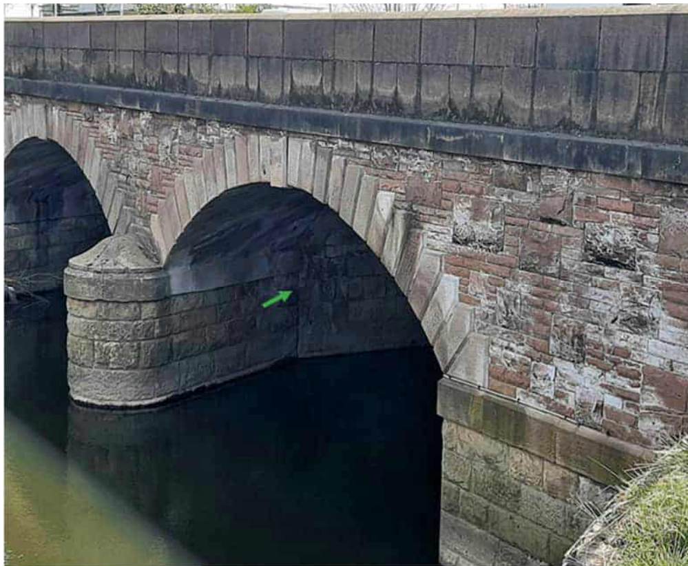
Photo 5.1: North-west, upstream elevation of Harvey's Gate Bridge looking north east. Arrow shows the joint between the original fabric and the widened structure of 1911.
