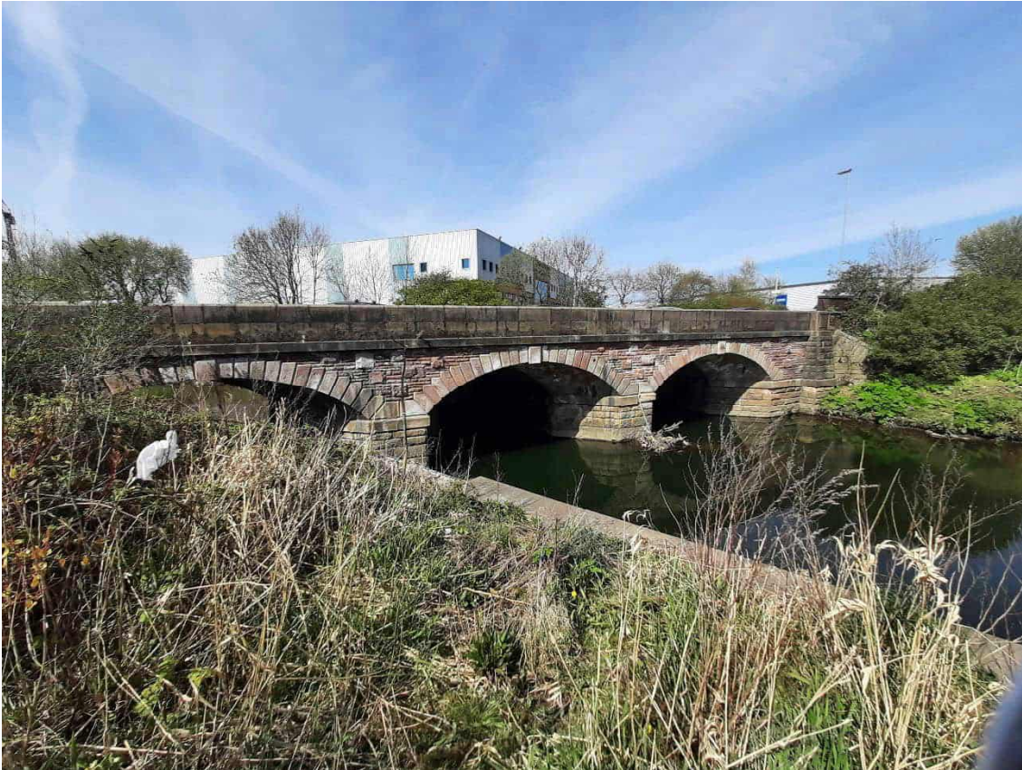
Photo 1.1: View of the Bridge, facing north-east.
