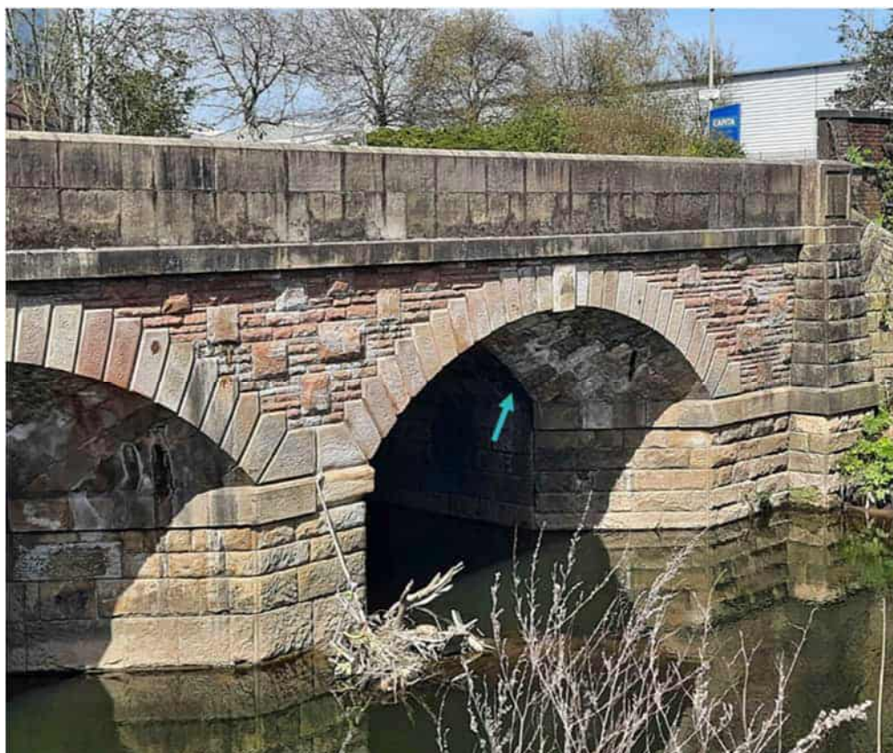
Photo 5.2: South-east, downstream face of Harvey's Gate Bridge looking north-west. Arrow shows joint between the original fabric and the widened structure of 1911.
