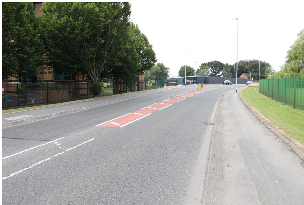
3A-3B Pilsworth Road
