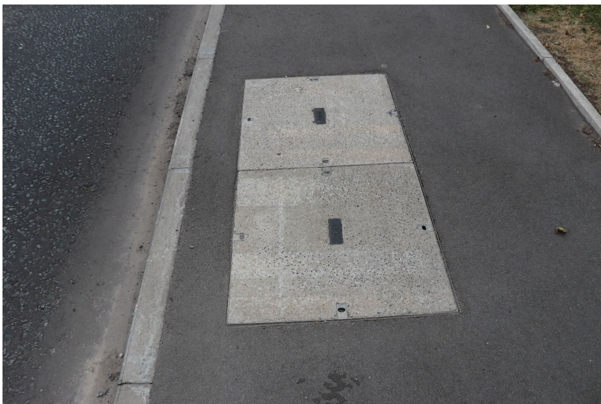
2A-2B Pilsworth Road
