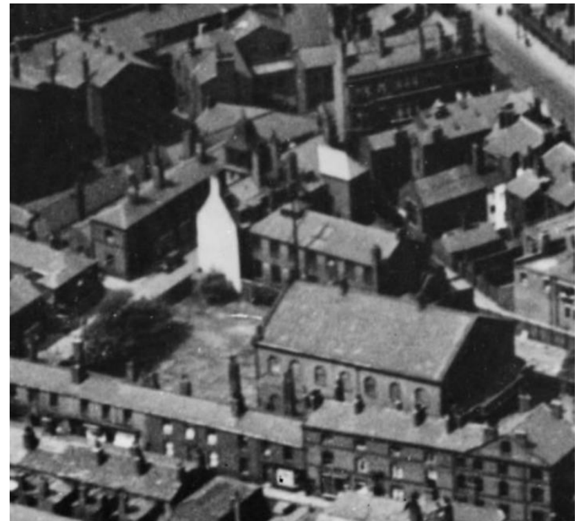
Image 8 - Archive aerial image of the former Post Office (1927), with its white end gable visible, and the Union Street Wesleyan Chapel with its burial ground (subject site).
