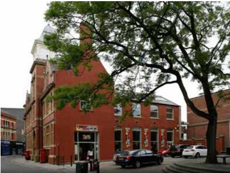
Image 10 - Photograph of the former Post Office building dating from its time in use as a nursery.
