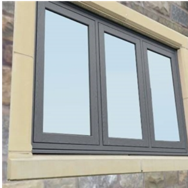
PROPOSED GREY FRAMES, DOOR, SOFFITS & SANDSTONE SURROUNDS
