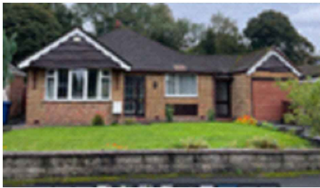
PHOTO WEST ELEVATION
