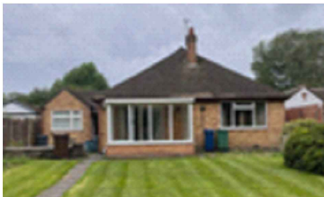
PHOTO EAST ELEVATION
