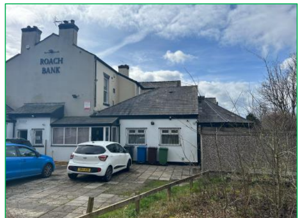
The northeast elevation of the building
