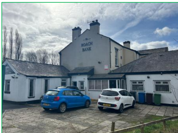
The northeast elevation of the building
