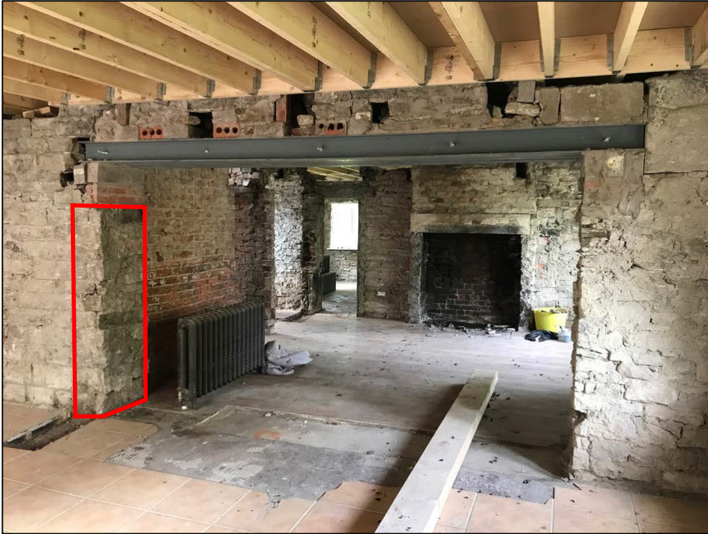
5.8 Proposed exposed stone section (3) to remain visible within former external wall of c. 1739.
