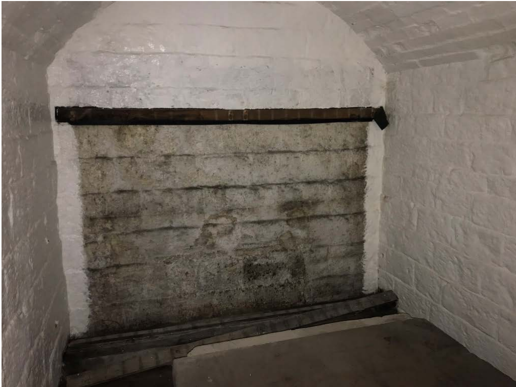
5.14 Partially historic stonework within lower sections of cellar walls.
