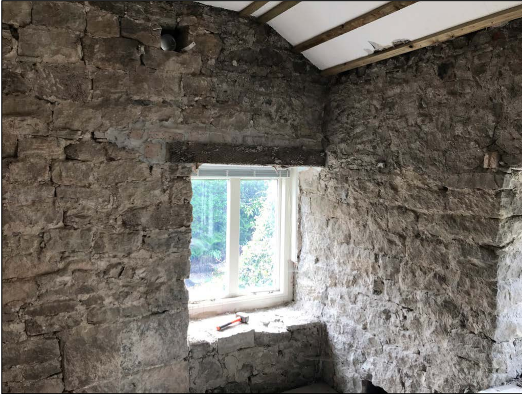
5.10 Natural stone faces of external walls generally dry with no major water ingress above ground.
