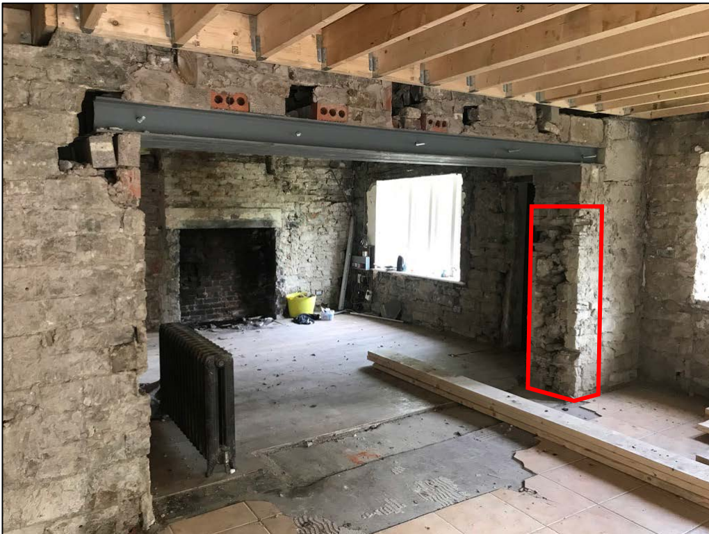
5.9 Proposed exposed stone section (4) to remain visible within former external wall of c. 1739.
