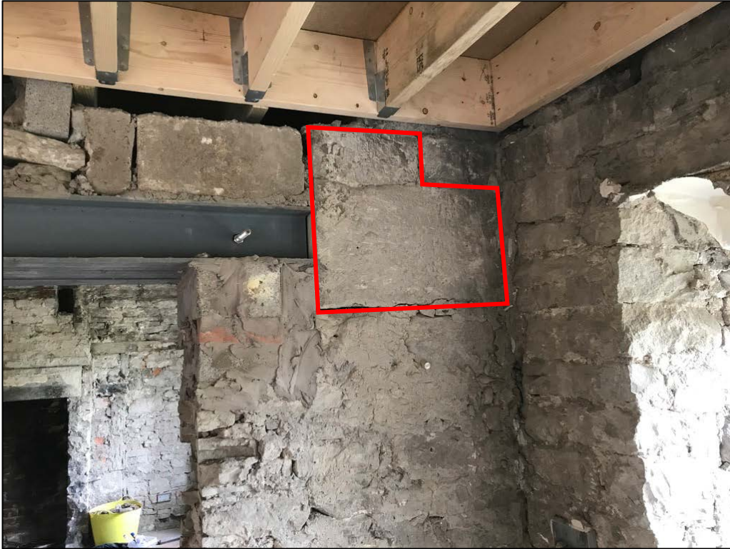
5.6 Proposed exposed stone section (1) to remain visible within former external wall of c. 1739.
