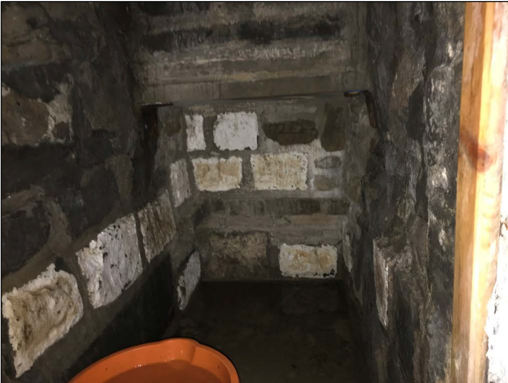
5.15 Modern niche within cellar.
