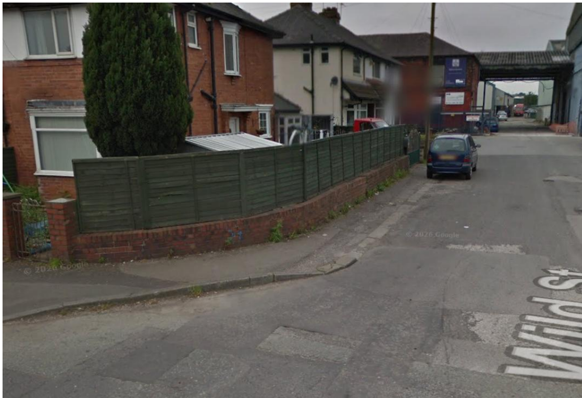
Fig 4: Southern edge of Wild Street with demarked pedestrian route but now kerb upstand to differentiate for vehicles
