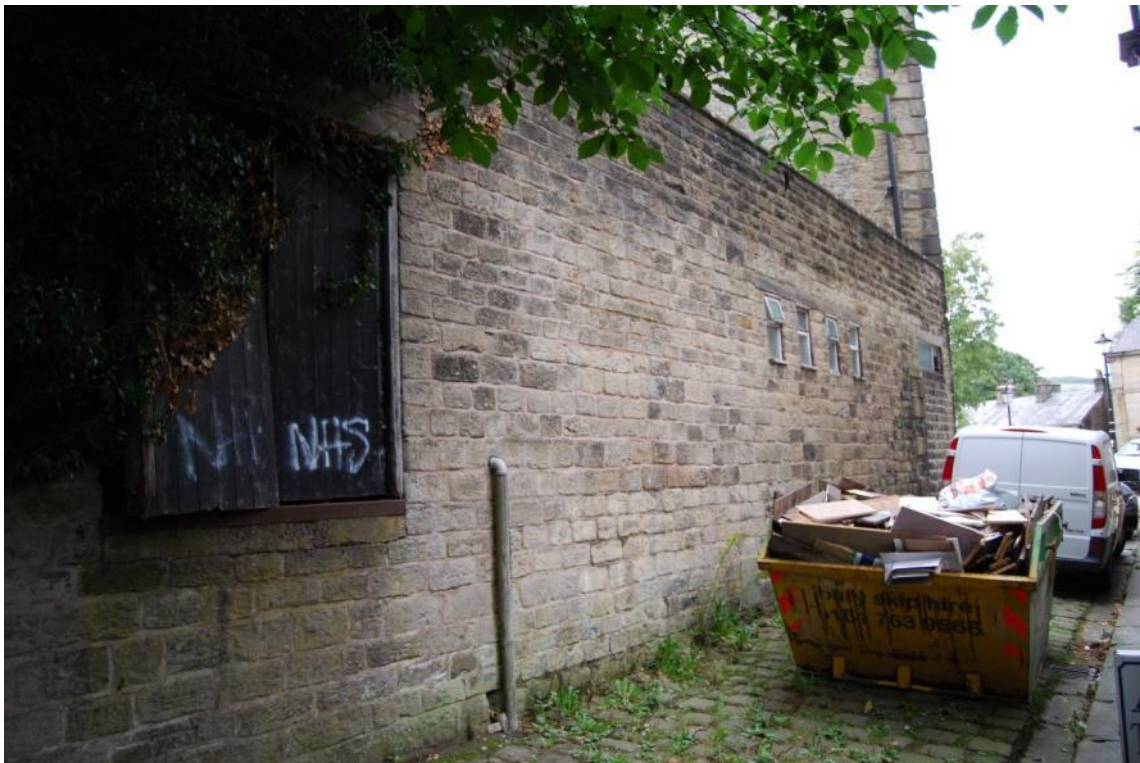
Figure 13. Elevation from Back Carr Street forming the side wall of the existing WCs.
