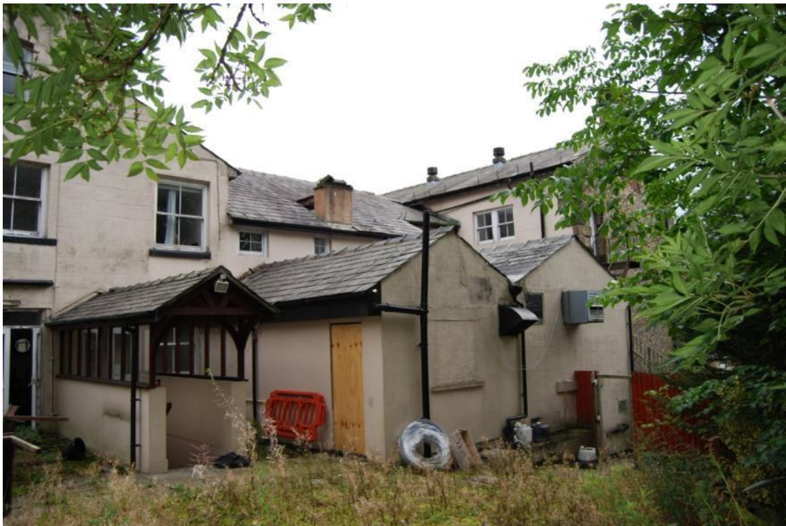
Figure 7. Elevation from the garden (from north west). This illustrates the later additions of the single storey extension with dual pitched roof enclosing the existing kitchen.
