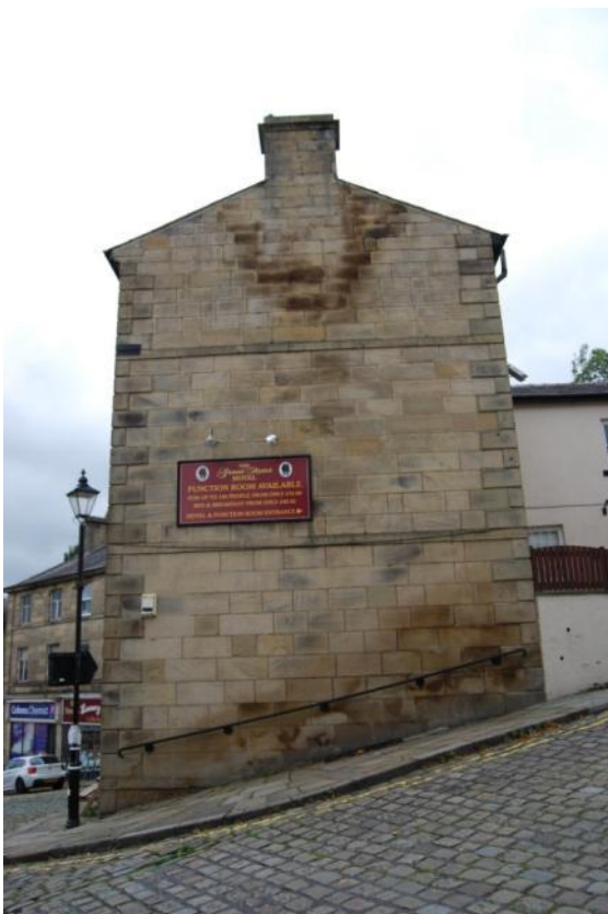
Figure 3. East gable formed with ashlar masonry.
