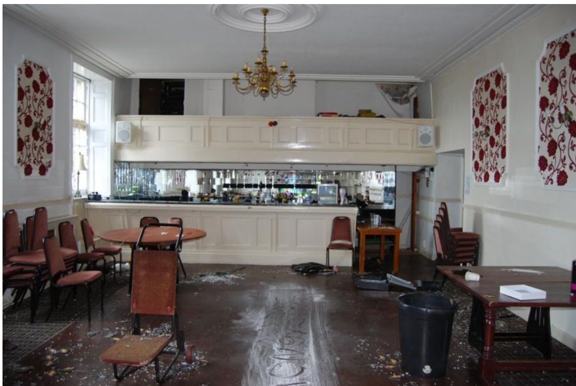
Figure 23. Upper ground floor function room (looking from the east). Decorative cornices and ceiling roses.
