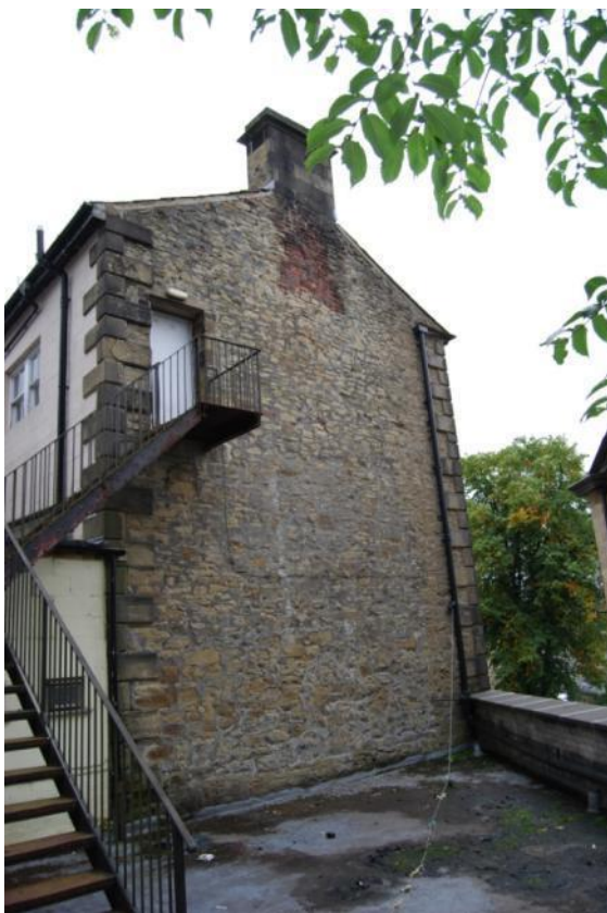
Figure 11. View of frontage building gable from the west, built in random rubble. Note brick infill below chimney.
