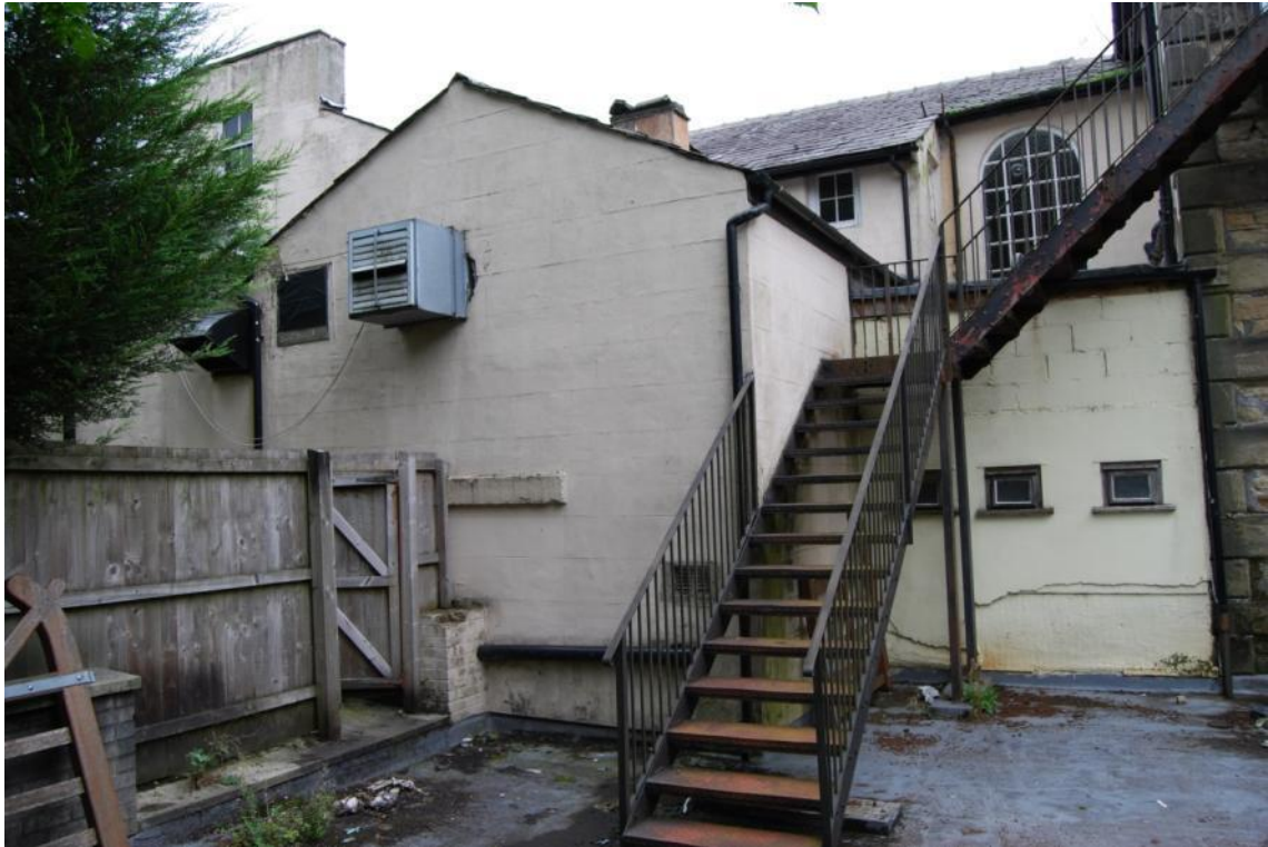
Figure 10. View of later extensions from the west including the steel fire escape from the upper floor of the frontage building.
