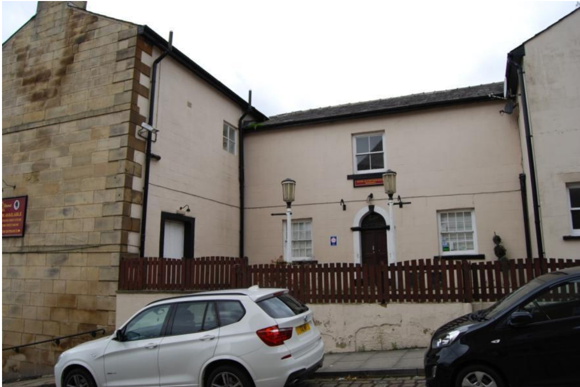
Figure 4. Elevation from the east indicating the rear extension with render finish.
