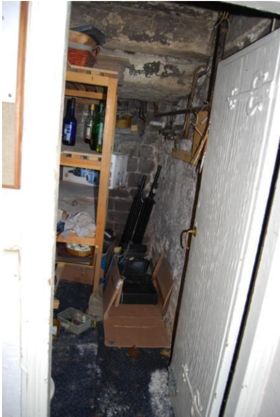
Figure 20. Lower ground floor understairs store.
