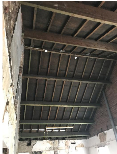
Replacement roof constructions
