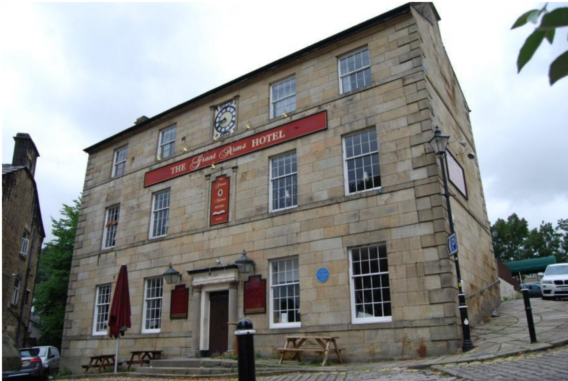
Figure 2. Frontage and gable from the south east. Imposing frontage, fine ashlar detailing.
