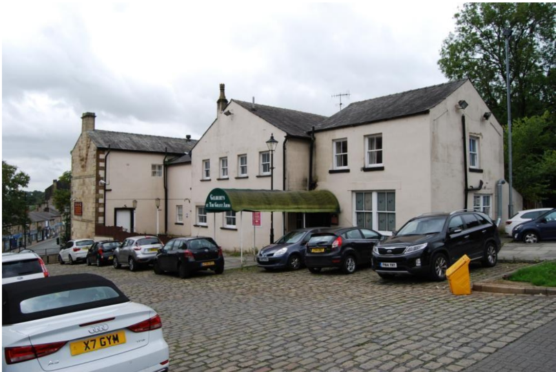
Figure 5. Elevation from north east (for context reasons).
