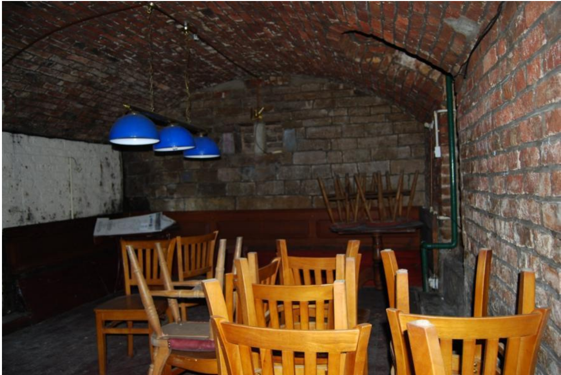
Figure 22. Lower ground floor cellar 2. Combination of stone and brick walls with brick barrel vaulted ceiling.
