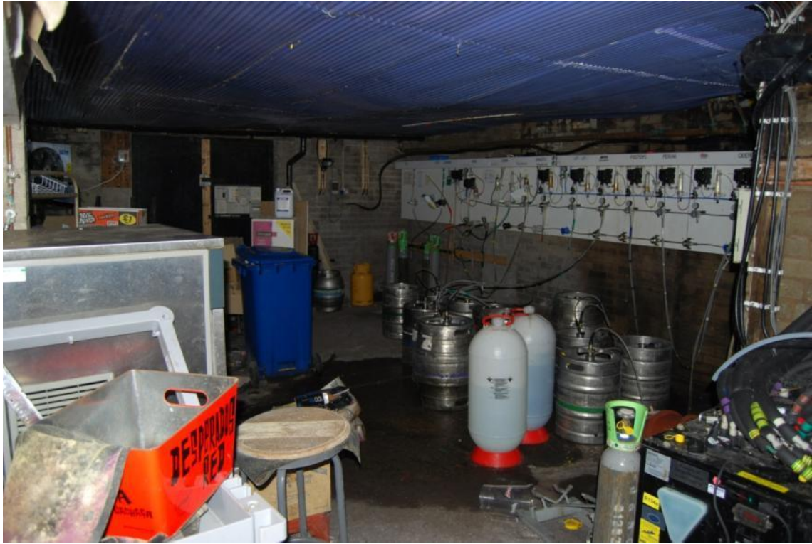
Figure 16. Lower ground floor beer cellar.
