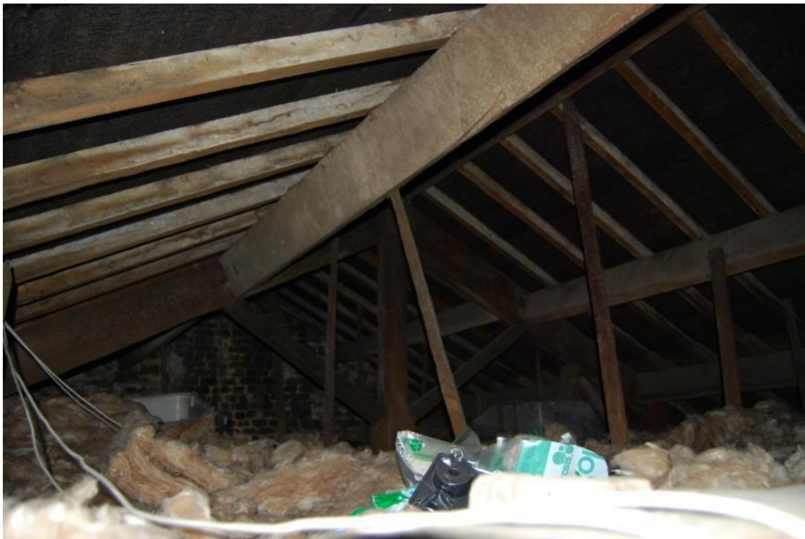
Figure 36. Roof over frontage building illustrating king post trusses, purlins and rafter construction with hangers supporting binders and ceiling joists.
