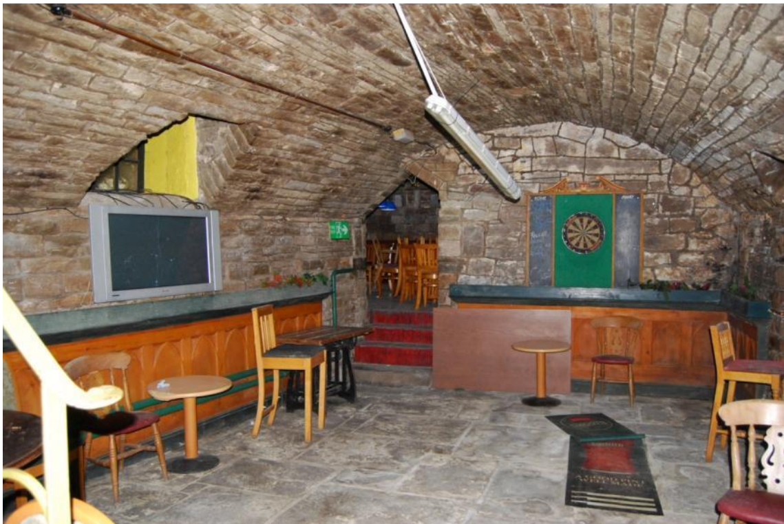
Figure 21. Lower ground floor cellar 1. Flag floor with stone barrel vaulted ceiling.
