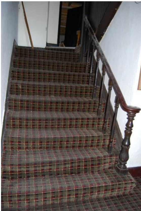
Figure 19. Lower ground floor carpeted stone stair.
