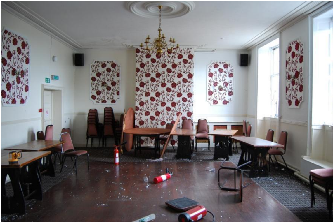
Figure 24. Upper ground floor function room (looking from the west). Note bench seating to alcove of windows and dado panelling. Decorative cornices and ceiling roses.
