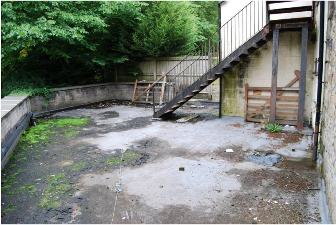
Figure 12. Flat roof over the later 1970s (assumed) extensions with parapet wall.
