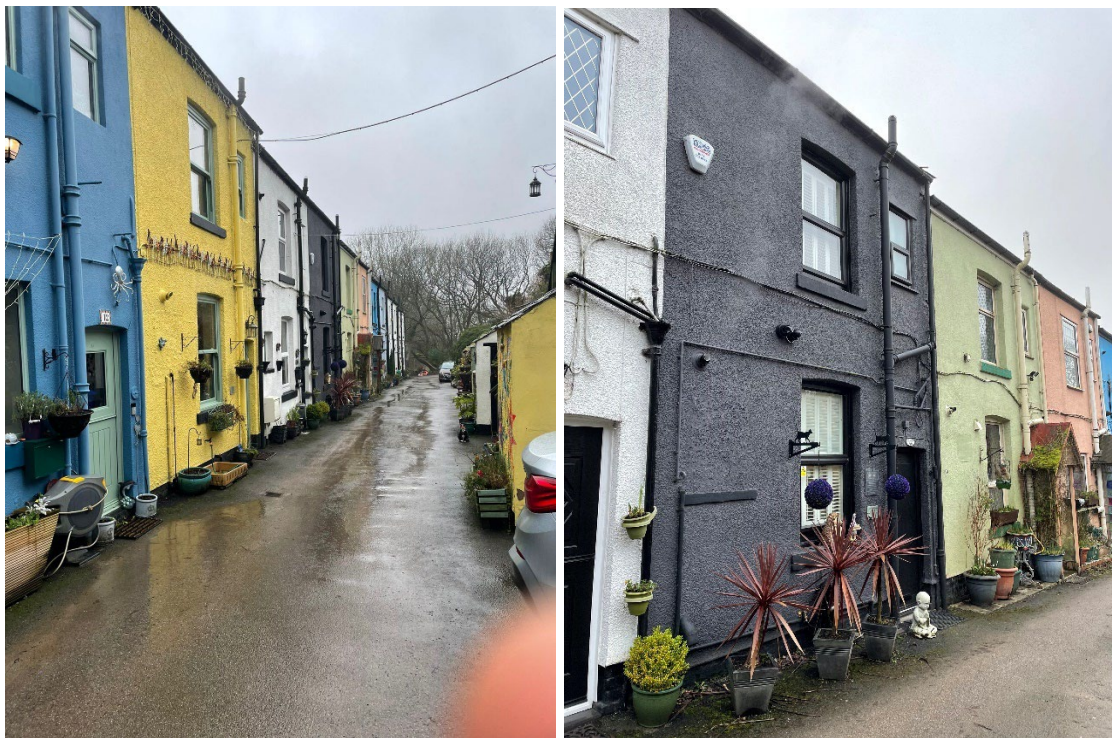
Figure 4 – Photographs showing the frontage of the terraced properties on Broad Oak Terrace and No.9 painted dark grey in colour
