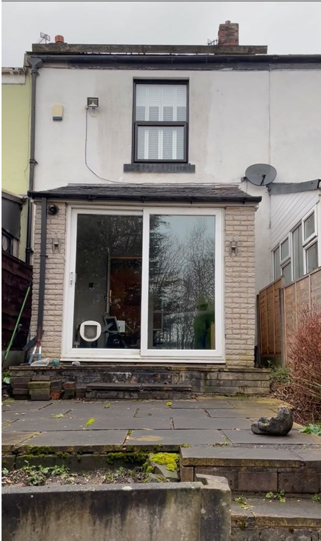
(Figure 5 – Photograph showing rear elevation of the property including the existing single storey extension and garden patio area that are in situ)
