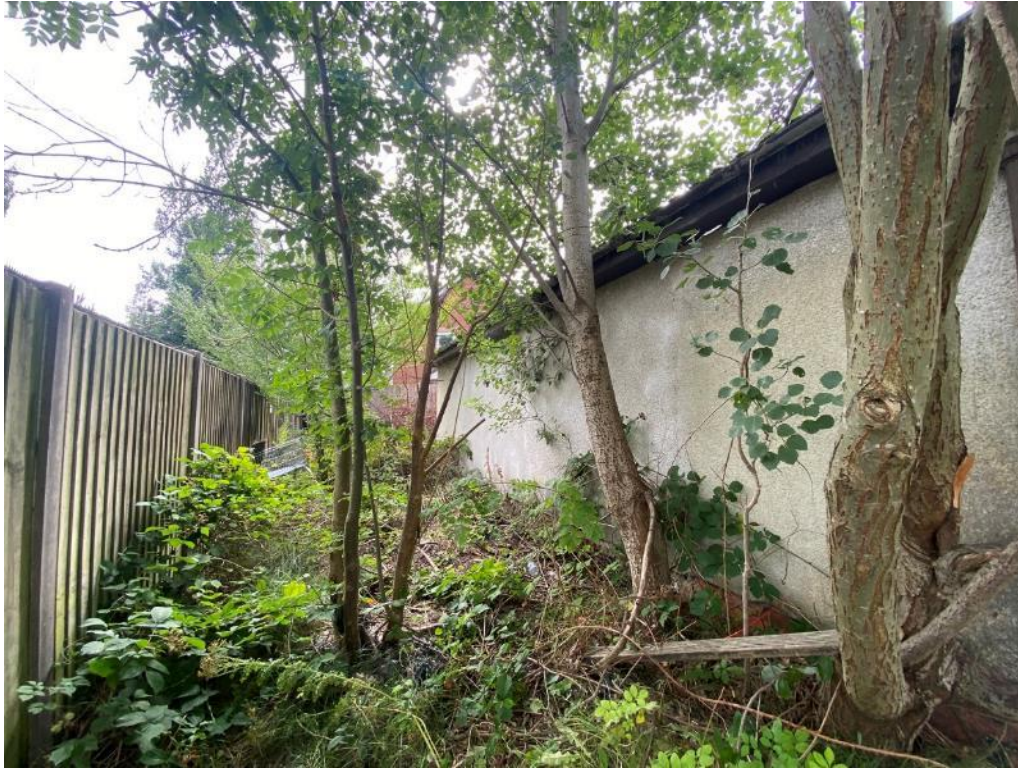
Plate 16: Character of the eastern elevation of the building.
