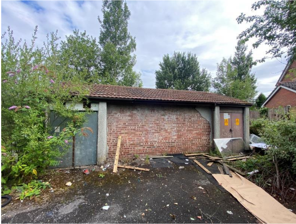
Plate 14: Character of the south-eastern elevation of the building.
