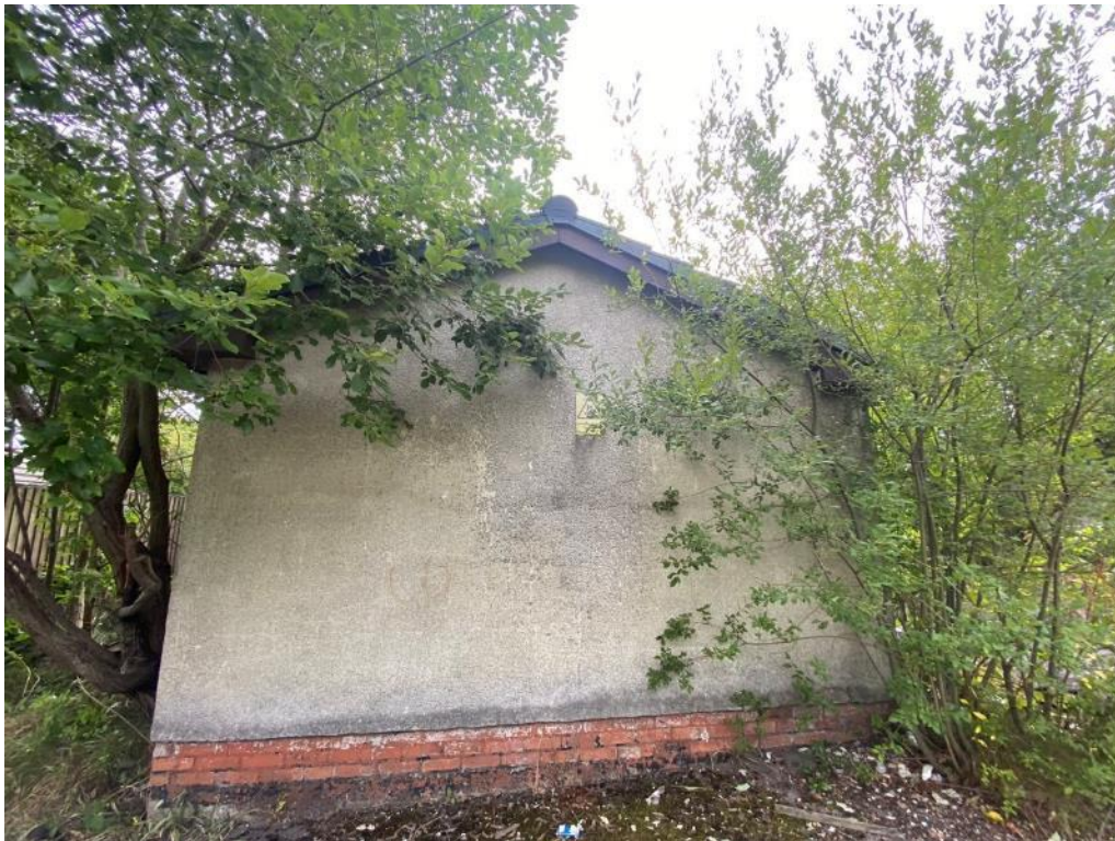
Plate 15: Character of the northern elevation of the building.
