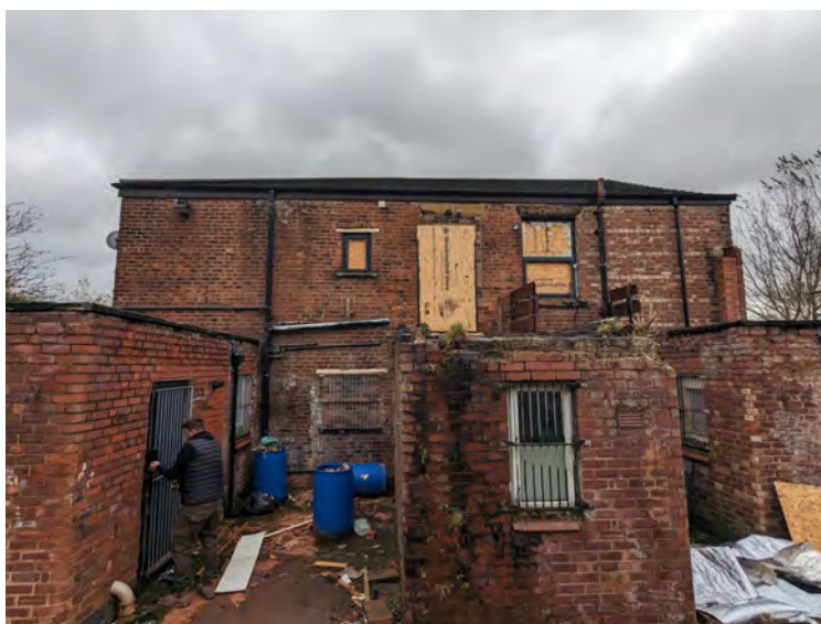
Photo showing the northern elevation of B1
