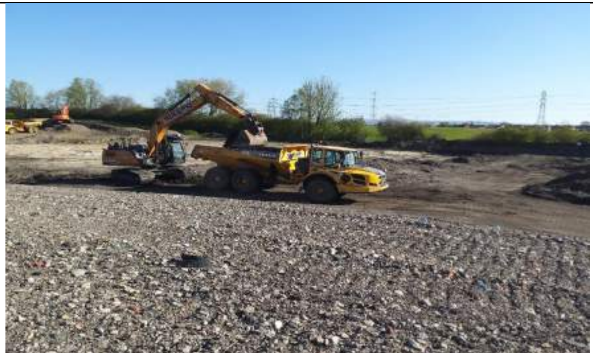
Photograph 4: Excavation of dark landfill Made Ground in the north.
