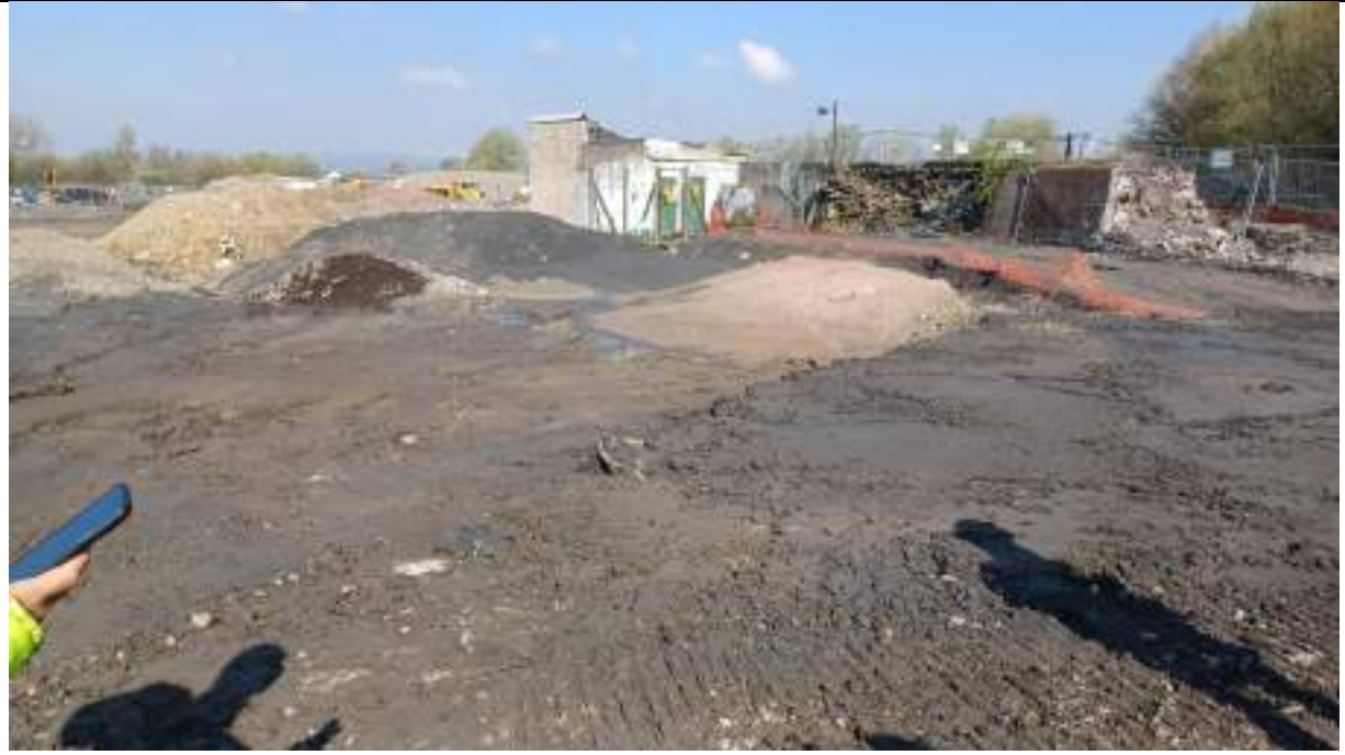
Photograph 1: Location of Shaft 006. Surplus pfa and sand still present at the site
