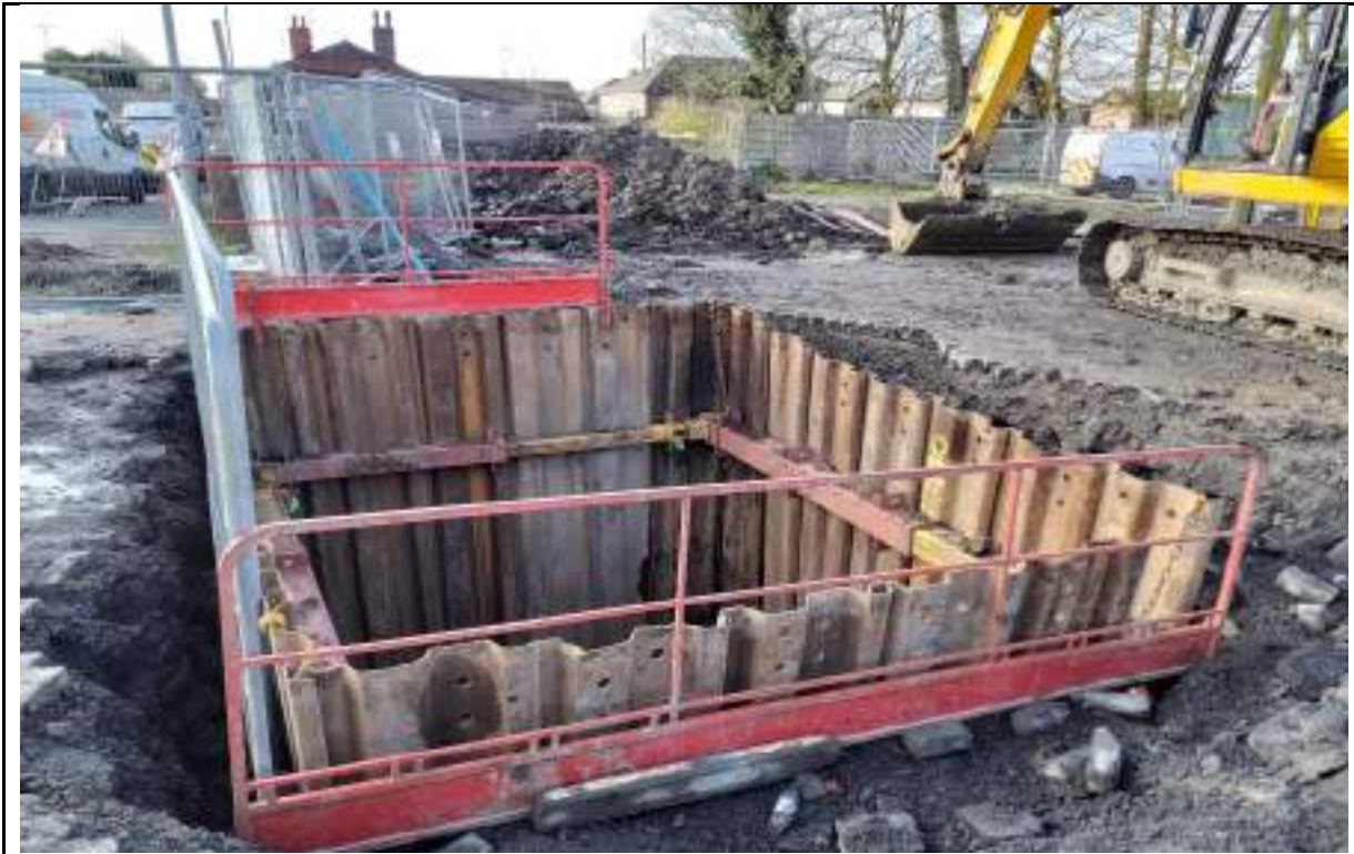
Photograph 1: Excavation and installation of sheet piles for drainage in the southeast.
