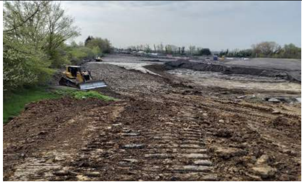
Photograph 9: Placed fill in the east using excavated dark landfill Made Ground from the centre north.
