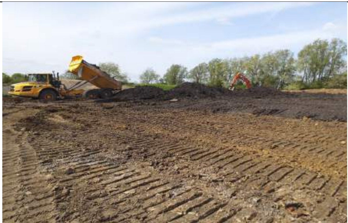
Photograph 6: Backfilling borrow pit using peat material from peat stockpile in the northwest.
