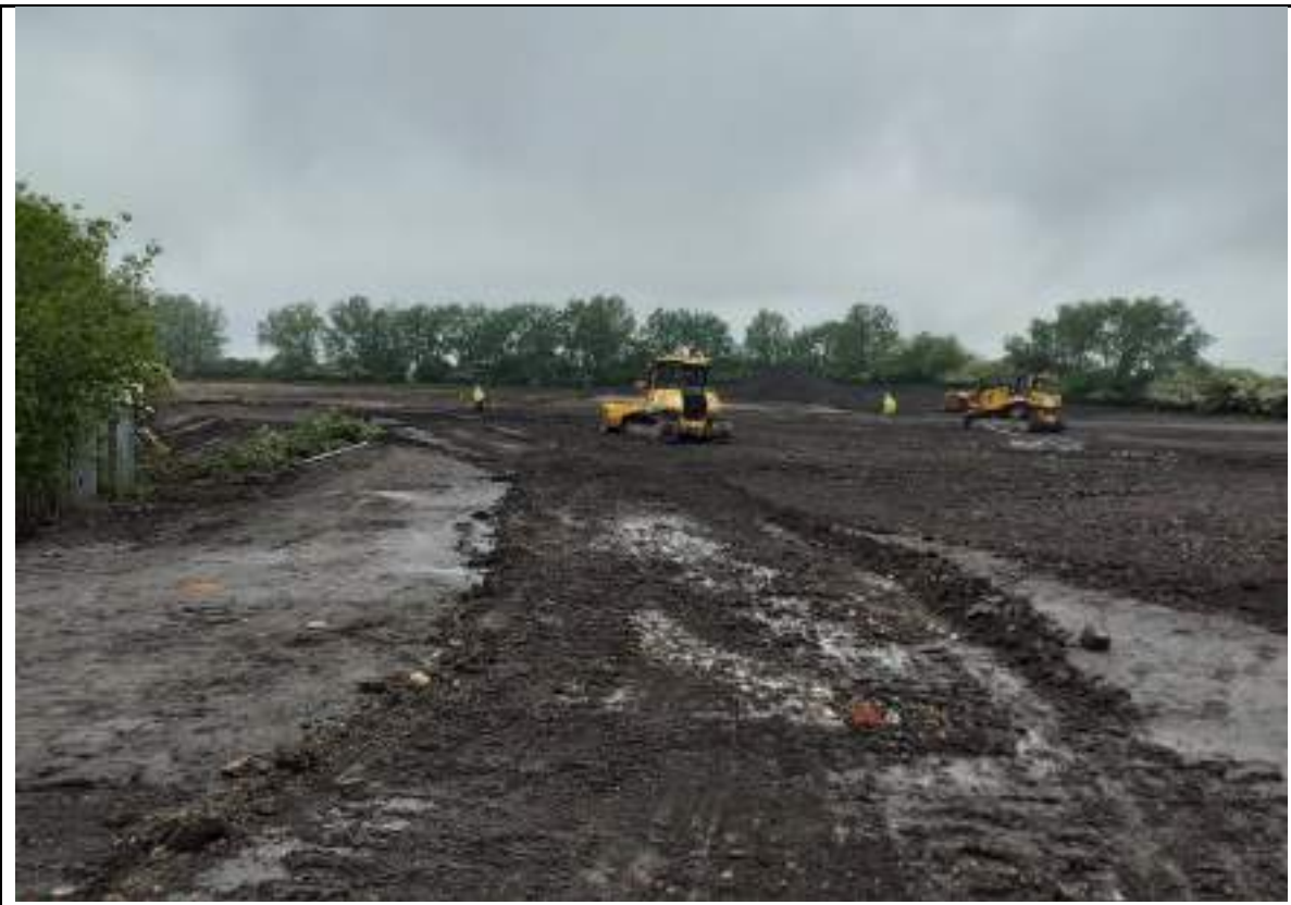
Photograph 6: Trimming place fill in the northwest. Surveyor is checking levels.
