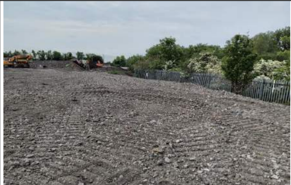
Photograph 11: Capping layer in the western boundary of the site. Looking towards the south.
