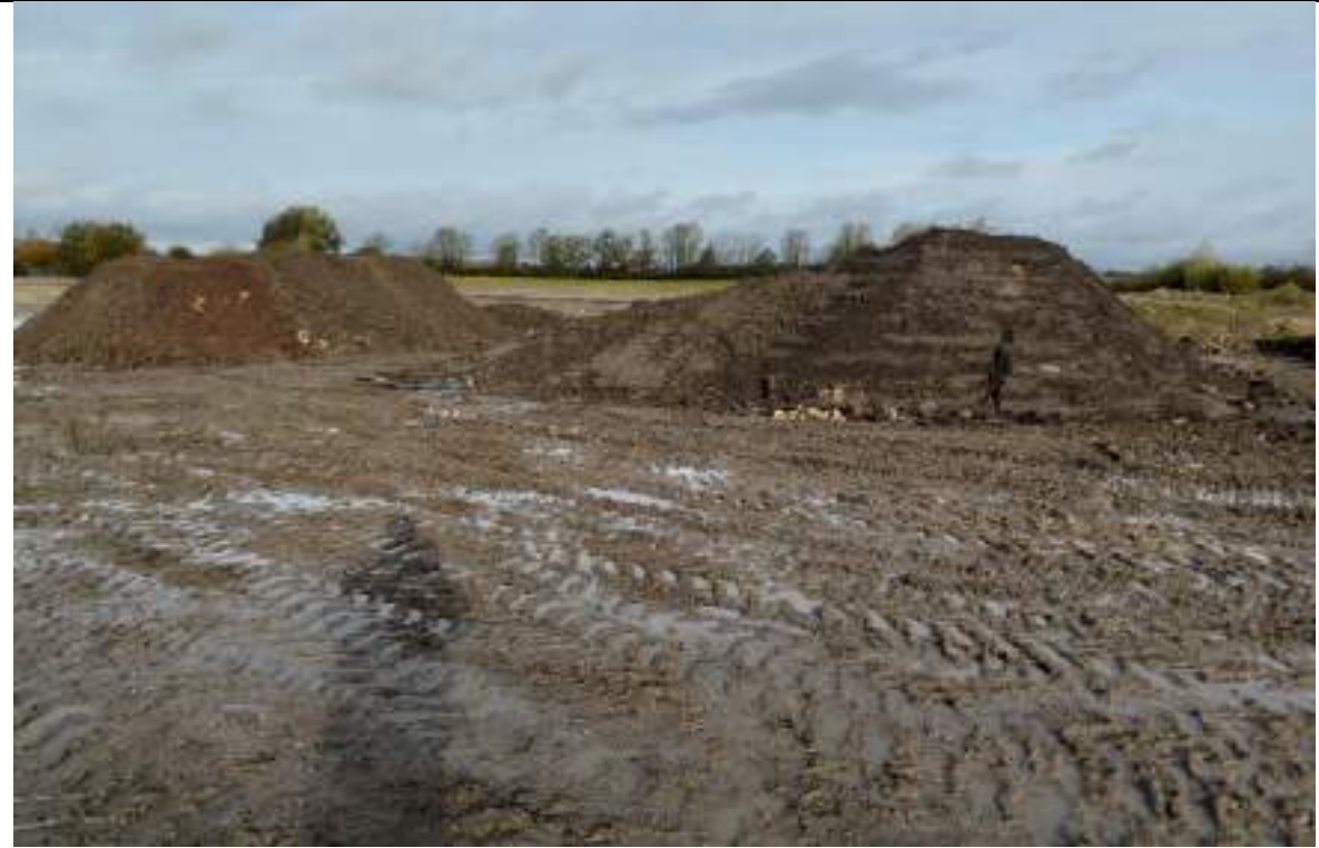
Photograph 3: Stockpile of potentially TPH contaminated material on a black visqueen barrier adjacent to electrical substation and wet material stockpile. Material excavated from location of shaft no.7.
