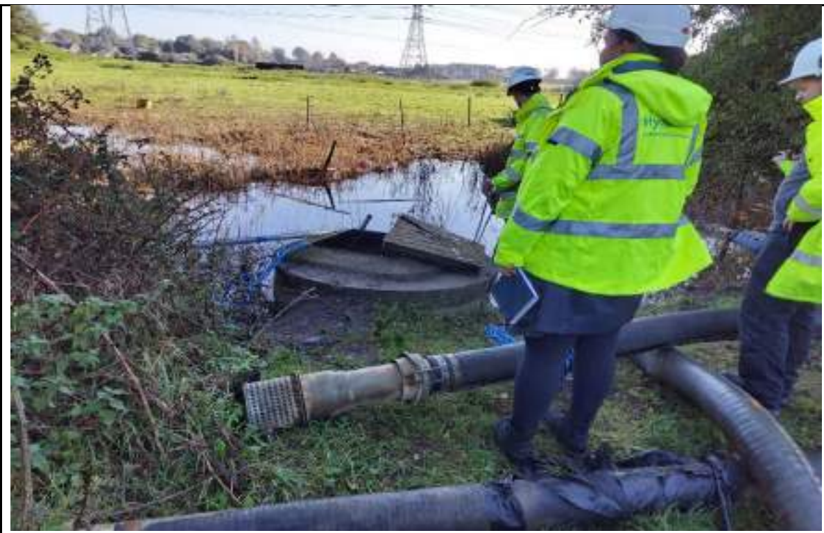
Photograph 6: Manhole of the culvert and pumping equipment in the west outside boundary of the site.
