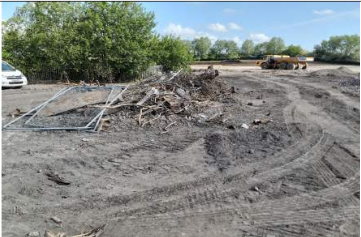
Photograph 124: Stockpile of deleterious material in the northwest.
