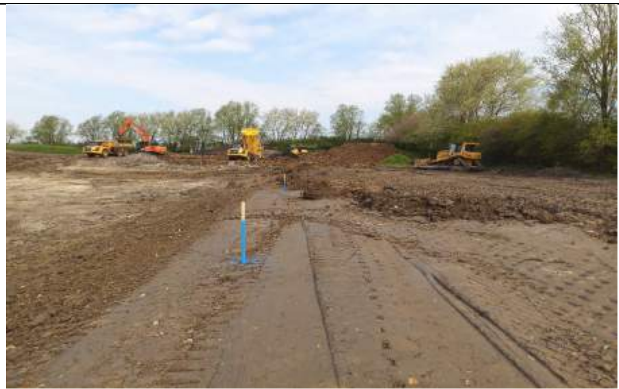
Photograph 10: Stockpile of excavated material from borrow pit in the northeast.
