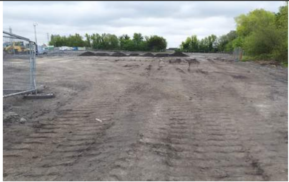
Photograph 11: Final layer of fill placed and proof rolled in the west.
