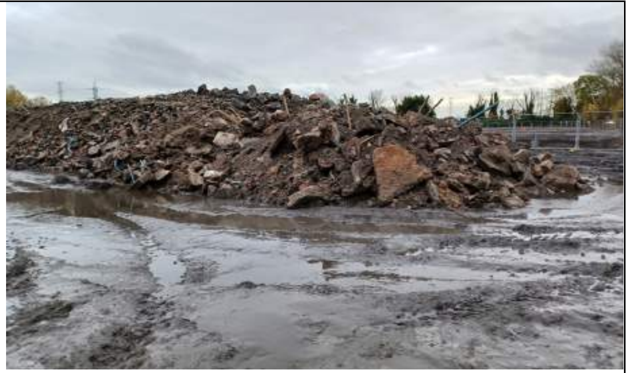
Photograph 9: Oversize material to be crushed and processed
