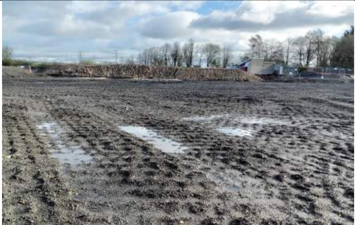
Photograph 13: Stockpile of brown glacial clay in the east. Source testing outstanding.
