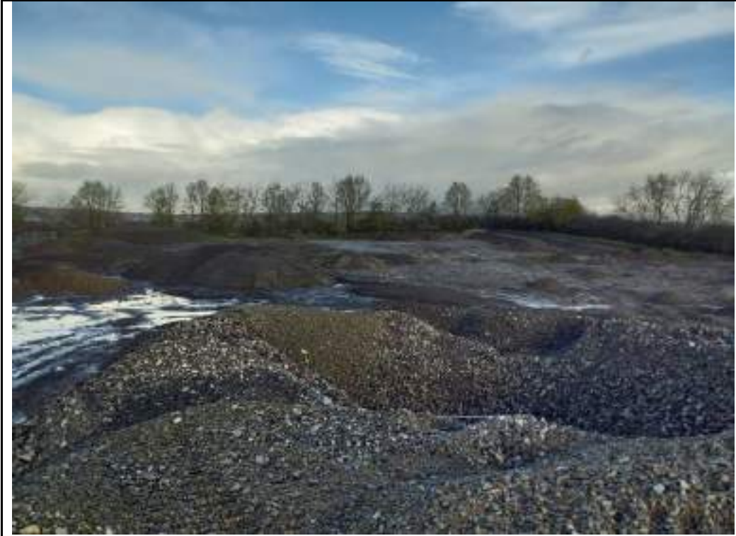
Photograph 11: Overview of stockpiles in the north. Looking towards the north.
