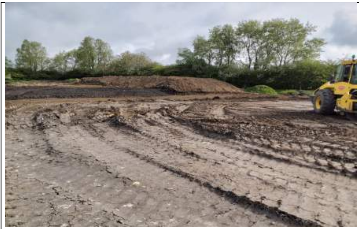
Photograph 6: Stockpile of low strength Glacial till excavated from the borrow pit.
