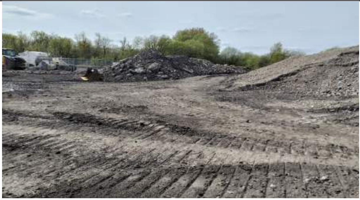
Photograph 10: Stockpile of oversized and concrete material in the western part of the site.
