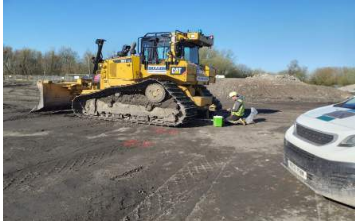
Photograph 3: Plate load testing on fill material in the center east.
