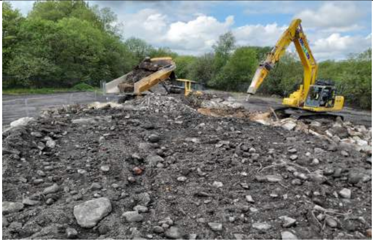
Photograph 11: Stockpiling and breaking of concrete in the northwest. Concrete from excavation in the east.
