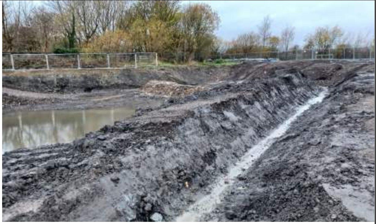
Photograph 11: Temporary drainage ditches to control surface water
