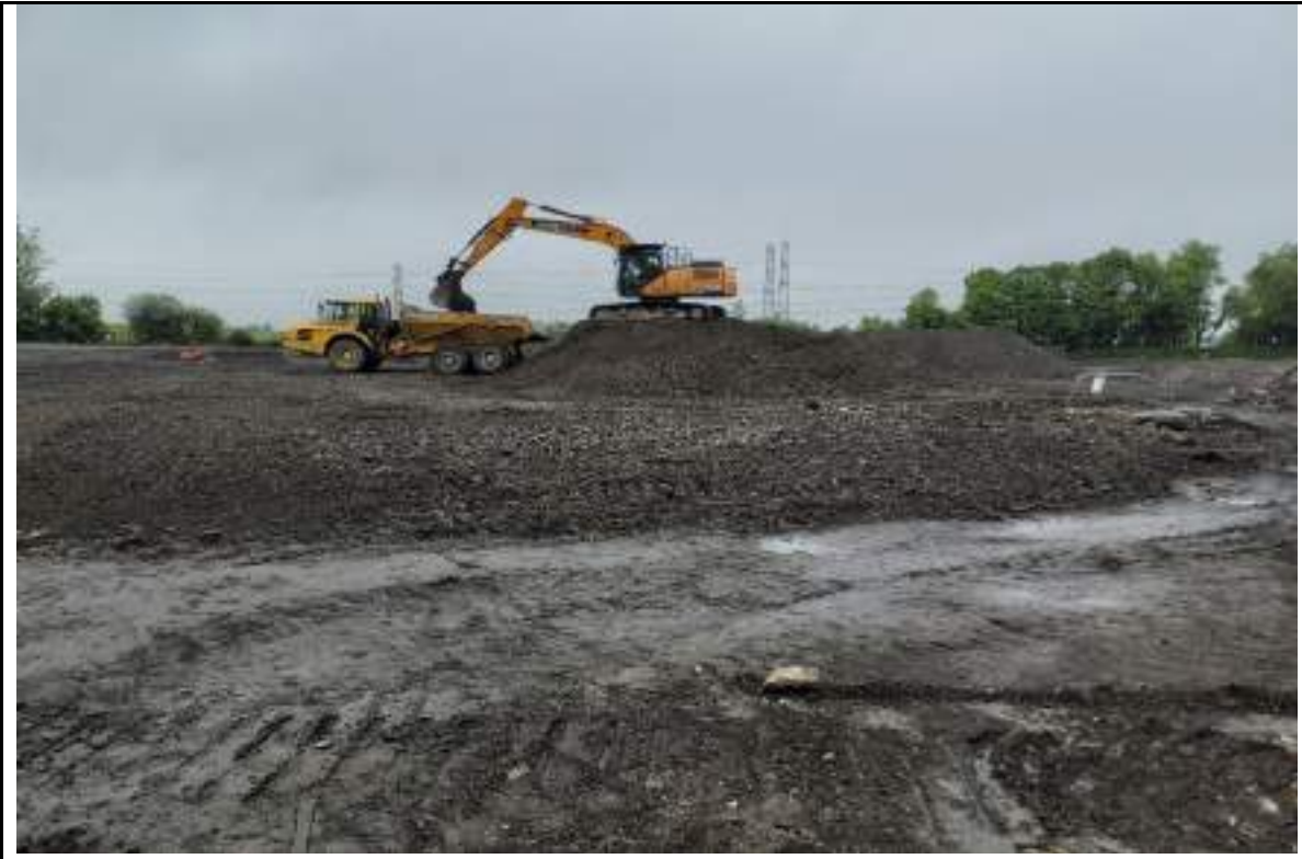
Photograph 7: Removing stockpile of 6F2 material for capping of the southwest.
