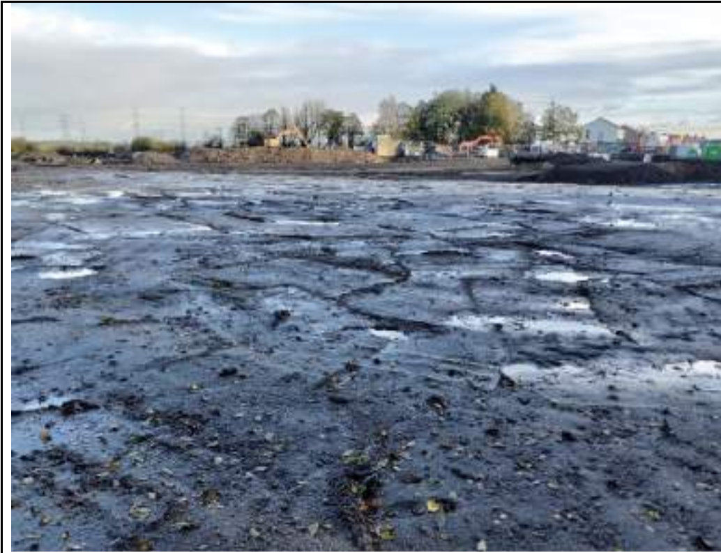
Photograph 19: Overview of the southern part of site. Looking towards the northeast.
