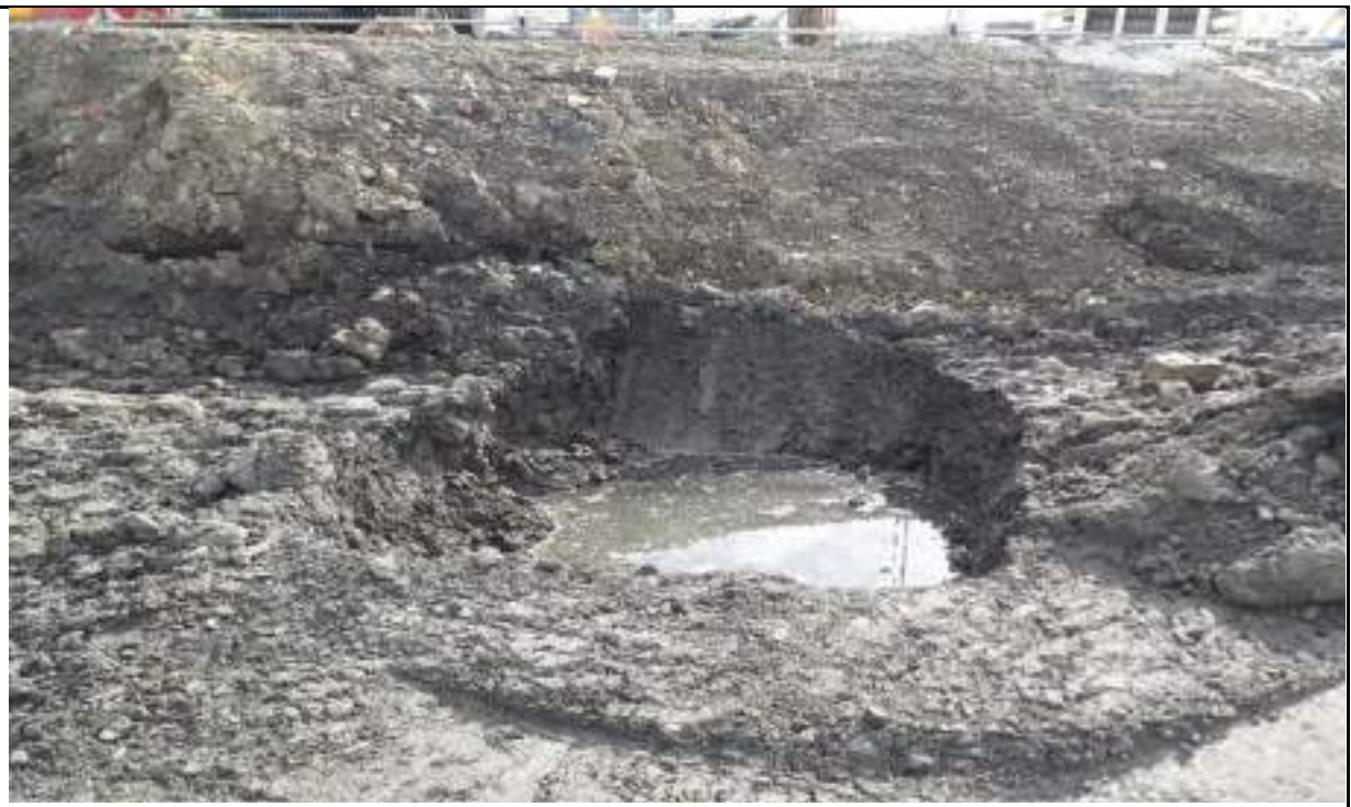
Photograph 12: Trial pit for groundwater monitoring in the centre south. Water observed in three trial pits in the centre south.
