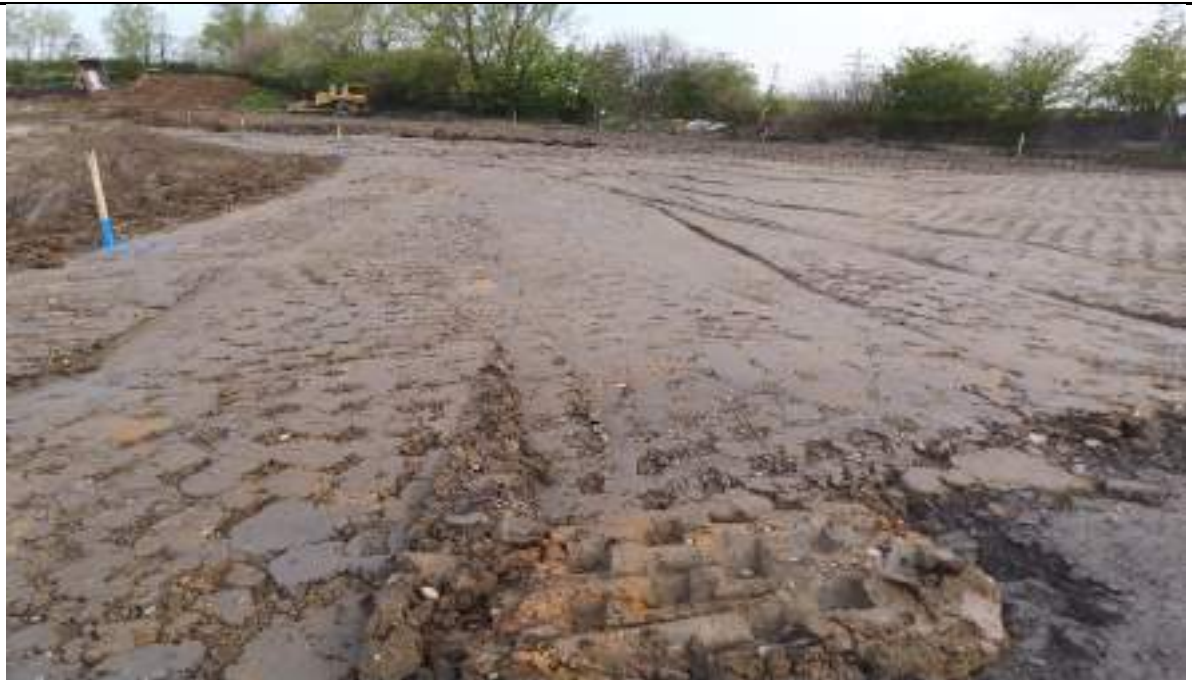
Photograph 4: Placed fill in the northeast and proof rolled with sheepfoot roller. Material from Glacial Till excavation of borrow pit.
