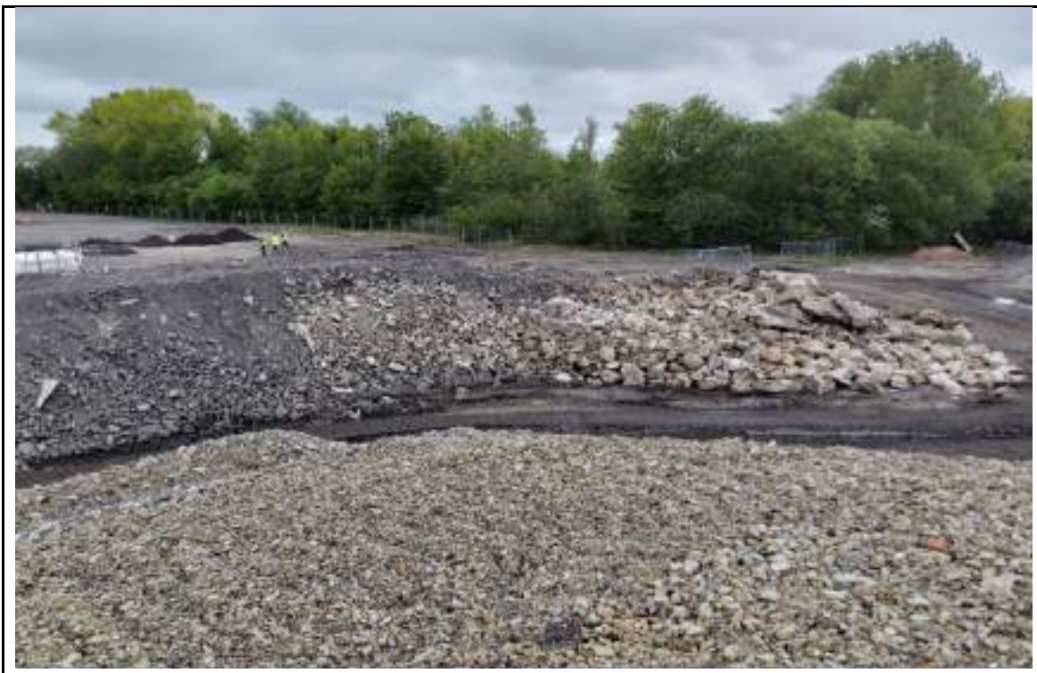
Photograph 8: Stockpile of concrete and oversize material in the northwest.
