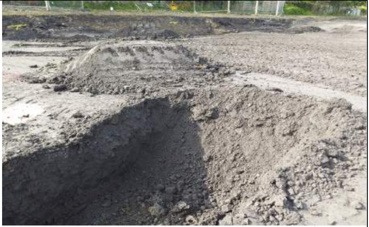
Photograph 17: 3 no. trial pits for groundwater monitoring in the southeast.
