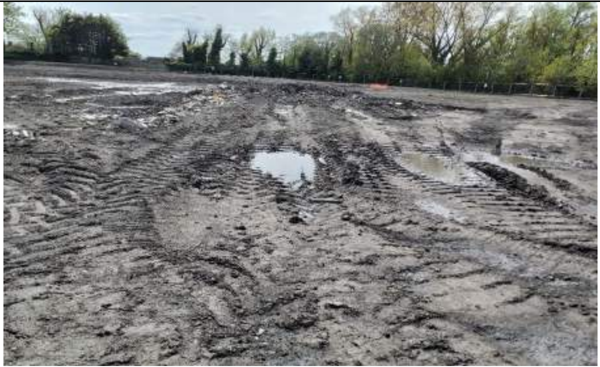
Photograph 11: Temporary Road constructed with oversize material during the wet season in the southwest to be removed.
