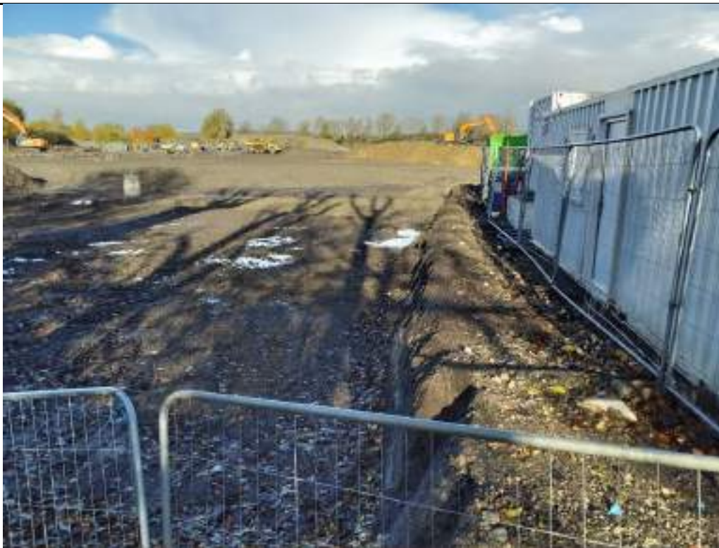
Photograph 24: Backfill in the northwest of VHE compound.
