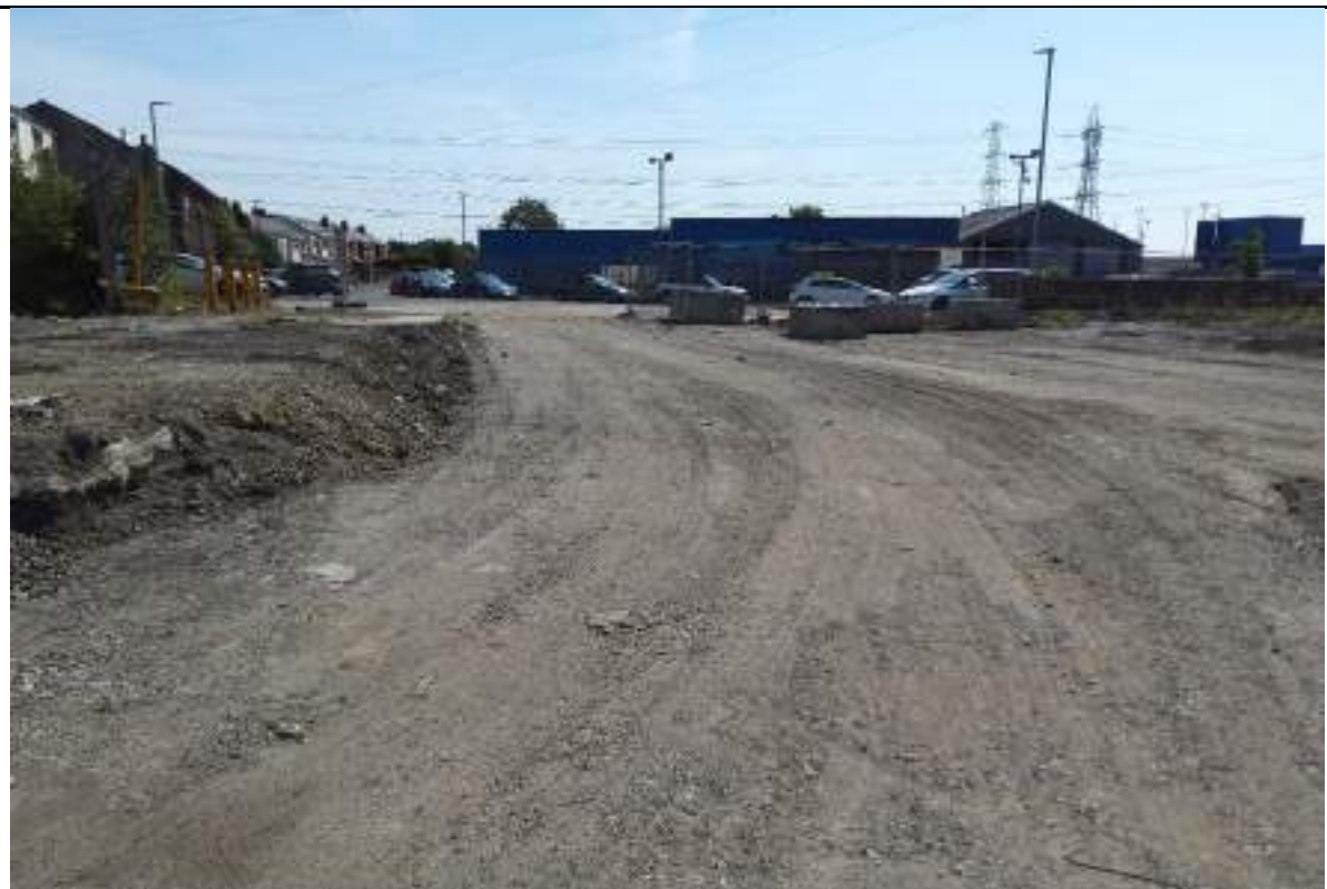
Photograph 2: Completed earthworks in the main gate area.
