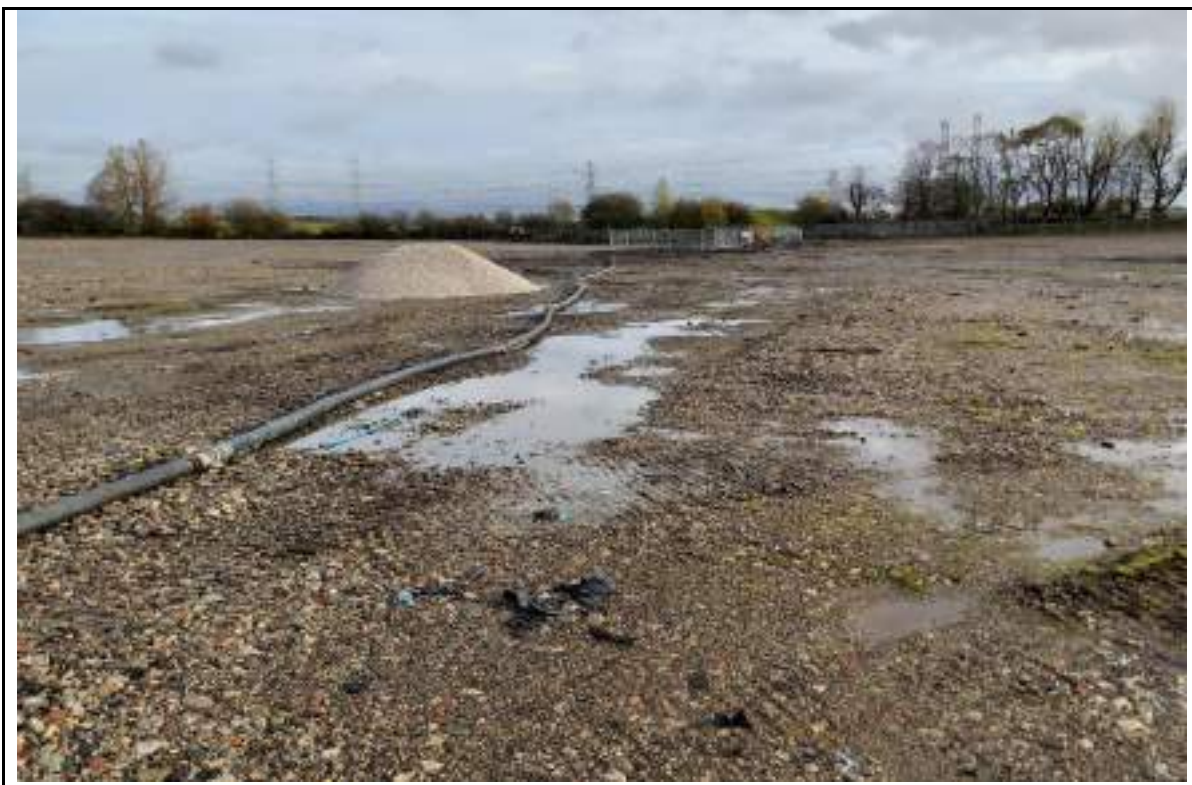
Photograph 6: Pumping water from culvert to the northern and western sewer system.
