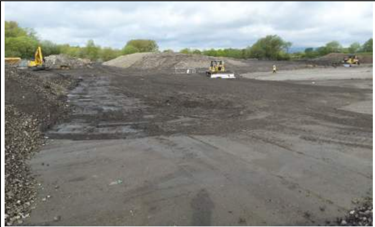
Photograph 3: Stockpiles of 6F2 and oversize materials in the northwest.
