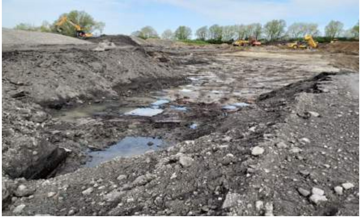
Photograph 3: Peat excavation in the centre east.
