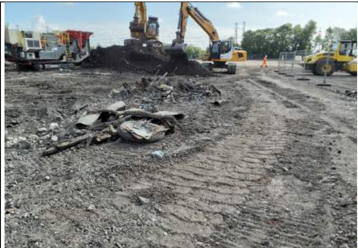
Photograph 4: Stockpile of deleterious material in the northwest.
