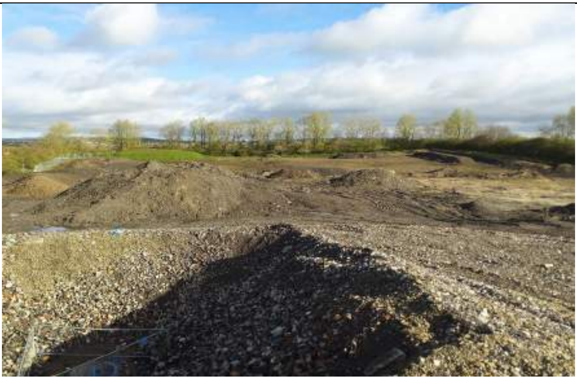
Photograph 6: Stockpiles of excavated peat, organic and unsuitable material in the north.
