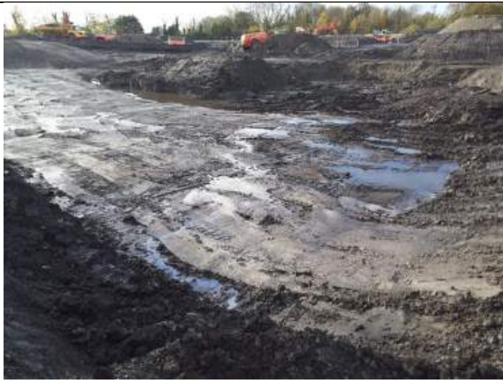
Photograph 6: Excavation in the northeast where organic made Ground was removed.
