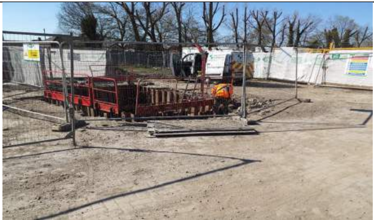
Photograph 12: Thrust bore excavation for drainage in the southeast close to entrance gate completed. Waiting for boring.
