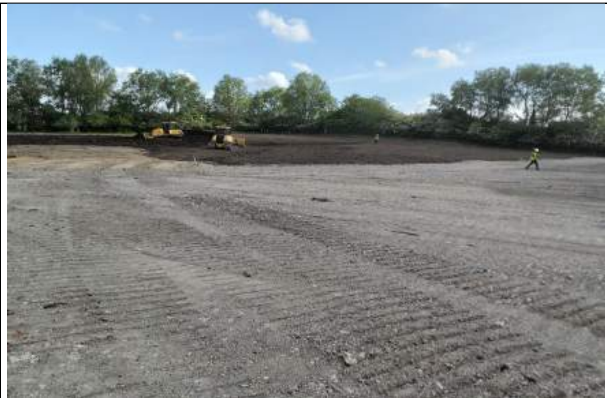
Photograph 8: Placing topsoil in the POS area in the north.
