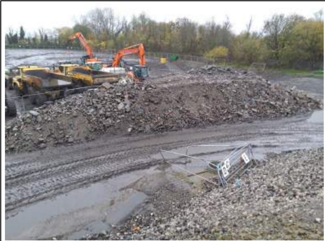
Photograph 93: Stockpile of oversize and concrete materials in the west.
