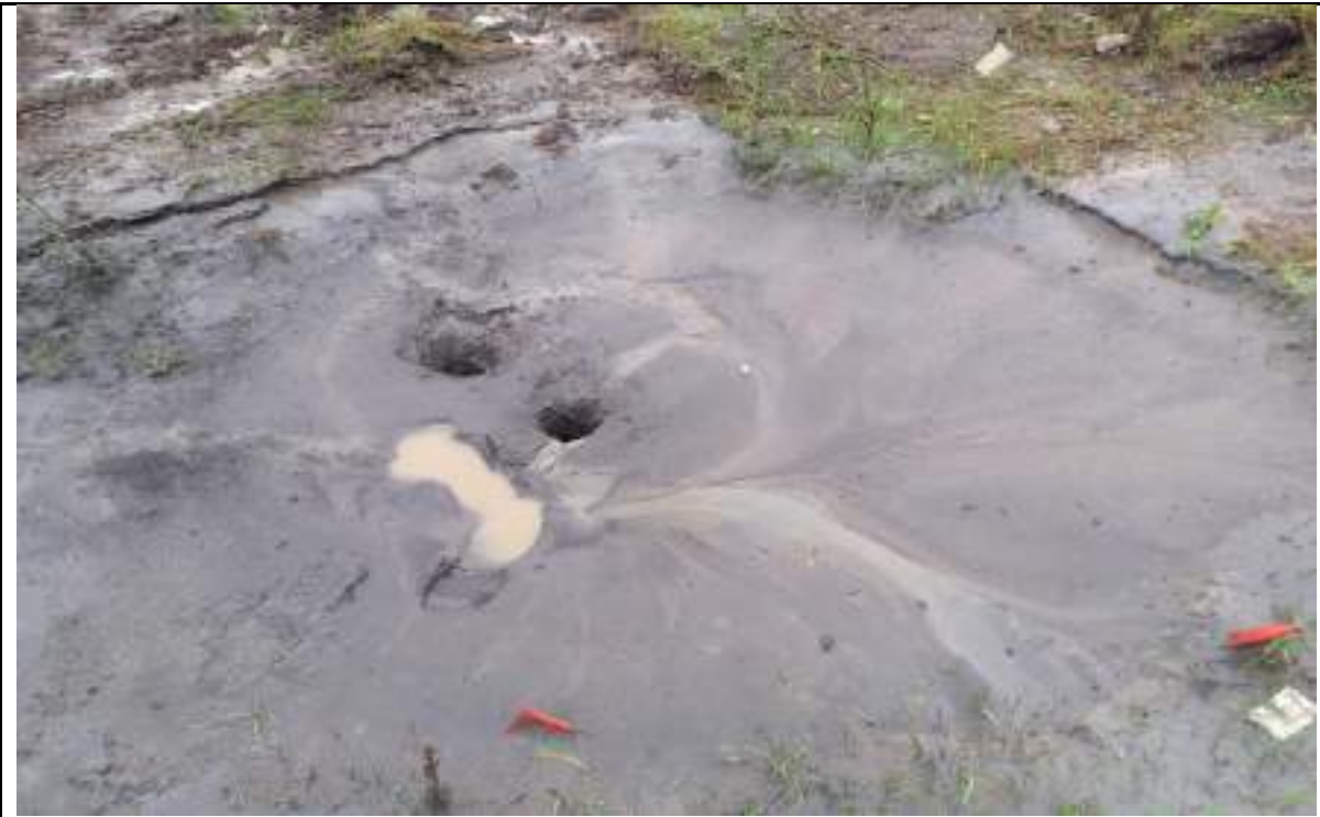
Photograph 1: Grouted boreholes for shaft no.8.
