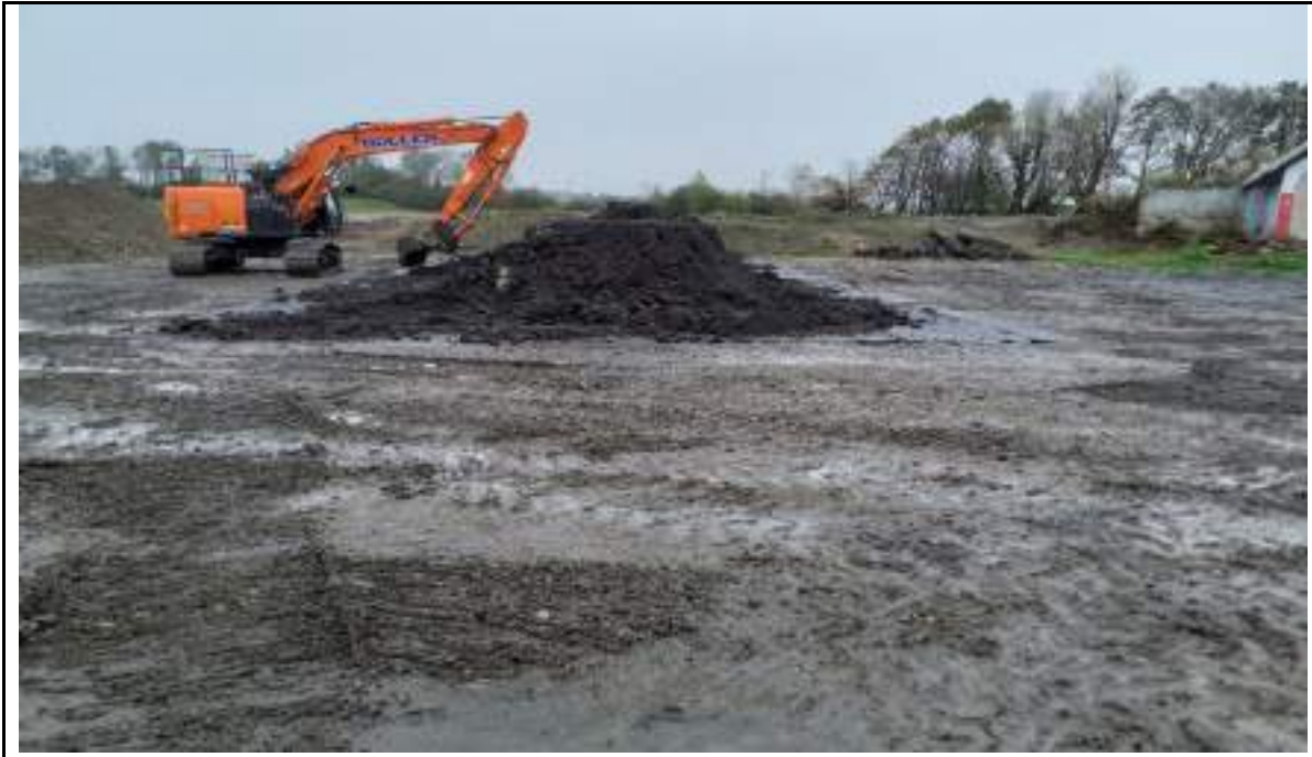
Photograph 3: Stockpile of potentially TPH contaminated material on a black visqueen barrier adjacent to electrical substation. Material excavated from location of shaft no.7.
