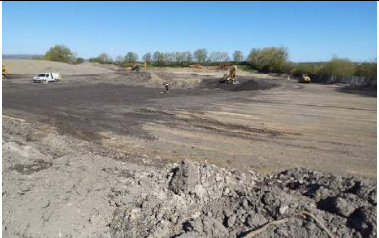
Photograph 11: NDG testing on fill material in the center east.
