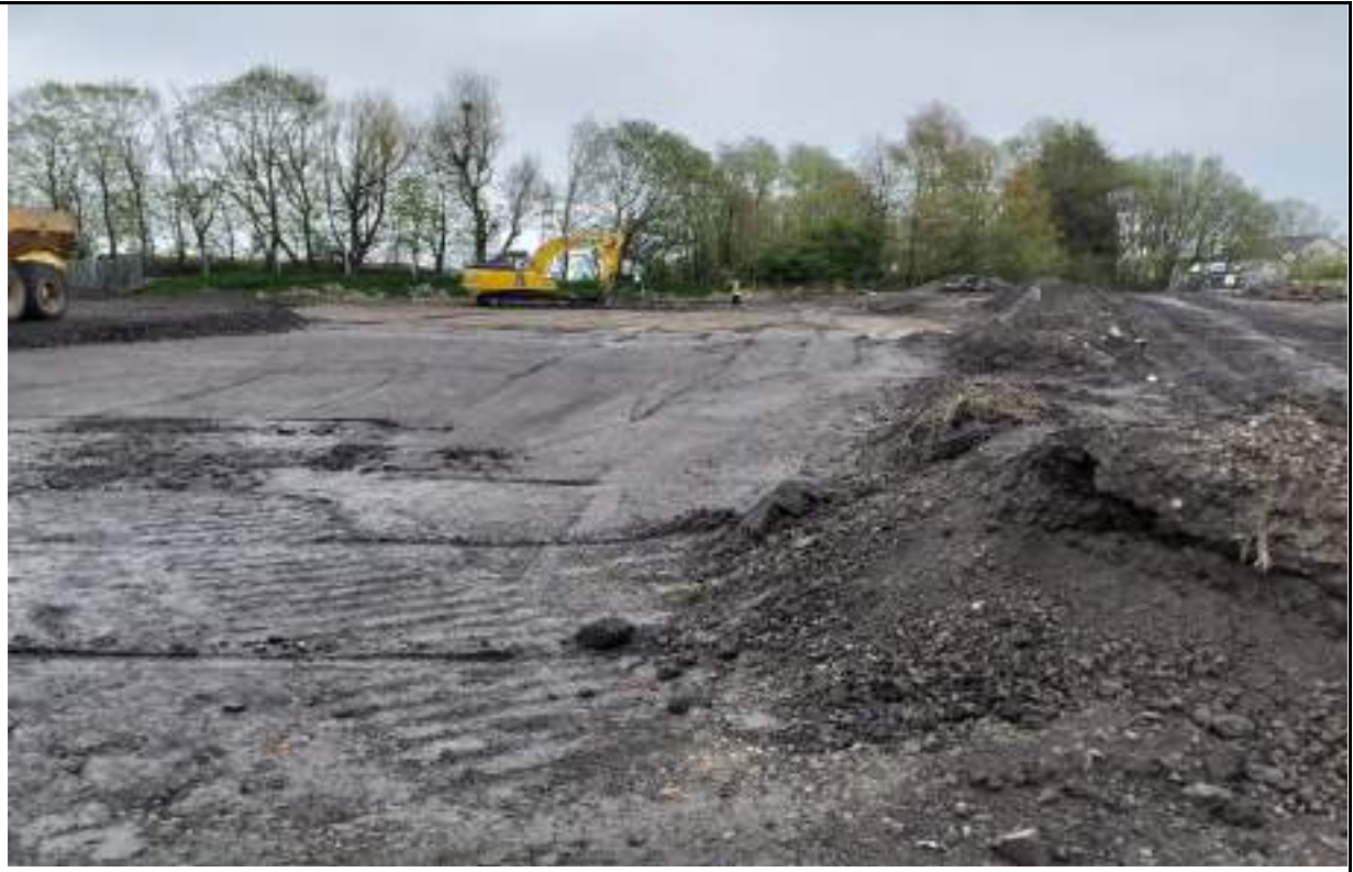
Photograph 13: Site surveying in the east.
