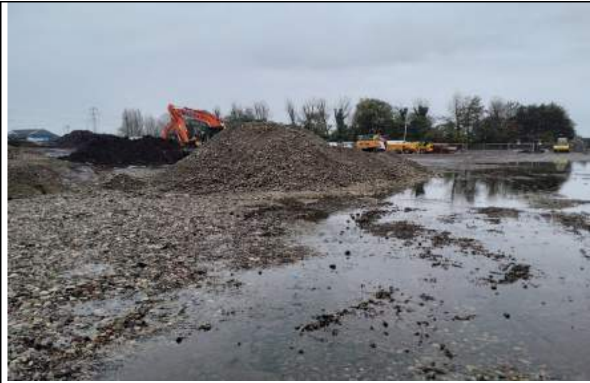
Photograph 7: Stockpile of 6F5 imported material in the southeast adjacent to electrical substation.
