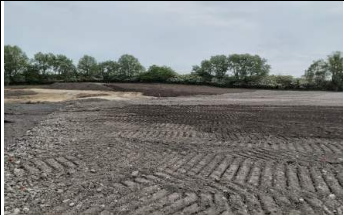
Photograph 7: Placed topsoil and stockpile of topsoil in the POS in the northeast.
