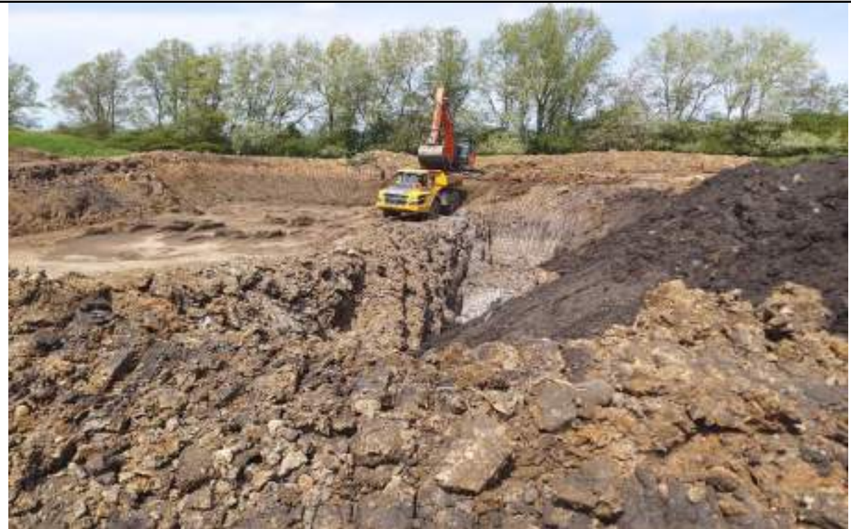
Photograph 7: Excavation of Glacial Till from the borrow pit in the centre north.
