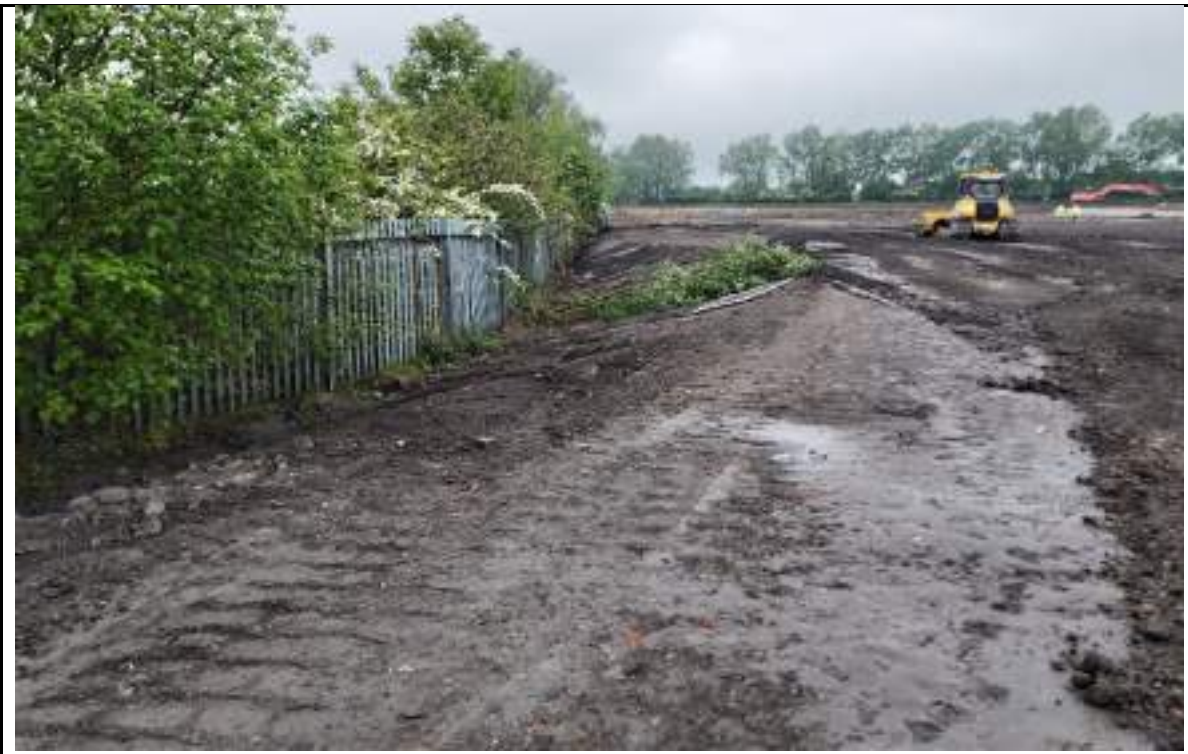
Photograph 8: Place fill sides battered in the northwest.
