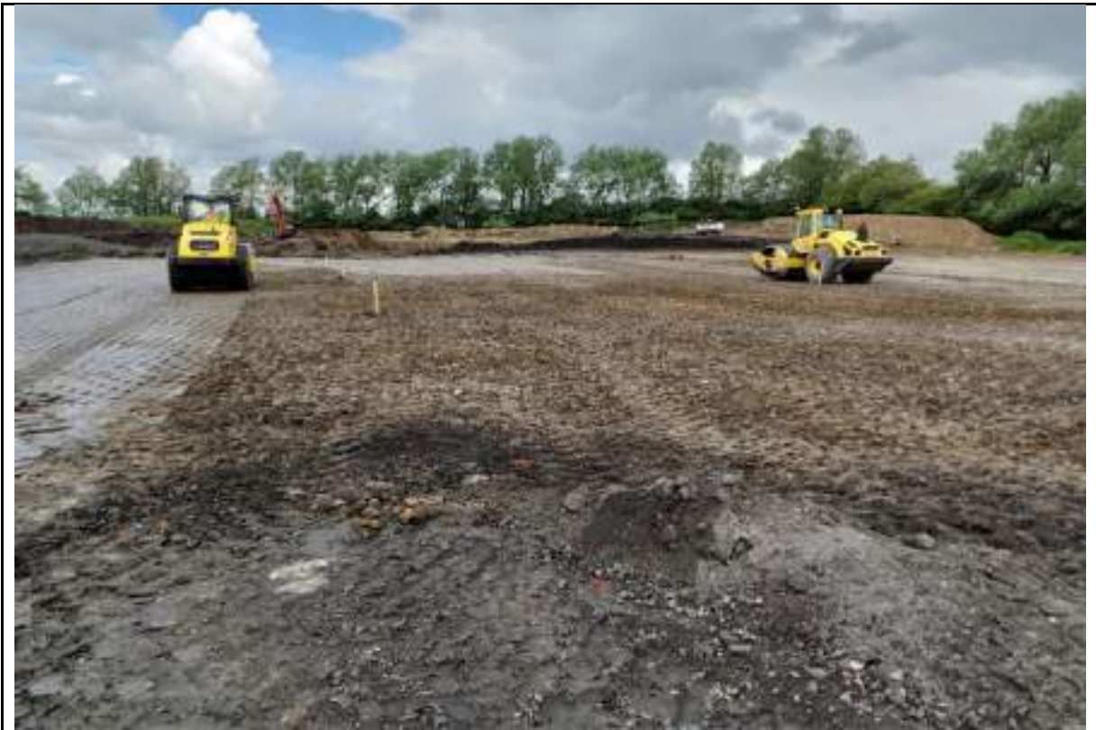
Photograph 6: Proof rolling of placed fill in the north. Material from Glacial Till excavation of the borrow pit.
