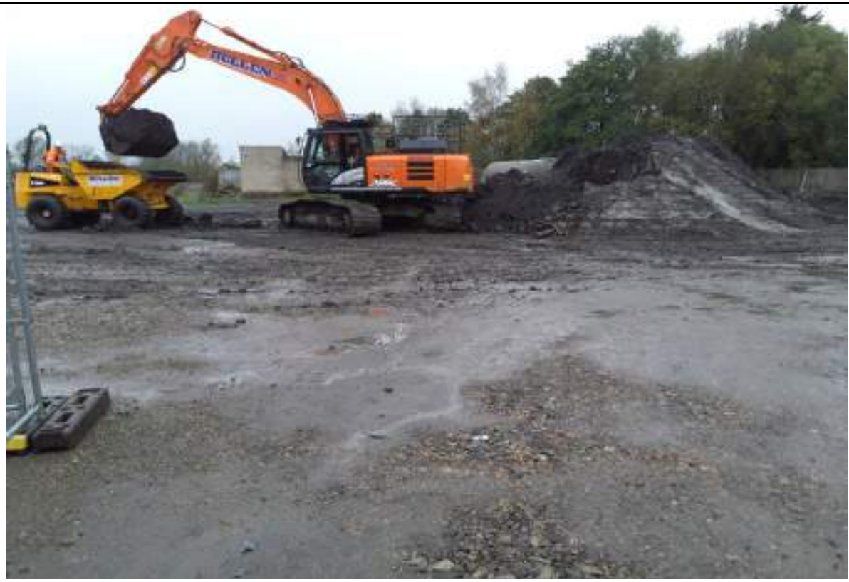
Photograph 2: Stockpile of potentially TPH contaminated material excavated from location of shaft no.7.
