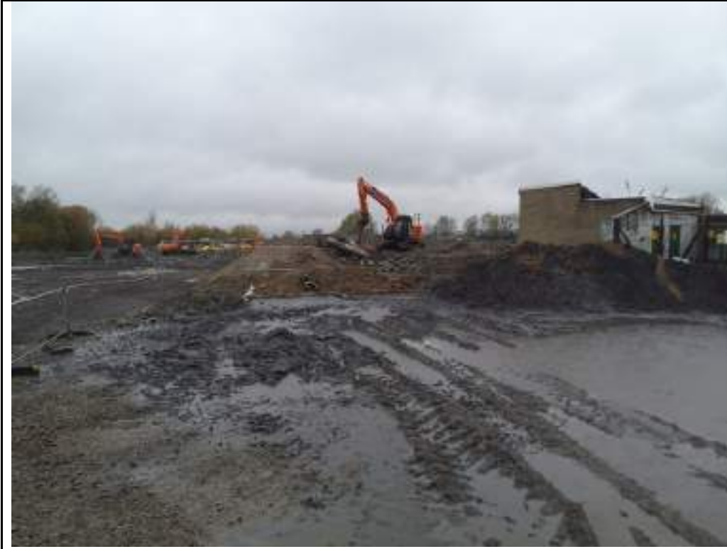
Photograph 19: Removing and breaking concrete in the southeast.
