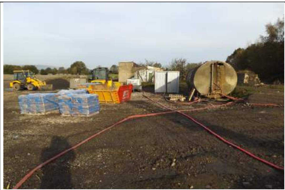
Photograph 2: PFA and OPC stockpiles, water tank and grout mixer adjacent to the shaft no.007.
