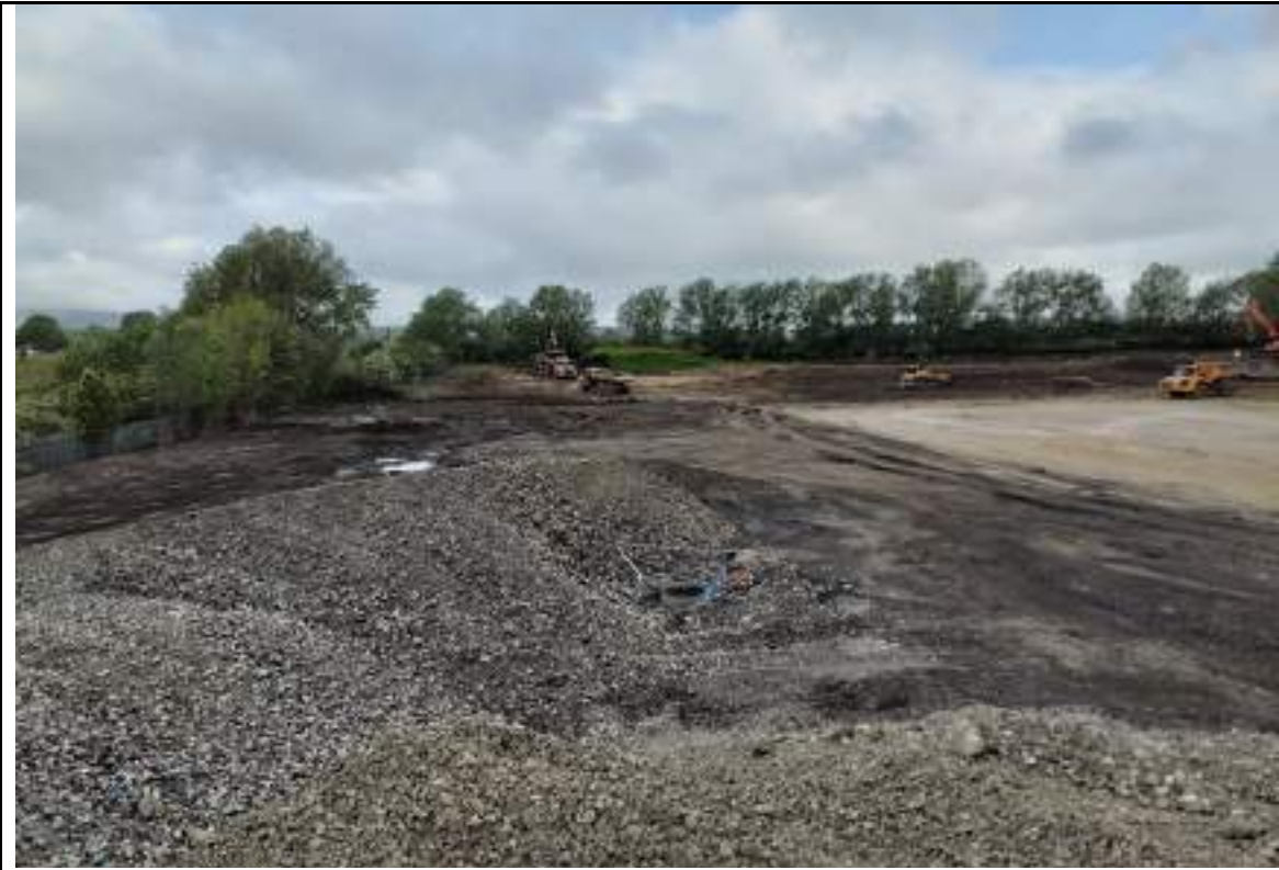
Photograph 9: Removing of stockpile of topsoil in the northwest to backfill the borrow pit.
