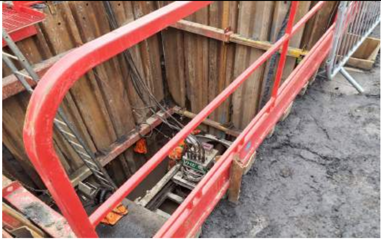
Photograph 12: Boring of thrust bore drainage in the southeast.
