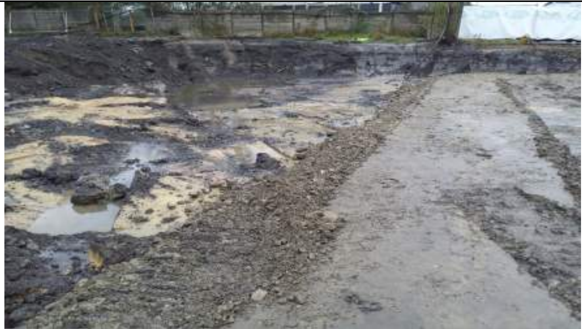
Photograph 1: Excavation of Potentially TPH contaminated Made Ground in the location of shaft no.7. Glacial till at the base of the excavation observed. 6F5 material placed in the southern part to provide running layer.
