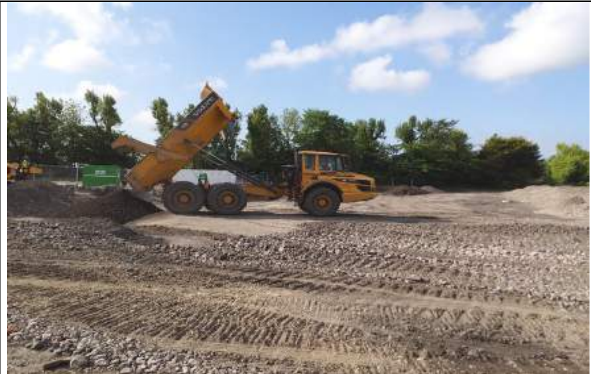
Photograph 1: Placing fill in the southeast near VHE compound. Fill material from crusher's fine materials in the northwest.
