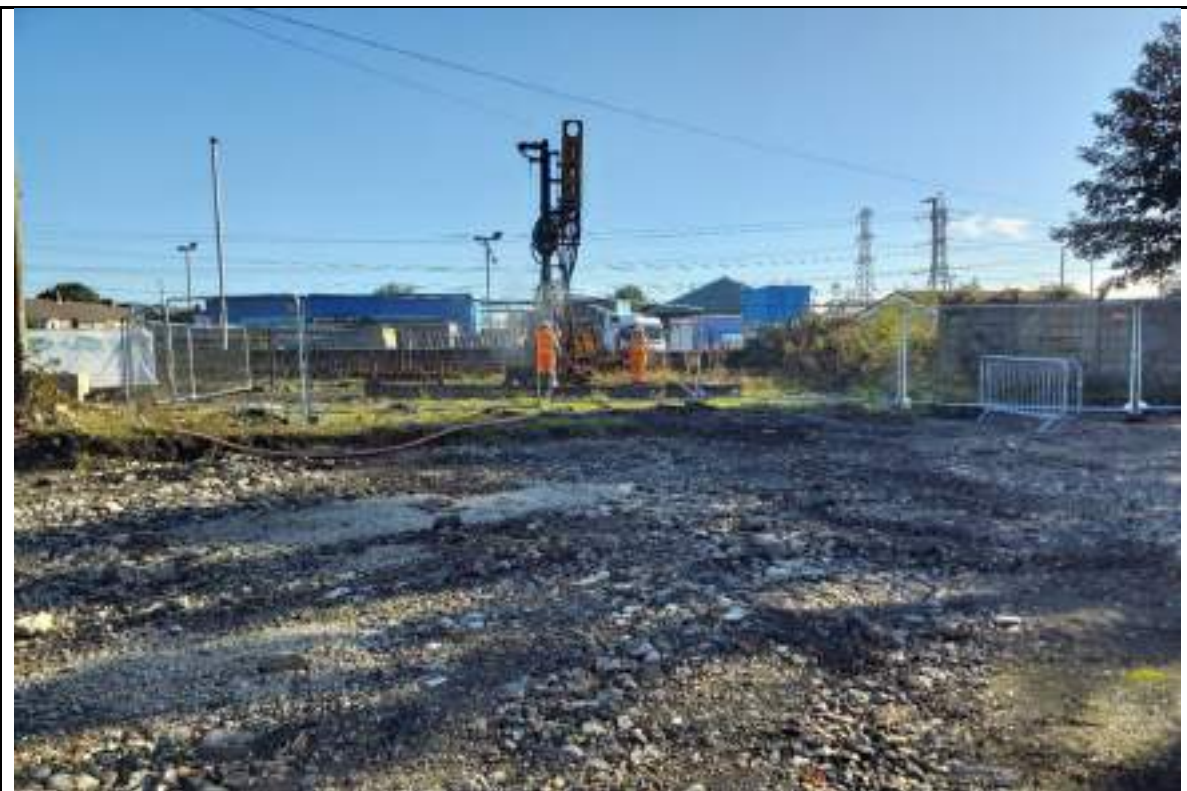
Photograph 4: Grouting of shaft no.8.
