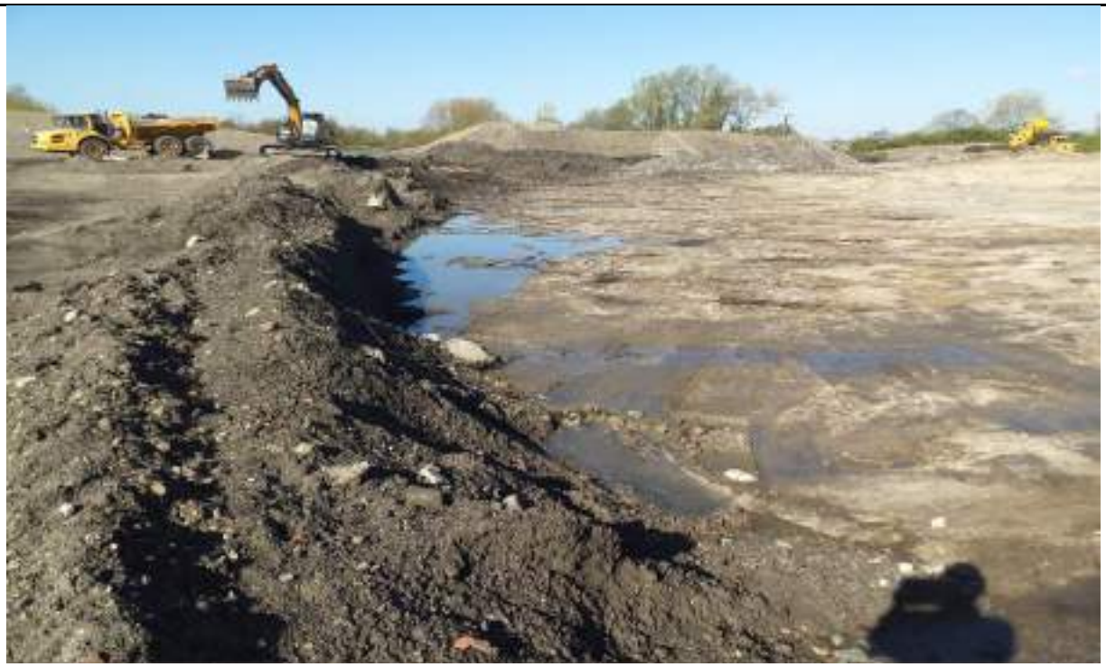
Photograph 8: Standing water in excavation in the northeast. Glacial till is visible at the base of excavation.
