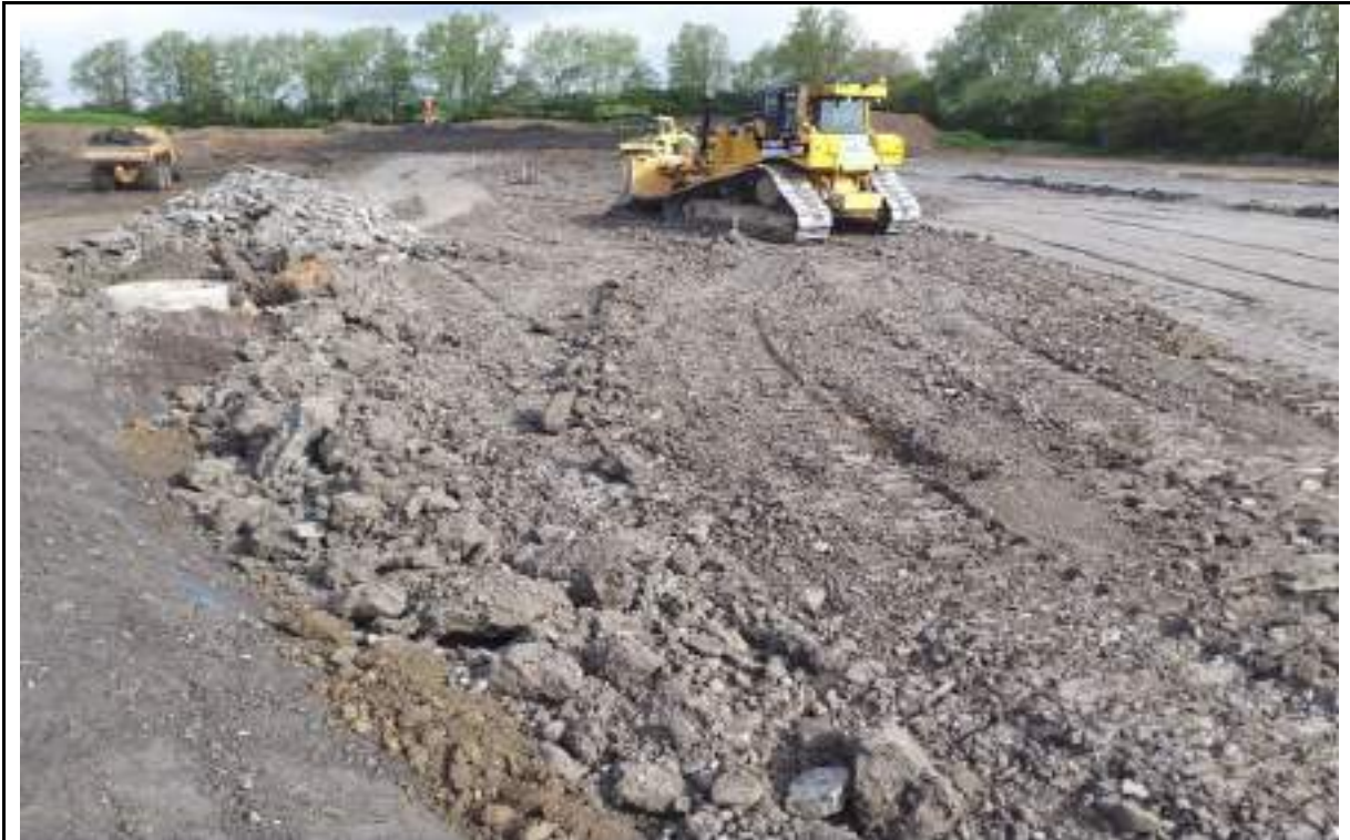
Photograph 5: Placing excavated mudstone from borrow pit in the centre northeast. Fill is proof rolled using sheepfoot roller.
