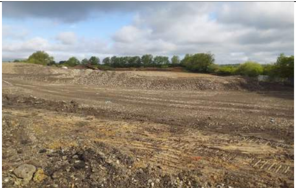
Photograph 2: Stockpile of 6F2 material in the east.
