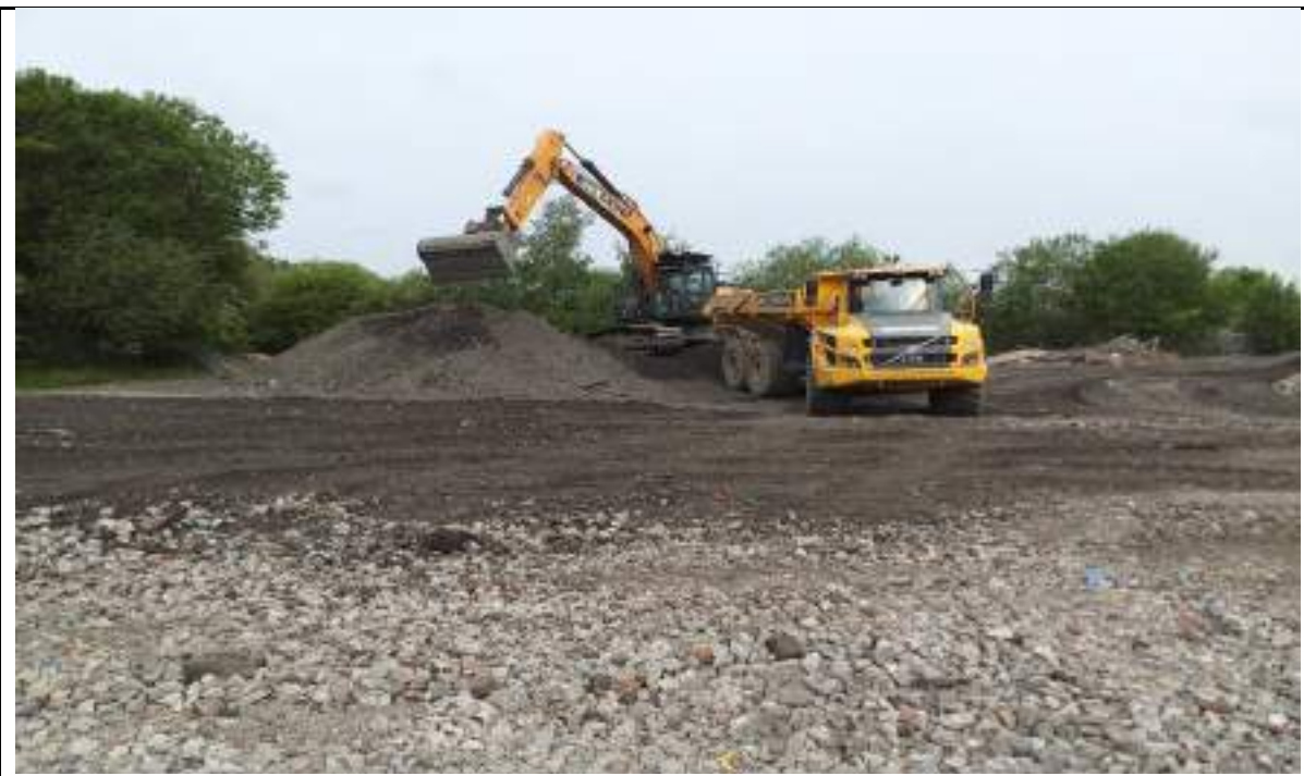
Photograph 2: Stockpile of fine material from crusher and stockpile of deleterious materials in the northwest.
