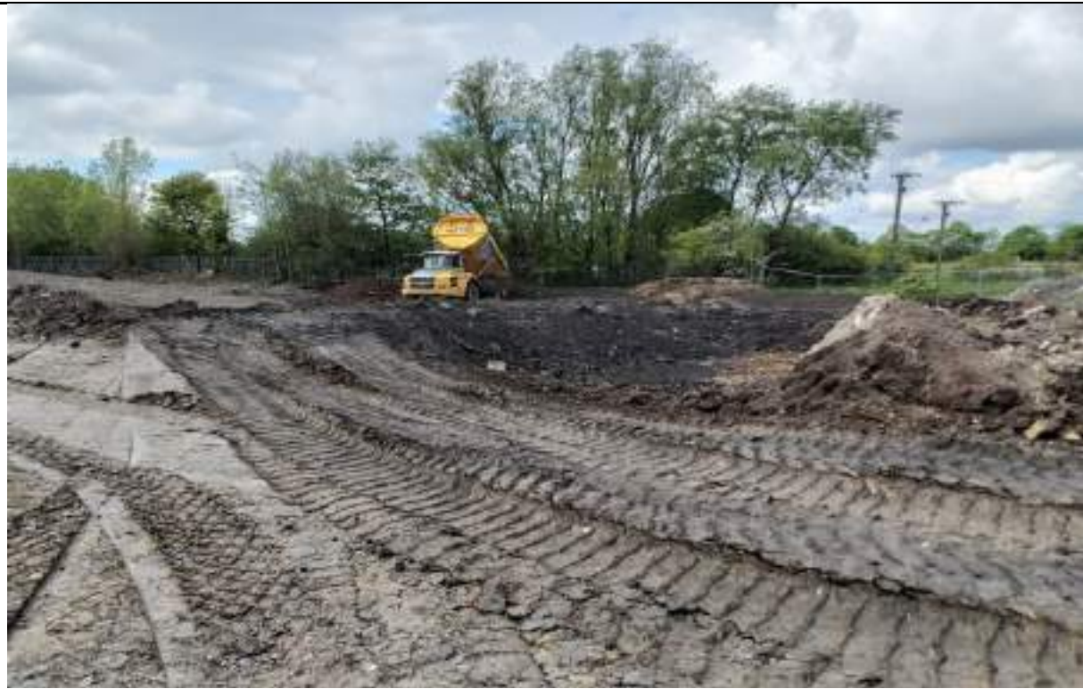
Photograph 2: Stockpiling excavated Glacial Till from the east in the northwest.
