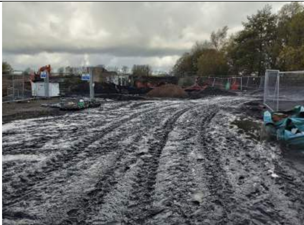
Photograph 2: Grouting platform after completion of grouting shaft no.6 in eastern part of the site.
