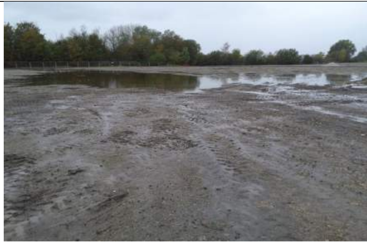
Photograph 6: Standing water in the centre of the site.
