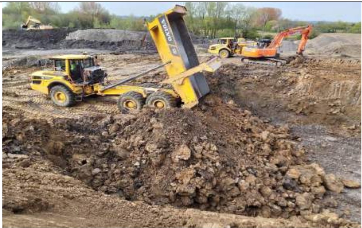
Photograph 8: Unloading excavated unsuitable Glacial Till in the south of the borrow pit.
