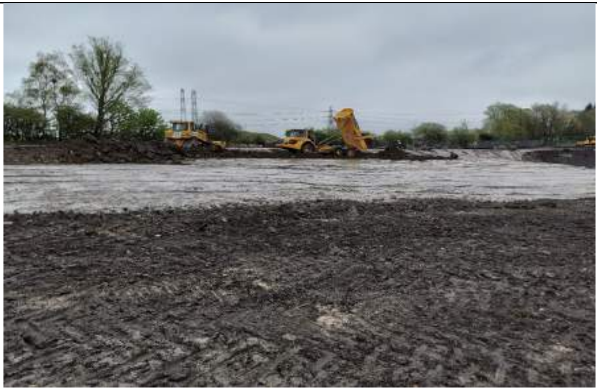
Photograph 8: Placing fill in the northeast. Glacial till material from the borrow pit.
