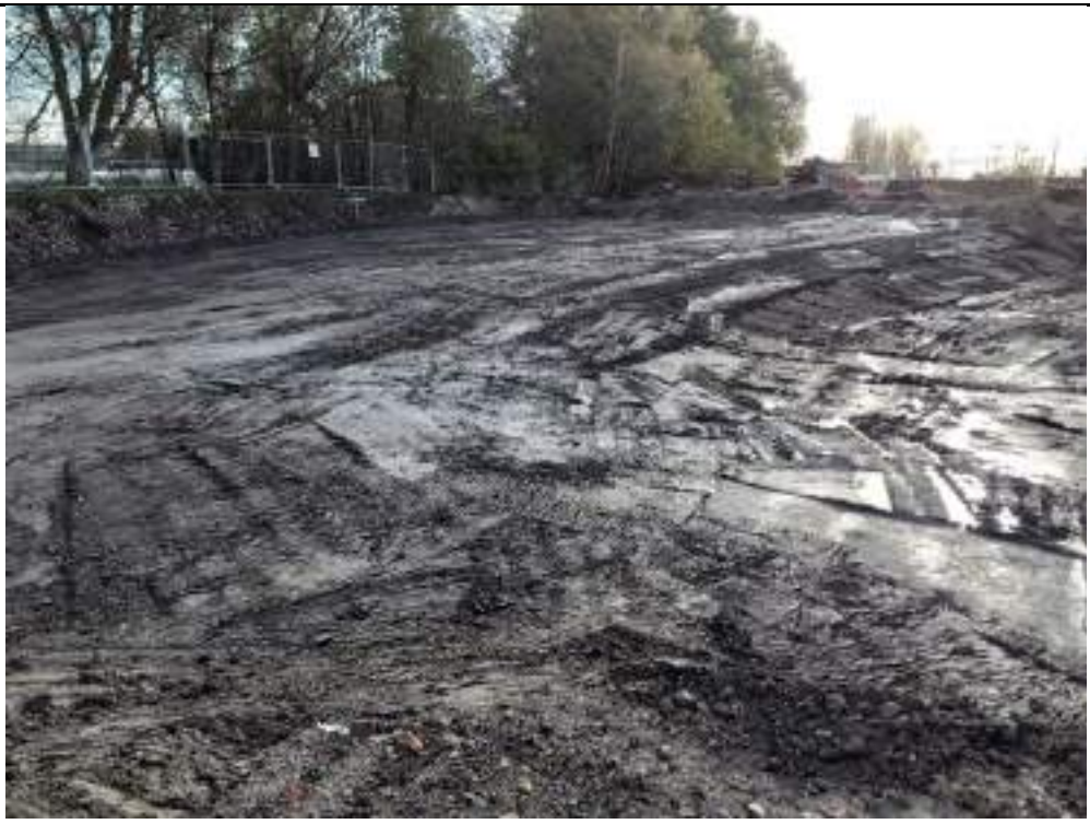
Photograph 4: Eastern part of site backfilled with lime treated soil.
