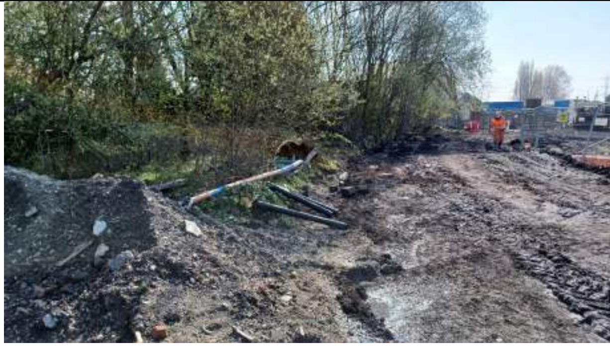
Photograph 2: Southeastern boundary where additional excavation required between electric cable and site boundary
