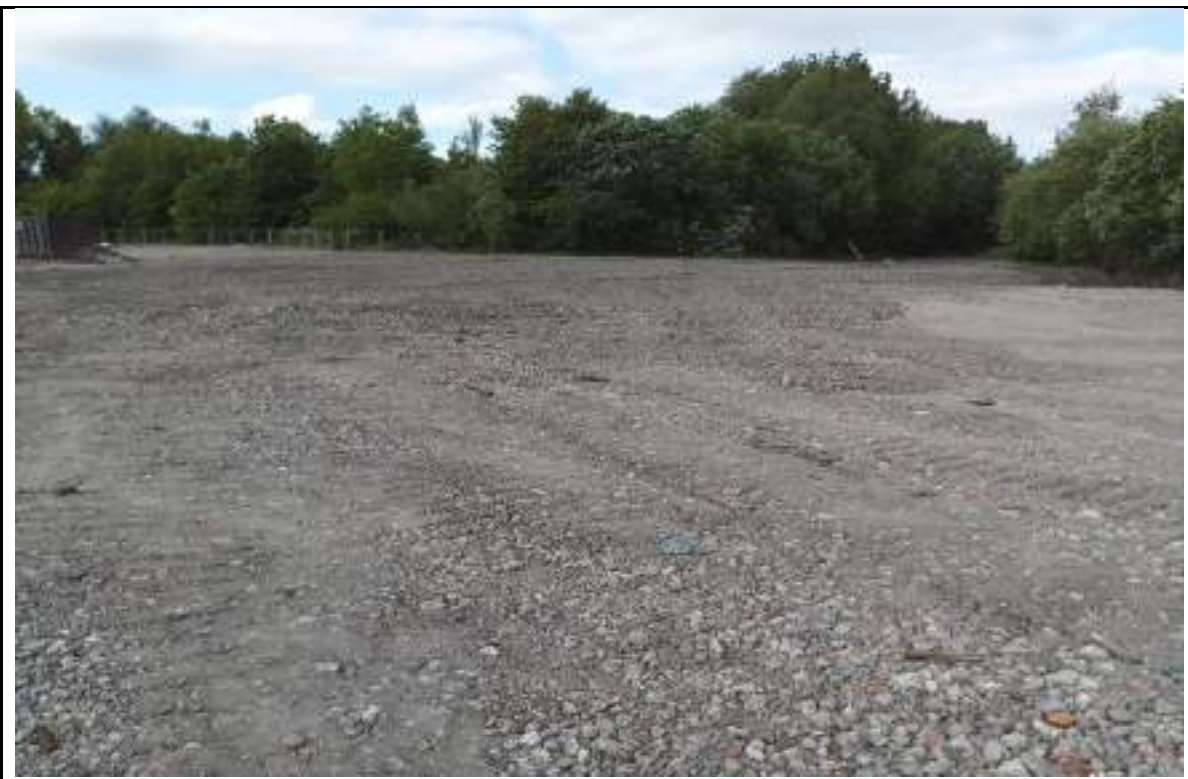
Photograph 8: Capping layer placed in the northwest.
