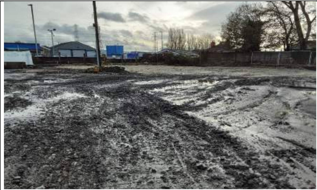
Photograph 1: Shaft no.8 backfilled with 6F5 material.
