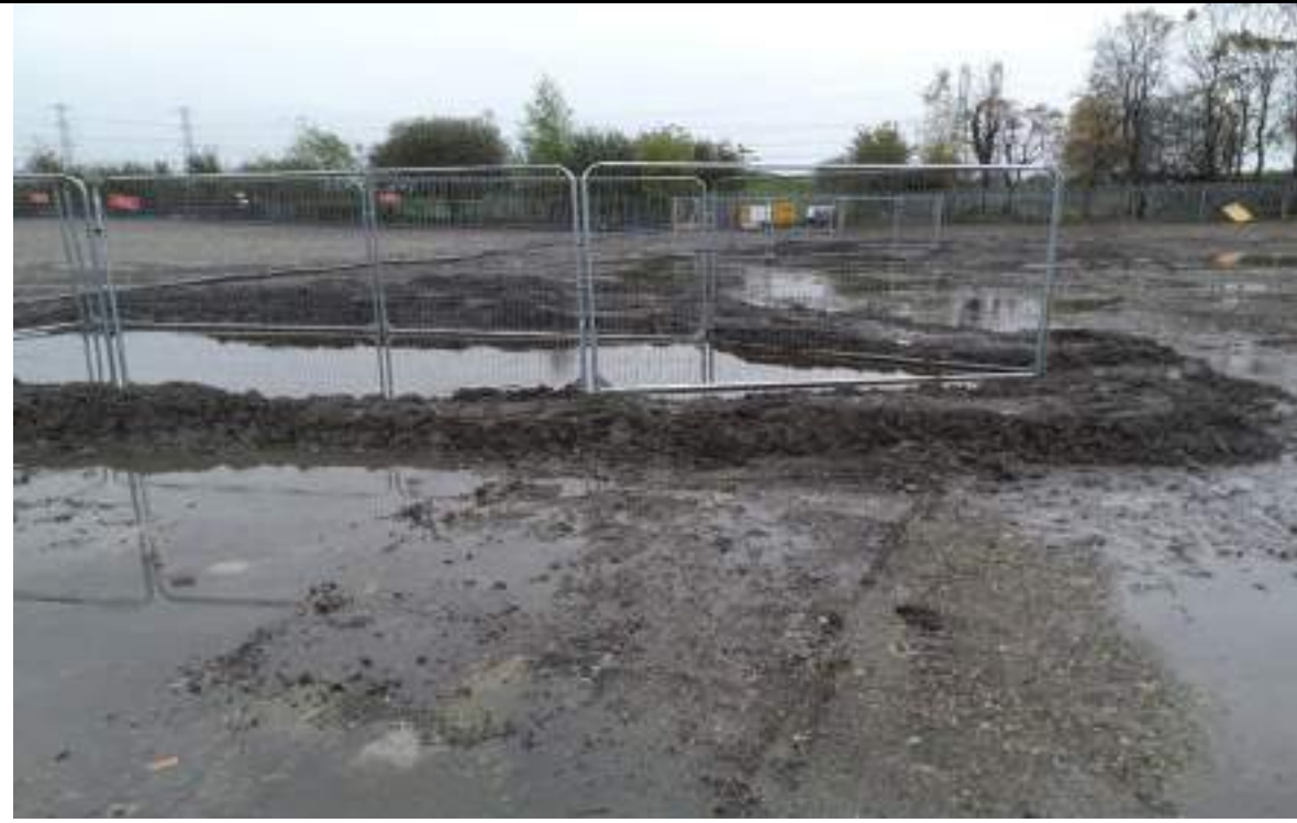
Photograph 5: Excavations in the centre and east to find location of culvert.
