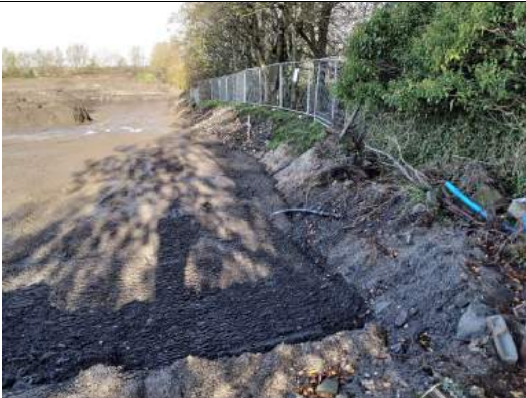
Photograph 28: Southeastern boundary of site. Looking towards the north.
