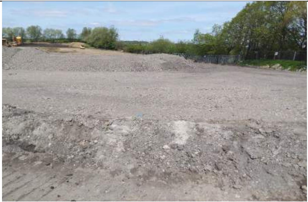
Photograph 2: 6F2 material placed in the east.
