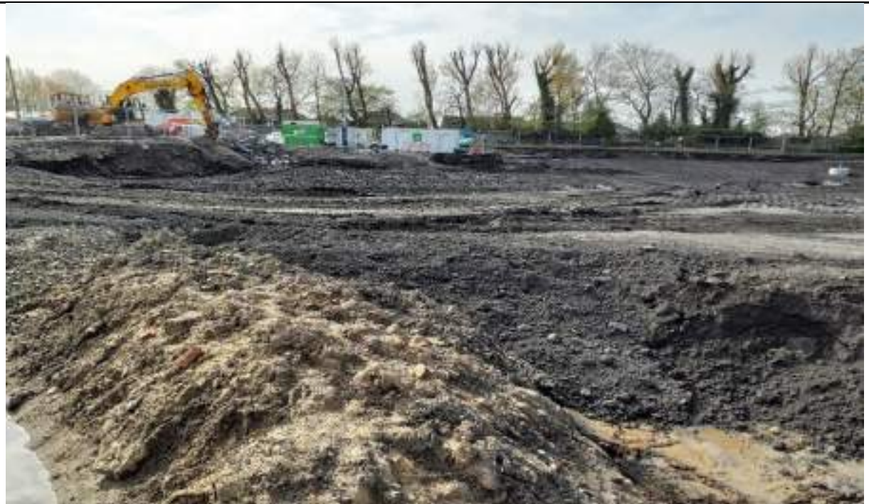
Photograph 16: Placed fill in the southeast. Fill proof rolled with sheepfoot roller.
