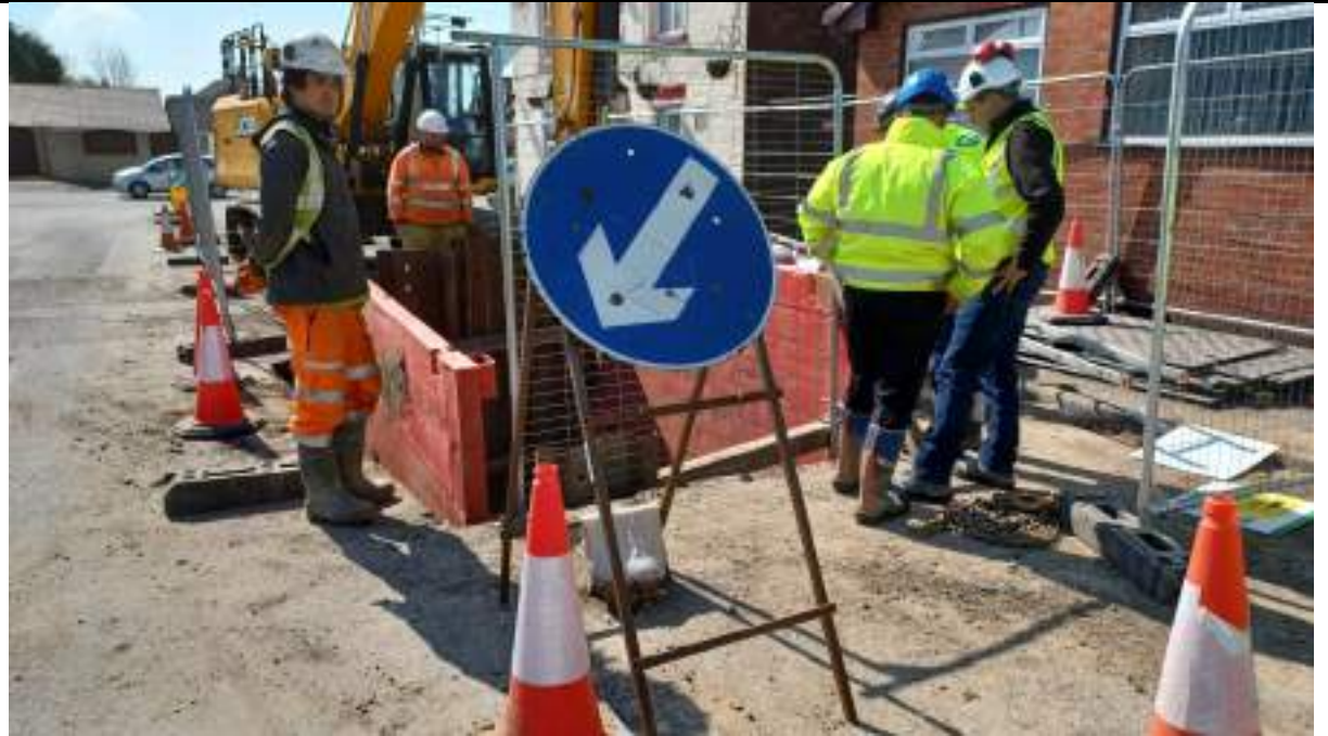
Photograph 10: Southern end of thrust bore excavation on Stopes Road for drainage connection
