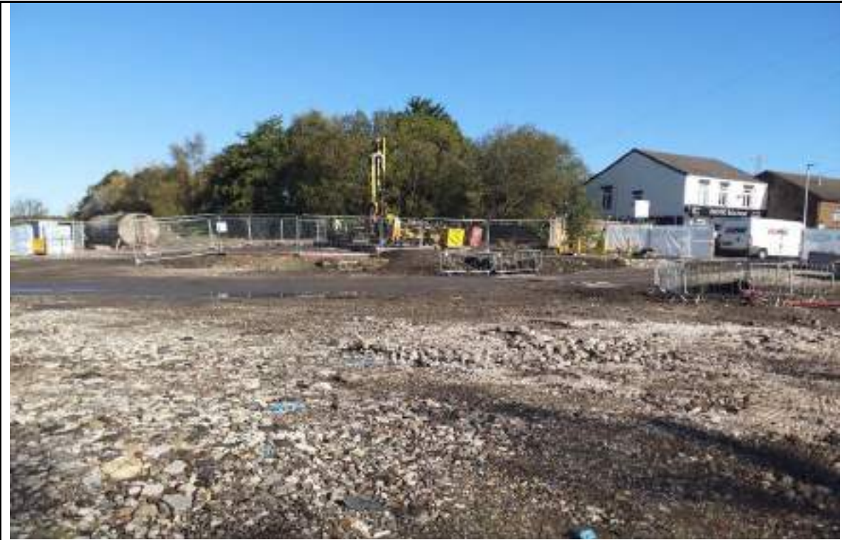
Photograph 3: Grouting started after backfilling of the shaft no.7.
