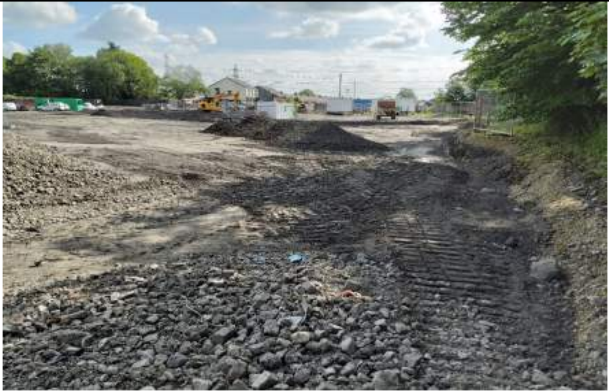
Photograph 113: Demobing VHE's compound in the southern boundary.
