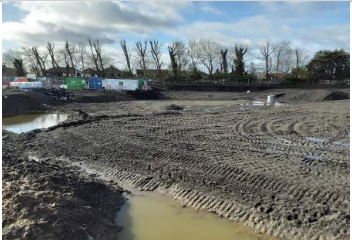
Photograph 16: VHE compound area in the southeast.
