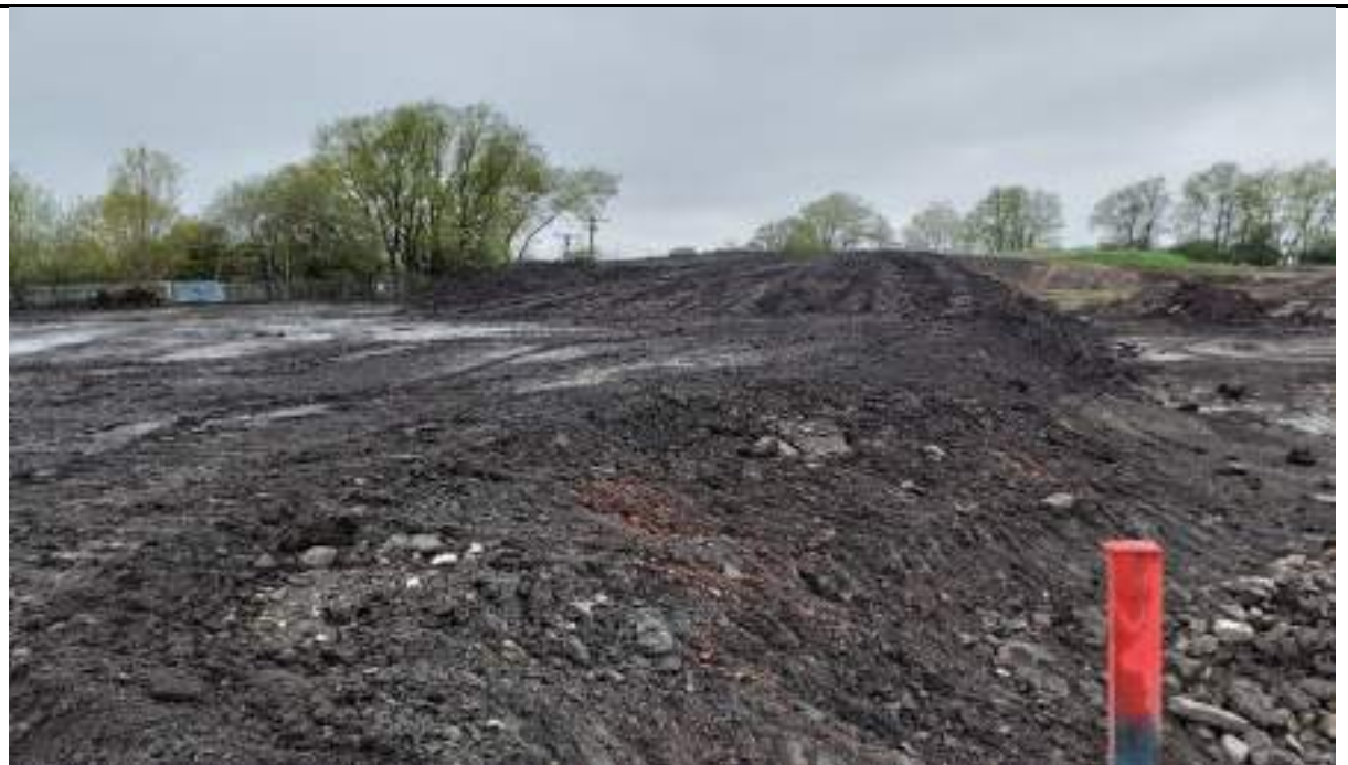
Photograph 10: Stockpile of peat and organic material in the northwest.
