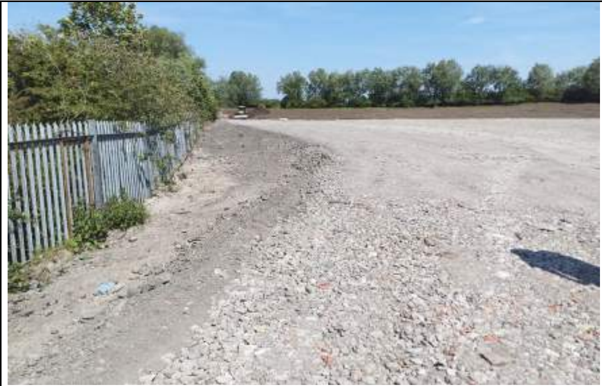
Photograph 7: The northwestern boundary of the site. Looking towards the north.
