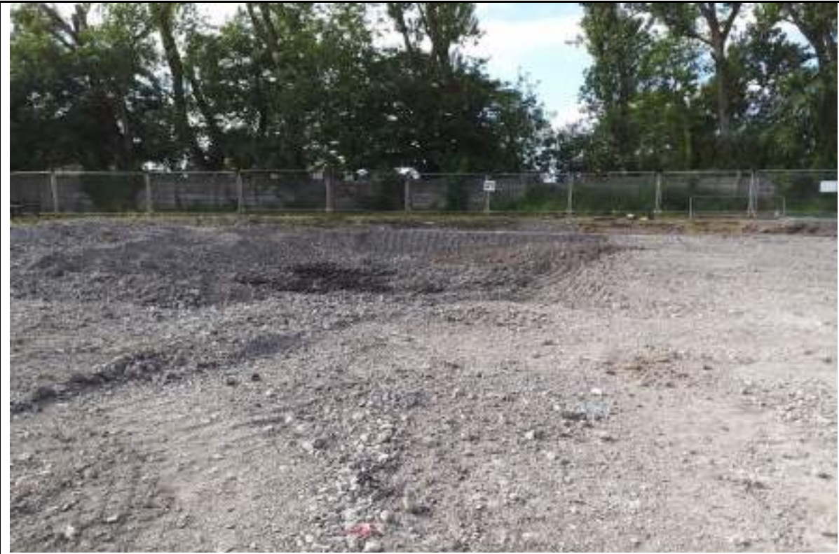
Photograph 1: Re-excavation of 6F2 material in the southeast.
