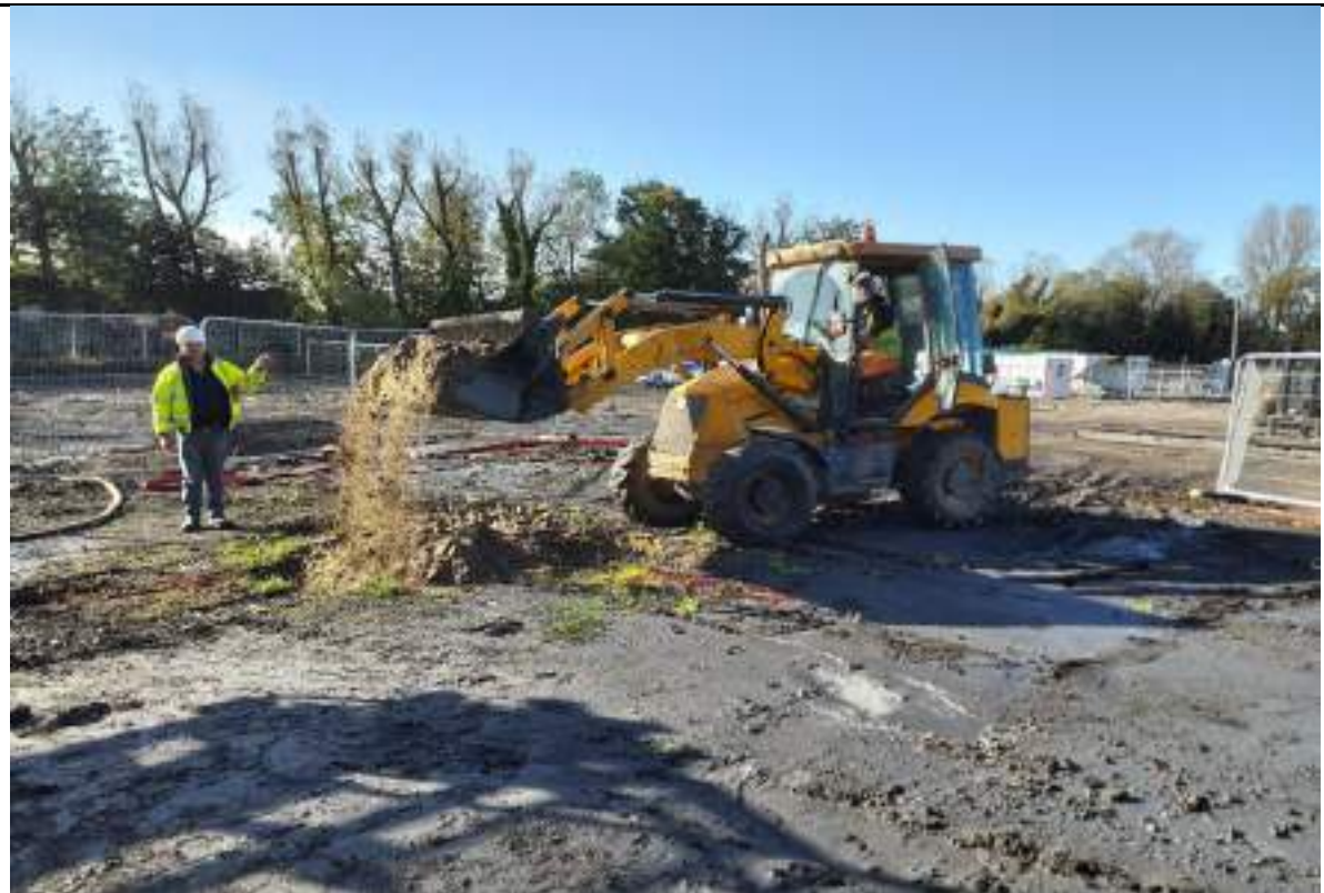
Photograph 2: Backfilling the shaft no.7 surface settlement.
