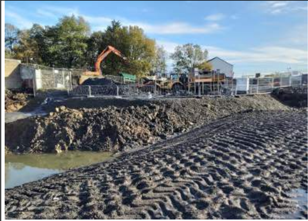
Photograph 21: Mine shaft treatment platform after completion of grouting shaft no.006.
