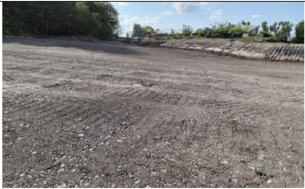
Photograph 12: Capping layer placed in the east and haul road in the southeast.
