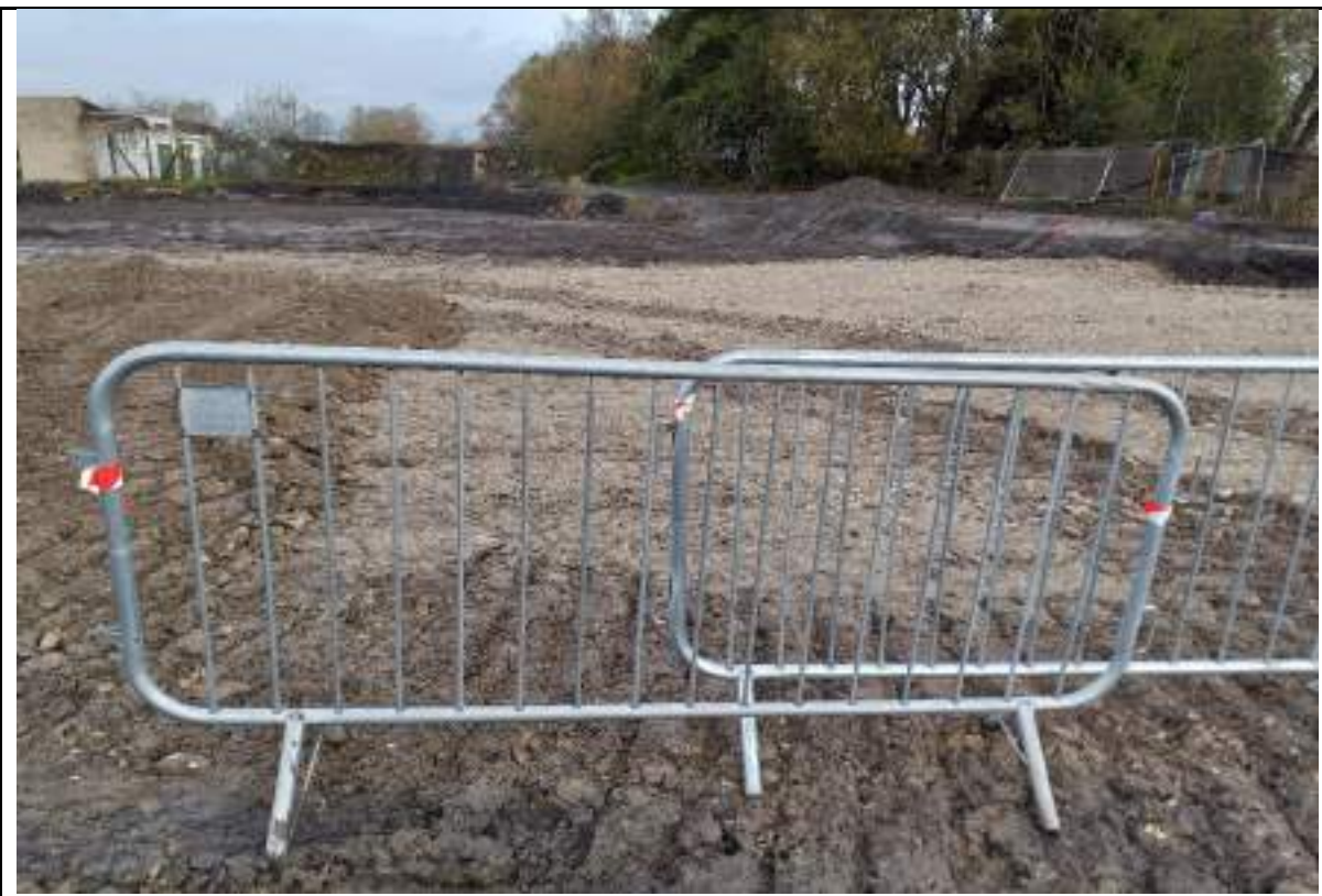
Photograph 2: Ongoing backfilling of excavation in location of shaft no.7 with 6F5 material
