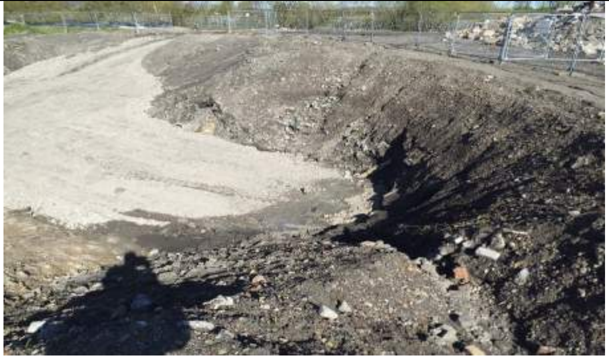
Photograph 13: Grouting of abstraction well in the northwest completed. Over-steepened slopes around abstraction borehole to be re-profiled
