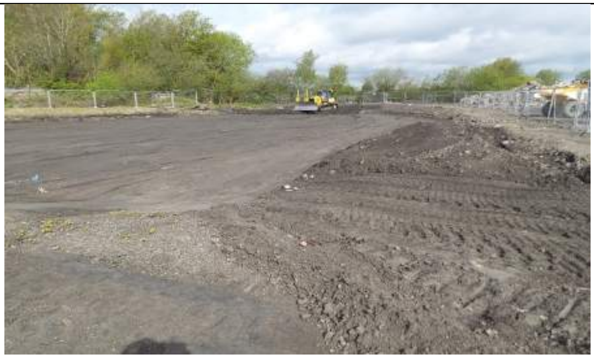
Photograph 10: Placing fill in the western boundary near grouted abstraction well. Material from excavated landfill Made Ground in the eastern boundary.
