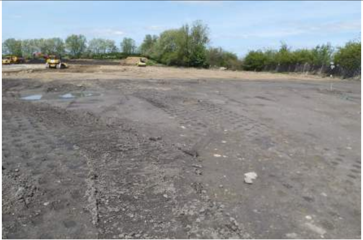
Photograph 3: placed fill in the northeast.
