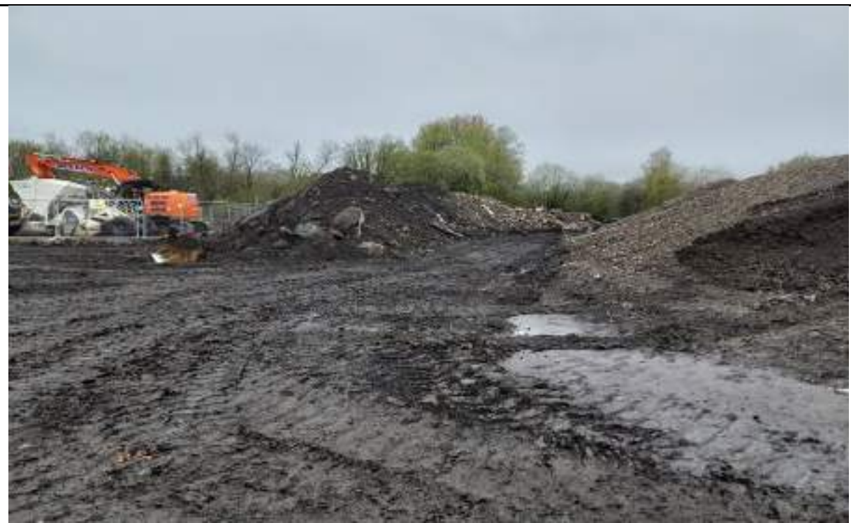
Photograph 12: Stockpile of concrete and oversized material in the northwest.
