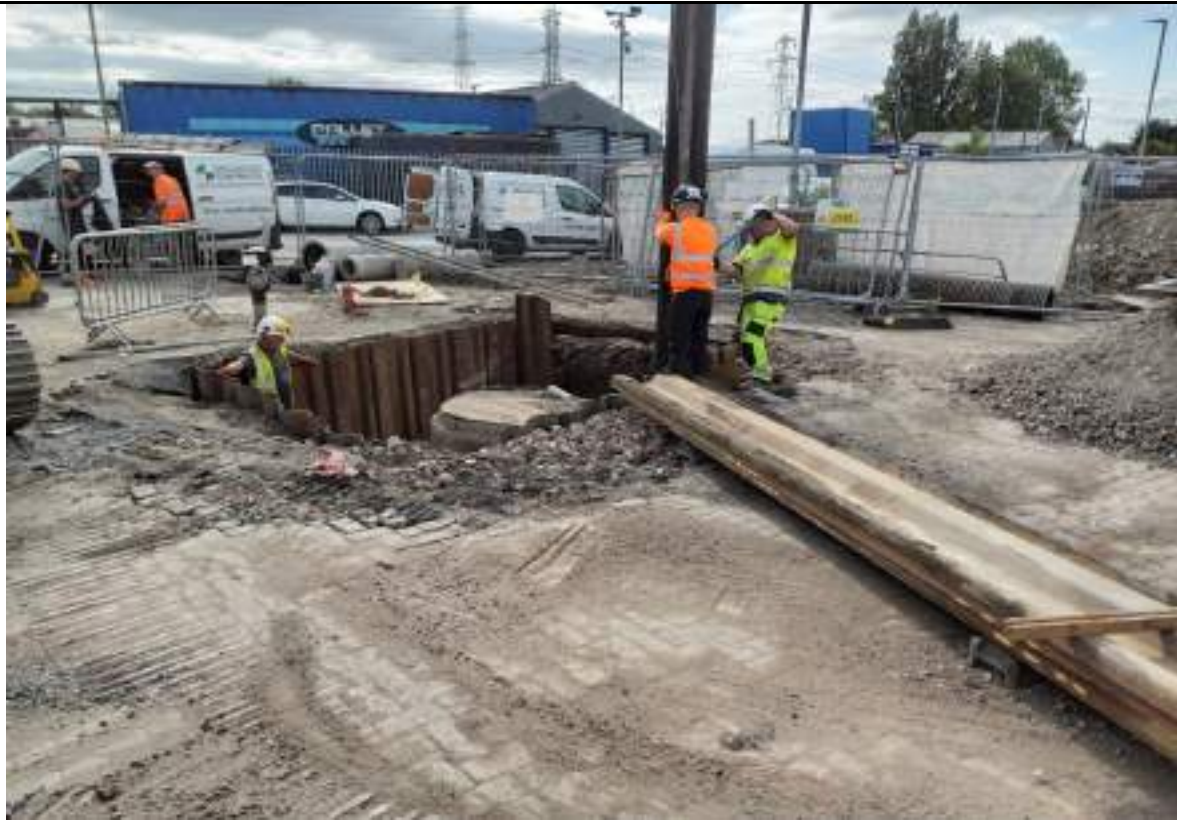
Photograph 9: Removing sheet piles around thrust boring drainage excavation in the southeast.
