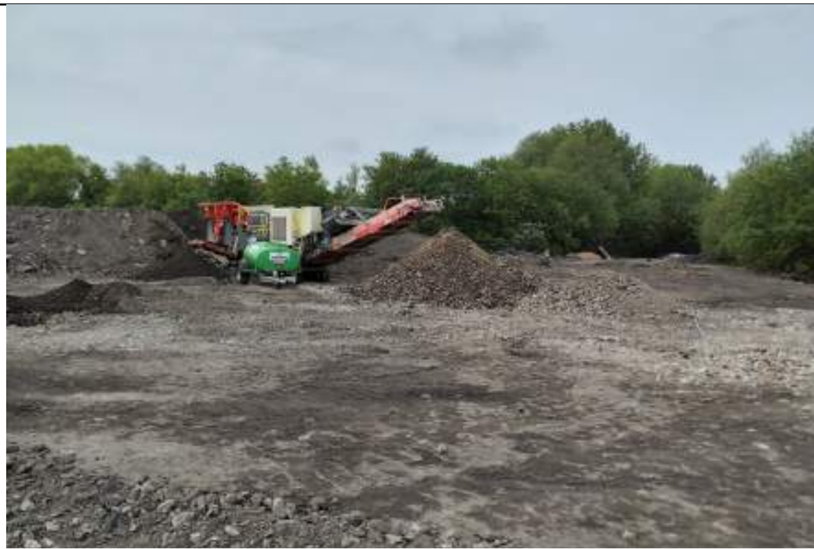
Photograph 10: Crusher and stockpile of oversize and concrete material in the northwest.
