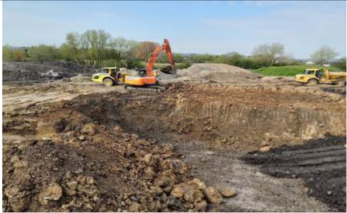
Photograph 7: Excavation of Glacial Till from the borrow pit in the north.
