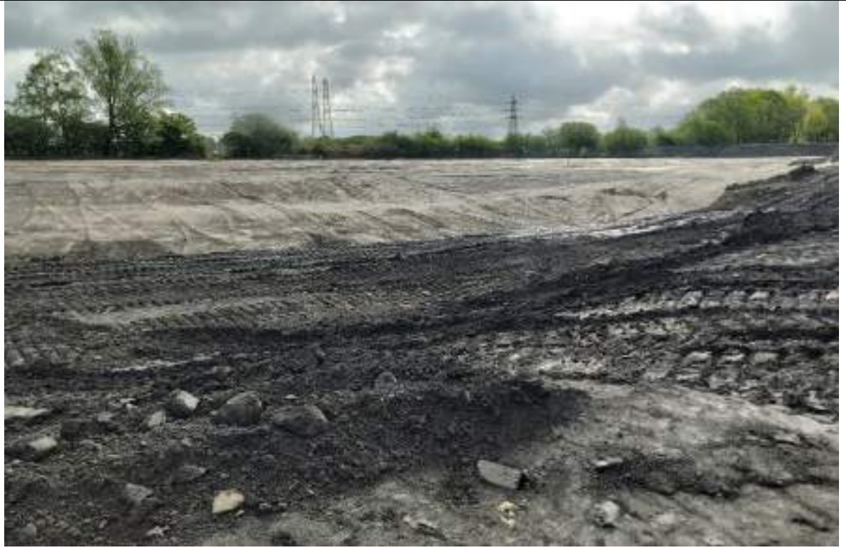
Photograph 7: Placed fill in the northeast.
