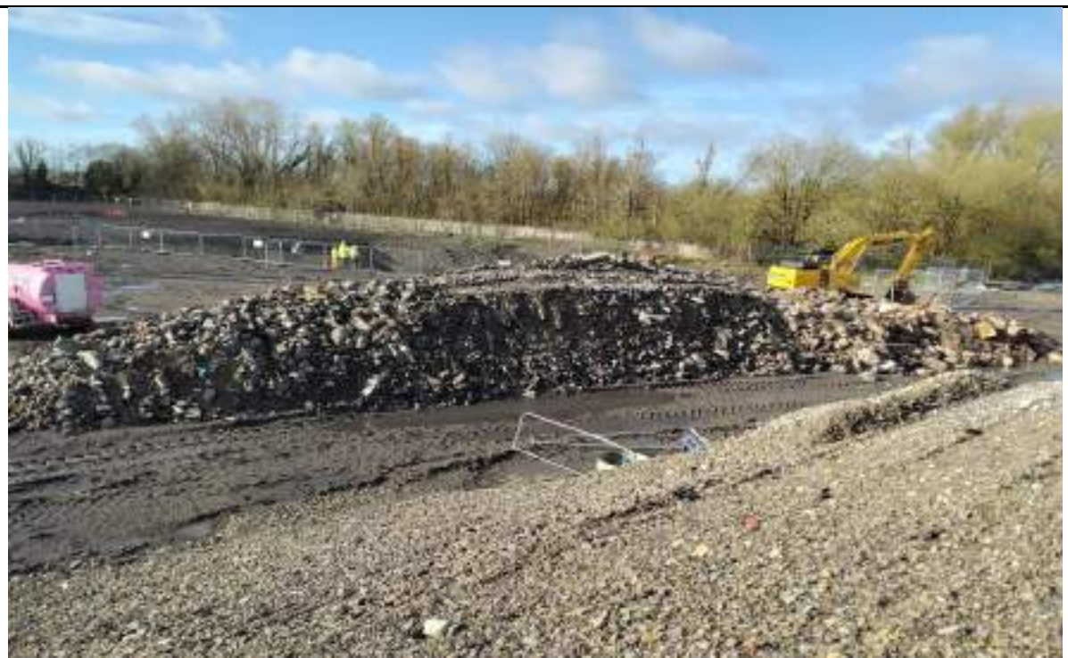
Photograph 8: Stockpile of oversize material in the west. Material to be crushed and processed.
