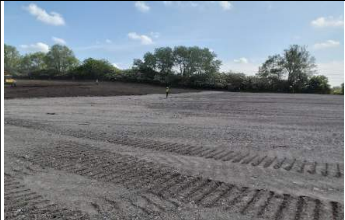
Photograph 7: Site surveying in the northern part of the site.
