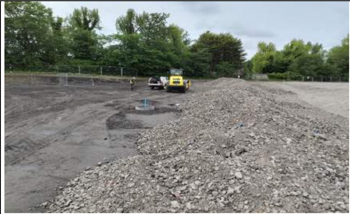
Photograph 5: Plate load testing on final layer of general fill in the south.
