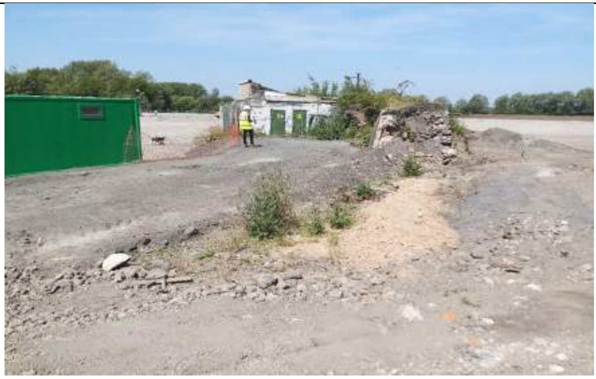
Photograph 10: Grouted shaft no.6 next to electricity transformer in the centre east.
