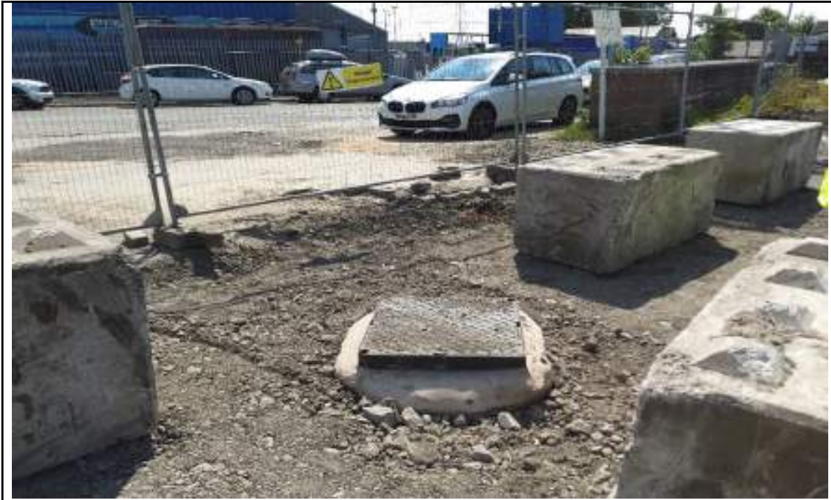
Photograph 5: Drainage manhole in the southeast.
