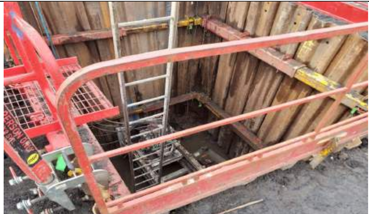
Photograph 14: Preparation of thrust bore drainage for boring in the southeast.
