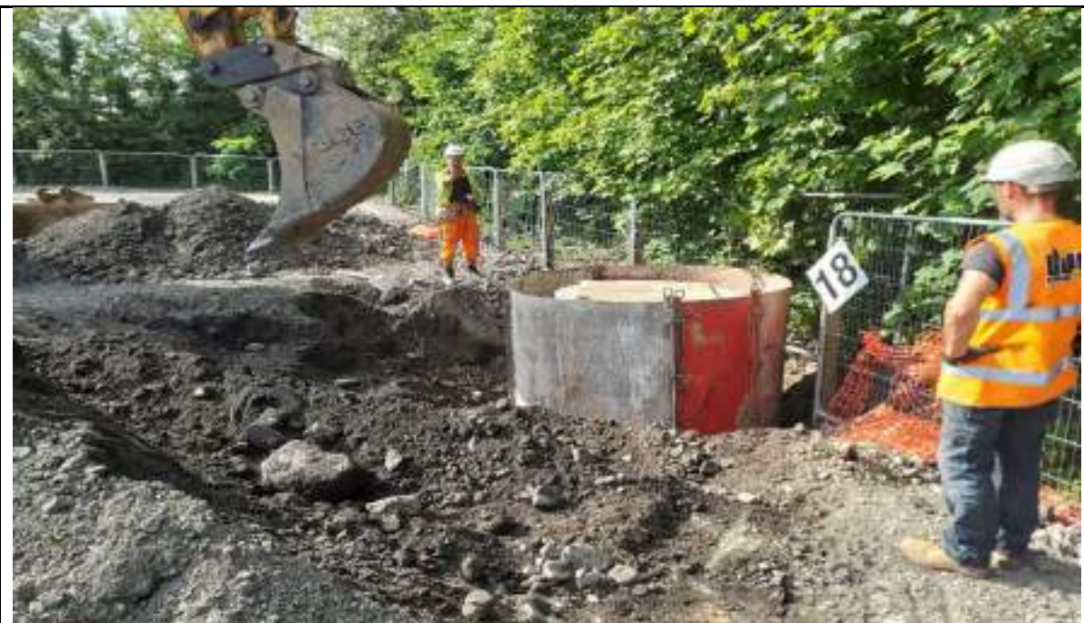
Photograph 2: Backfilling constructed drainage manhole in the southwest. Level raise is necessary for placing drainage manhole.
