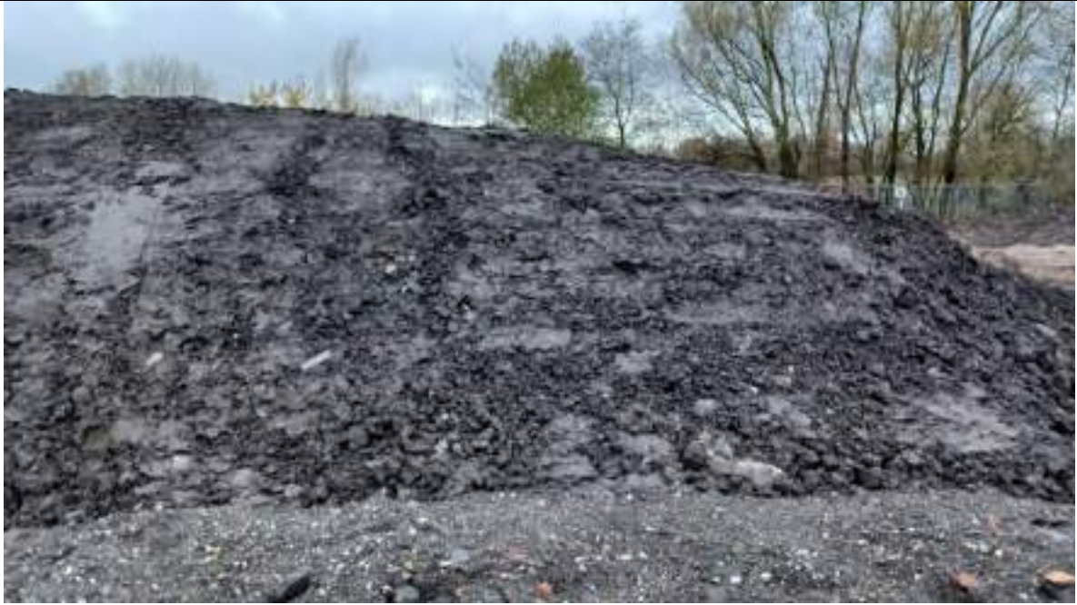
Photograph 7: Organic material stockpiled separately for placement in borrow pit
