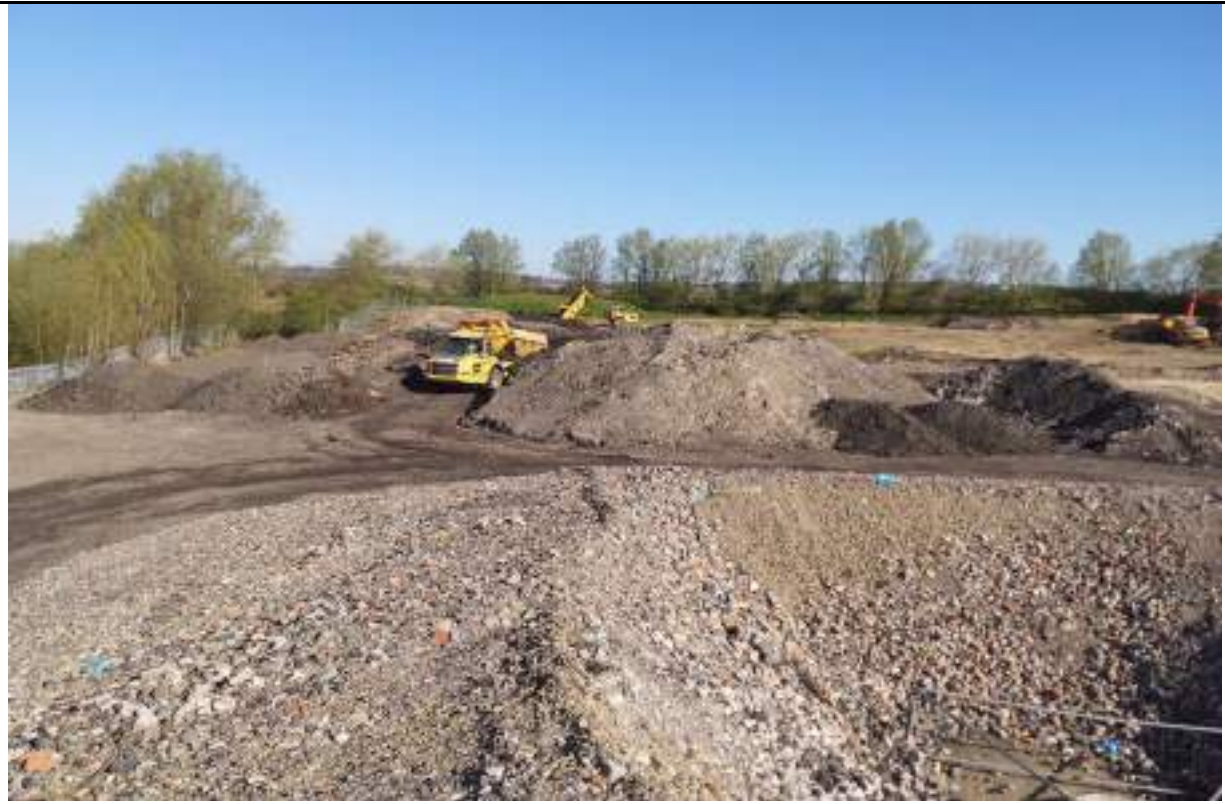
Photograph 5: Stockpiling excavated dark landfill Made Ground and unsuitable material in the northwest. Material from excavation in the north and stockpile of unsuitable material in the northeast.
