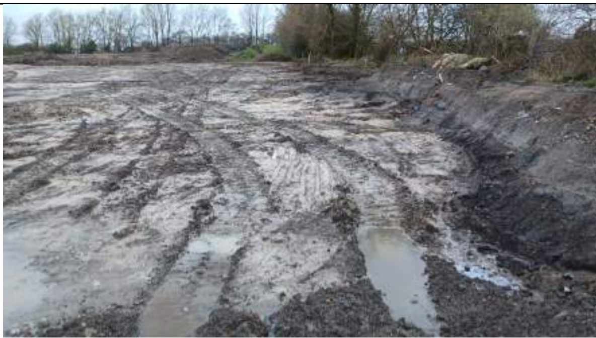
Photograph 6: Natural soils exposed at surface during over-dig.
