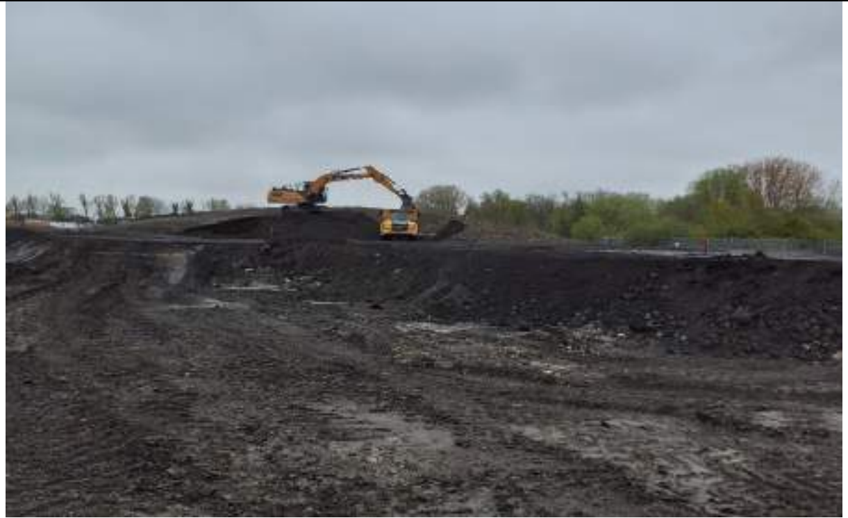
Photograph 9: Removing 6F2 material for capping the eastern part of the site.
