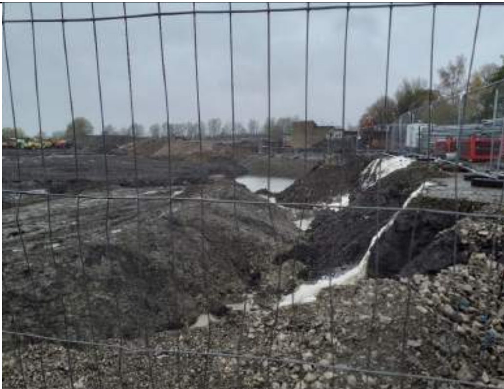
Photograph 18: Standing water in the southeast.
