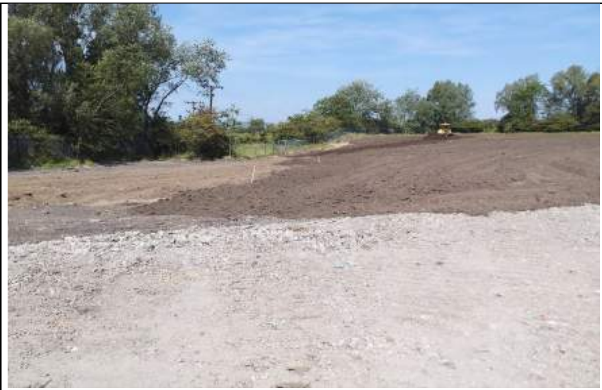
Photograph 8: Placing topsoil in the northwest of POS area.
