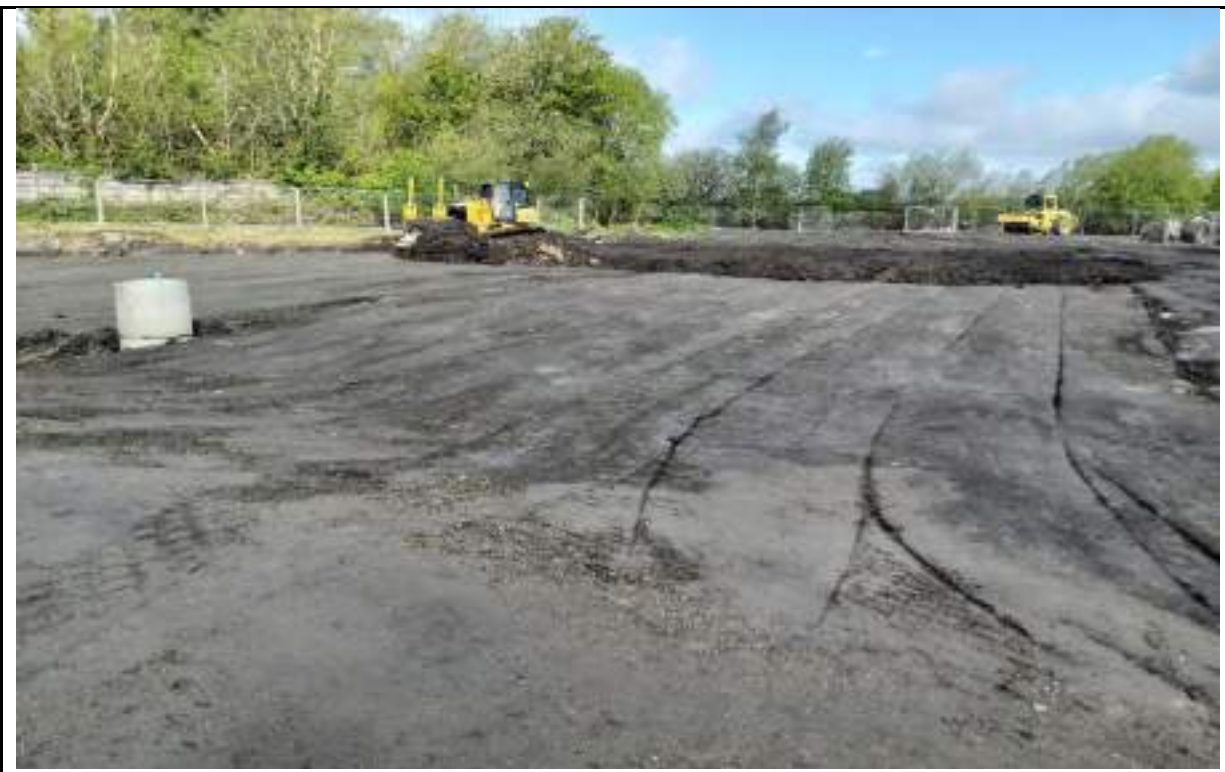
Photograph 4: Placing fill in the western boundary. Material from excavation of landfill Made Ground in the east.
