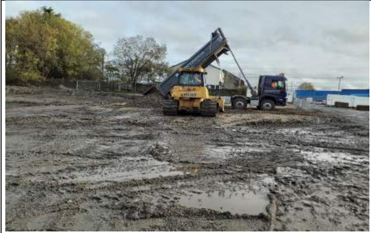
Photograph 5: Importing 6F5 material for backfilling of excavation in the location of shaft no.7.
