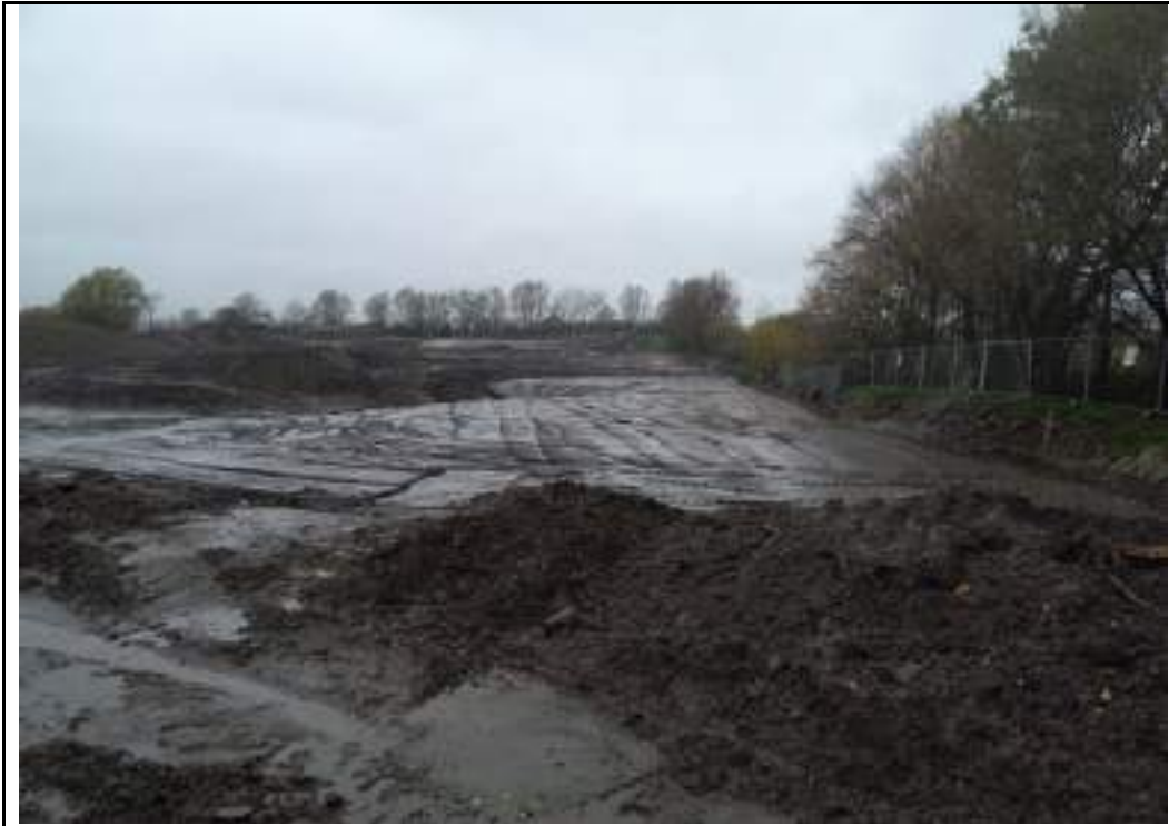
Photograph 1: Overview of eastern part of the site. Looking towards the north.
