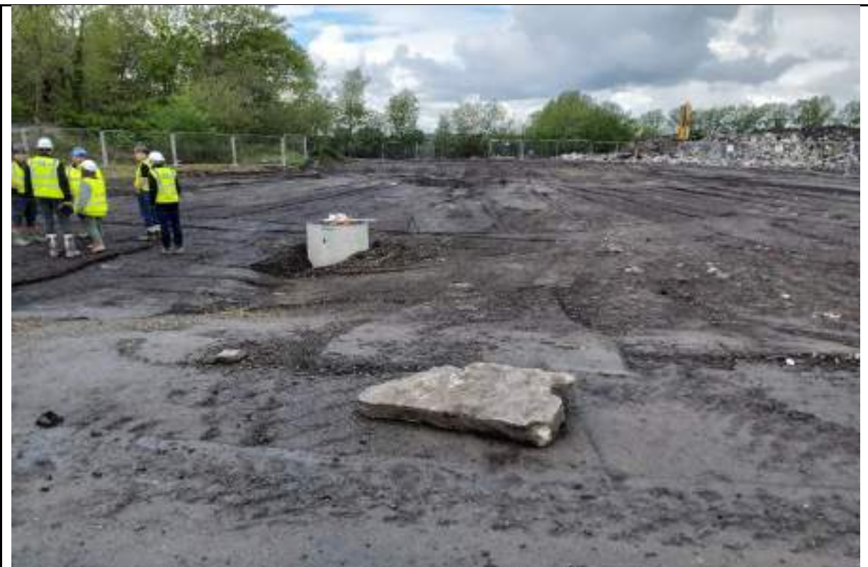
Photograph 4: Placed fill in the west. One more layer to be placed before capping.
