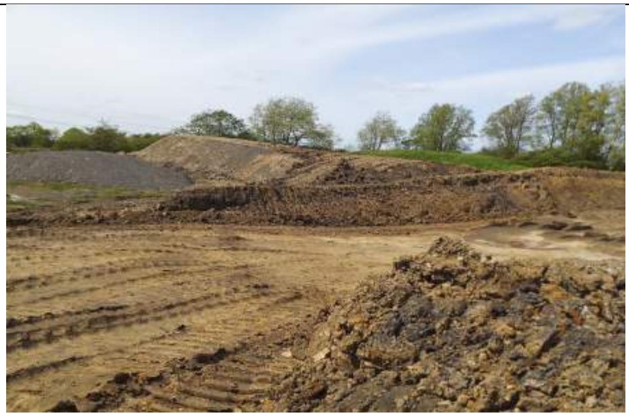
Photograph 8: Stockpiles of topsoil and unsuitable material in the northwest.
