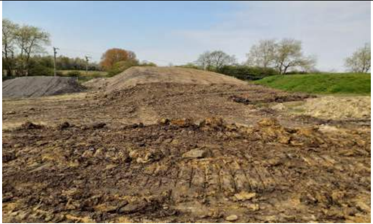
Photograph 11: Stockpiles of topsoil and unsuitable materials in the northwest.
