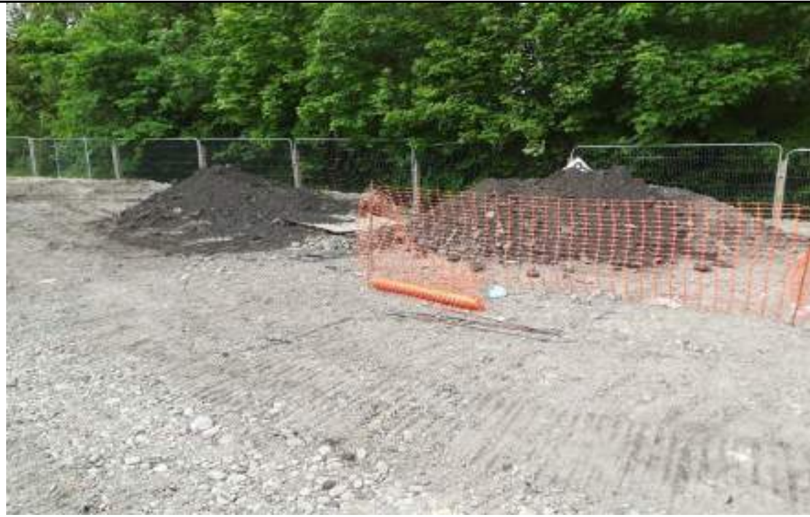
Photograph 9: Excavation for construction of manhole drainage in the southwest.
