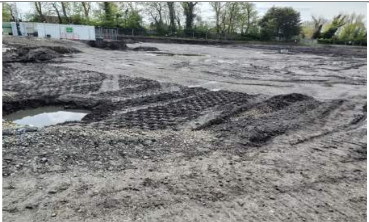
Photograph 16: Trial pits for groundwater monitoring in the southeast. Three trial pits in the centre south are filled with water.
