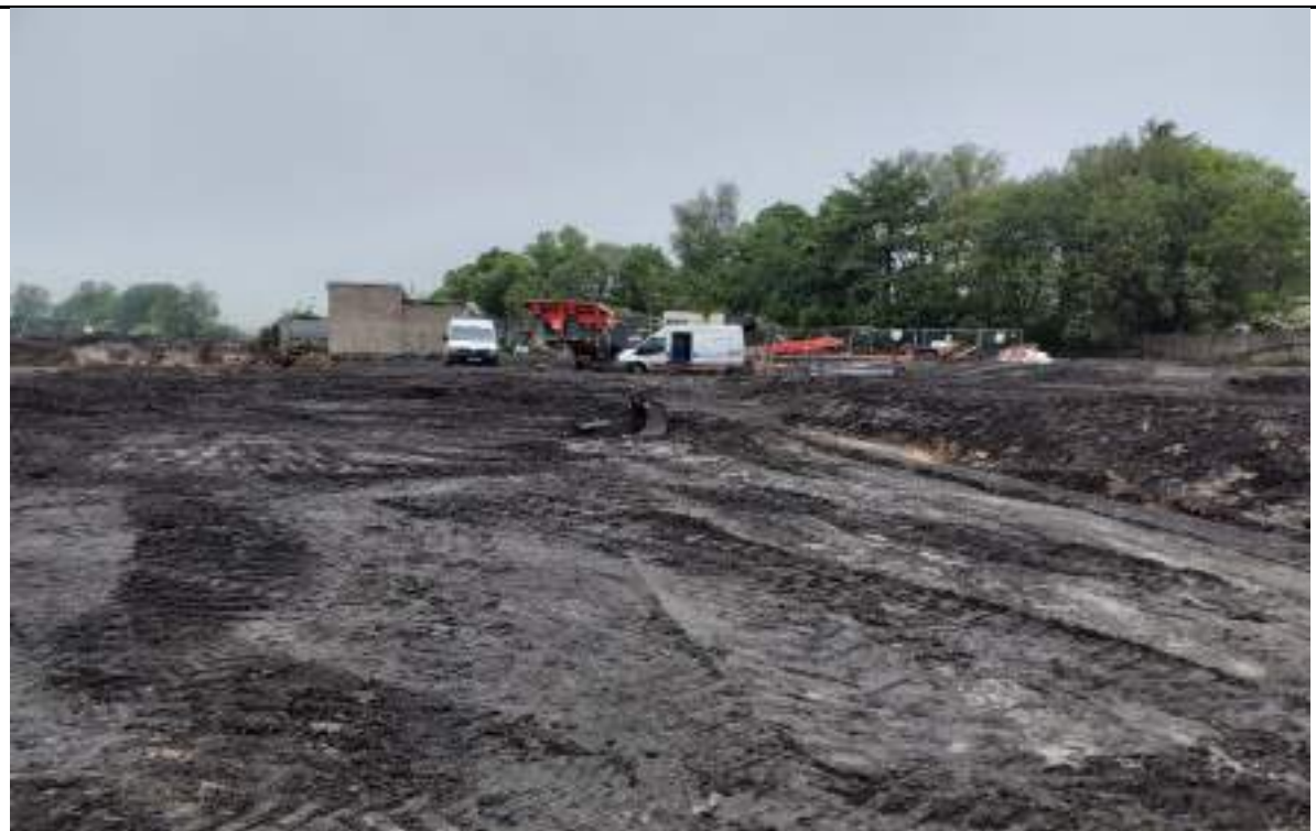
Photograph 2: Crusher is being prepared in the southeast.
