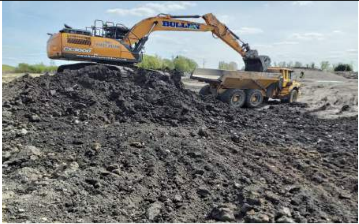
Photograph 5: Removal of peat stockpile to backfill the borrow pit.
