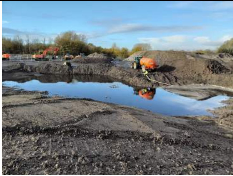
Photograph 5: Dewatering excavation in the northeast.
