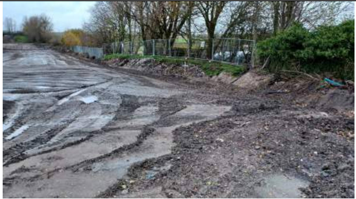
Photograph 3: Eastern boundary of the site. Looking towards the north. Boundary checks required by VHE
