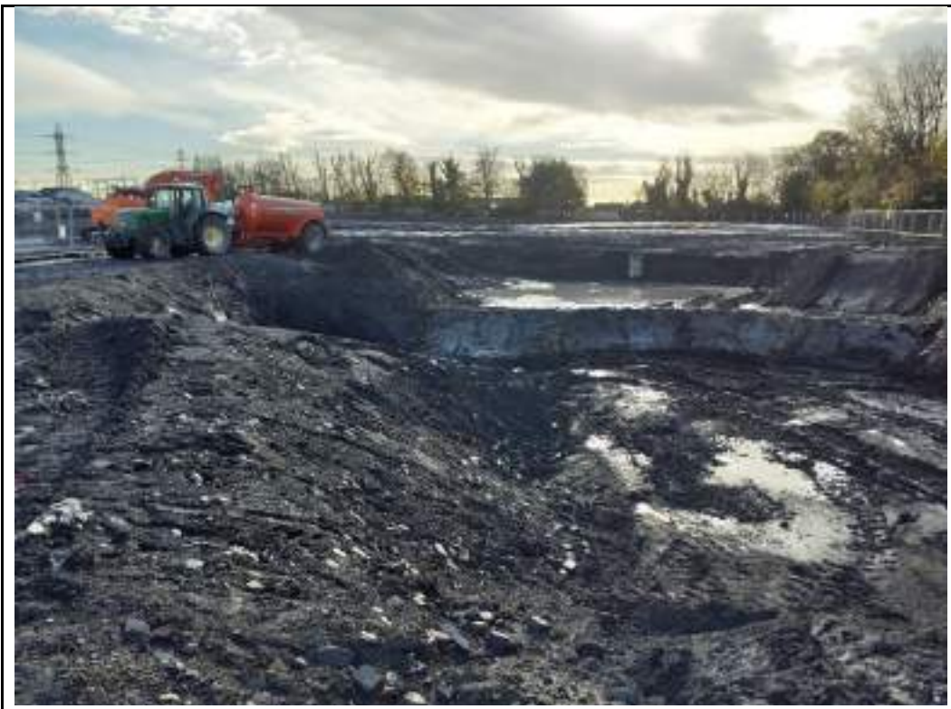
Photograph 14: Discharging water in excavation in the western boundary of site. Water pumped from excavation in the northeast.
