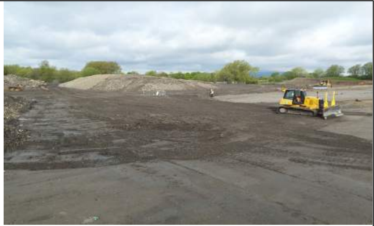
Photograph 13: Surveying the site in the centre north.
