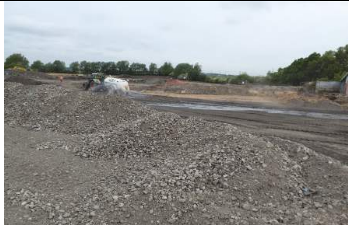
Photograph 113: Dust suppression unit controlling dust on site.
