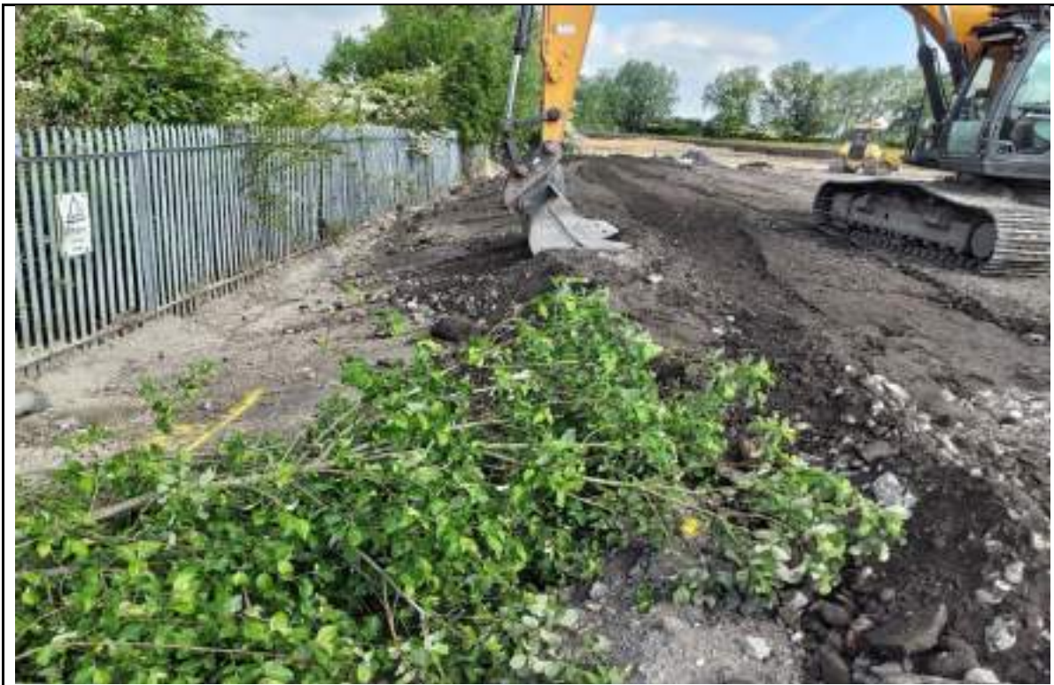
Photograph 6: Rectifying boundary dispute in the northwestern boundary. Re-excavation and refilling are undertaken.
