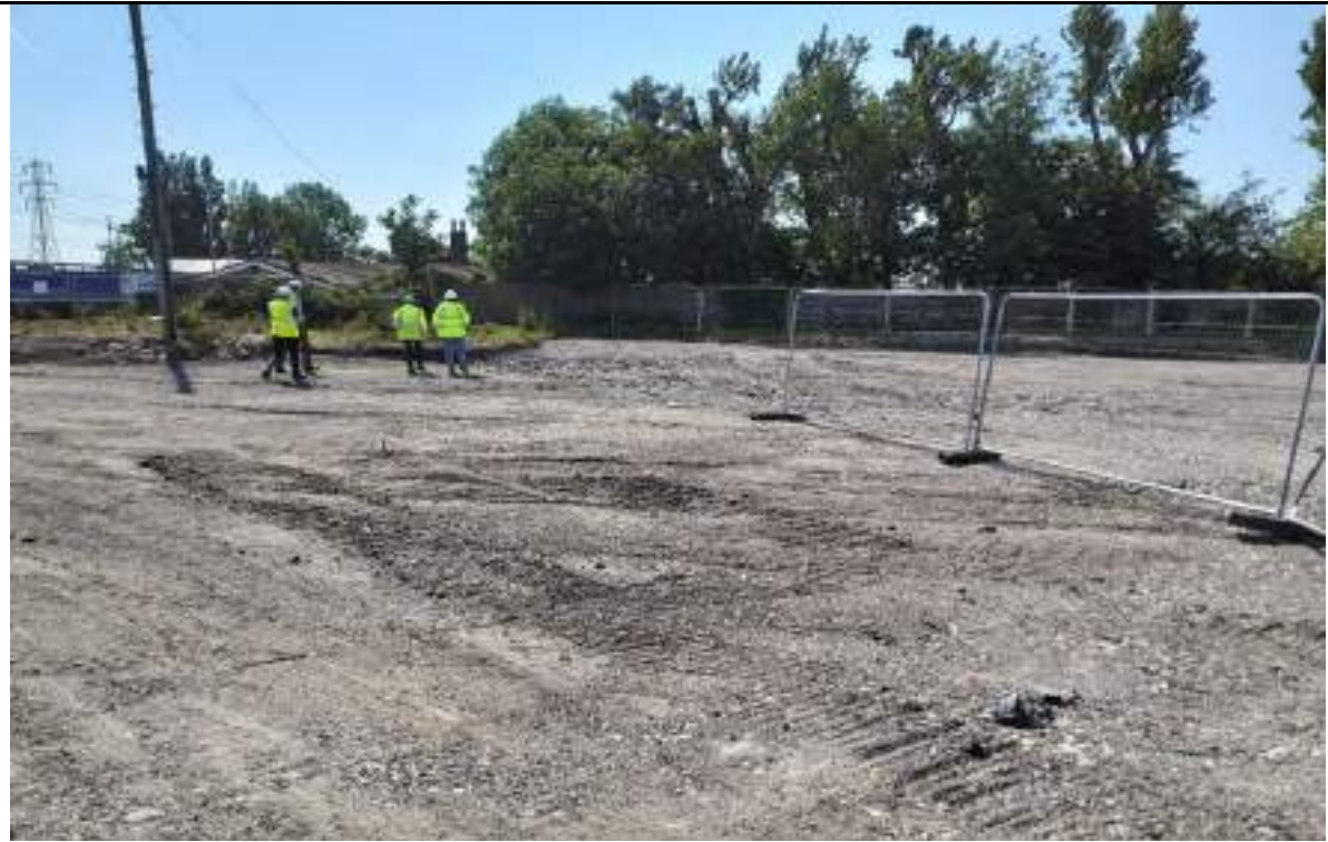
Photograph 1: Running layer placed in the southeast, near location of shaft no.8 and the main gate area.
