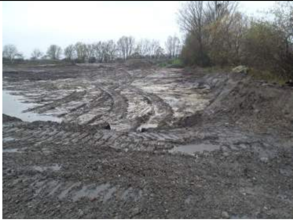
Photograph 5: Excavation in the northeast.
