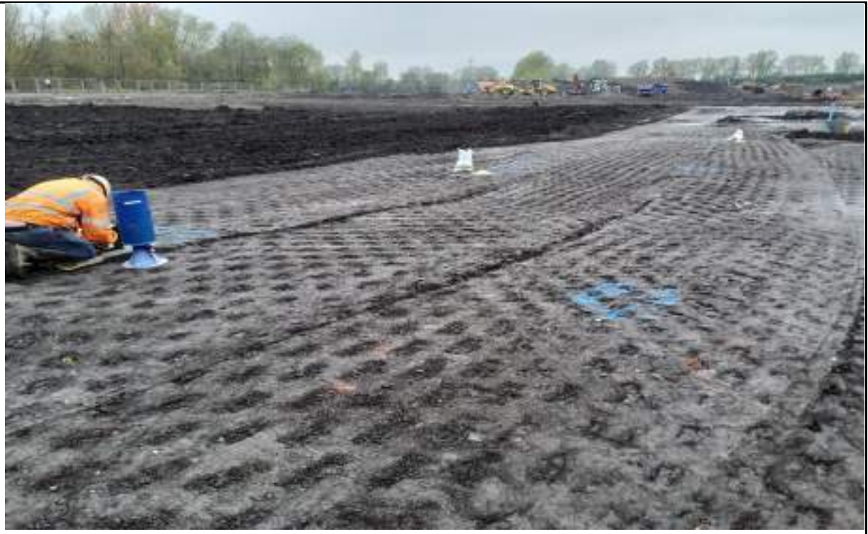
Photograph 2: Sand Replacement Density test on placed fill in the south.
