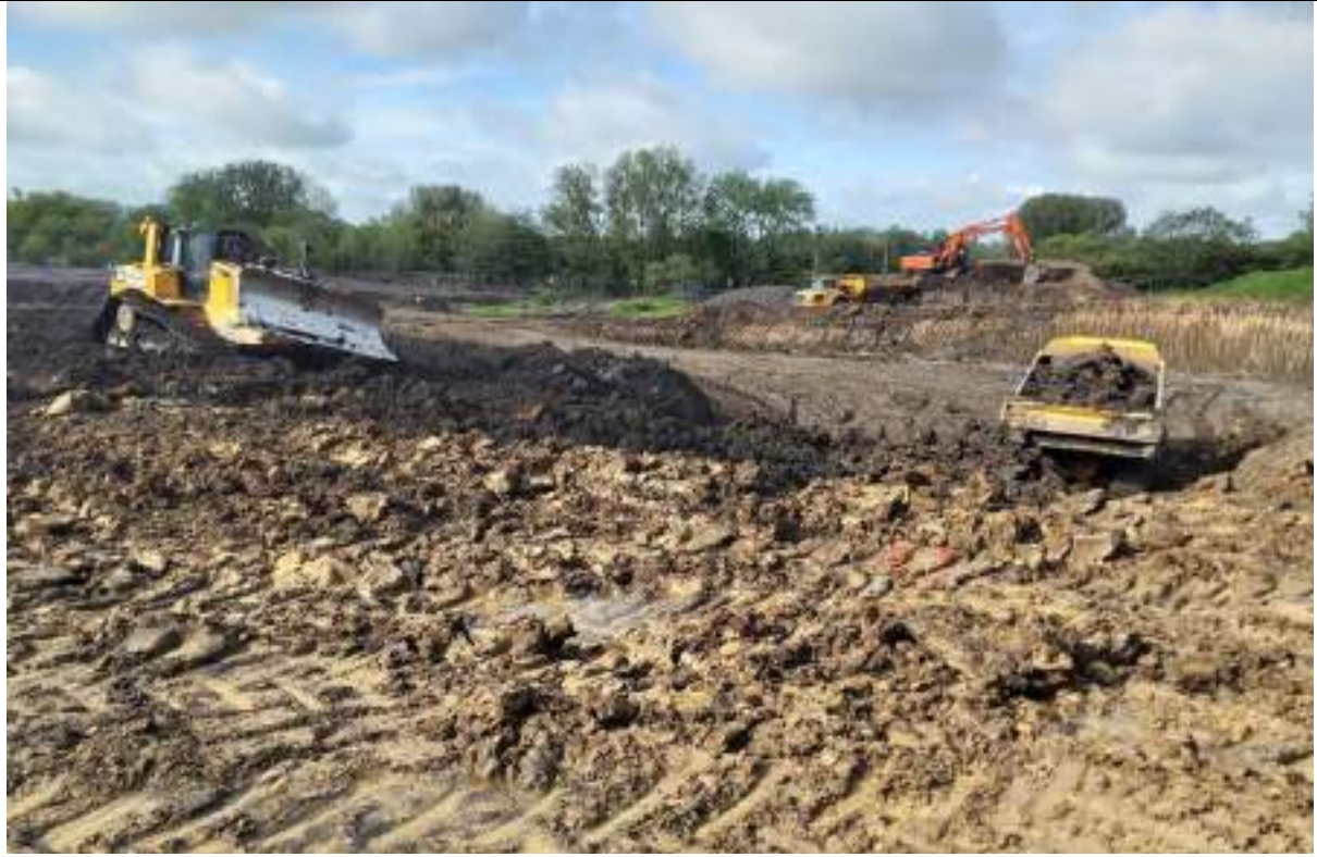
Photograph 9: Backfilling the borrow pit in the north.
