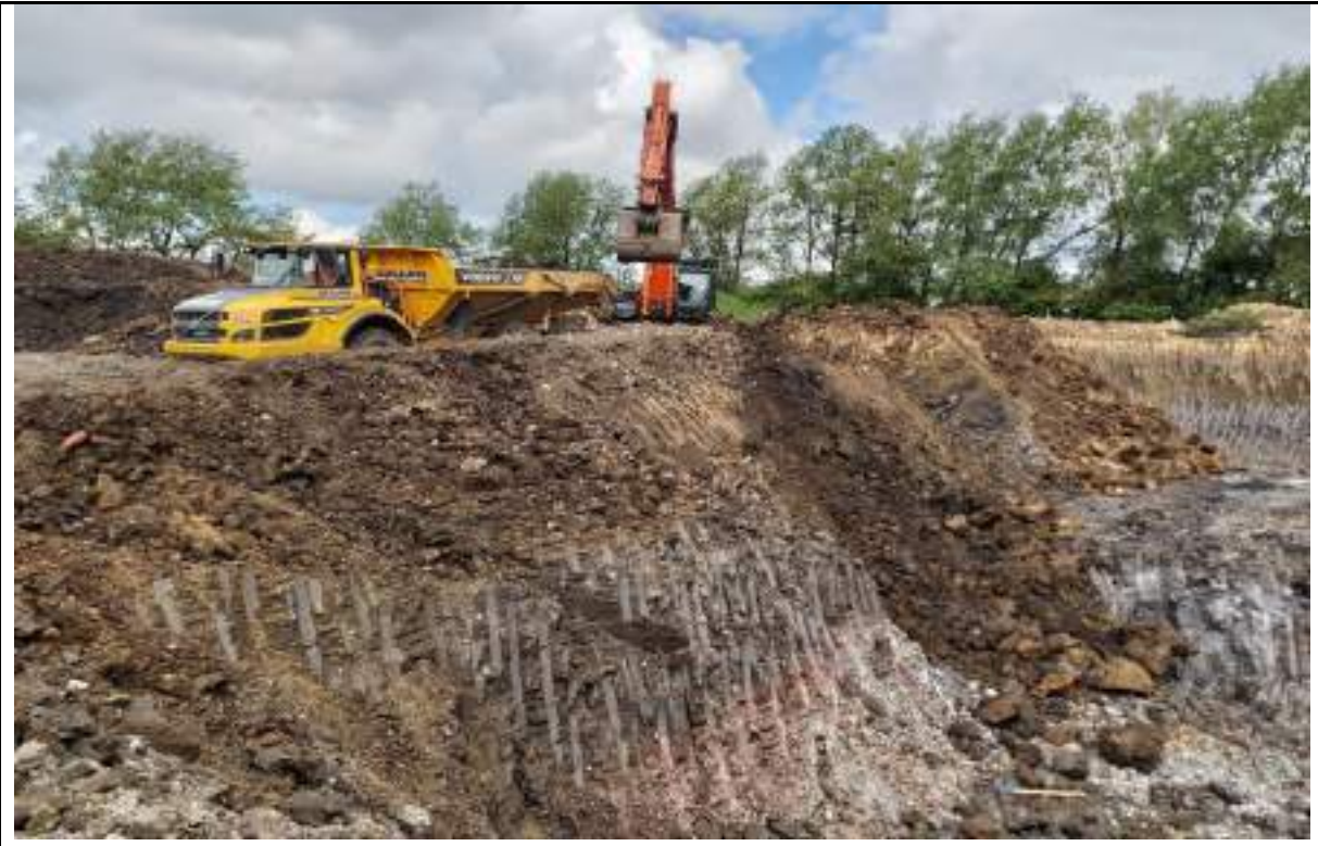
Photograph 7: Excavation of Glacial Till from the borrow pit in the north.
