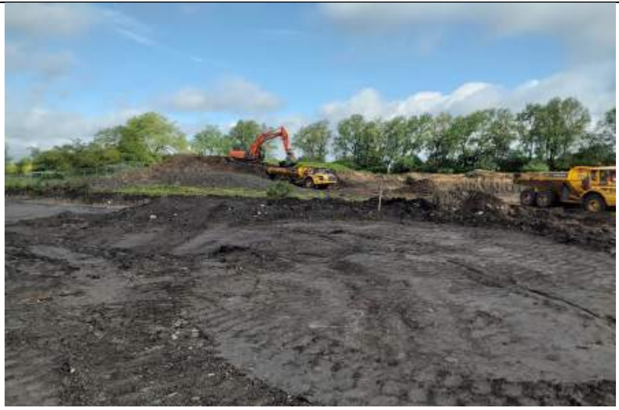
Photograph 6: Removing stockpile of unsuitable material to the borrow pit.
