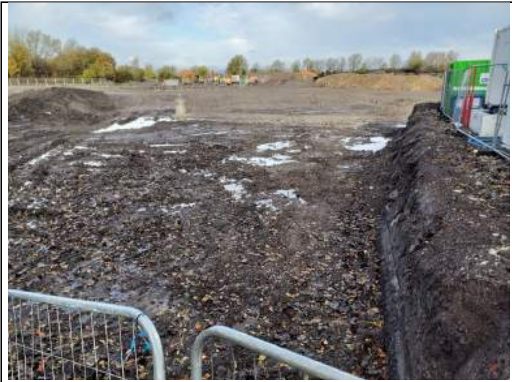
Photograph 14: Backfilled area in southern part of the site.
