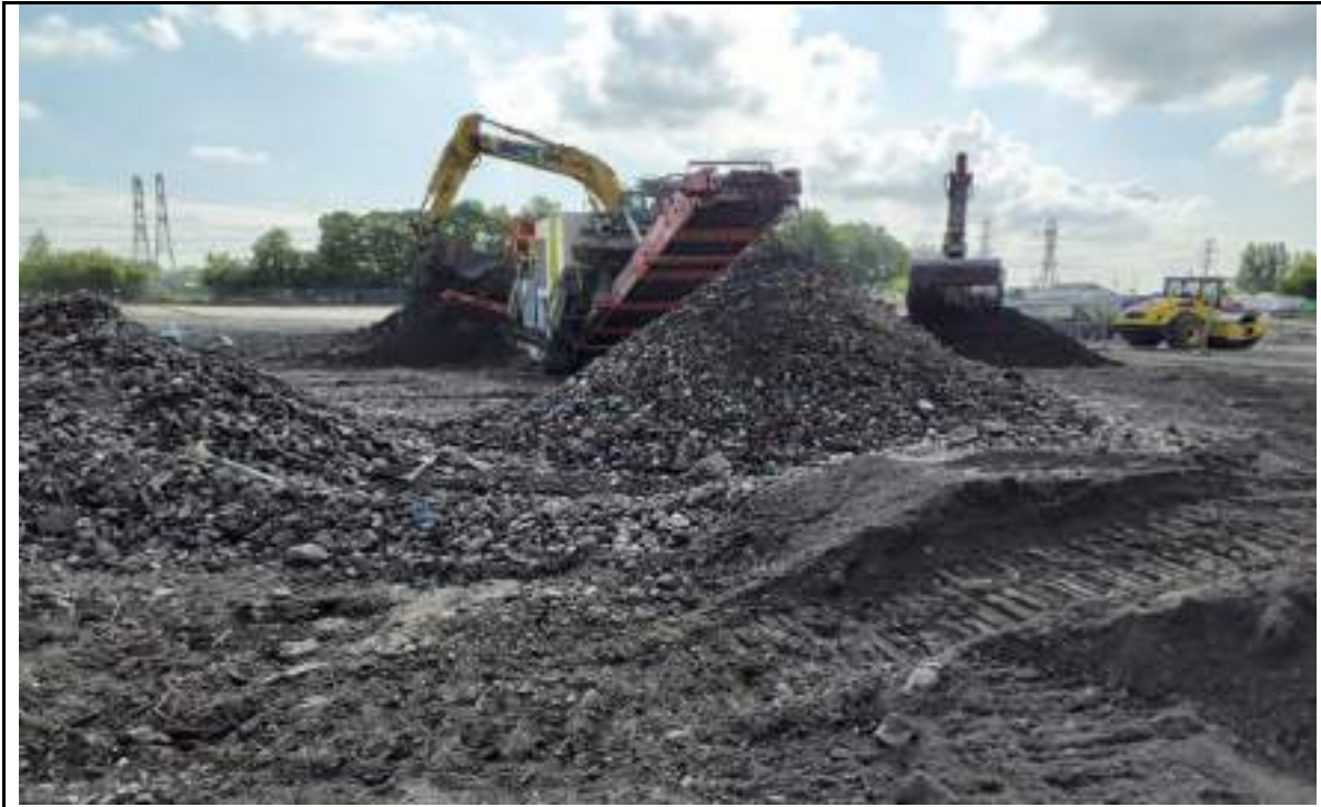
Photograph 5: Crushing stockpile of oversize and concrete materials in the northwest.
