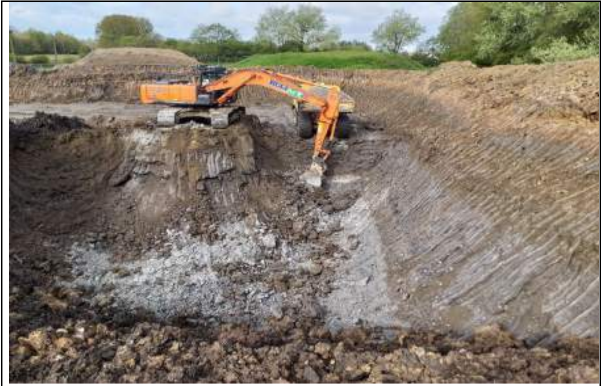
Photograph 7: Excavation of mudstone from the borrow pit in the north.
