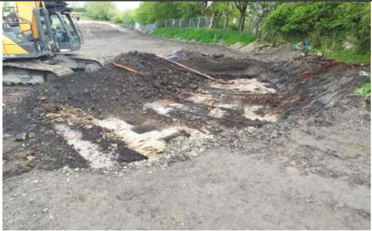
Photograph 1: Excavation of landfill Made Ground in the eastern boundary. Base of excavation is glacial till.
