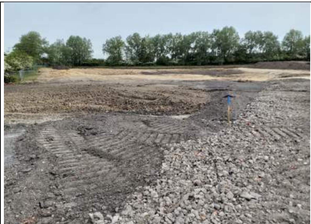
Photograph 6: The northwestern part of POS area still needs filling to reach final level.
