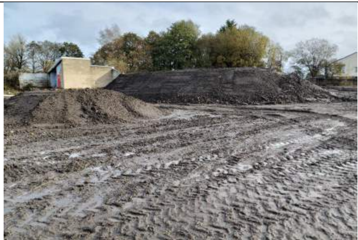
Photograph 4: Stockpile of wet unsuitable material in the southeast.
