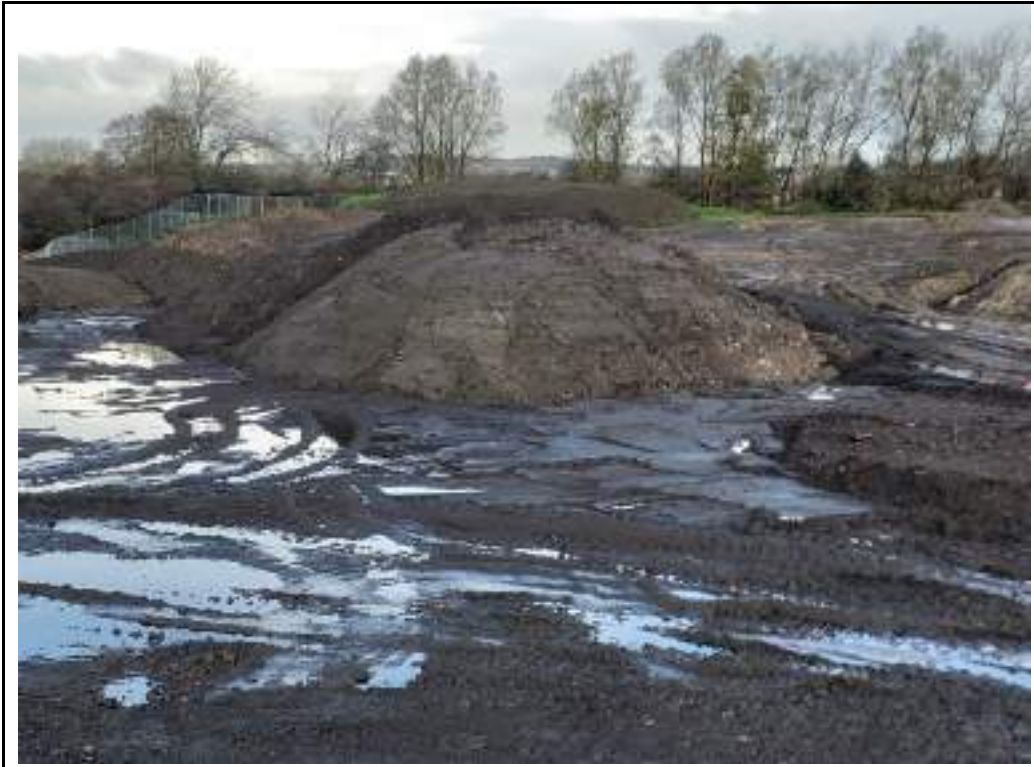
Photograph 9: Stockpile of peat materials in the northwest excavated from the northeastern part of the site.
