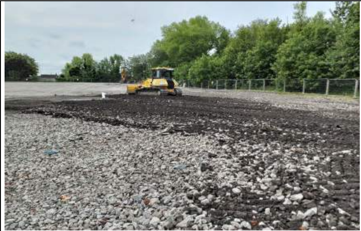
Photograph 3: Placing and levelling 6f2 material in the west.
