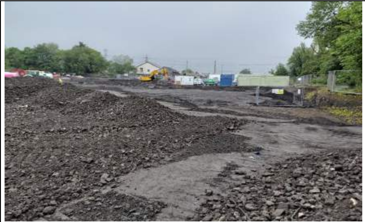
Photograph 3: Southern boundary of the site. Looking towards the east. A layer of fill to be placed to reach to the FGL.
