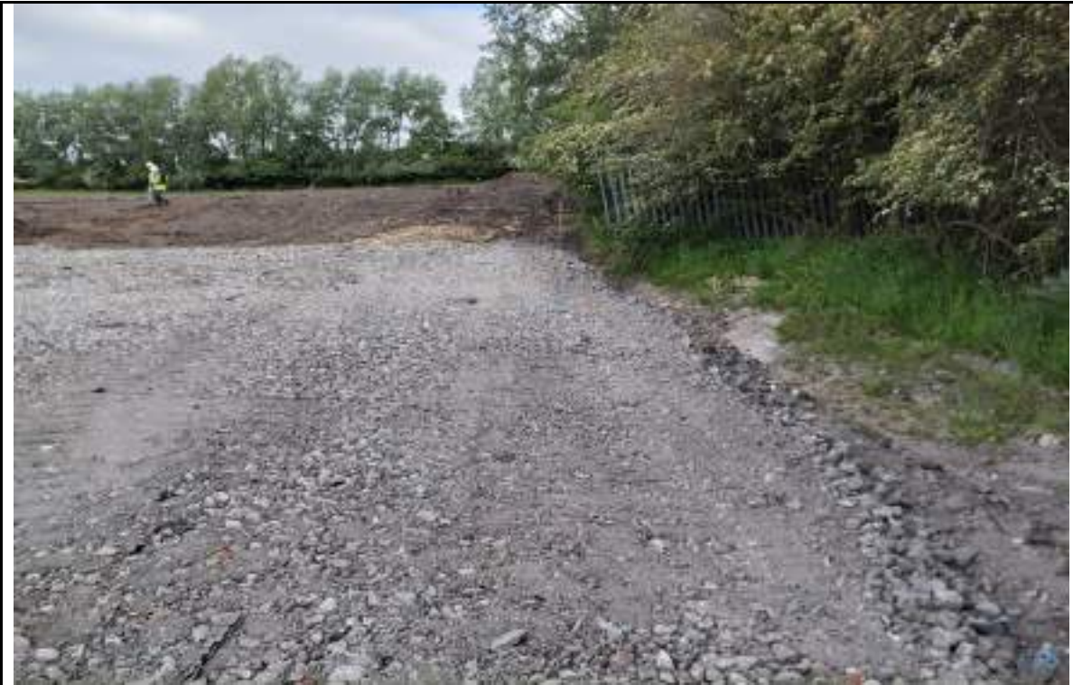
Photograph 7: The northeastern boundary of the site. Looking towards the north.
