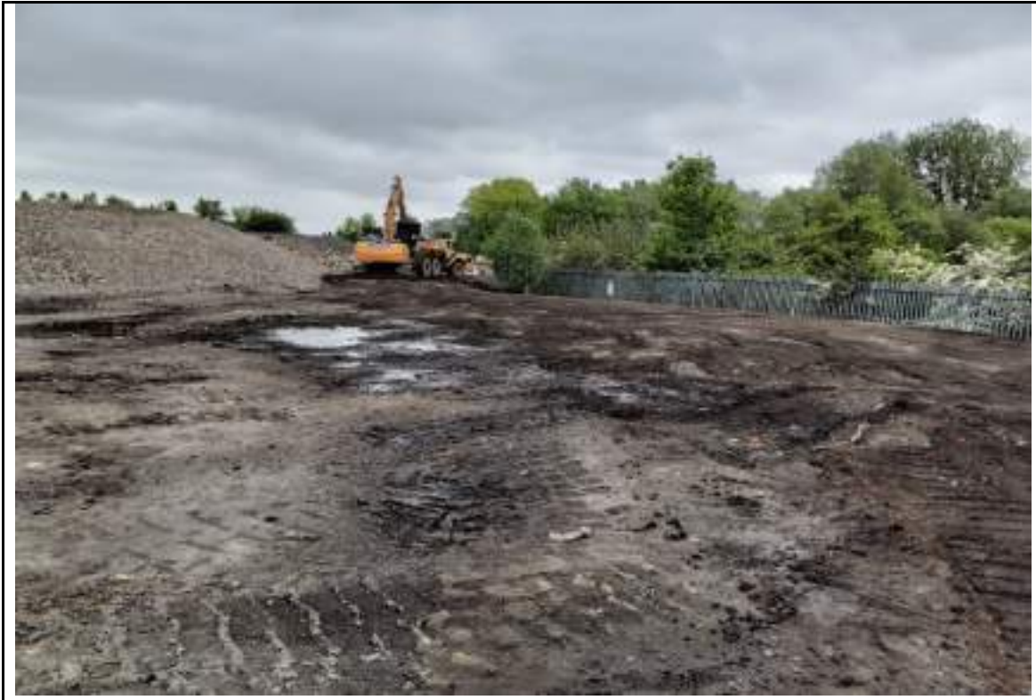
Photograph 7: Trimming of placed fill in the northwest.
