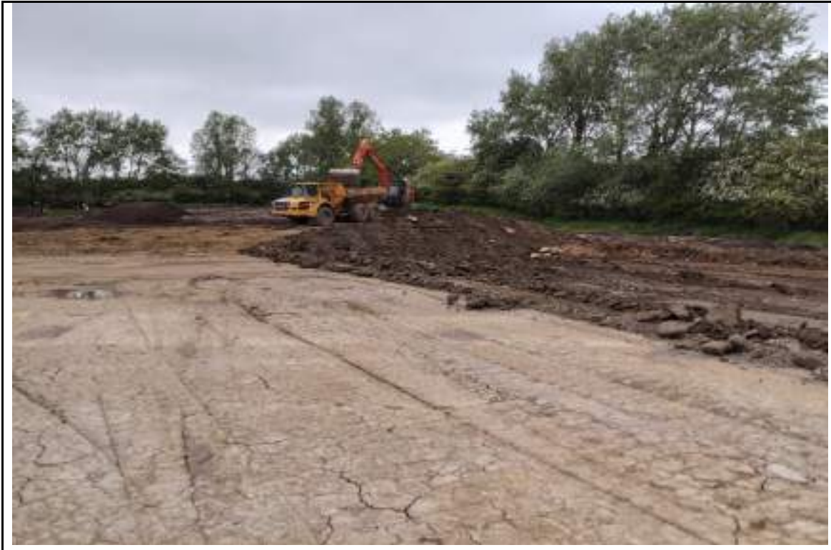
Photograph 5: Removing stockpiled low strength Glacial till to backfill the borrow pit.
