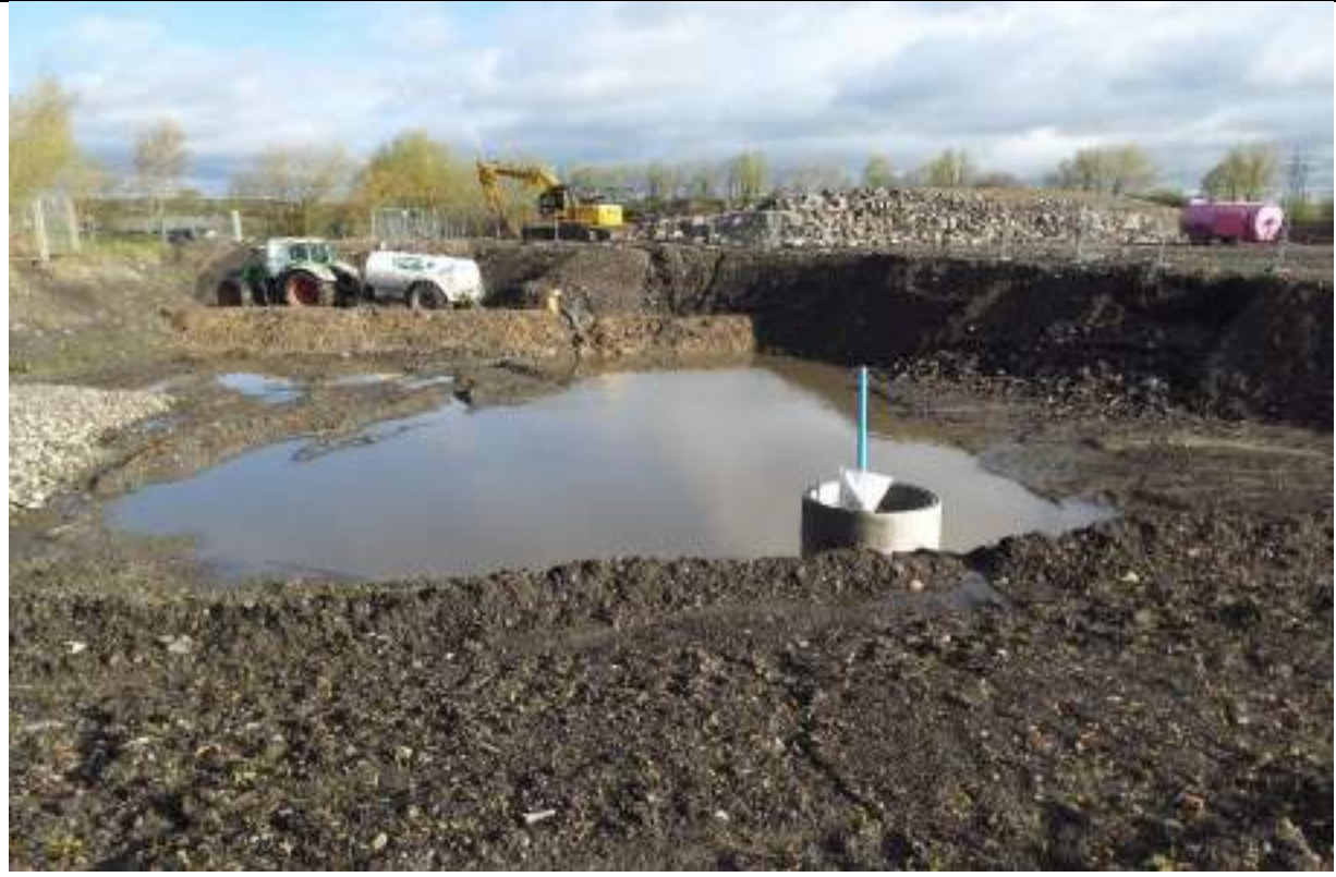
Photograph 9: Pumping standing water near abstraction well in the west.
