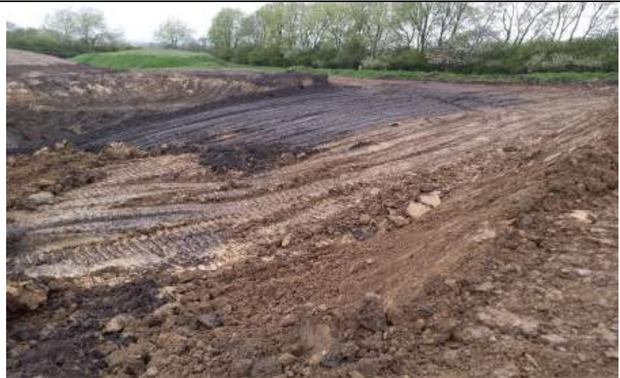
Photograph 11: The eastern part of the borrow pit backfilled with peat (from peat stockpile) and low strength Glacial Till (from borrow pit excavation).
