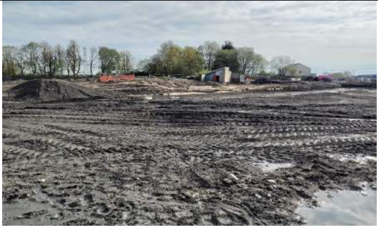
Photograph 13: Stockpile of yellow unsuitable Glacial Till moved to the borrow pit.
