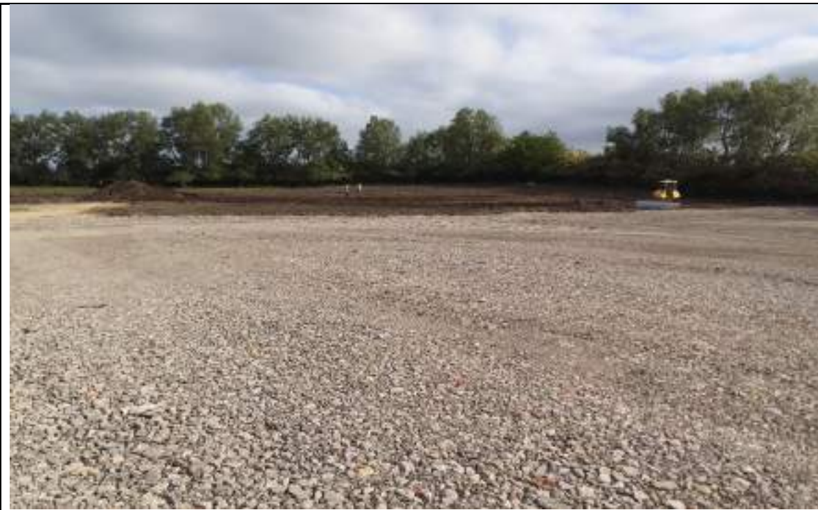
Photograph 4: Placing and levelling topsoil in the POS in the north. Surveyors are controlling levels.
