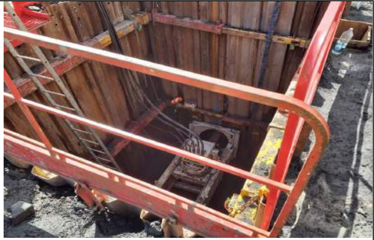
Photograph 11: Boring of thrust bore drainage in the southeast.
