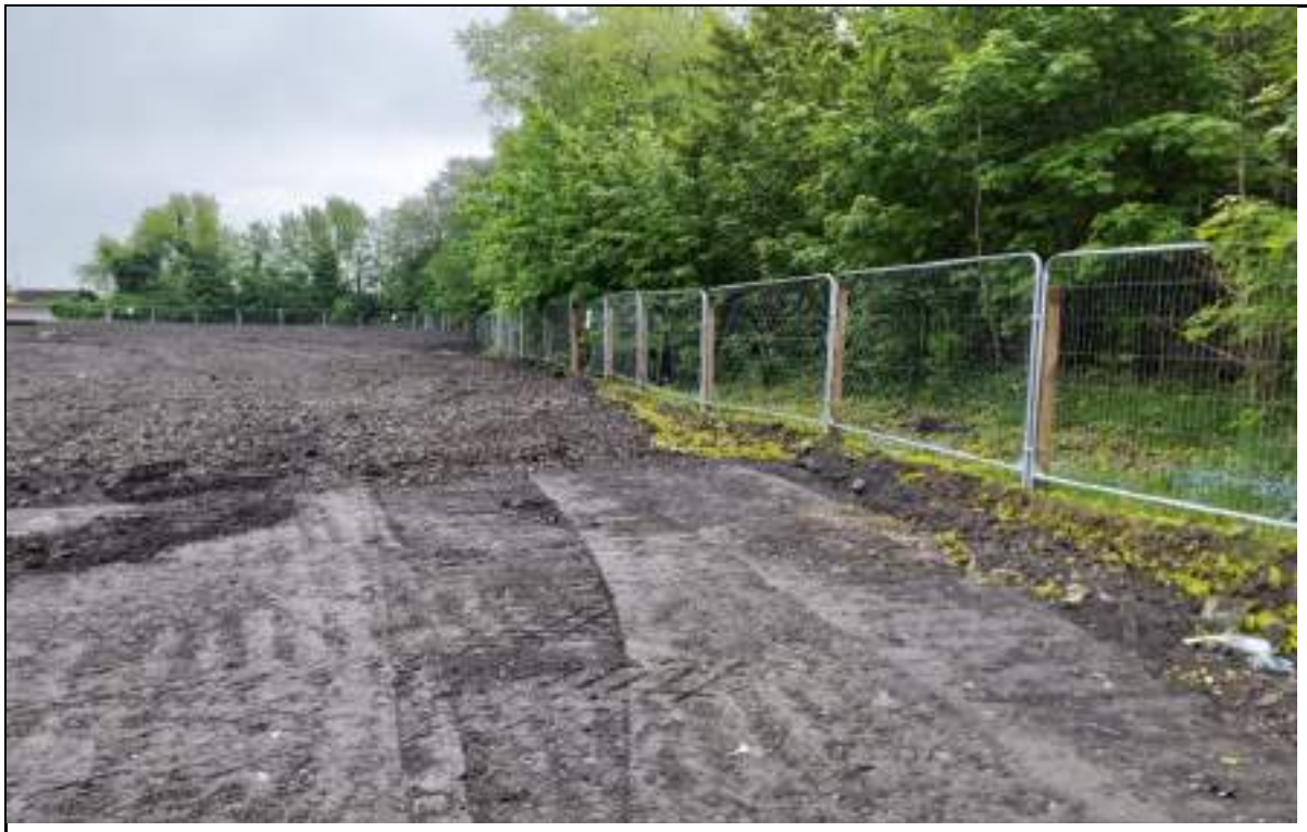
Photograph 4: Capping in the southwestern part of the site.
