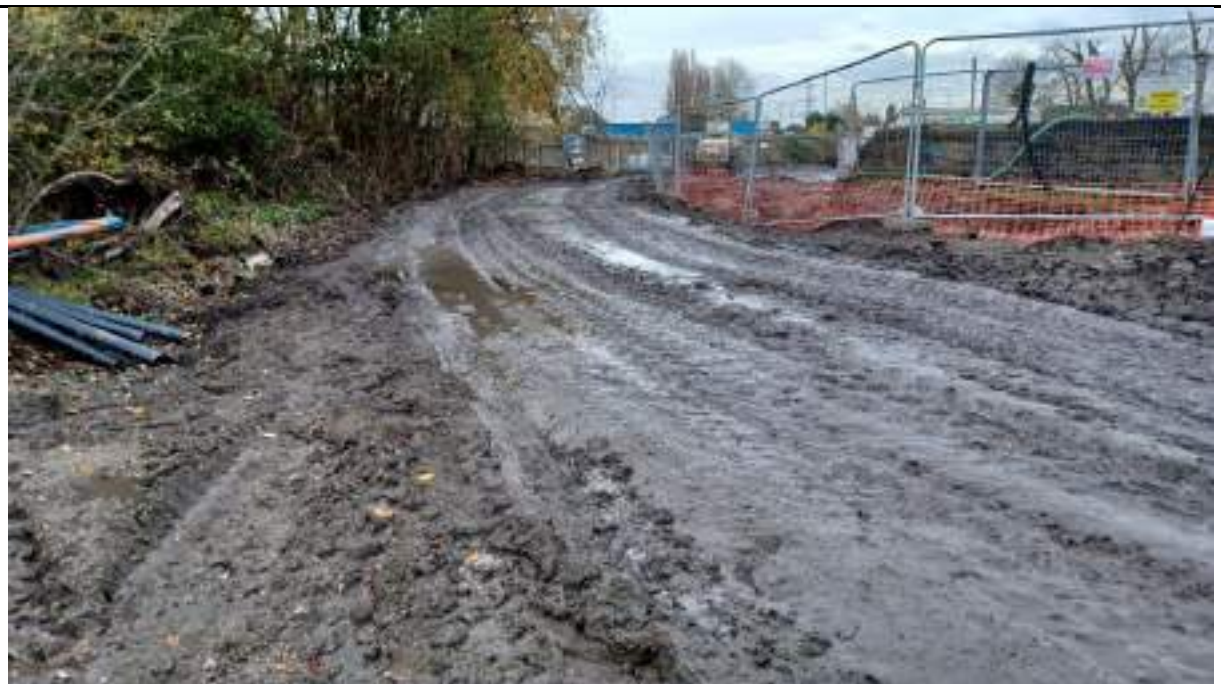
Photograph 2: Raised area behind retaining wall – VHE propose to leave some of the area in place
