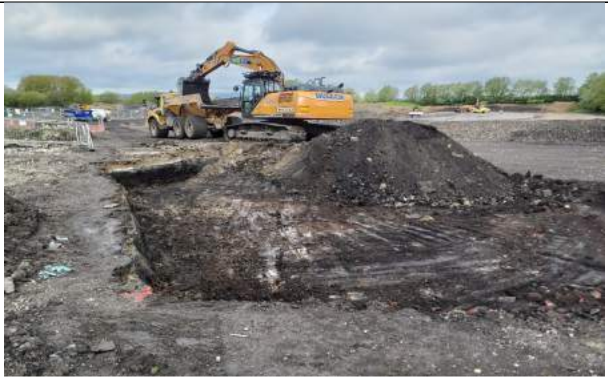
Photograph 2: Excavation of landfill Made Ground in the eastern boundary.
