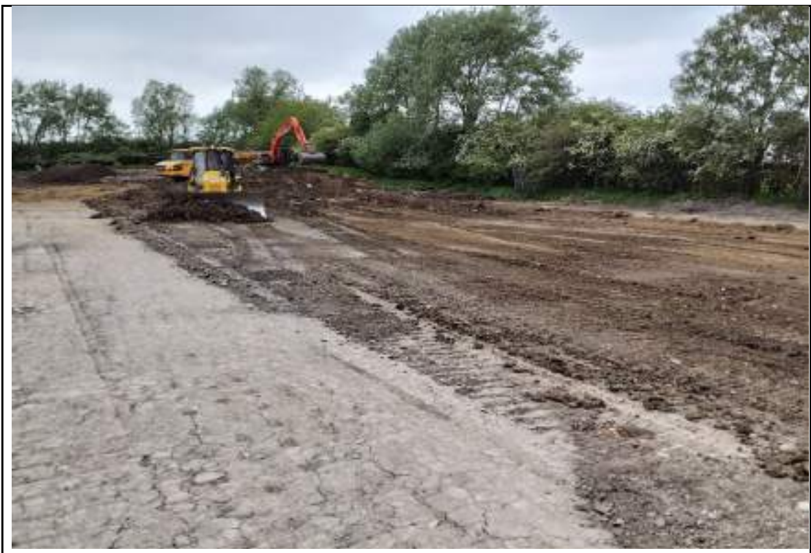
Photograph 4: Trimming of placed fill in the northeast by dozer equipped with GPS.
