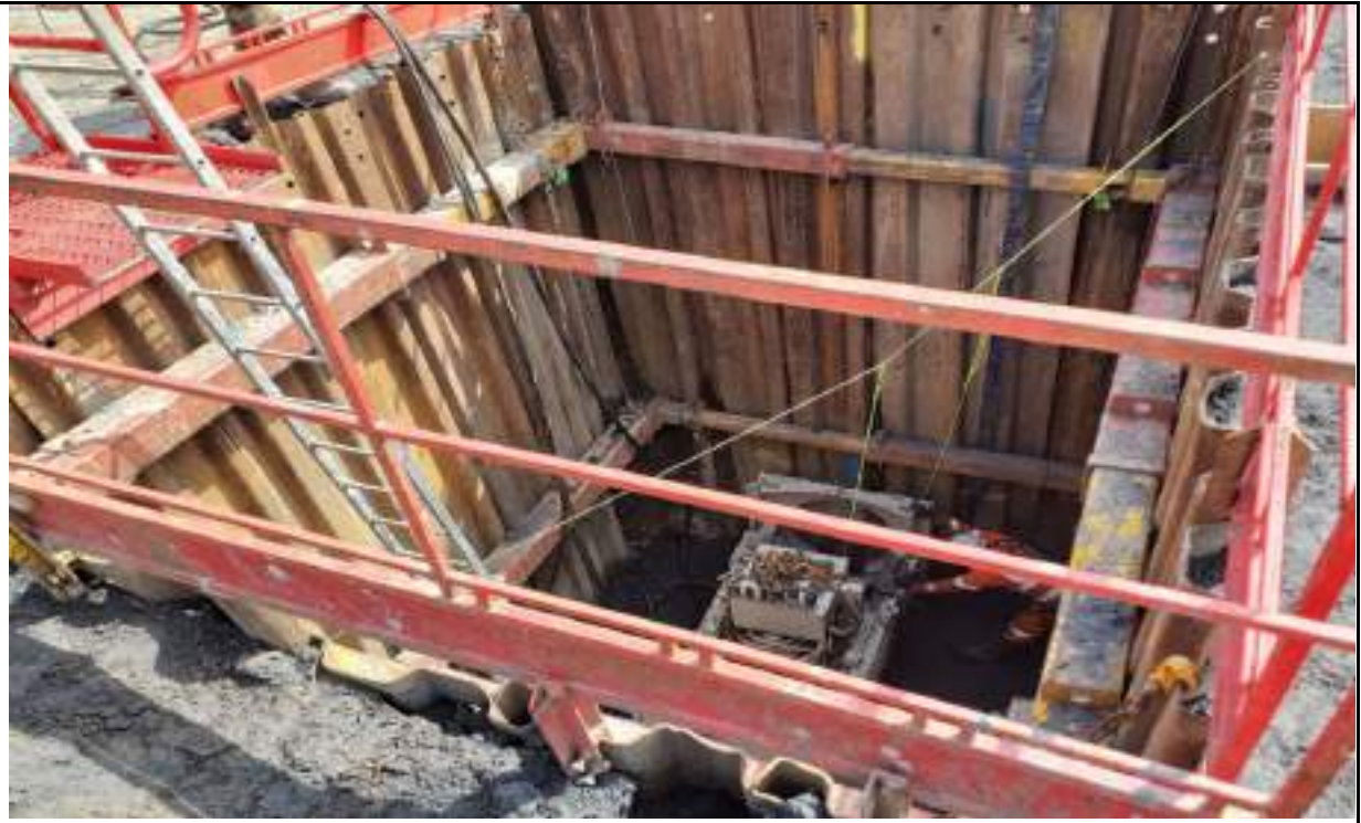
Photograph 16: Preparation of thrust bore drainage for boring in the southeast.
