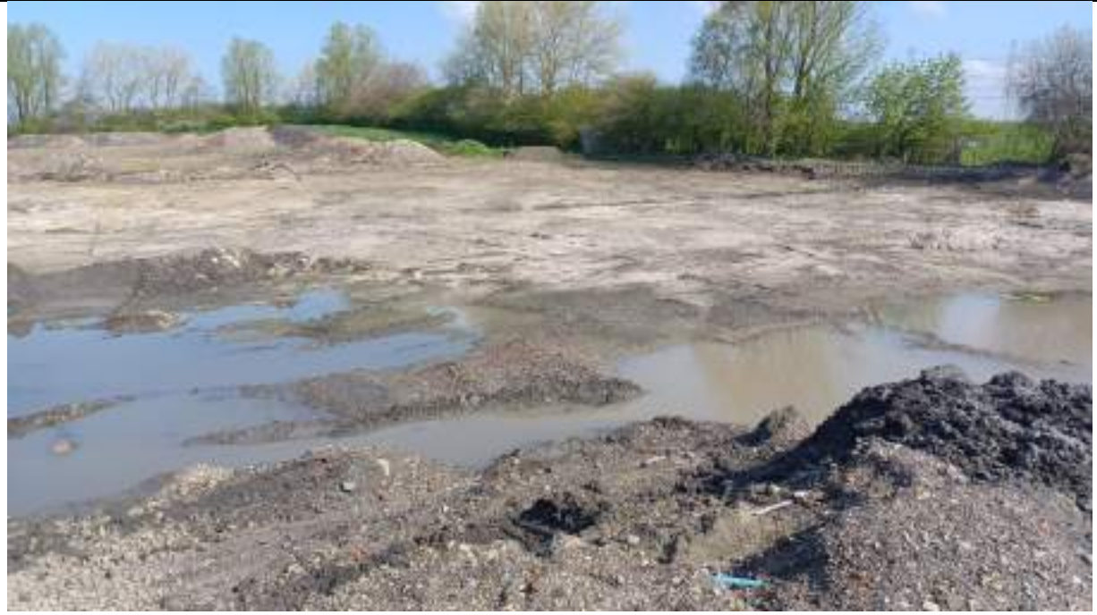
Photograph 5: Cut area in the northeast corner of the site. Some standing water observed
