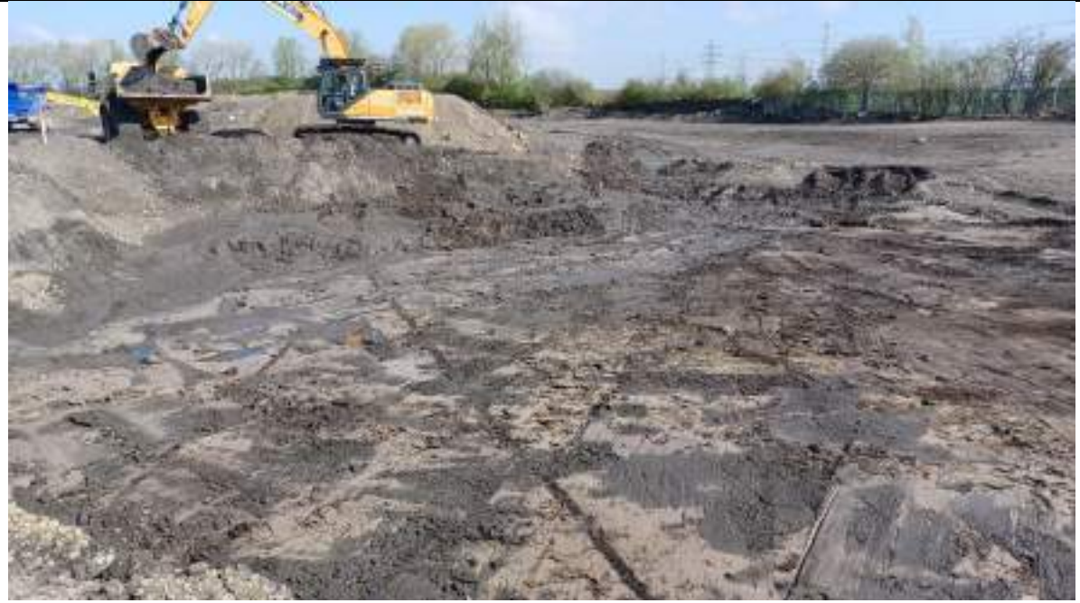
Photograph 3: Removal of sediment and silt from area of ponded water in the northeast. Natural Glacial Till exposed at the base.
