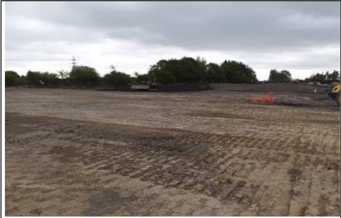
Photograph 3: Placing 6F2 material on top of placed general fill in the east and northeast.
