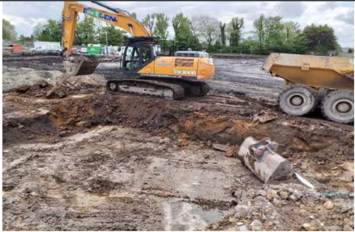
Photograph 1: Excavation of Glacial Till in the east.
