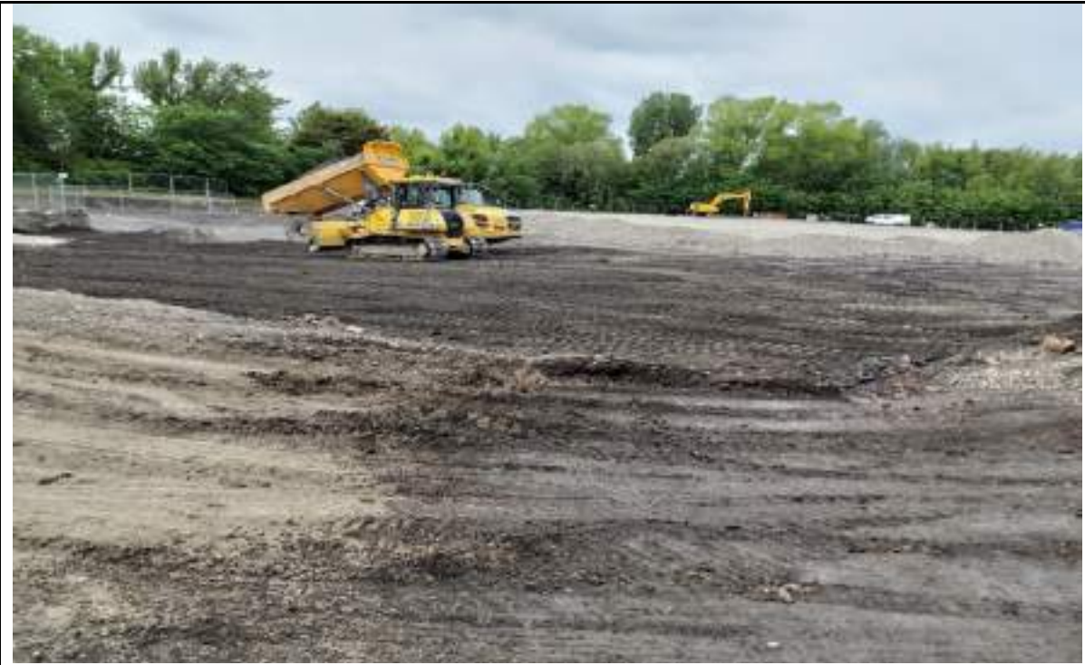
Photograph 1: Placing fill in the southeast near VHE compound. Fill material from stockpiles of fine material from crusher in the northwest.
