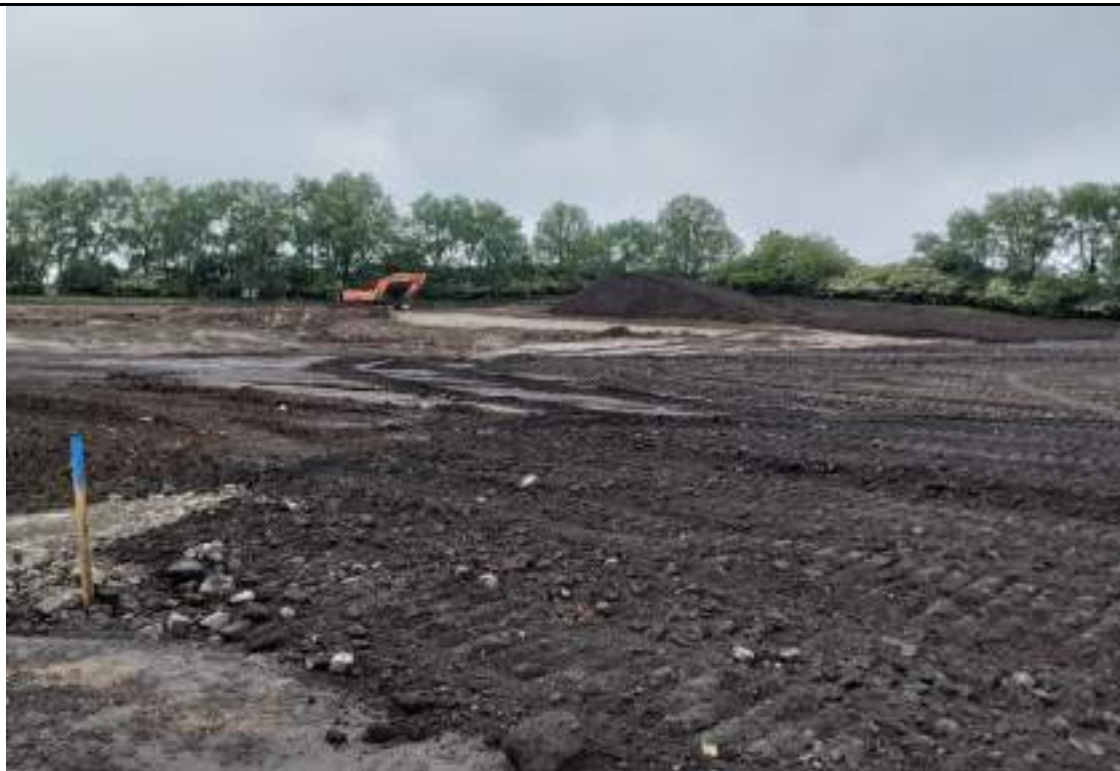
Photograph 10: Excavator trimming backfilled borrow pit.
