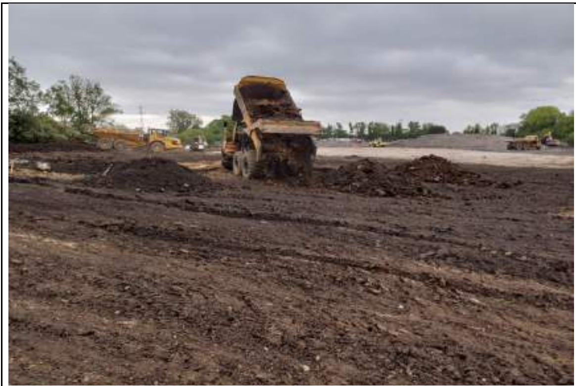
Photograph 6: Backfilling the borrow pit using material from low strength Glacial Till stockpile in the northeast.
