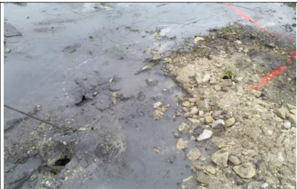
Photograph 2: Grouted boreholes for shaft no.7. Surface settlement of the shaft was backfilled by imported 6F5 material.
