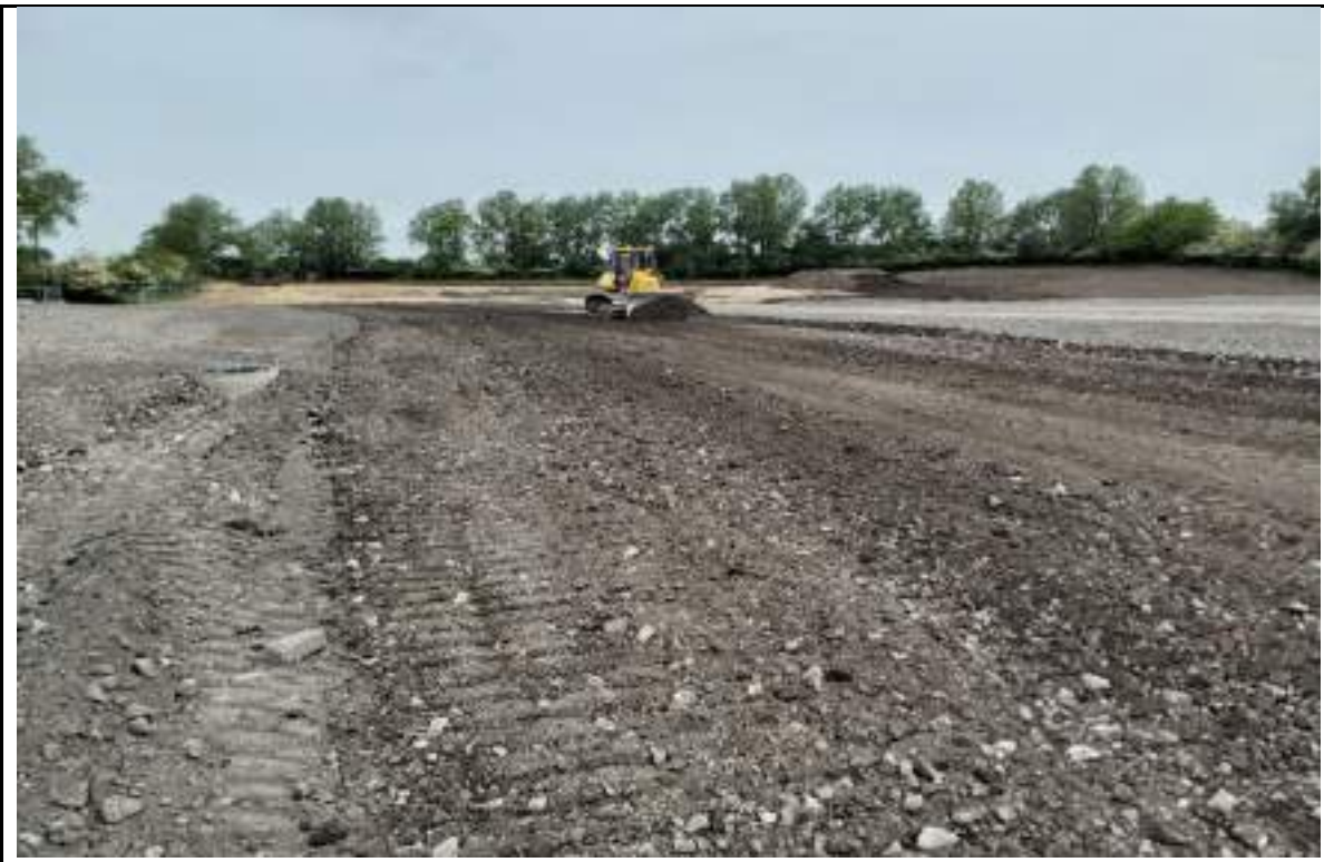
Photograph 4: Placing and levelling 6f2 material in the northwest.
