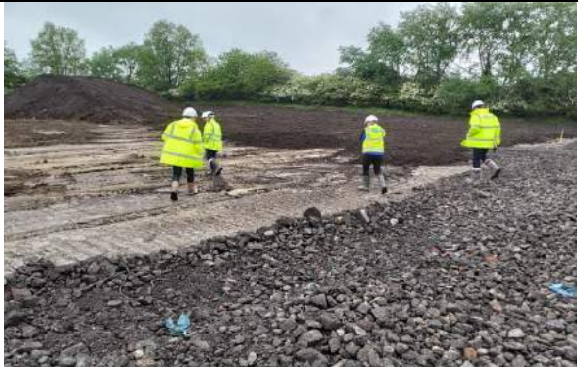
Photograph 11: Placed topsoil and stockpile of topsoil in the POS in the northeast.
