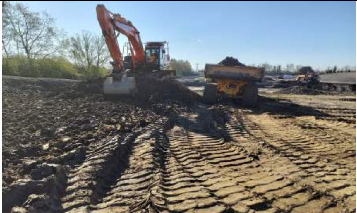
Photograph 9: Transferring stockpile of unsuitable material in the northeast to the northwest.
