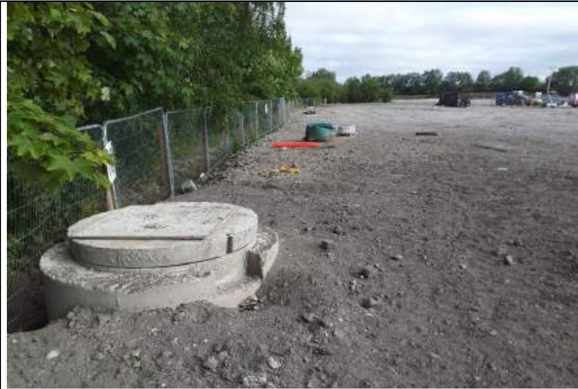
Photograph 3: Construction of two drainage manhole in the western boundary completed.
