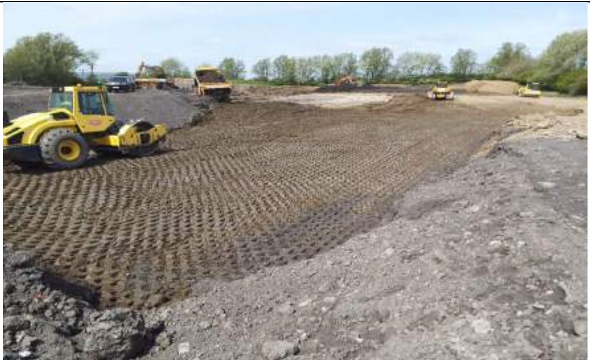
Photograph 4: Placing fill and proof rolling with sheepfoot roller in the center northeast. Material from Glacial Till excavation in the borrow pit.
