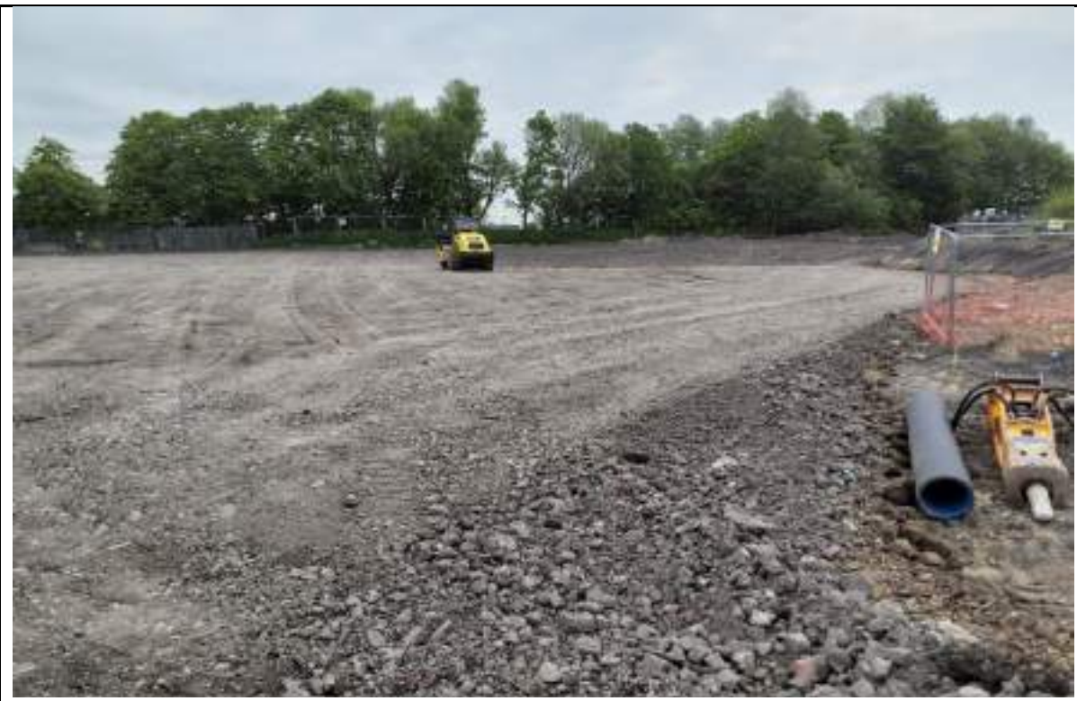
Photograph 12: Proof rolling of capping and in the east.
