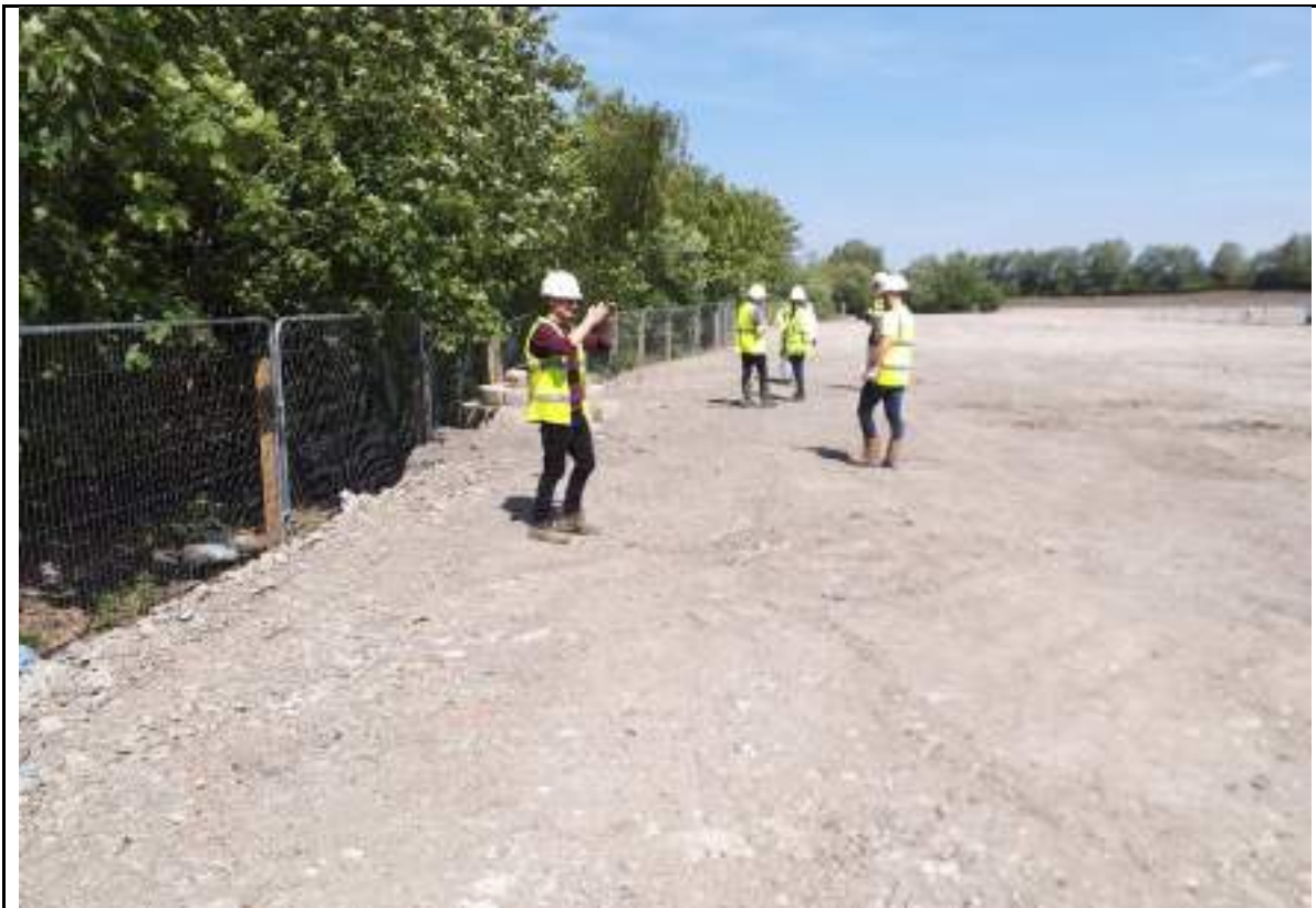
Photograph 6: Drainage manhole in the western boundary.
