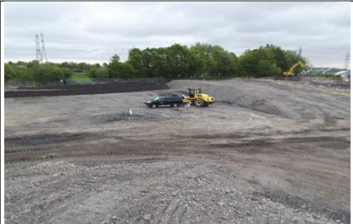
Photograph 10: Plate load testing by PSL on capping layer in the centre east.
