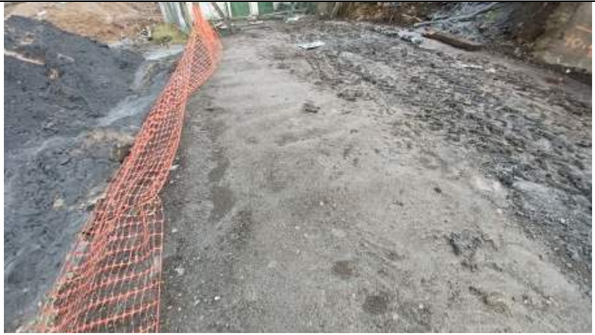
Photograph 1: Location of shaft 006 – treatment complete
