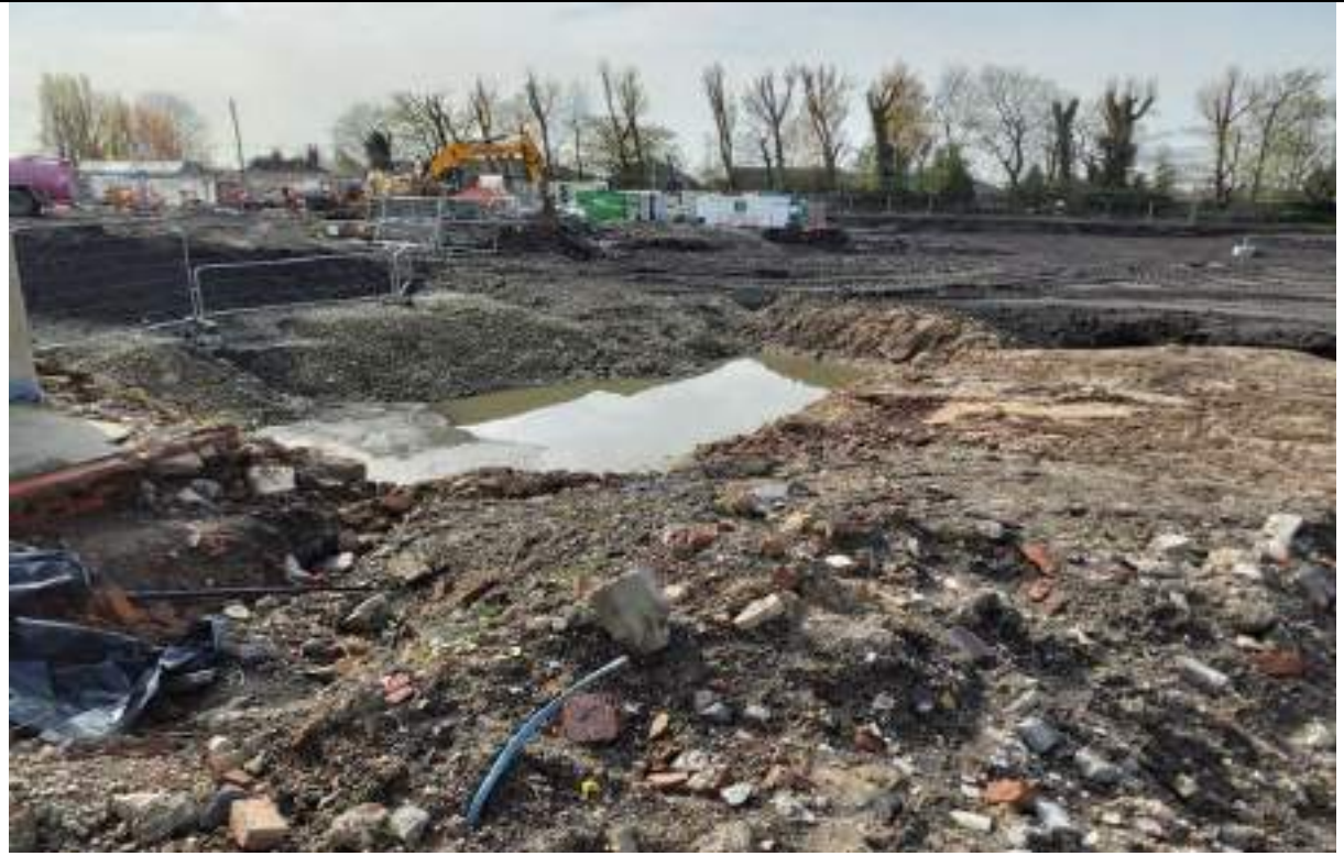
Photograph 15: Second standing water in the southeast.
