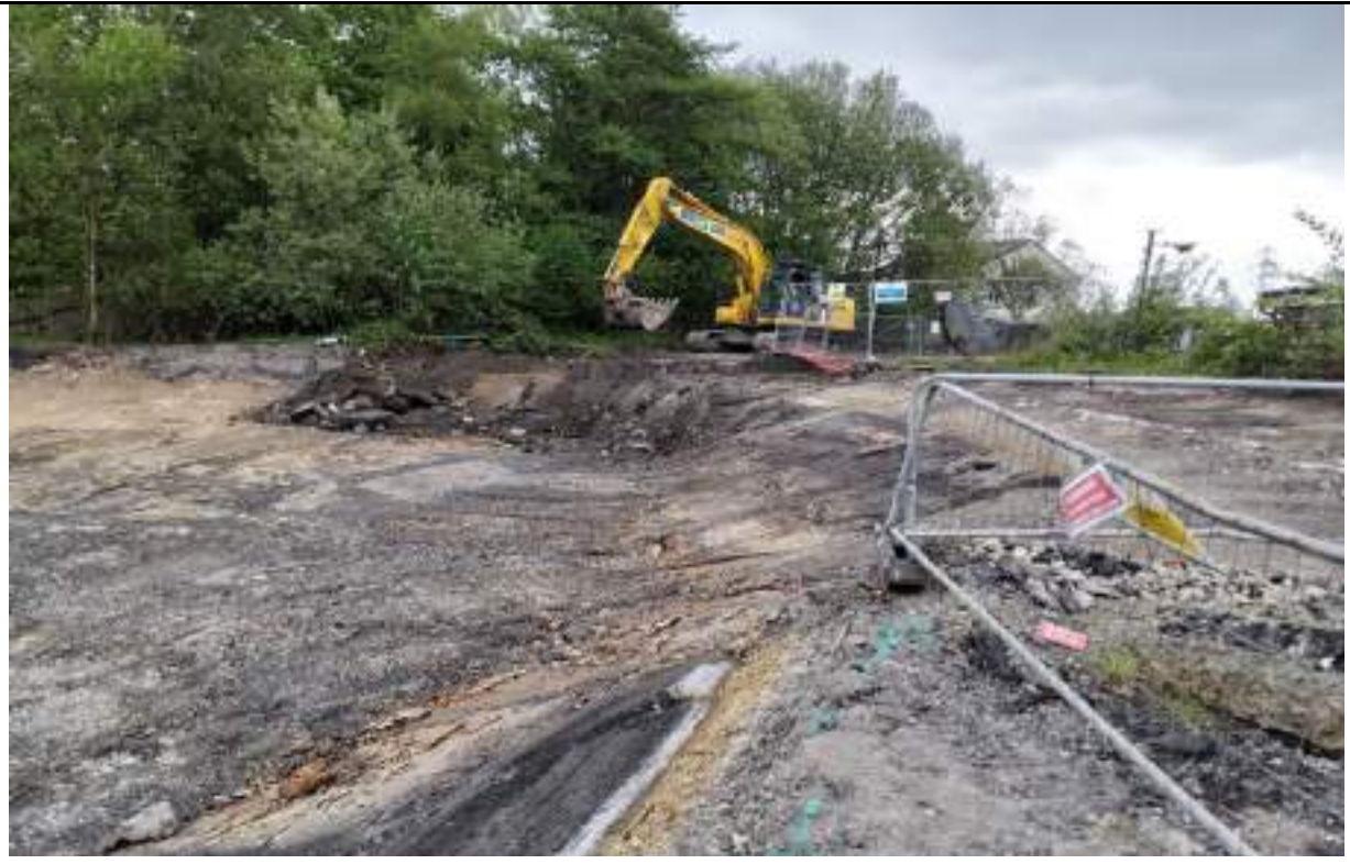
Photograph 1: Excavation of concrete and furnace Made Ground in the southeast.
