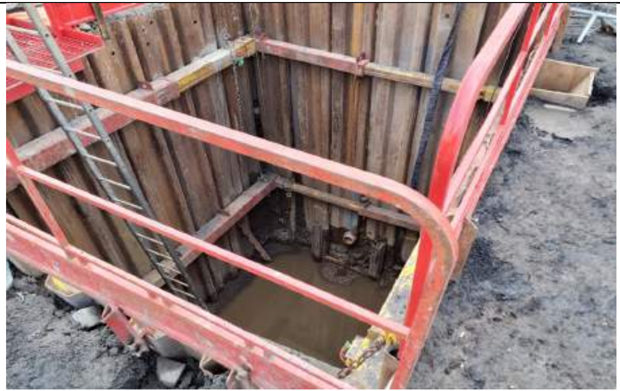
Photograph 12: Ceramic pipe placed in thrust bore drainage in the southeast.
