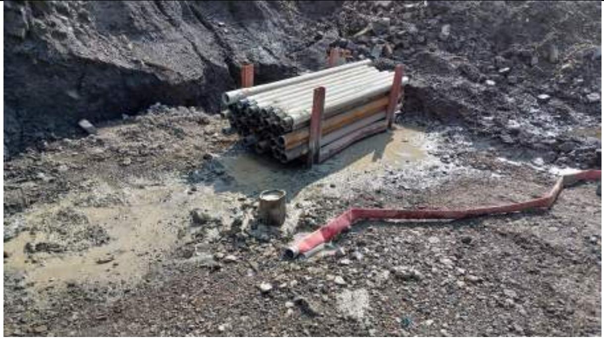
Photograph 7: Grouting complete for the observed borehole in the northwest of the site.
