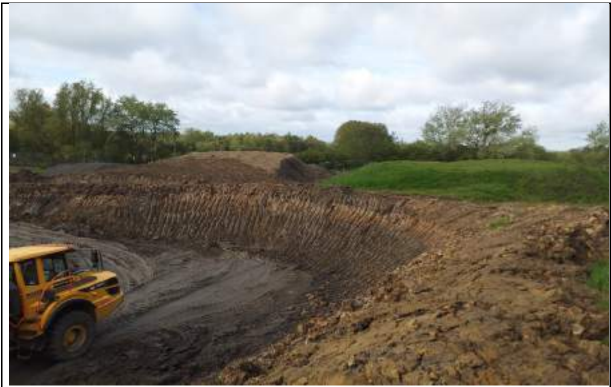
Photograph 8: Stockpiles of topsoil and unsuitable material in the western side of the borrow pit.
