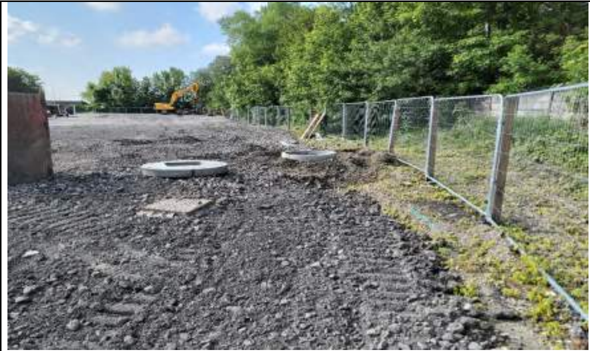
Photograph 3: Location of second drainage manhole placed in the western boundary.
