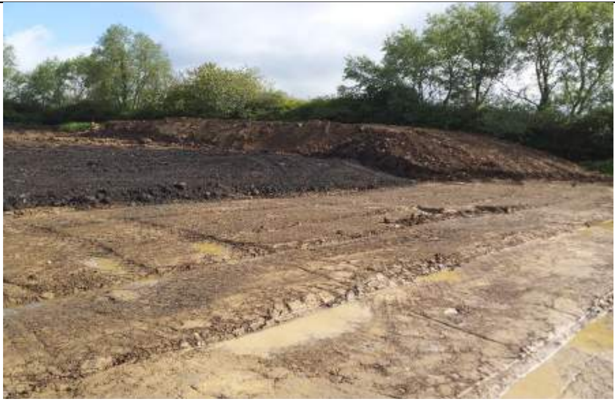
Photograph 8: Stockpiles of low strength glacial till excavated from the borrow pit area in the northeast.
