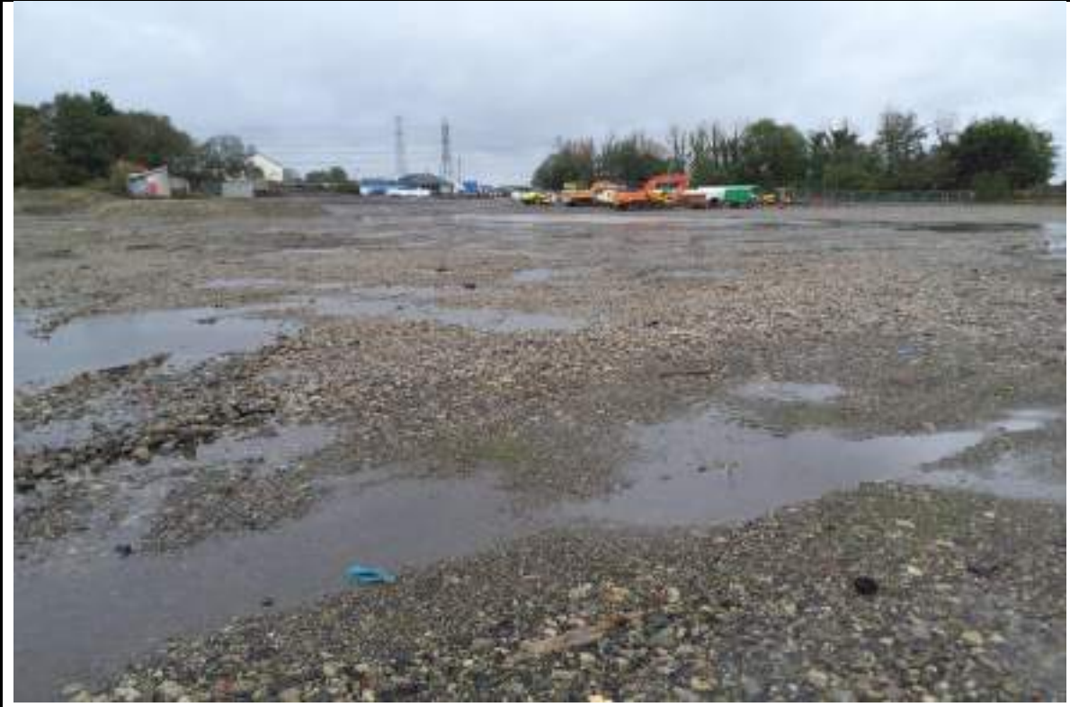
Photograph 5: Stockpile of imported 6F5 material and VHE earthwork machinery in the southeast.
