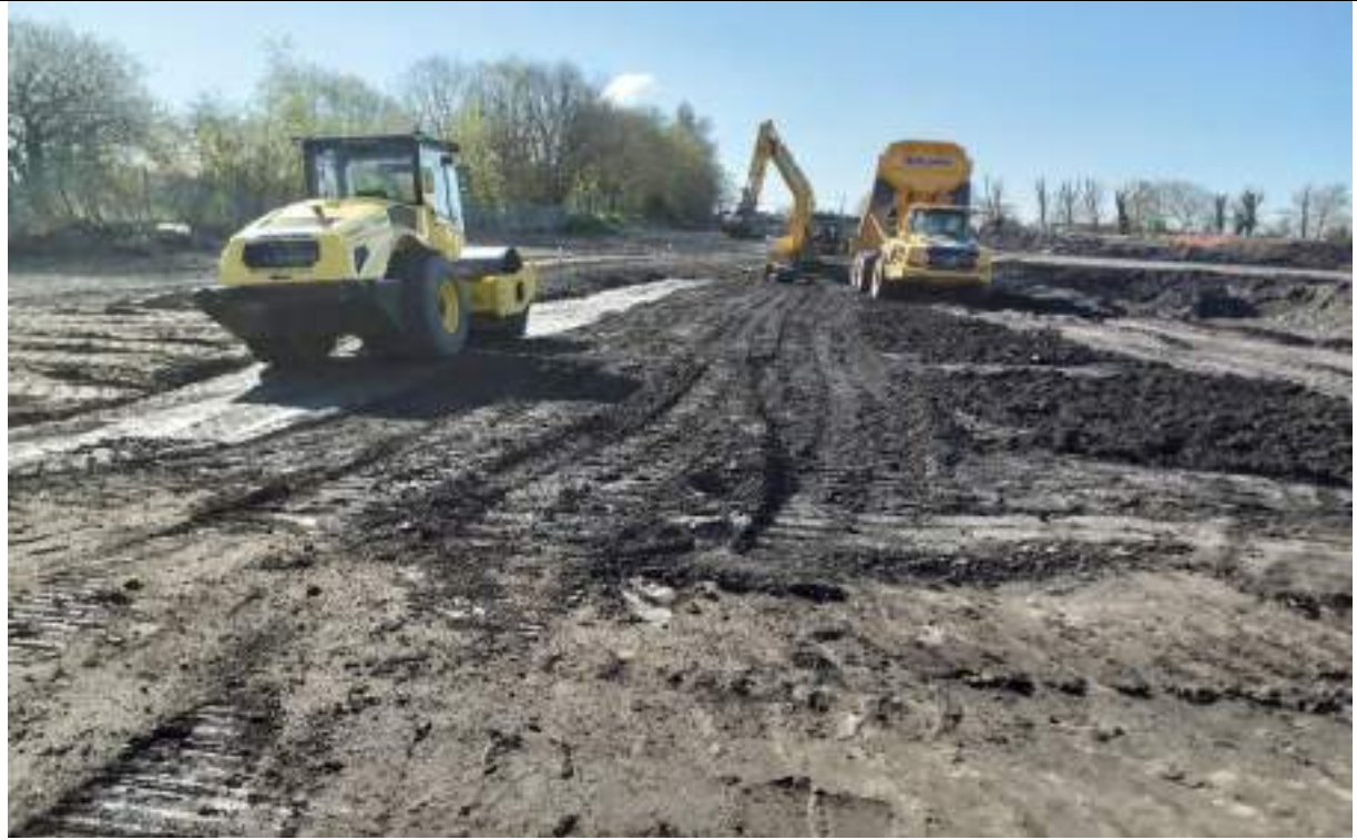
Photograph 7: Placing fill and proof rolling of fill material in the northeast.
