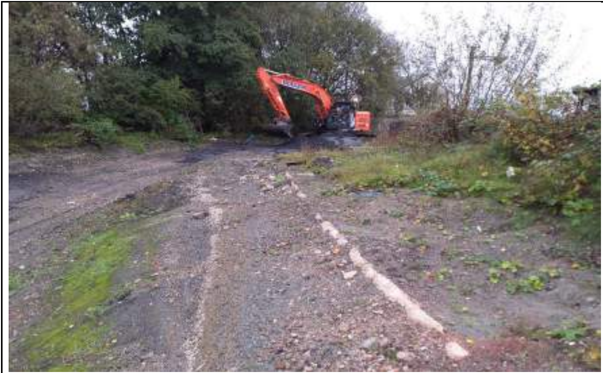
Photograph 3: Excavator removing surplus PFA material on access road in the southeast.
