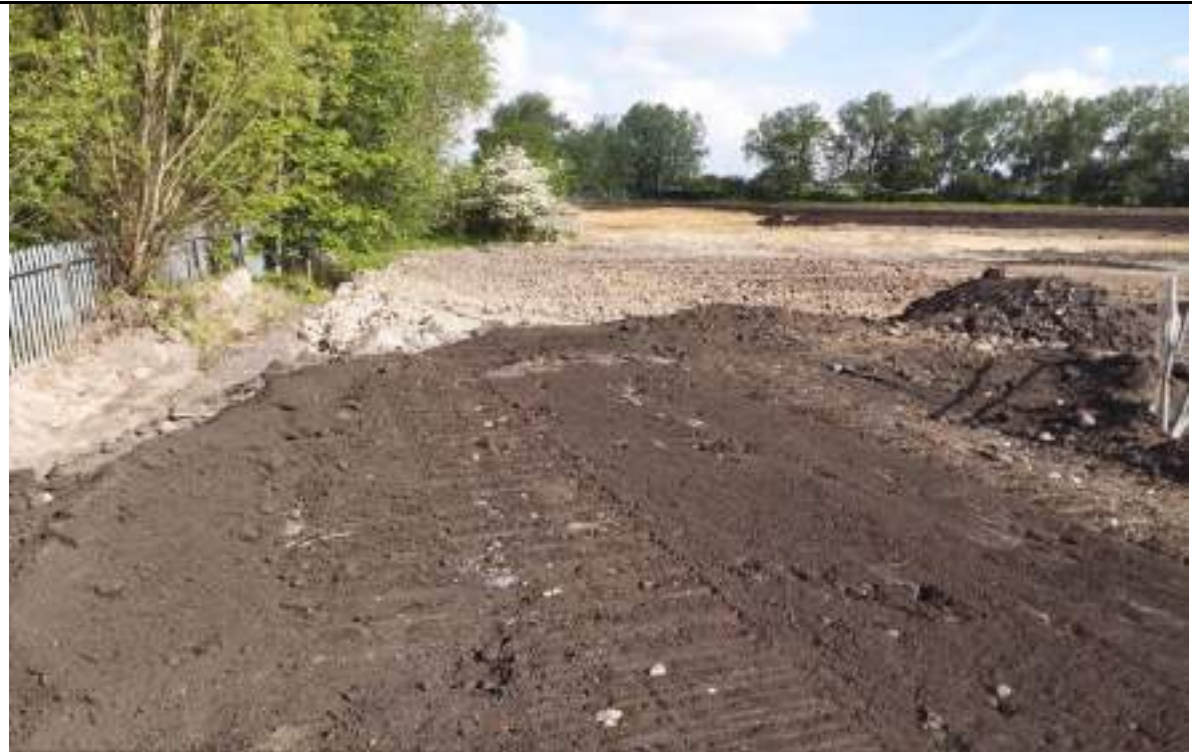
Photograph 11: POS area in the northwest still needs fill to reach final level.
