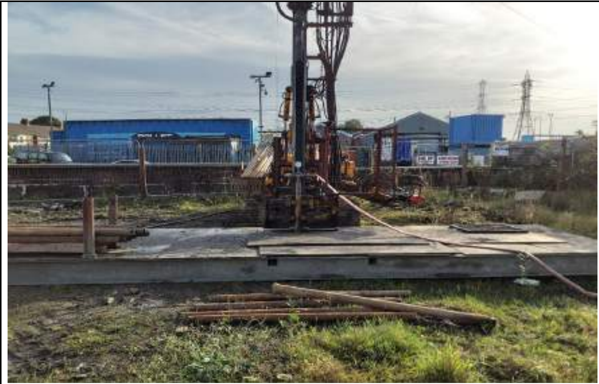
Photograph 3: Drilling rig and platform on top of shaft no.008.
