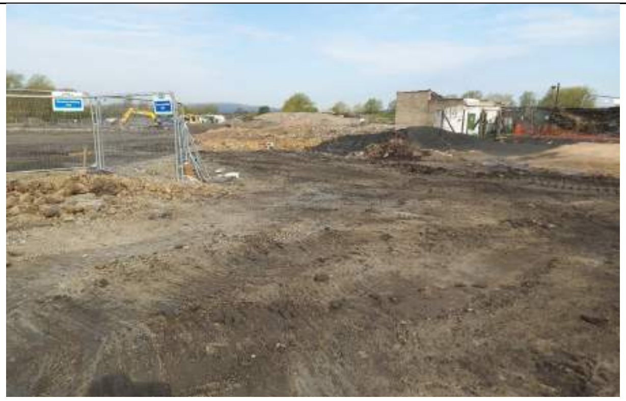
Photograph 2: Temporary new road constructed in the southeast near grouted shaft no. 006.
