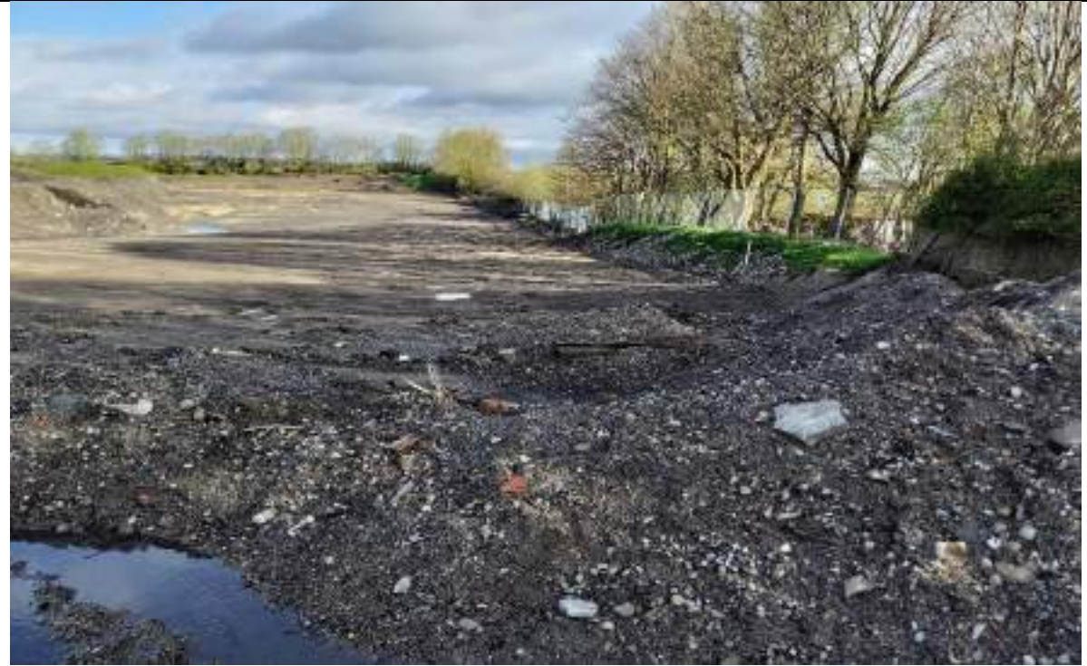
Photograph 3: Eastern boundary of the site. Looking towards the north. Boundary checks required by VHE.
