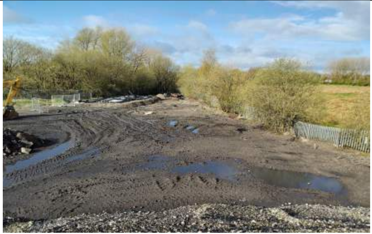
Photograph 7: Stockpile of TPH contaminated material arising from Hotspot 7.
