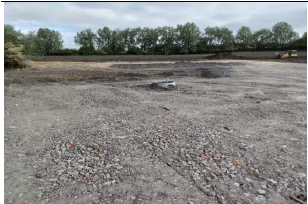
Photograph 6: Area in the northwest still needs filling material.
