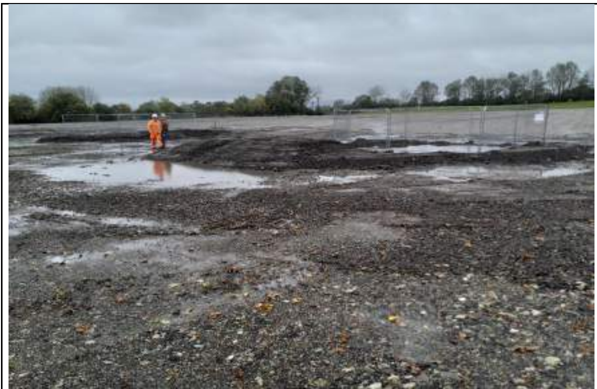
Photograph 4: Excavations in the centre and east of the site to find culvert location. Both excavations covered with water.
