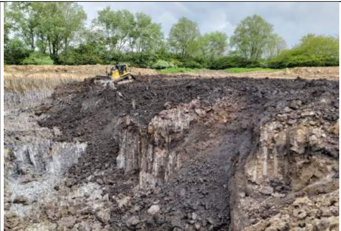
Photograph 7: Excavation of Glacial Till from the borrow pit in the north.
