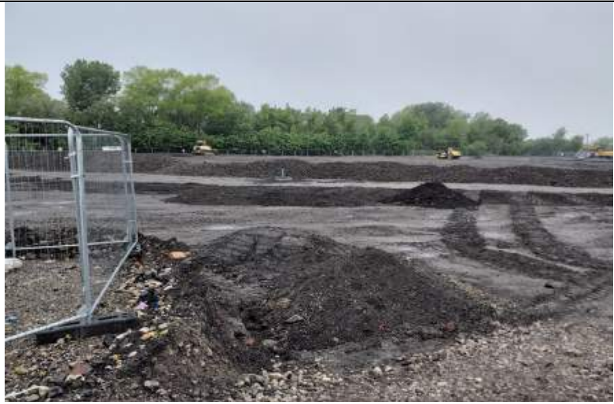
Photograph 1: Placing and proof rolling 6F2 capping in the southwest.
