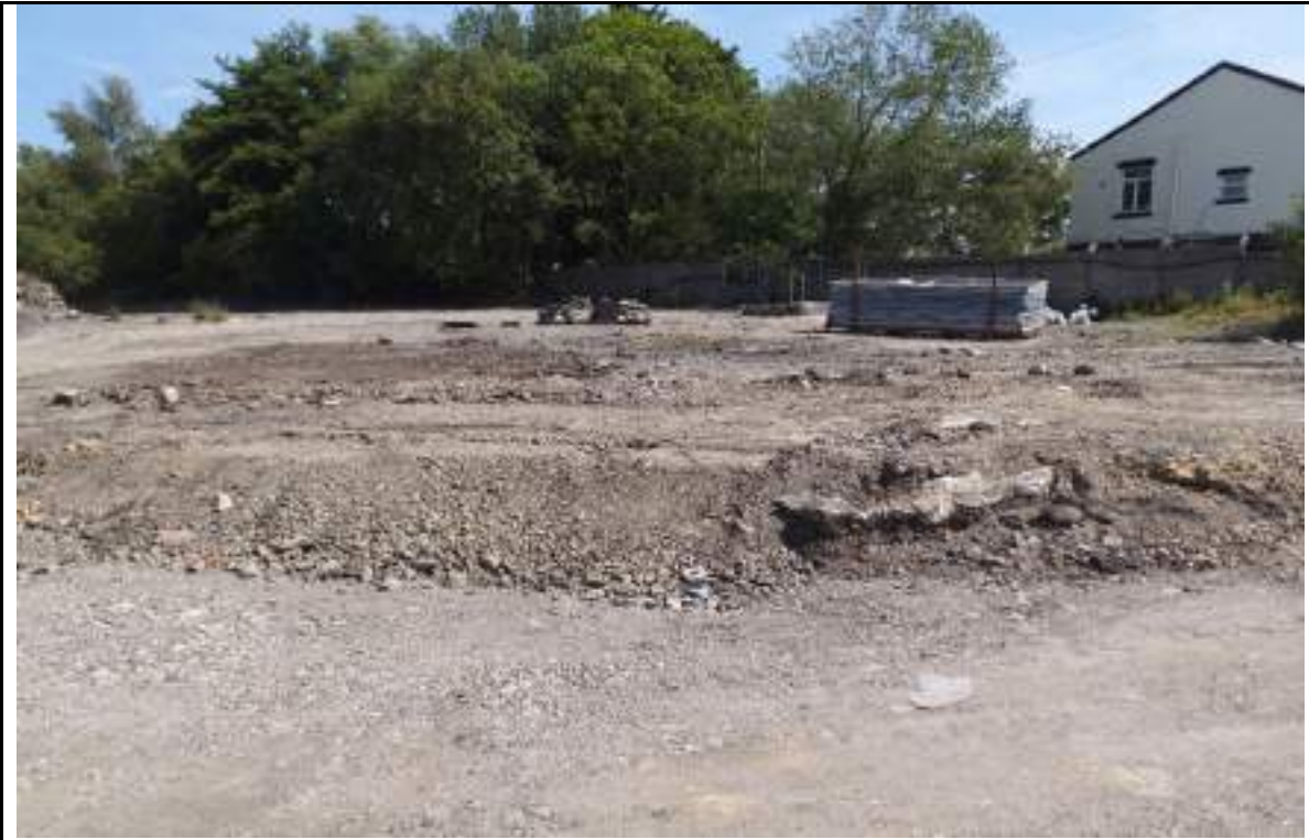
Photograph 3: Shaft no.7 area, not included in earthworks area.
