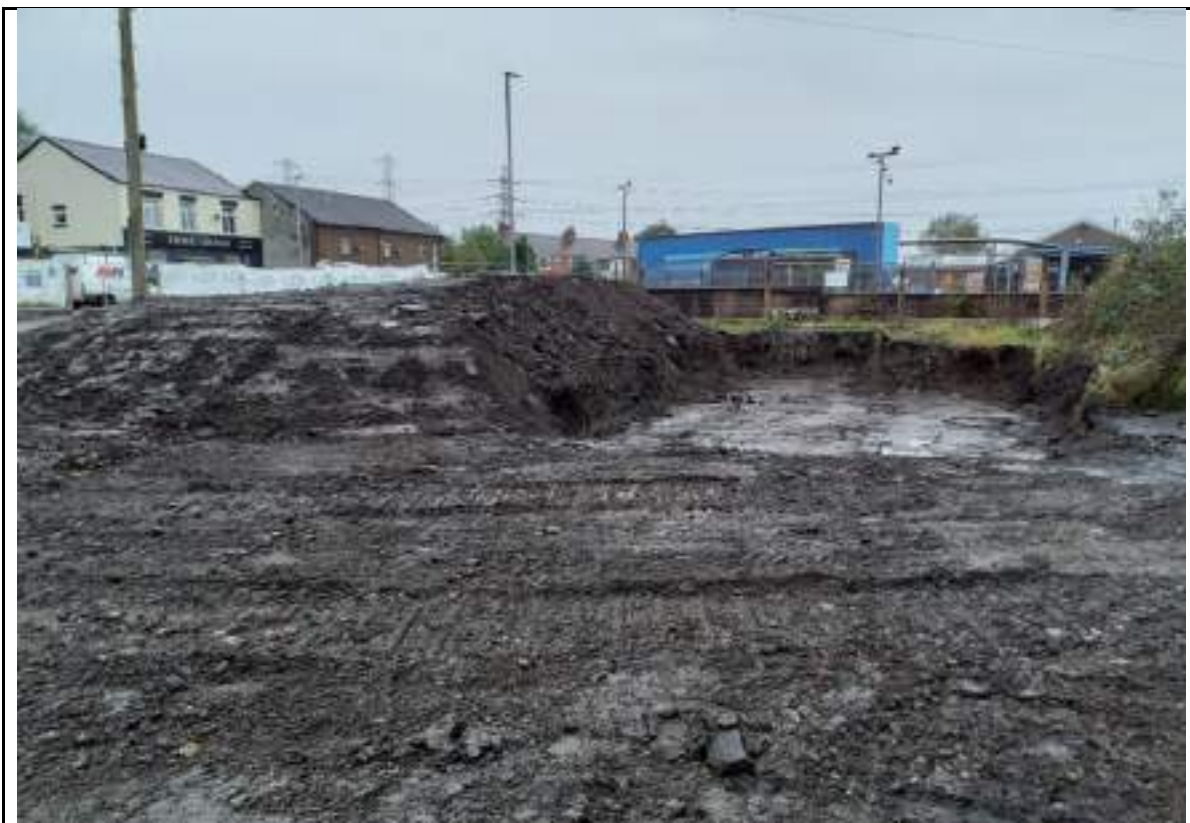
Photograph 4: Excavation of Made Ground in the location of shaft no.8. Material has high moisture content.
