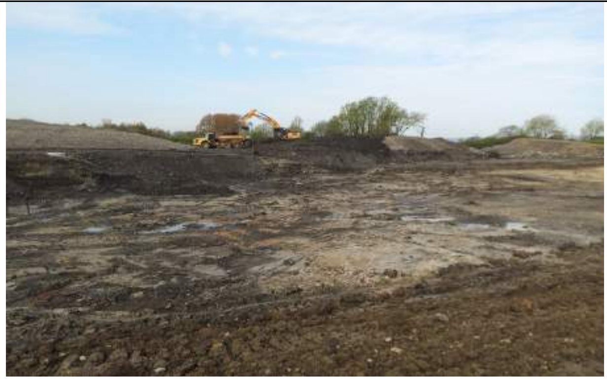
Photograph 5: Transferring peat from peat stockpile to borrow pit
