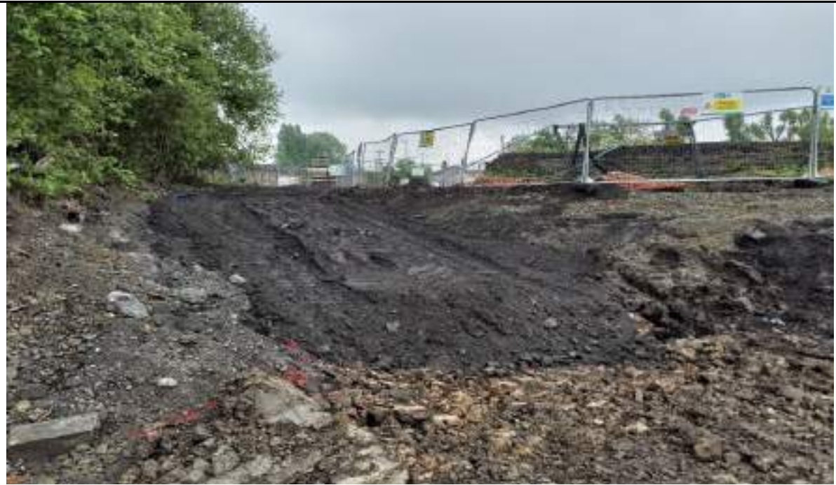
Photograph 113: Furnace Made Ground used to construct haul road in the southeast.
