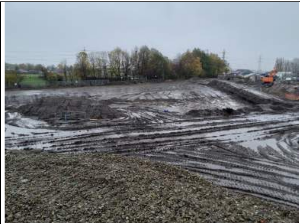
Photograph 14: Backfilled area in the east. Looking towards the east.
