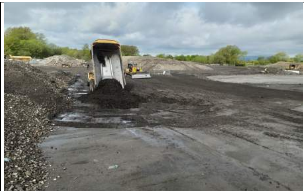
Photograph 4: Placing fill in the centre east of the site. Material from excavation of landfill Made Ground in the east.
