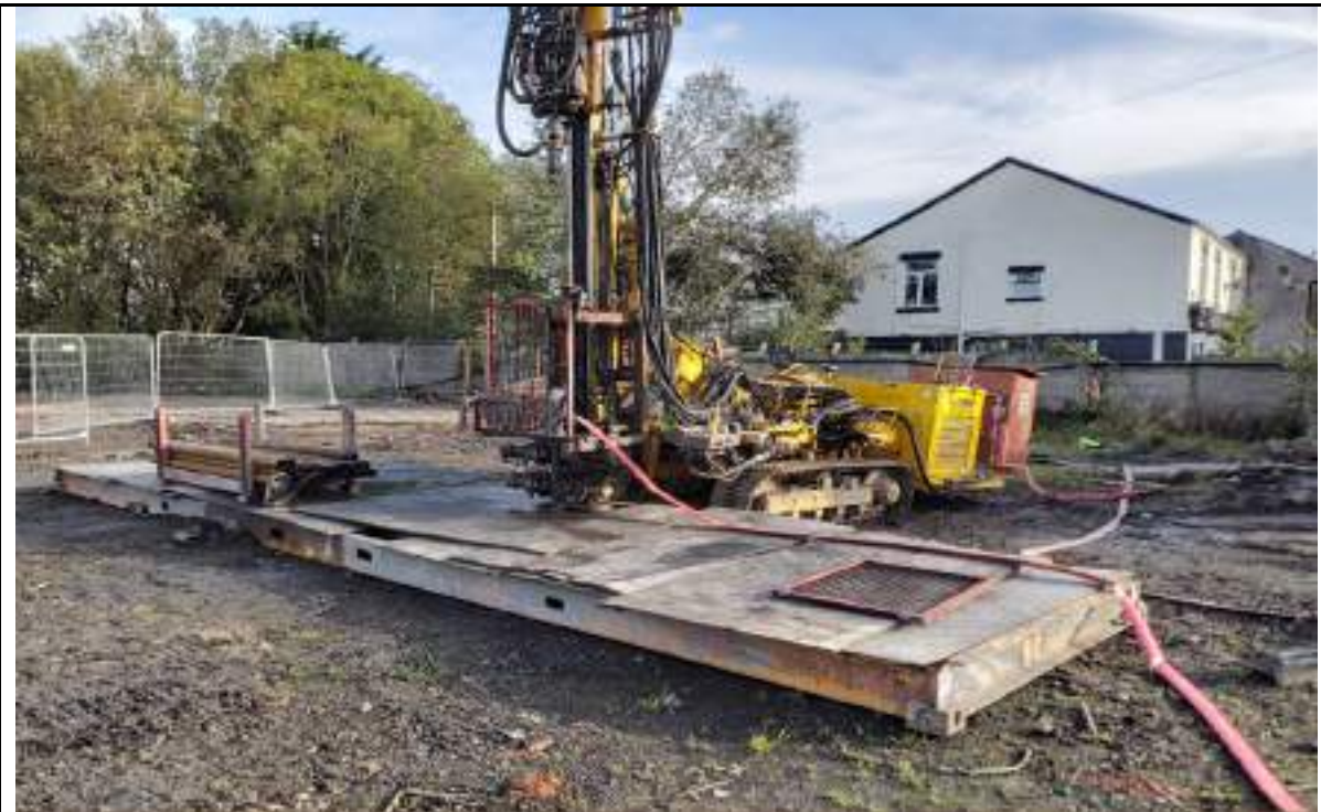
Photograph 1: Drilling rig and platform on top of shaft no.007.
