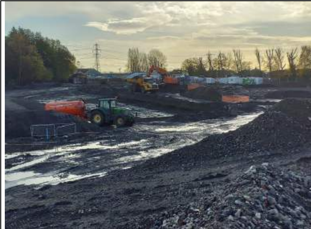
Photograph 25: Loading deleterious material into truck in the southeast.
