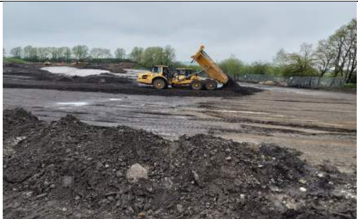
Photograph 4: Placing 6F2 material in the east. Material from 6F2 stockpile.
