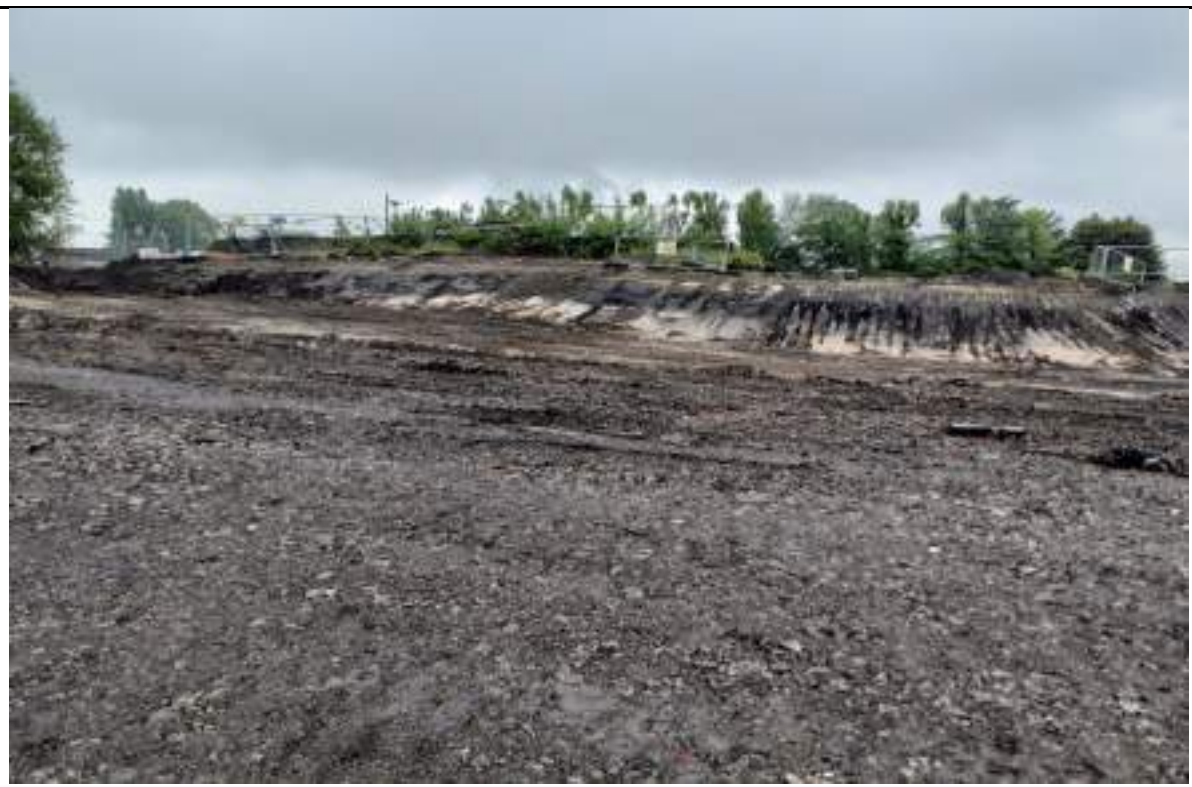
Photograph 12: Battered slope behind transformer house.
