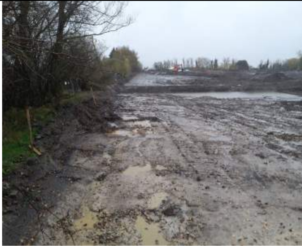
Photograph 7: Eastern boundary of the site. Looking towards the south.
