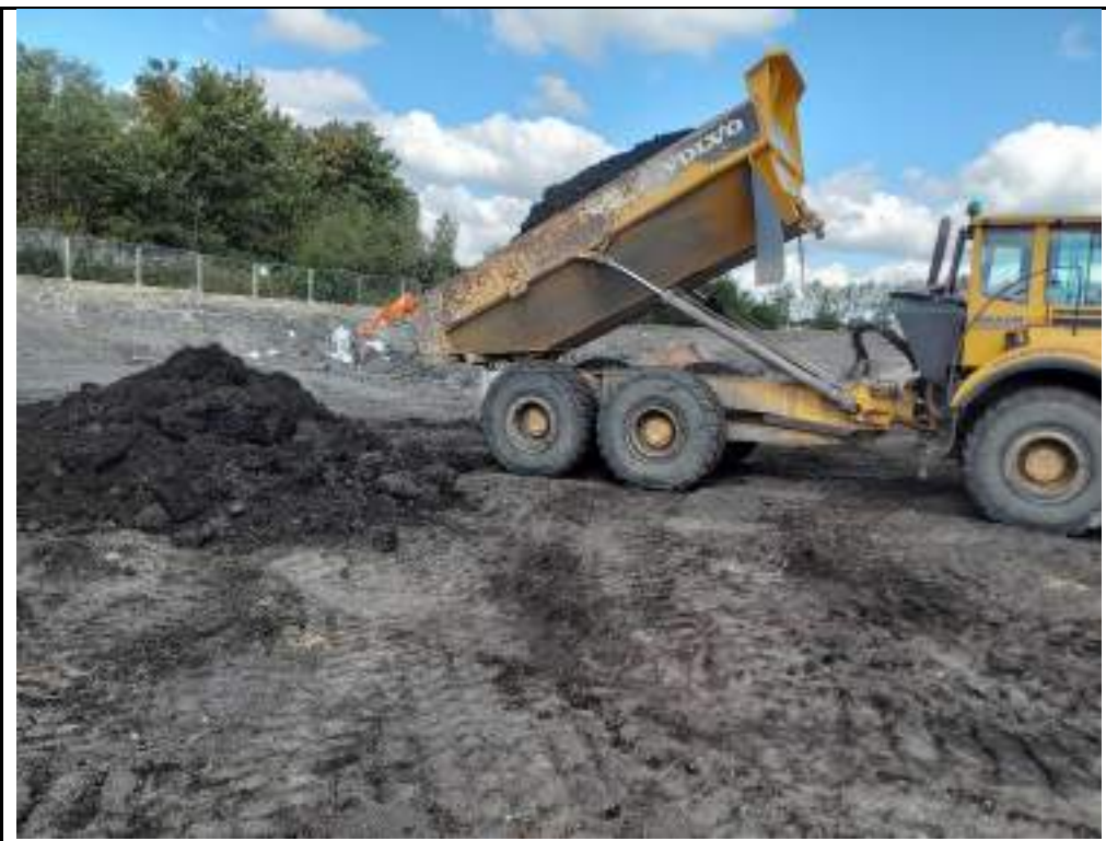
Photograph 4: Backfilling of western part of the site using excavated material from south of the site.
