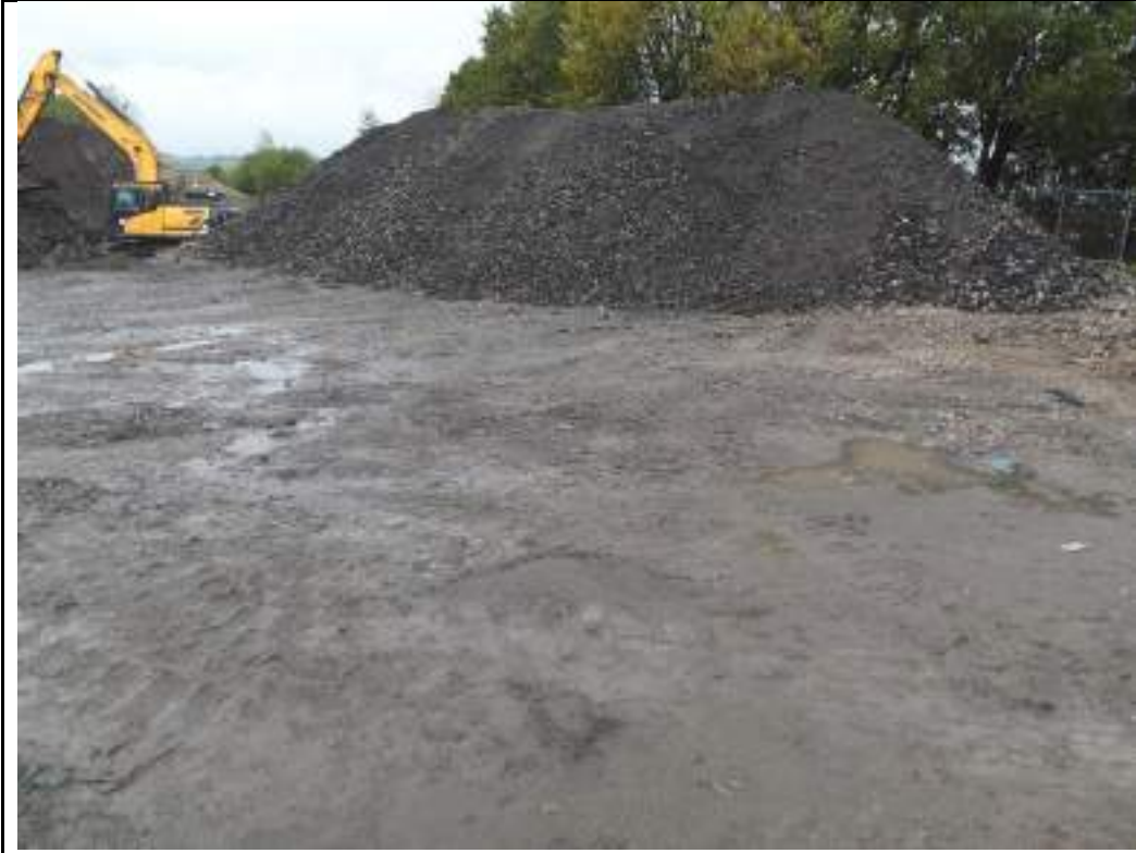
Photograph 9: Stockpiles of crushed concrete and asphalt in eastern part of the site.
