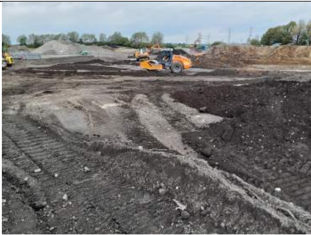
Photograph 6: Proof rolling of fill in central part of the site.
