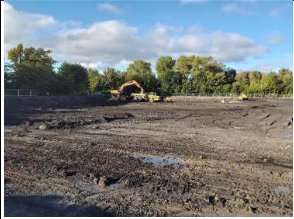
Photograph 3: Excavation of landfill Made Ground in southern part of the site.
