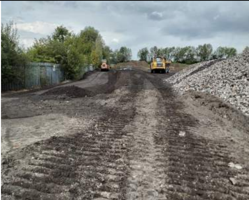
Photograph 158: Proof rolling of northwestern boundary of the site.
