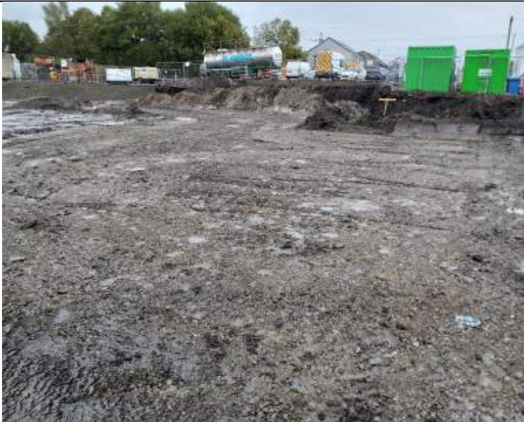
Photograph 20: Soft spot area backfilled with engineered fill in southern part of the site.
