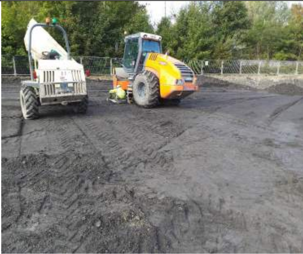
Photograph 8: Plate load testing on fill material in western part of the site.
