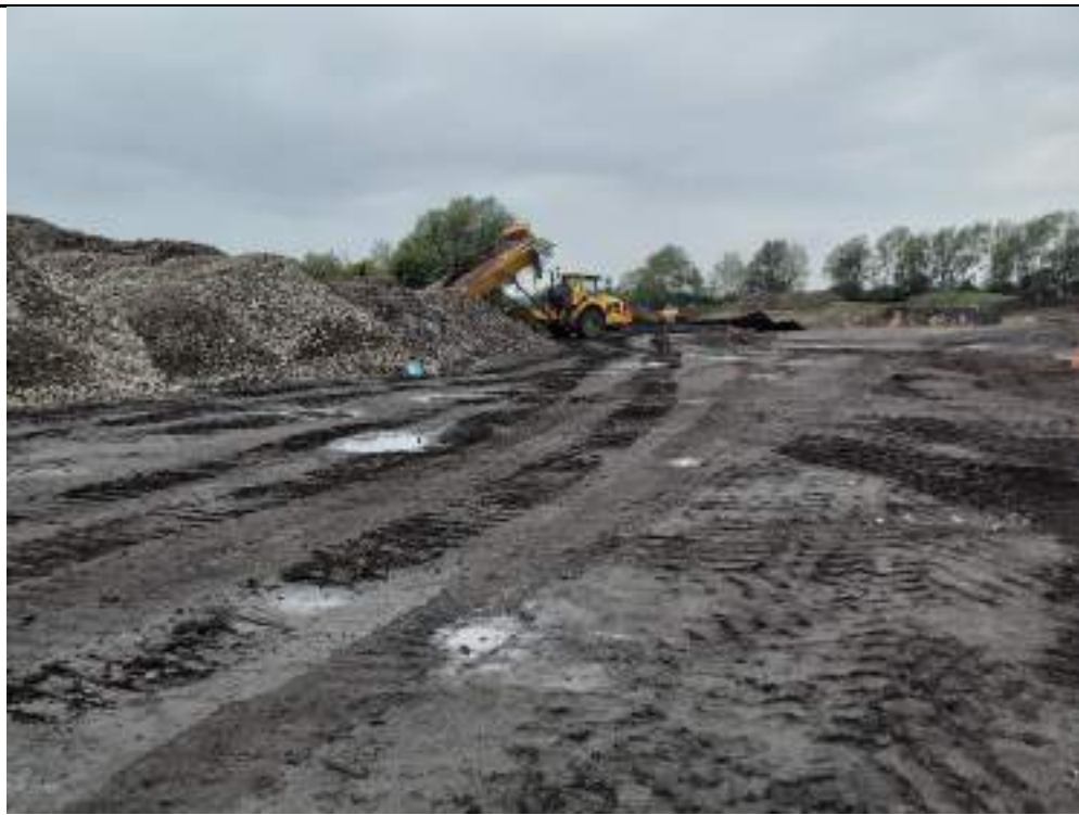
Photograph 6: Unloading crushed material from eastern stockpile in northwestern stockpile.
