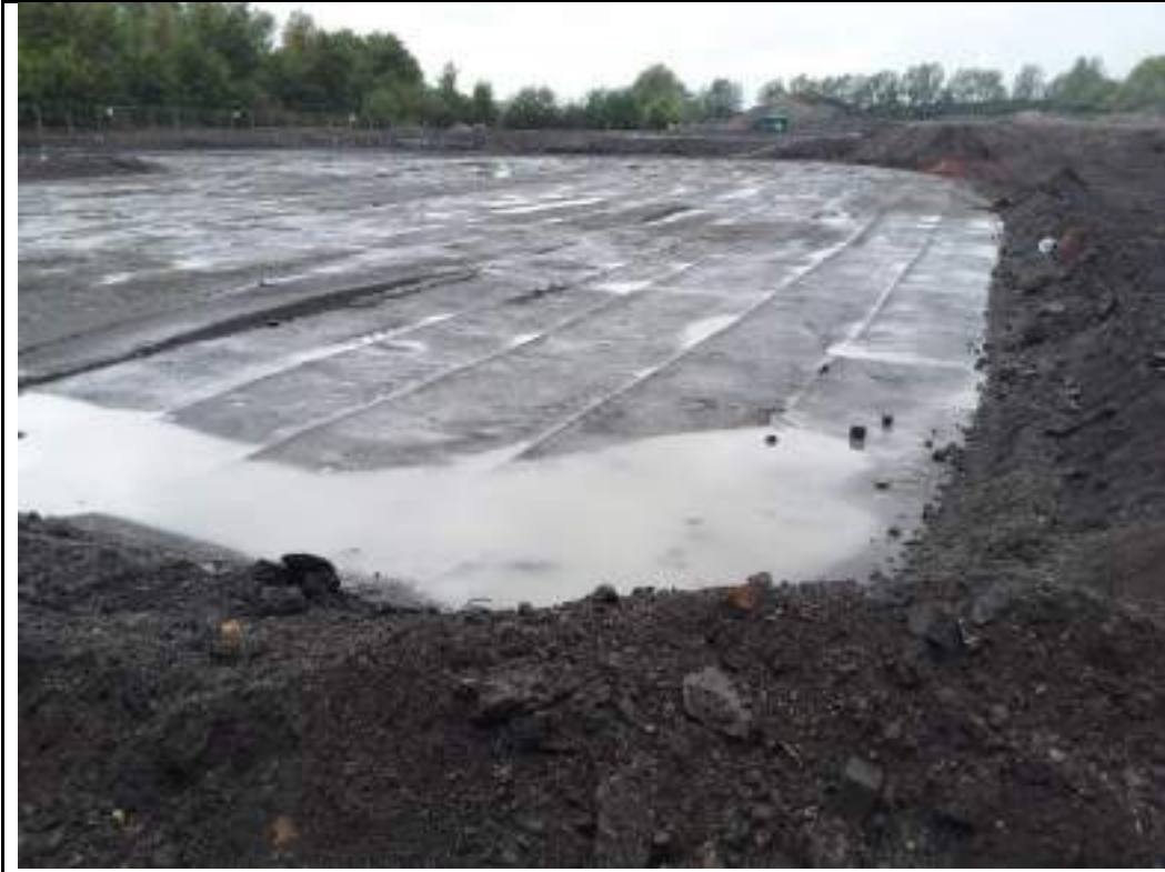
Photograph 7: Standing water in southern part of the site.
