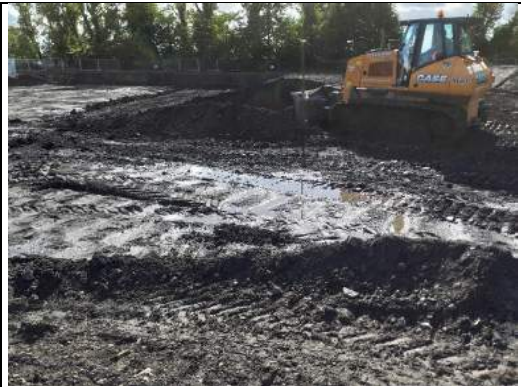
Photograph 14: Backfilling southern part of the site using material from excavation in southwestern part of the site.
