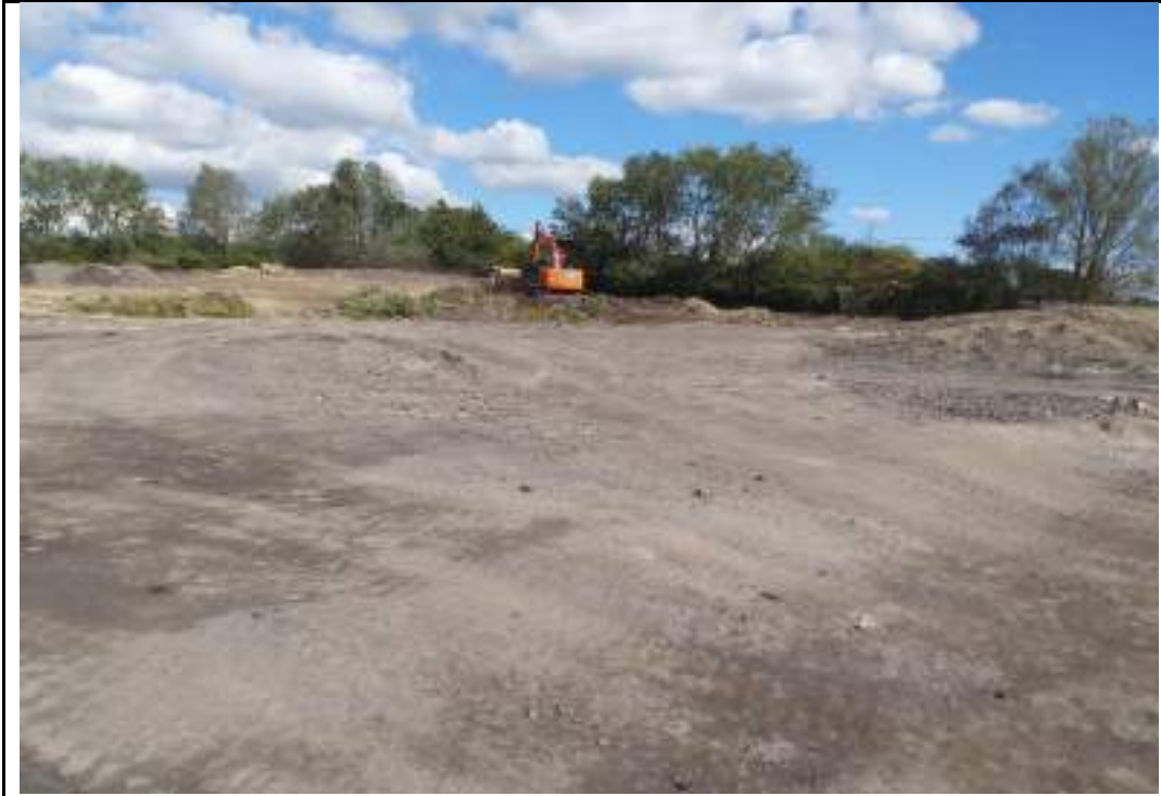
Photograph 179: Excavation of topsoil in northeast of the site.
