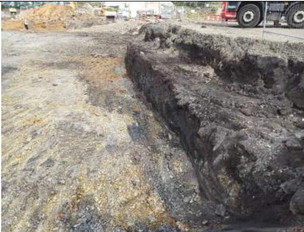
Photograph 30: Battered and stepped excavation in southeast of the site.
