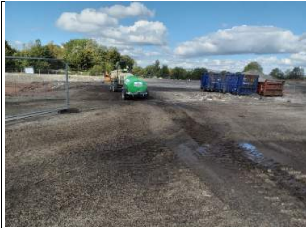
Photograph 199: Reducing dust on site using dust suppression unit.
