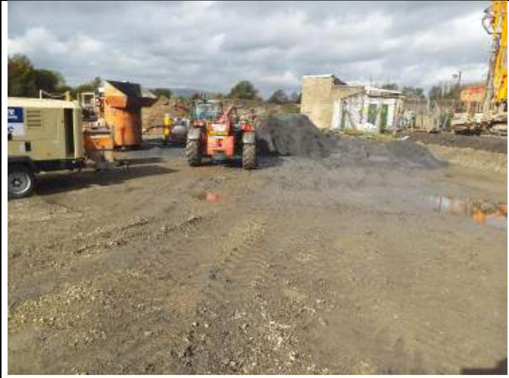
Photograph 3: Grout mixer and grout delivery in eastern part of the site.
