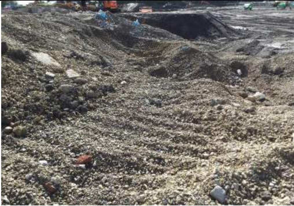
Photograph 19: Oversize materials in granular stockpile in northeast of the site.
