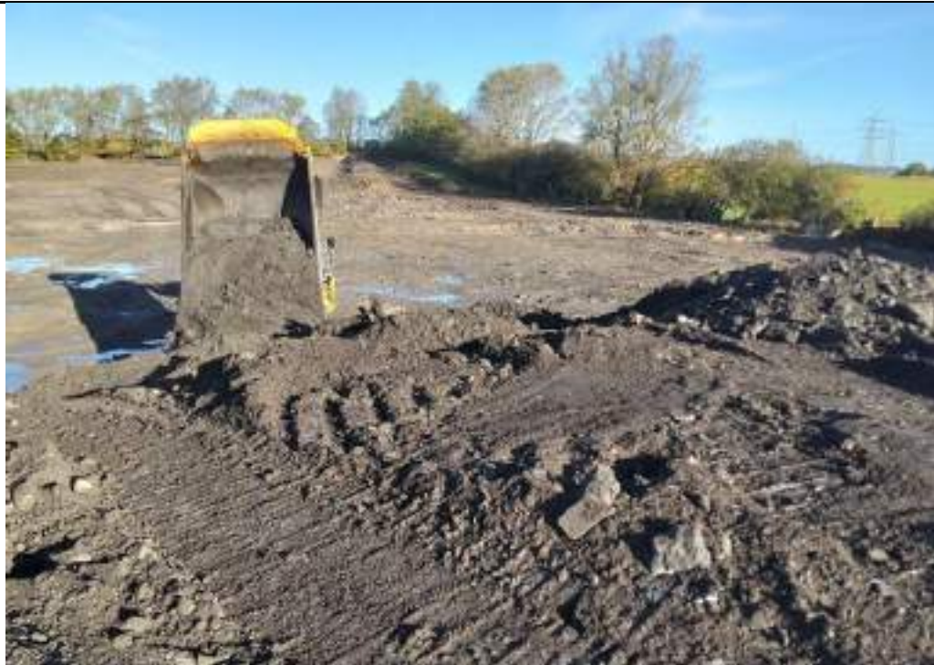
Photograph 16: Unloading excavated material from eastern excavation in northeastern part of the site.
