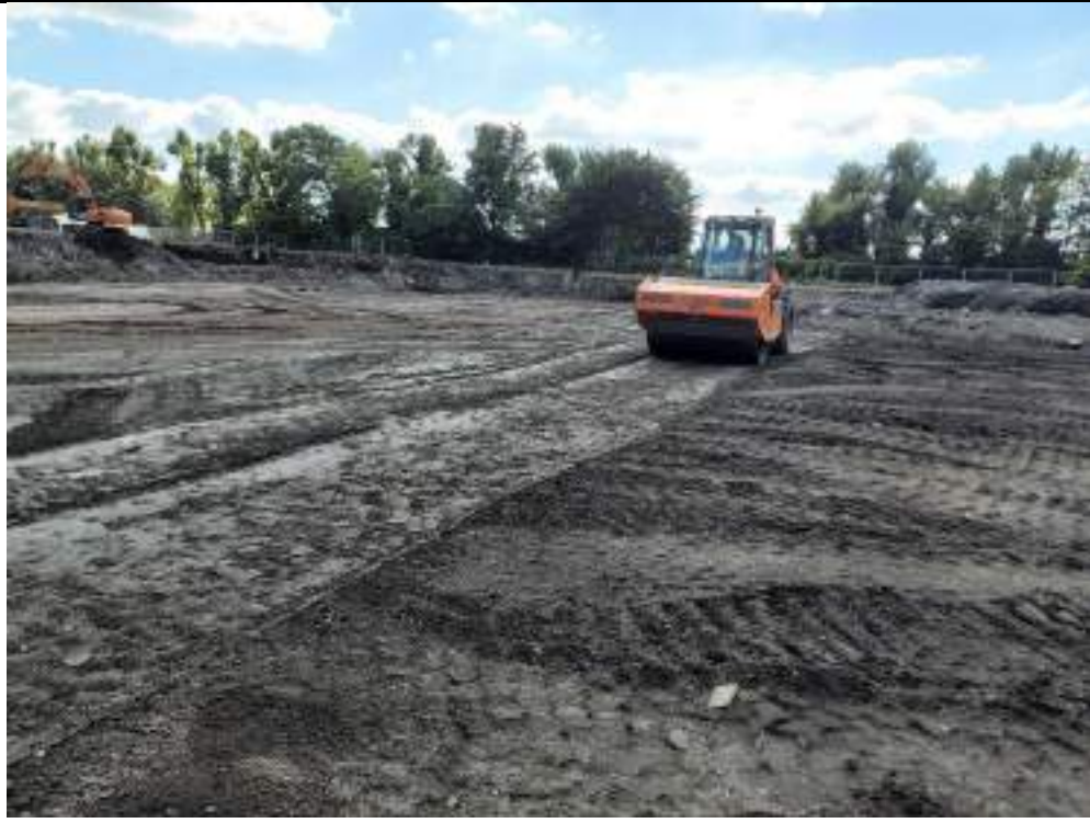
Photograph 5: Proof rolling of fill material in southern part of the site.
