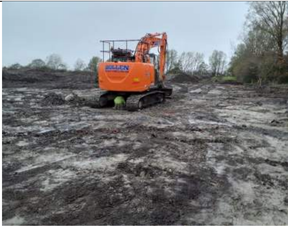
Photograph 8: Plate load testing on formation level (Glacial Till) in northeast of the site.
