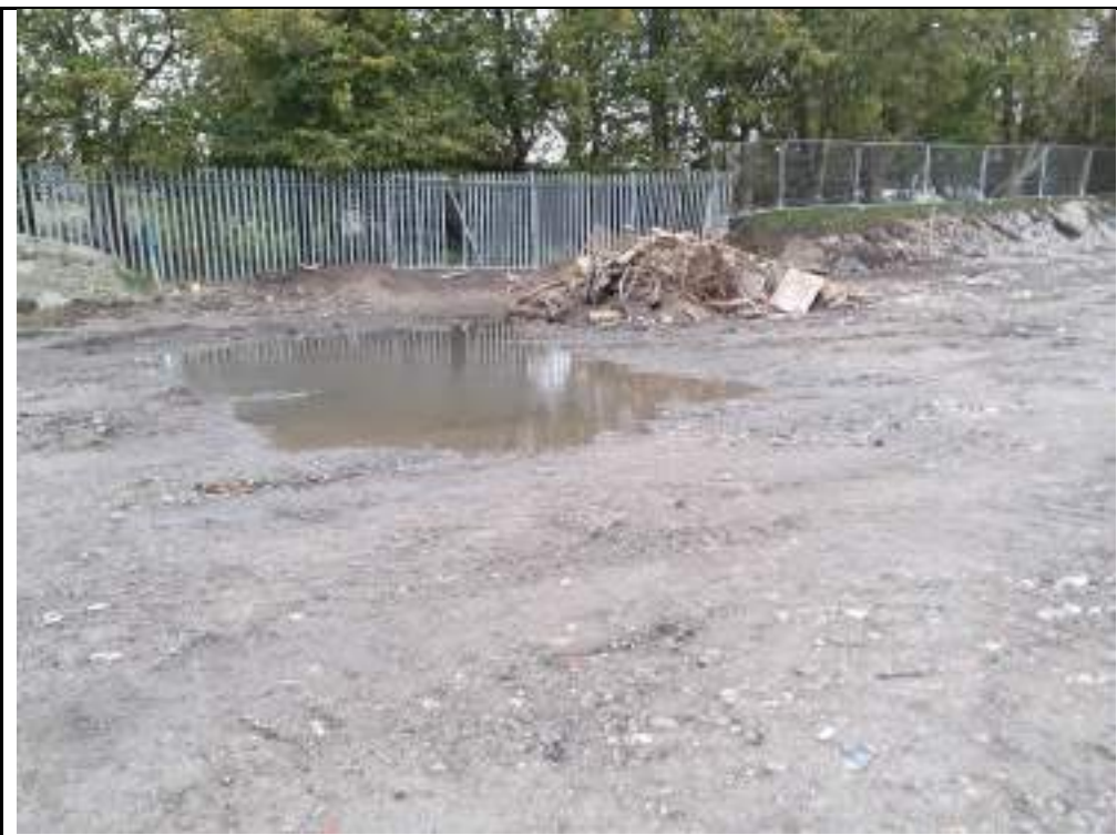
Photograph 4: Standing water and deleterious material in eastern boundary of the site.
