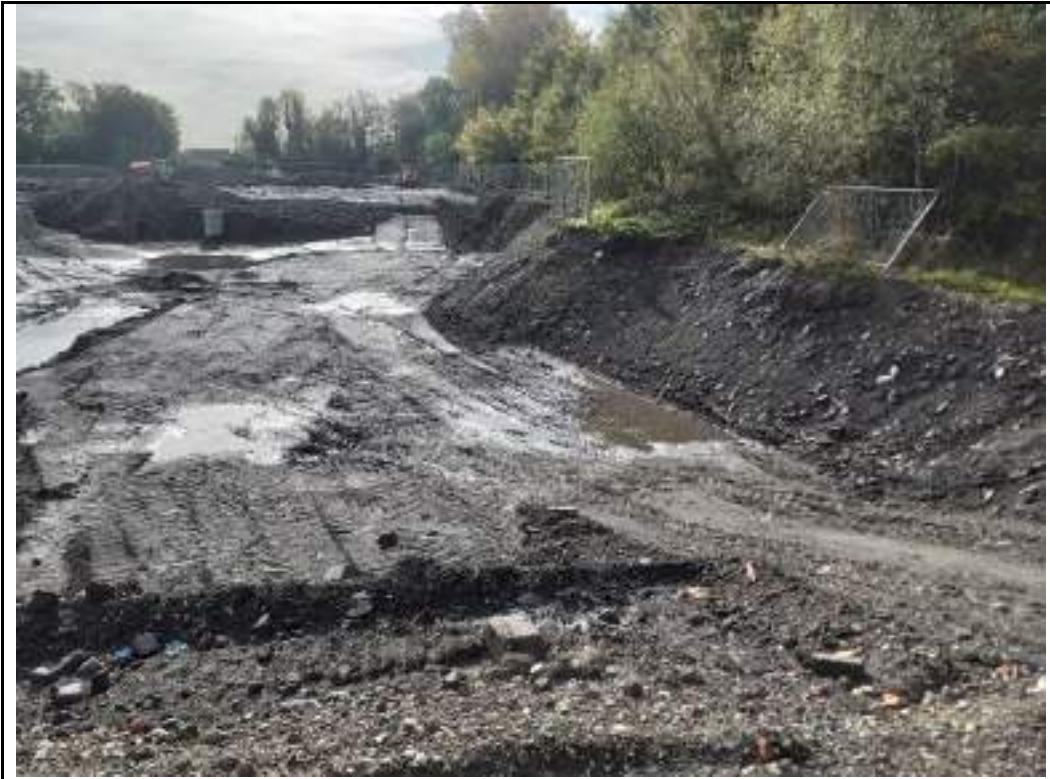
Photograph 93: Western boundary of the site. Looking towards the south.
