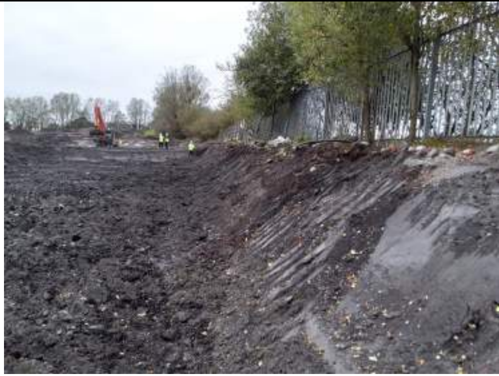
Photograph 5: Excavated peat area in northeastern part of the site and surveying of excavations.
