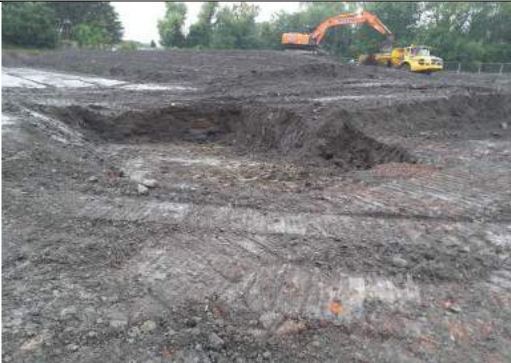
Photograph 20: Soft spot Excavation in southwestern part of the site.
