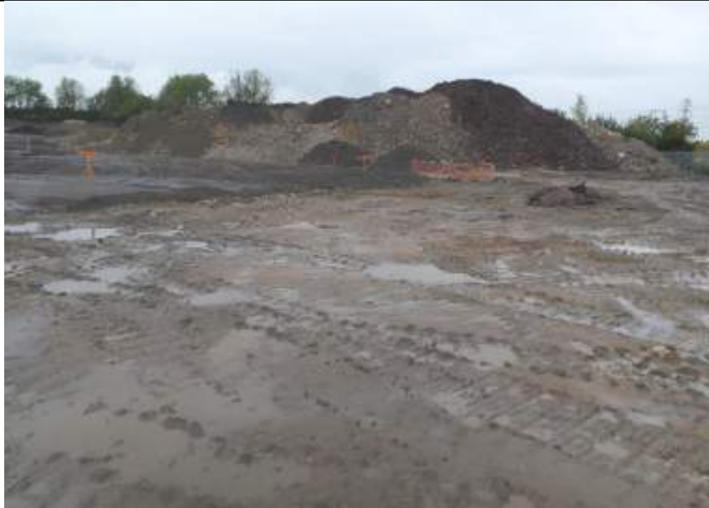
Photograph 14: Stockpile of general, granular and landfill Made Ground in northeastern part of the site. Looking towards the north.
