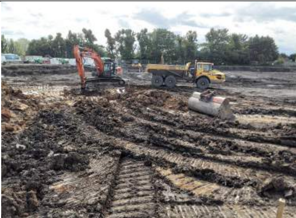
Photograph 22: Excavation of potentially TPH contaminated area in southeastern part of the site.
