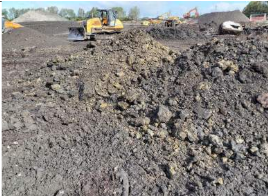
Photograph 136: Excavated material from southeast to backfill southern part of the site.
