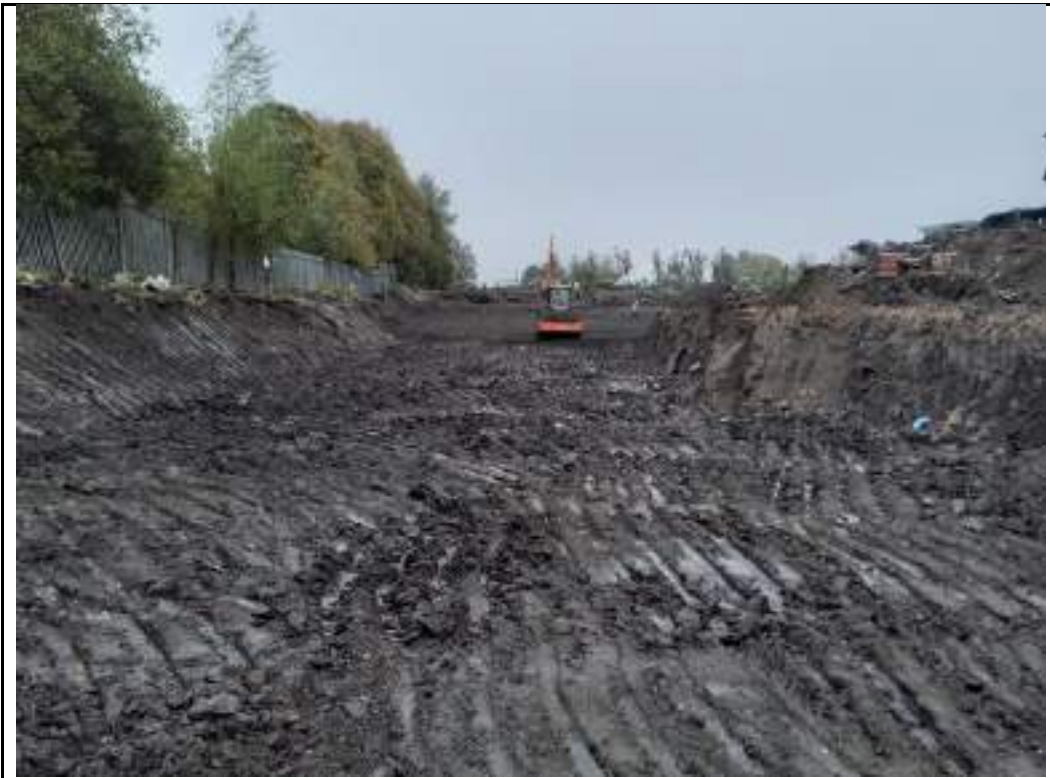
Photograph 14: Proof rolling of fill using sheepsfoot roller in northeast of the site.
