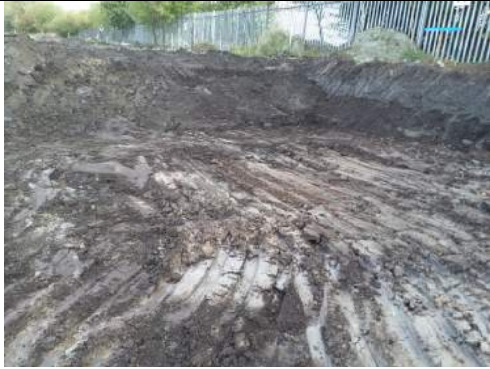
Photograph 5: Peat excavation in eastern boundary of the site (southern part of the culvert)
