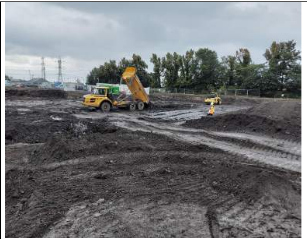
Photograph 12: Backfilling of soft spot excavation using crushed bricks as starter layer
