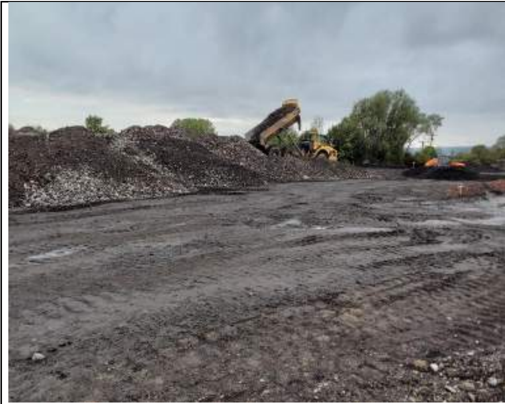
Photograph 91: Stockpiling crushed material in northwestern part of the site.
