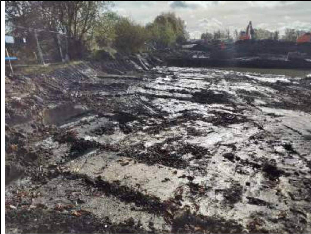
Photograph 19: Northeastern boundary of the site. Looking towards the south.
