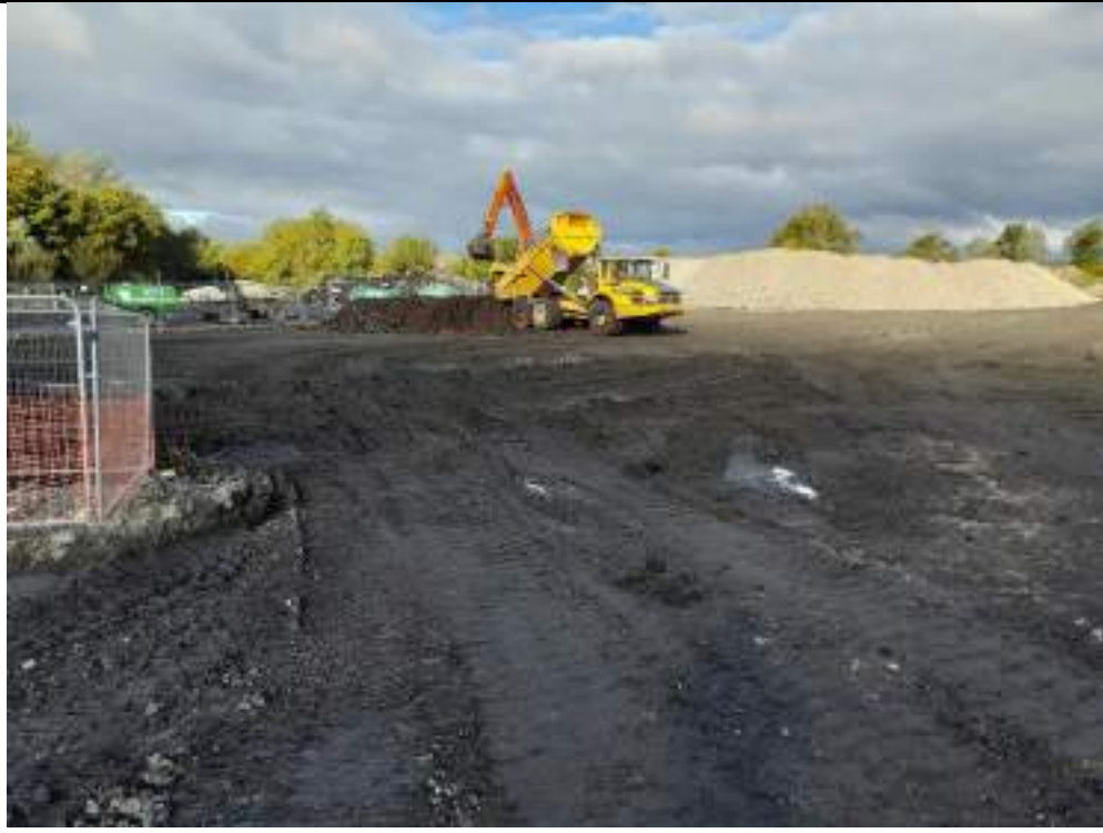
Photograph 5: Stockpiling excavated material from southeastern excavation in northwestern part of the site.
