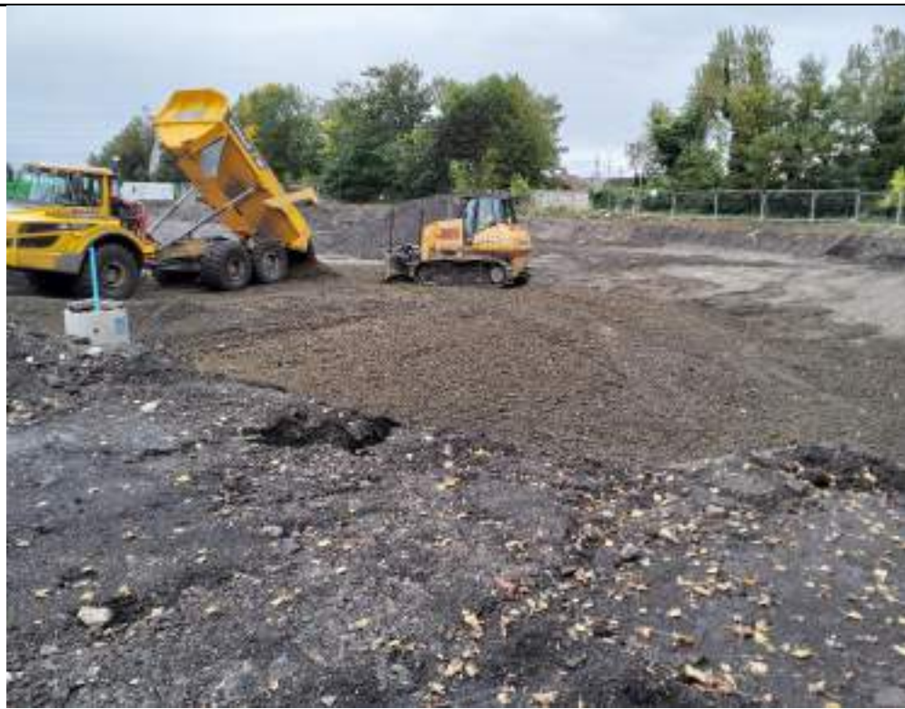
Photograph 8: Backfilling southwest of the site using granular material from northeastern stockpile.
