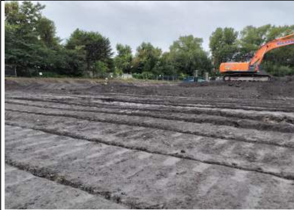
Photograph 23: Surveying of excavation in southern part of the site.
