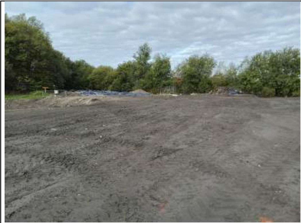
Photograph 113: TPH and asbestos contaminated stockpiles in northwestern part of the site.
