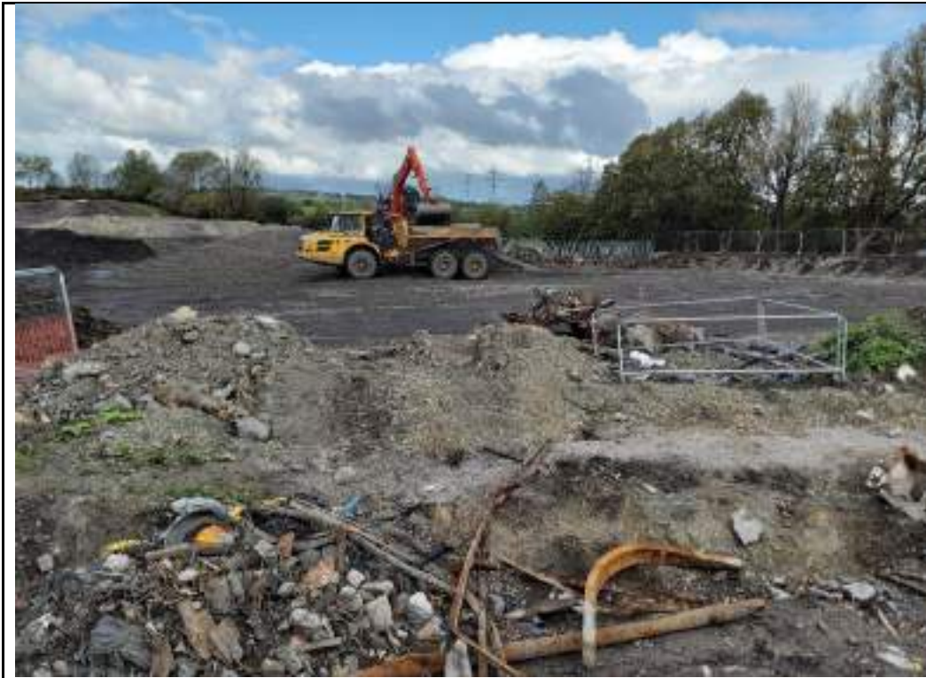
Photograph 21: transferring processed material from eastern stockpile to backfill southwestern part of the site.
