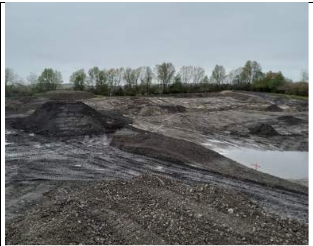
Photograph 12: Overview of stockpiles in northern part of the site.
