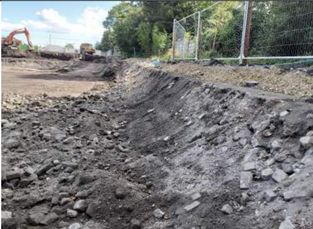
Photograph 136: Southern boundary of the site. Looking towards the east.
