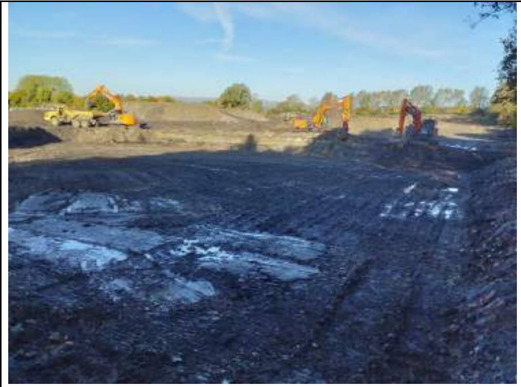
Photograph 3: Excavation of Made Ground in eastern part of the site.
