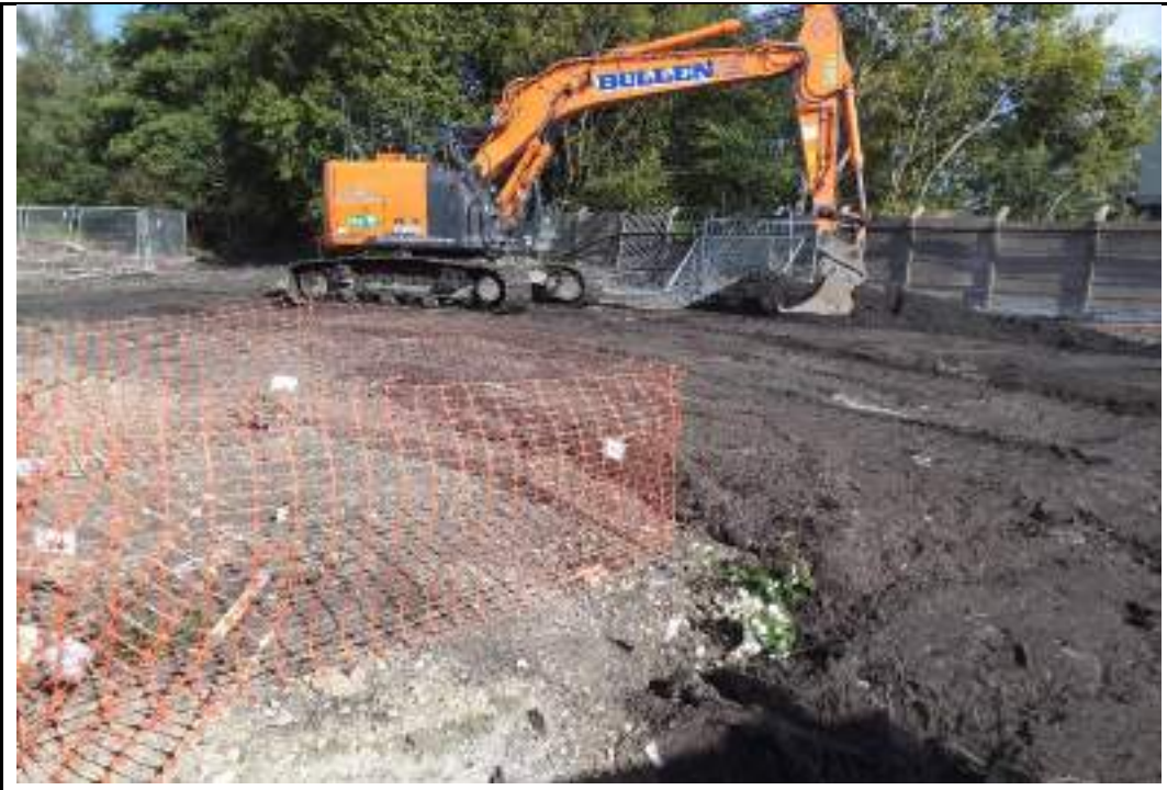
Photograph 11: Construction of shaft grouting platform in southeastern part of the site.
