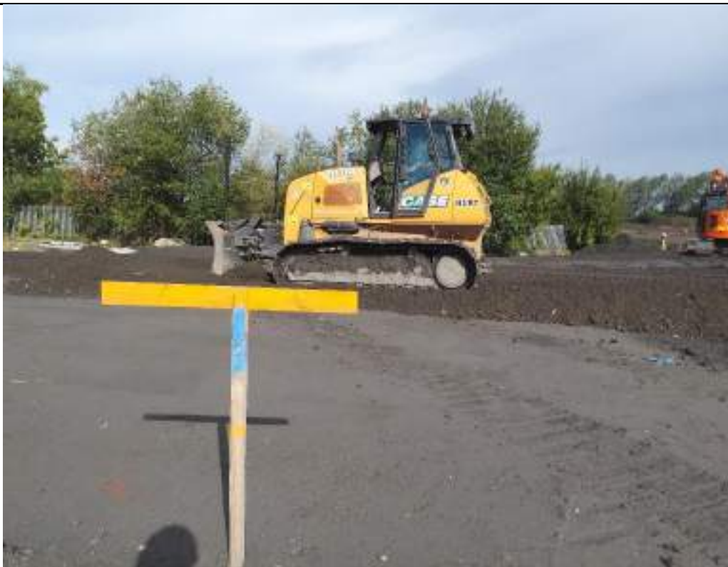
Photograph 136: Installed GPS on dozer to control ground level in northwest of the site.
