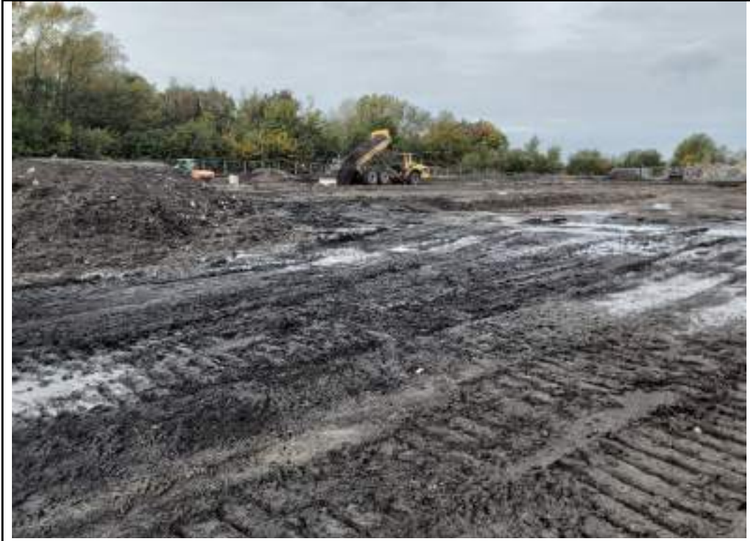
Photograph 23: Backfilling southwestern part of the site using excavated materials from eastern excavation.
