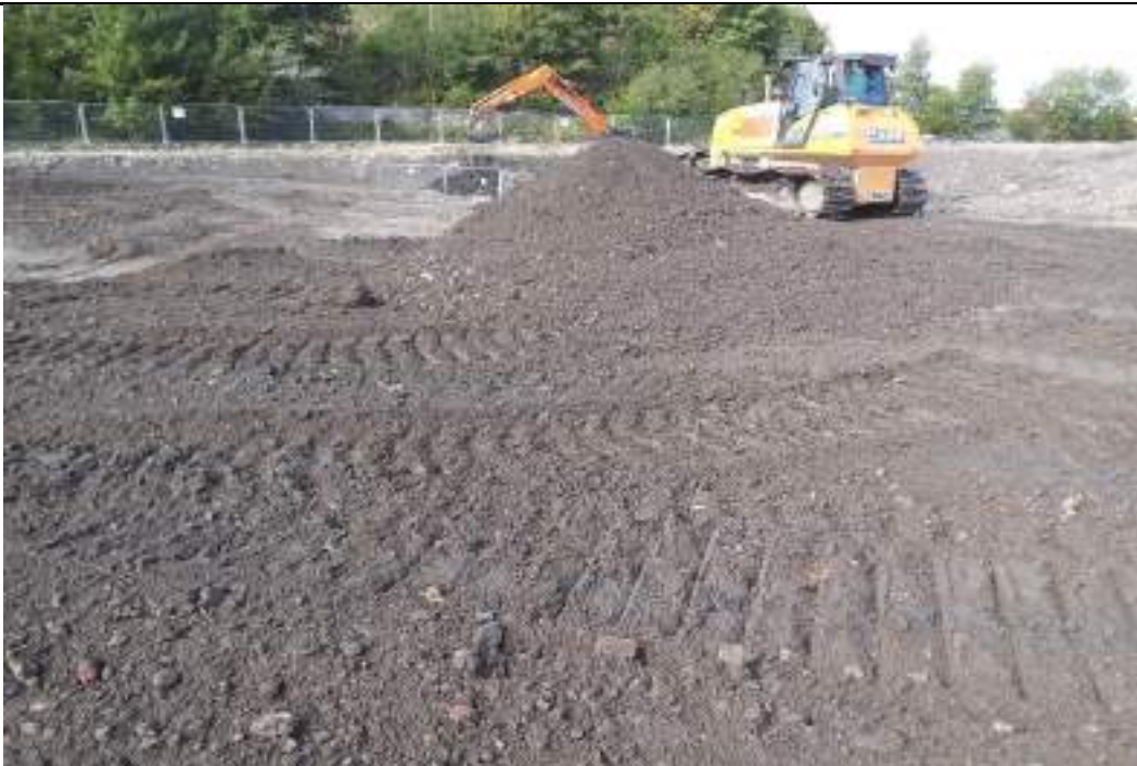
Photograph 28: Dozer pushing processed fill material in southwestern part of the site.
