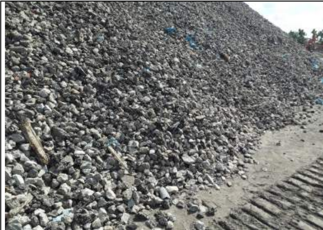
Photograph 169: Wood and plastic in crushed concrete and asphalt stockpile in northwest of the site. VHE to provide constituent parts testing
