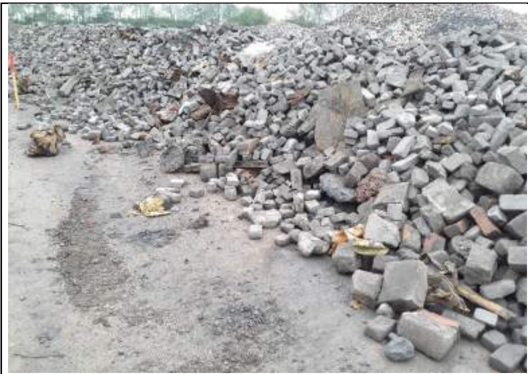
Photograph 14: Deleterious material in bricks stockpile in northwestern part of the site.
