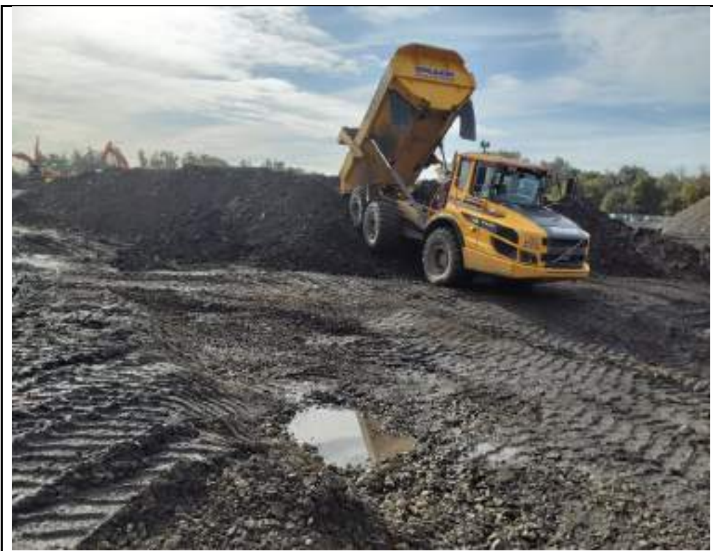
Photograph 10: Stockpiling excavated materials from eastern part of the site in northeastern stockpile.
