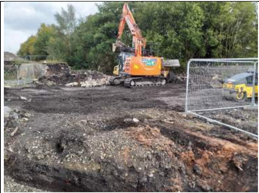
Photograph 4: Excavation of concrete in eastern part of the site.
