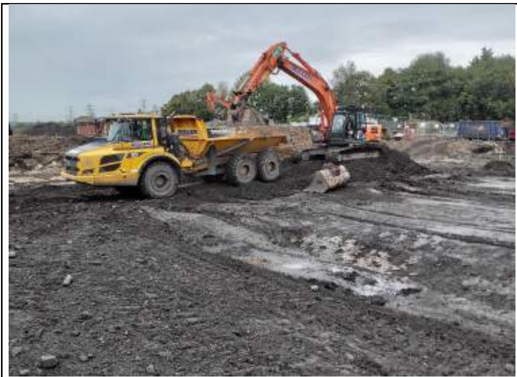
Photograph 2: Excavation of landfill Made Ground in southeastern part of the site.
