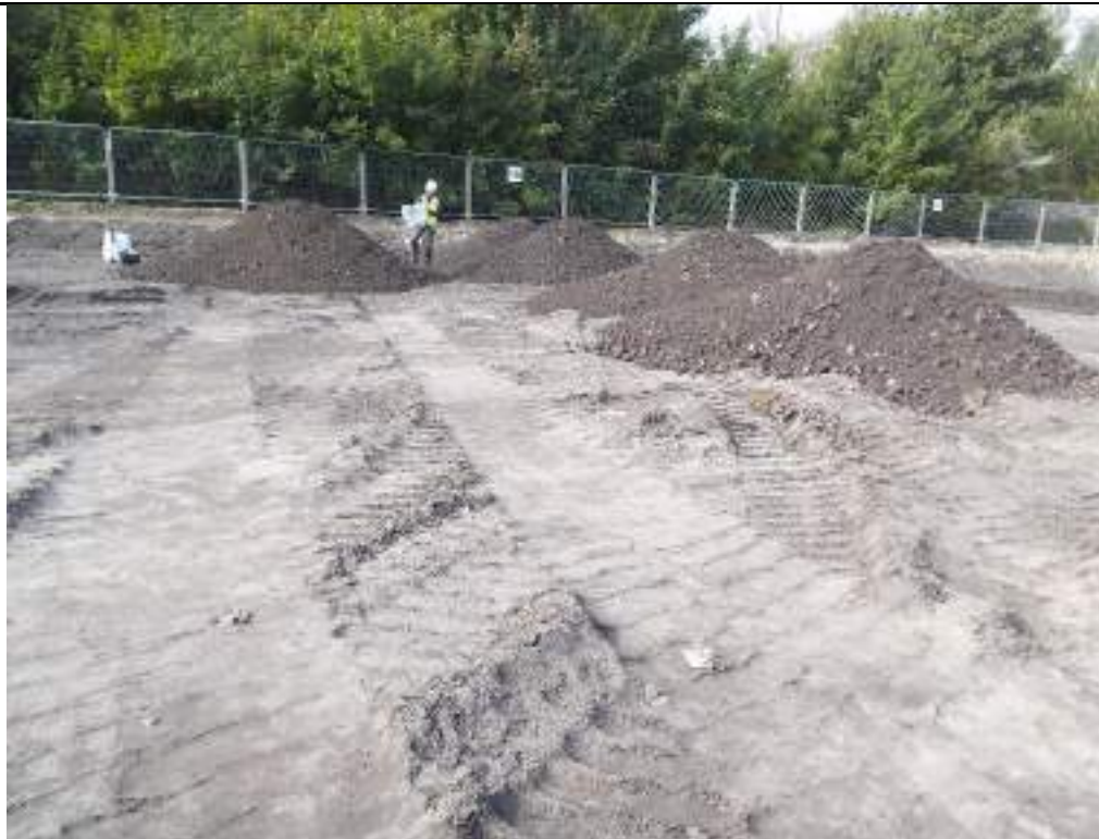
Photograph 26: Collection of geotechnical samples from fill material in western part of the site. Processed material from eastern stockpile.
