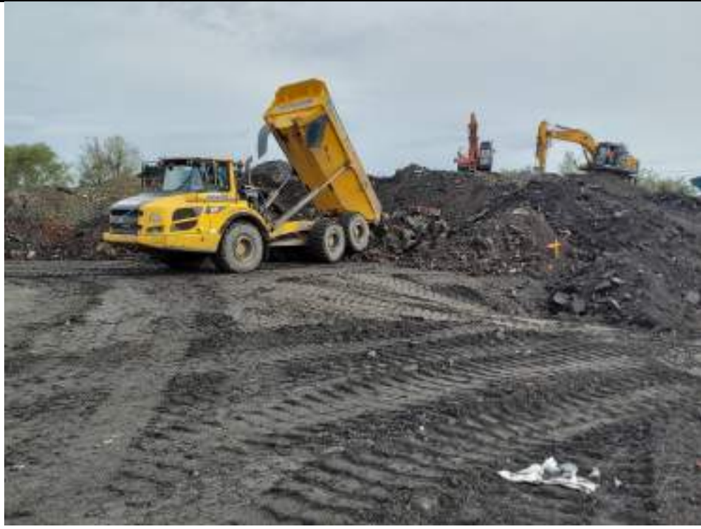
Photograph 5: Unloading excavated concrete from eastern part of the site in northeastern stockpile.
