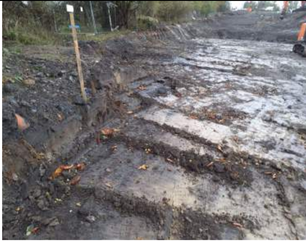
Photograph 7: Excavation of organic Made Ground area up to formation level in northeast of the site.
