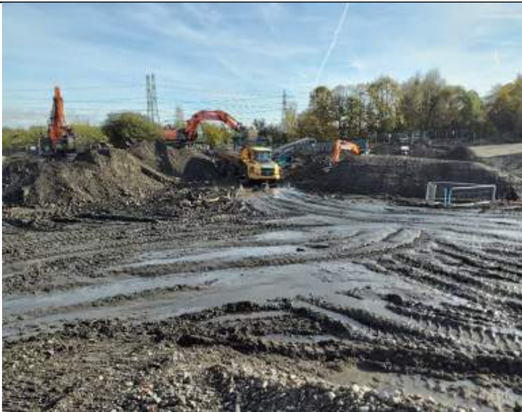
Photograph 16: Loading oversized materials to stockpile in northwestern stockpile.
