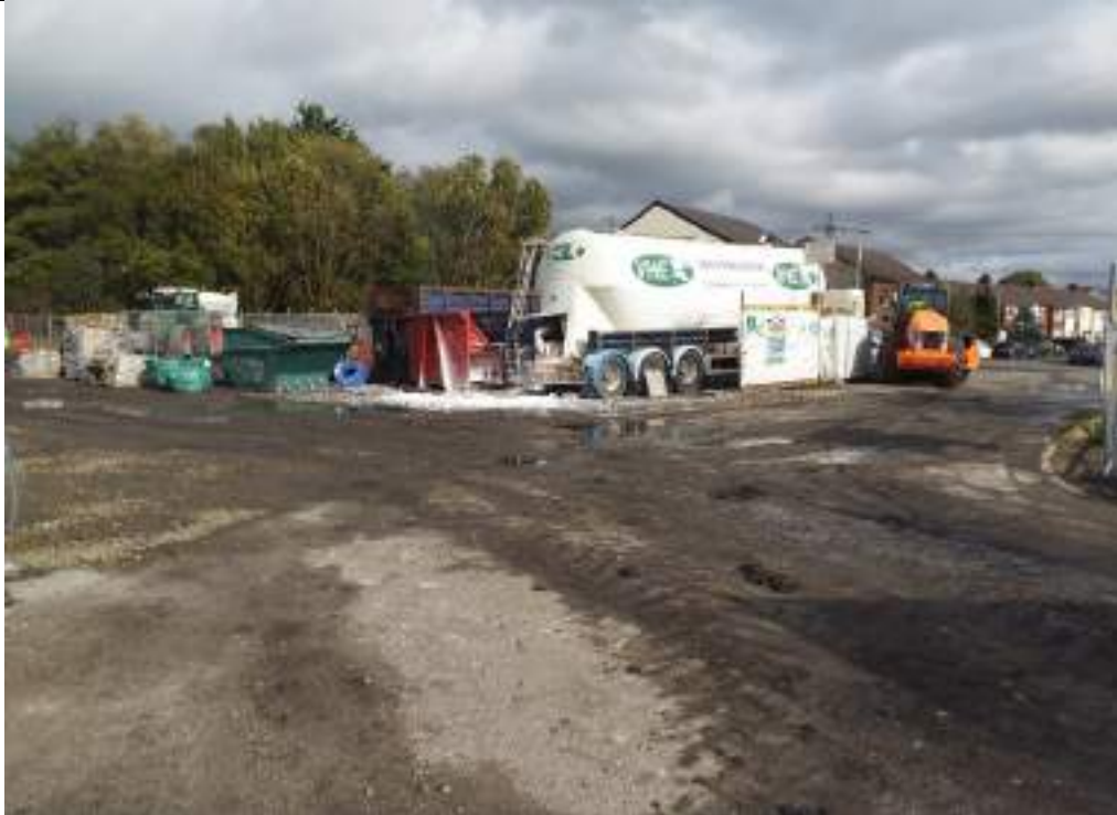
Photograph 22: Lime modification storage tanker in southeastern part of the site.
