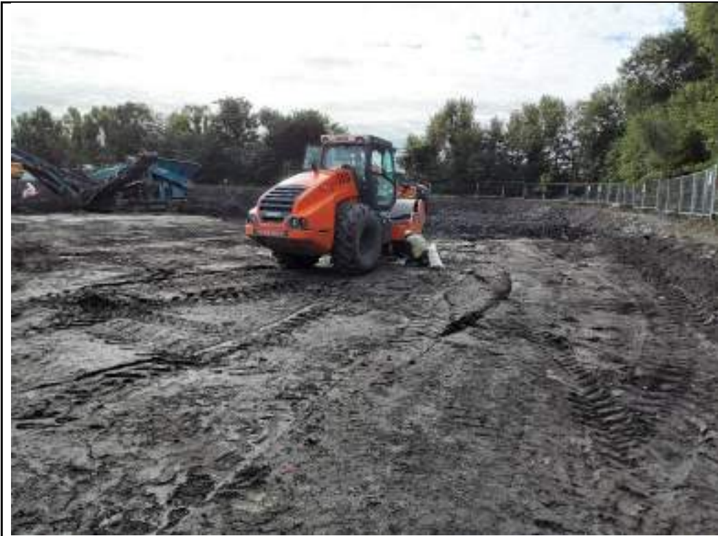
Photograph 147: Plate load testing in western part of the site.
