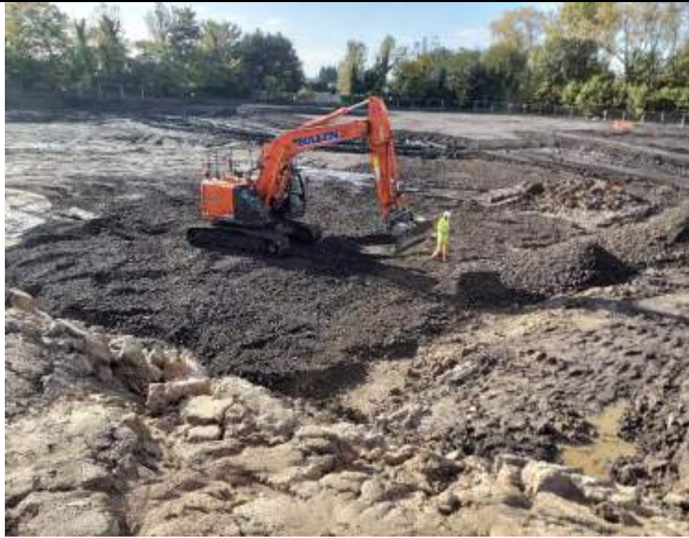
Photograph 7: Placing crushed fill material from northwestern stockpile in the southeast.
