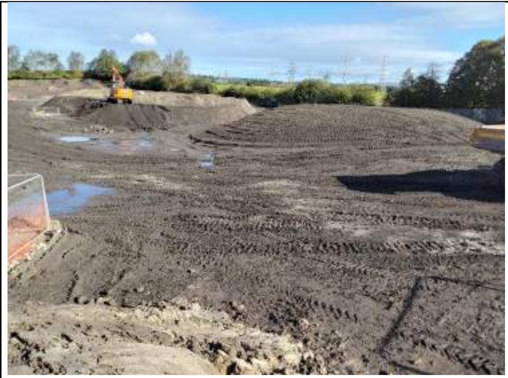
Photograph 3: Stockpiles of processed and excavated materials in eastern and northeastern part of the site.
