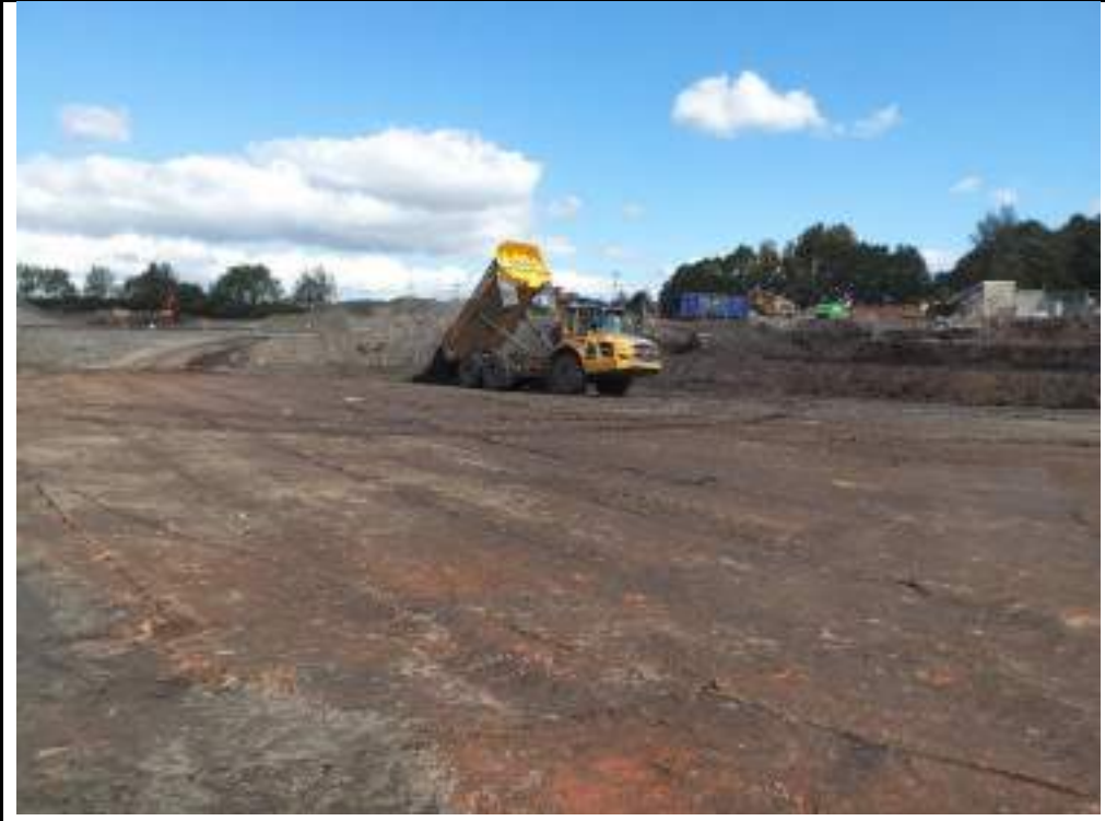
Photograph 3: Backfilling of central part of the site using excavated material from south of the site.
