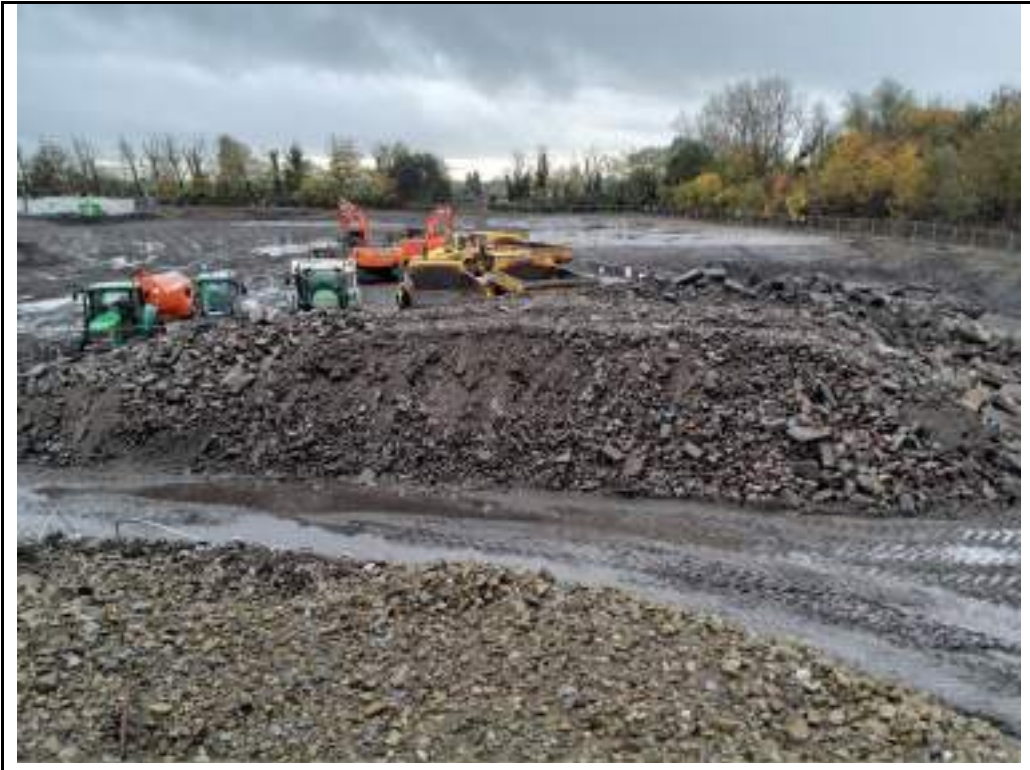
Photograph 9: Stockpile of concrete and oversized materials in northwestern part of the site.
