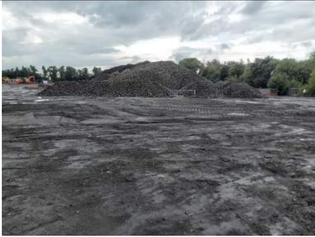
Photograph 11: Crushed concrete and asphalt stockpile in northwest of the site. Looking towards the south.
