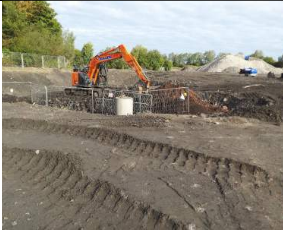
Photograph 7: Hand picking of asbestos in western part of the site
