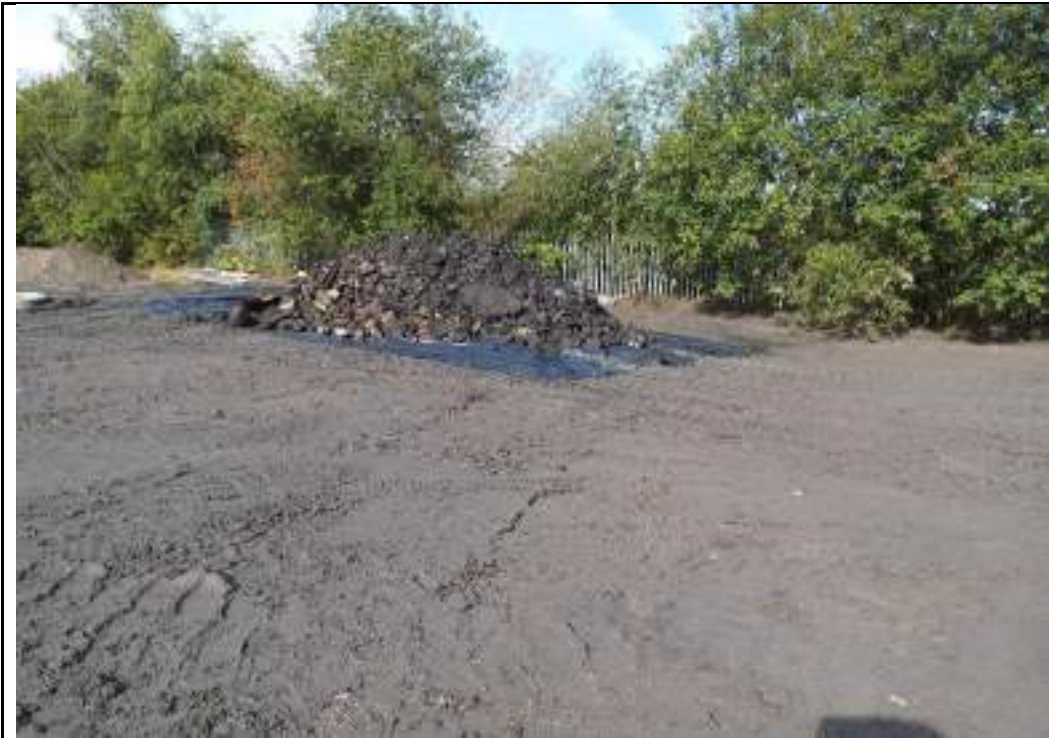
Photograph 91: Stockpile of potentially asbestos contaminated material in northwest of the site. Material from excavation in southeastern part of the site.
