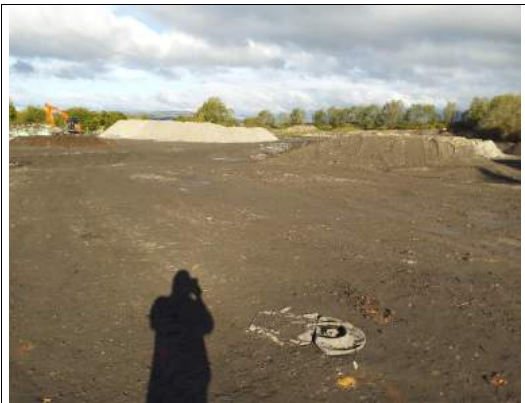
Photograph 12: Overview of stockpiles in northern part of the site. Looking towards the North.
