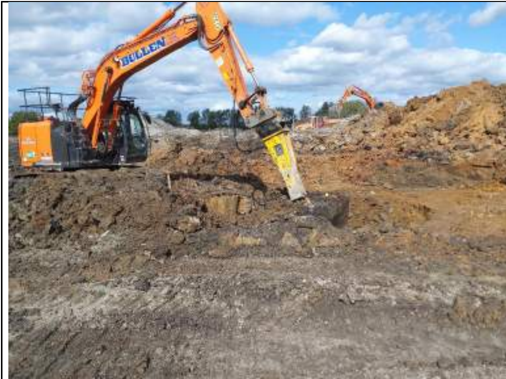
Photograph 25: Breaking concrete in southeastern part of the site.
