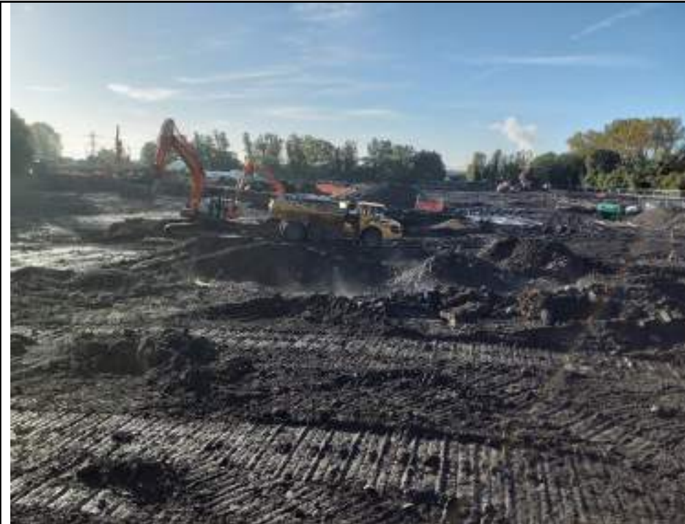
Photograph 1: Overview of the site. Looking towards the south.
