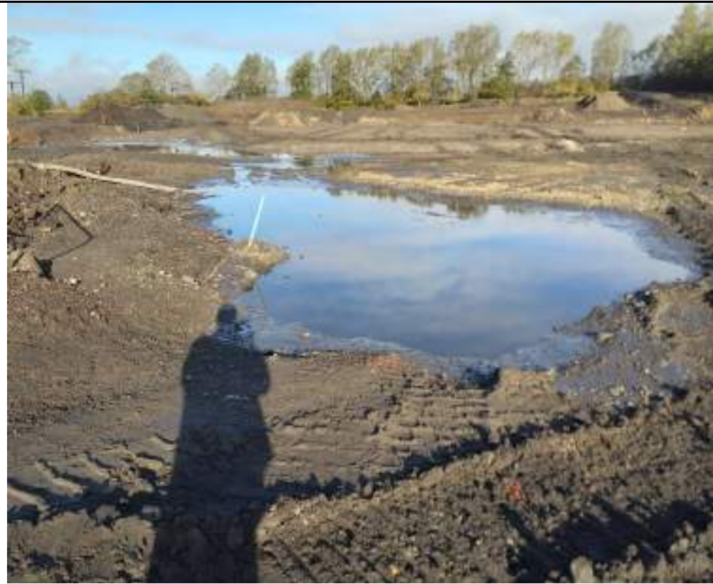
Photograph 9: Standing water in northern part of the site.
