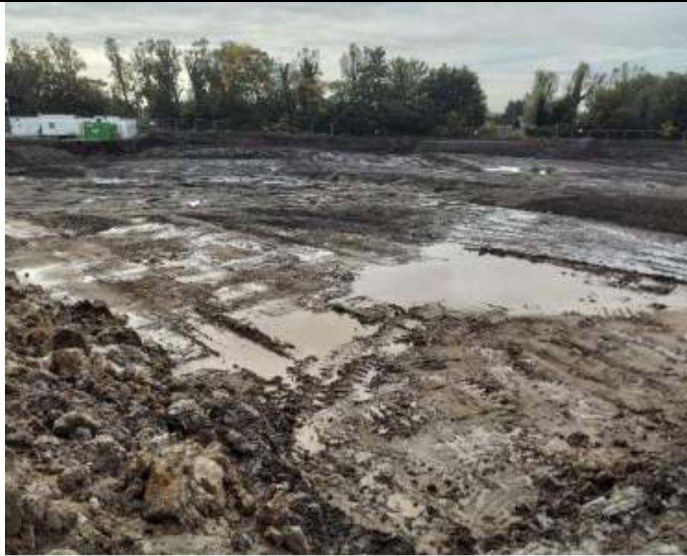
Photograph 7: Standing water in southeastern part of the site.
