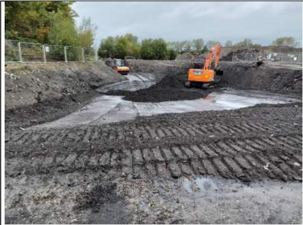
Photograph 93: Proof rolling of fill material in western part of the site.
