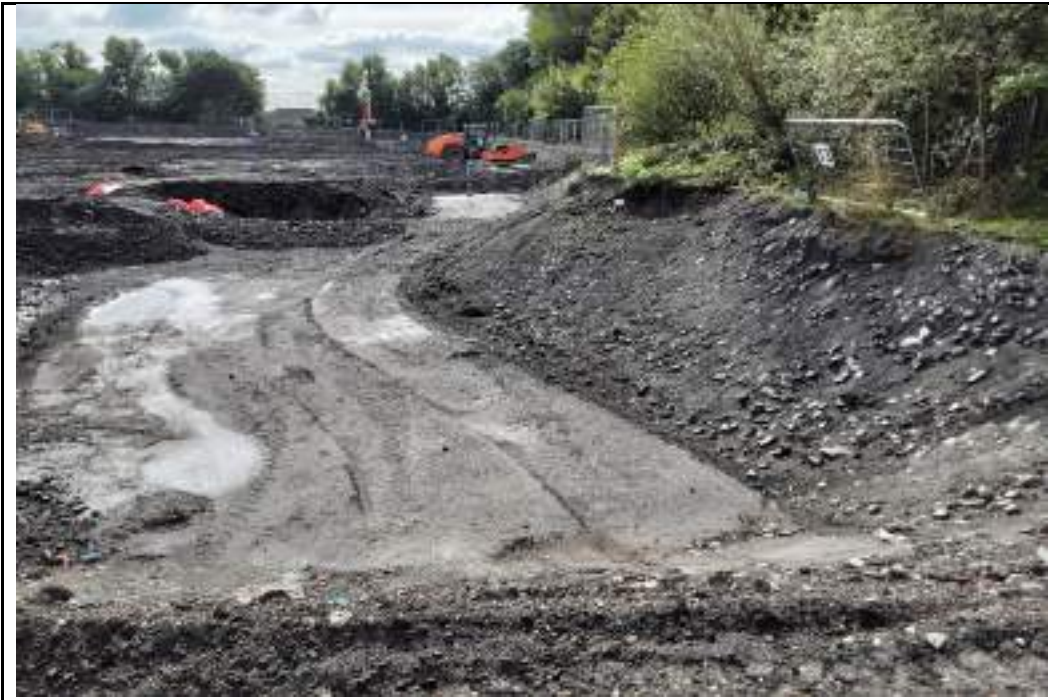
Photograph 21: Western boundary of the site. Looking towards the south.
