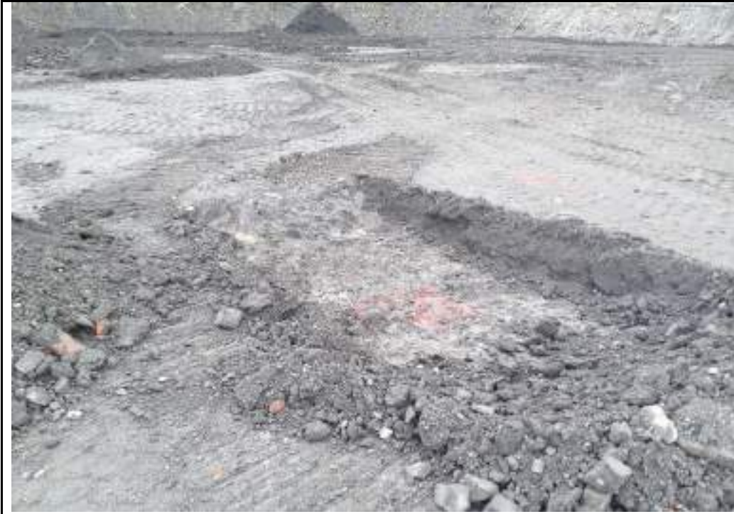
Photograph 25: Locations of NDM tests on fill material in southwest of the site.
