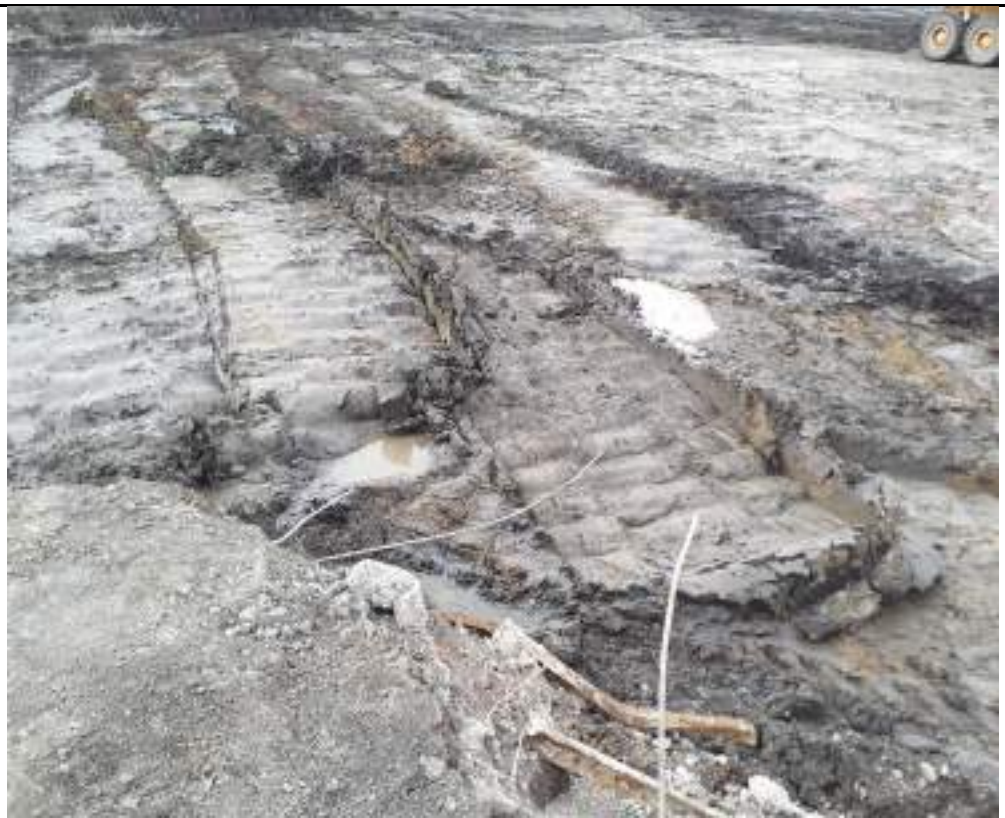
Photograph 8: Soft spot in southeastern part of the site.
