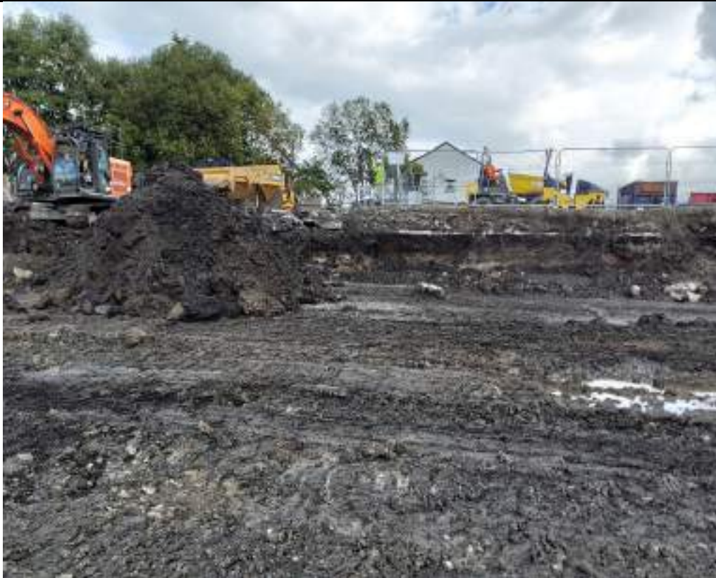
Photograph 20: Surveying of excavations in southeastern part of the site.
