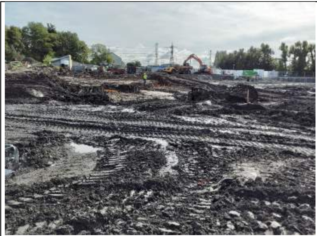
Photograph 14: Surveying of excavations in southeastern part of the site.
