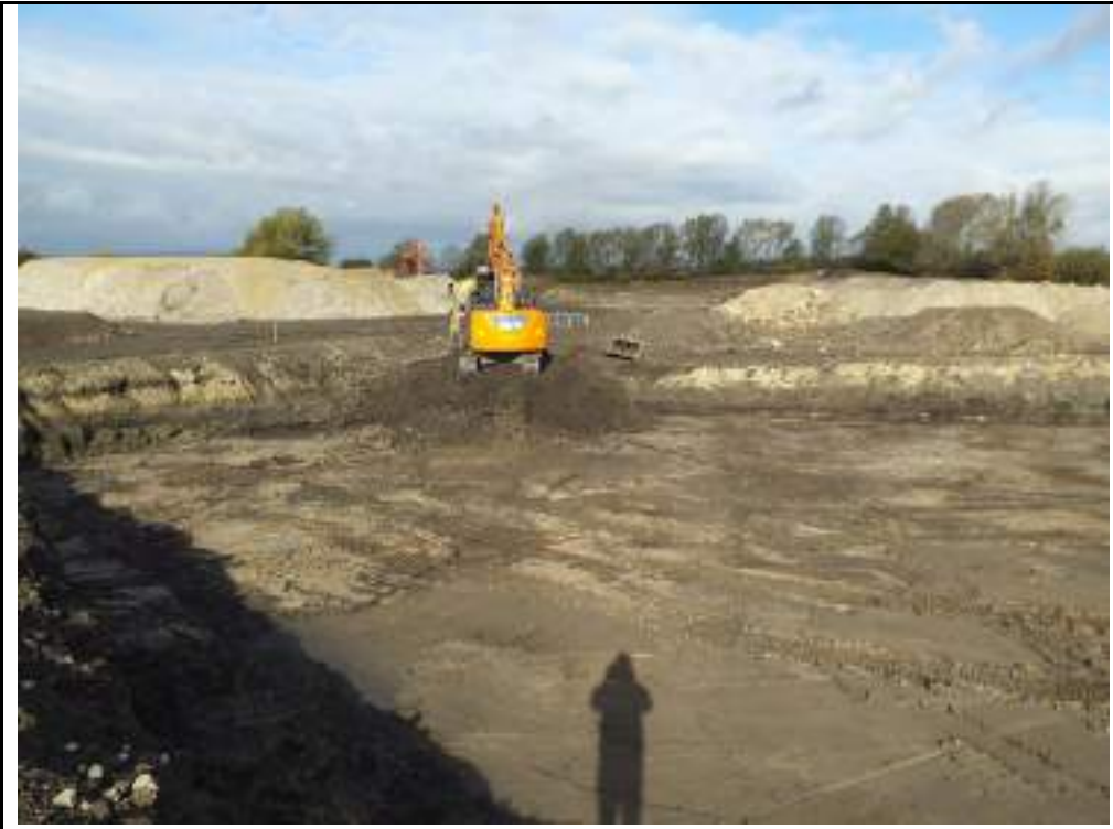
Photograph 3: Excavation of discovered peat in eastern part of the site (southern part of the culvert).
