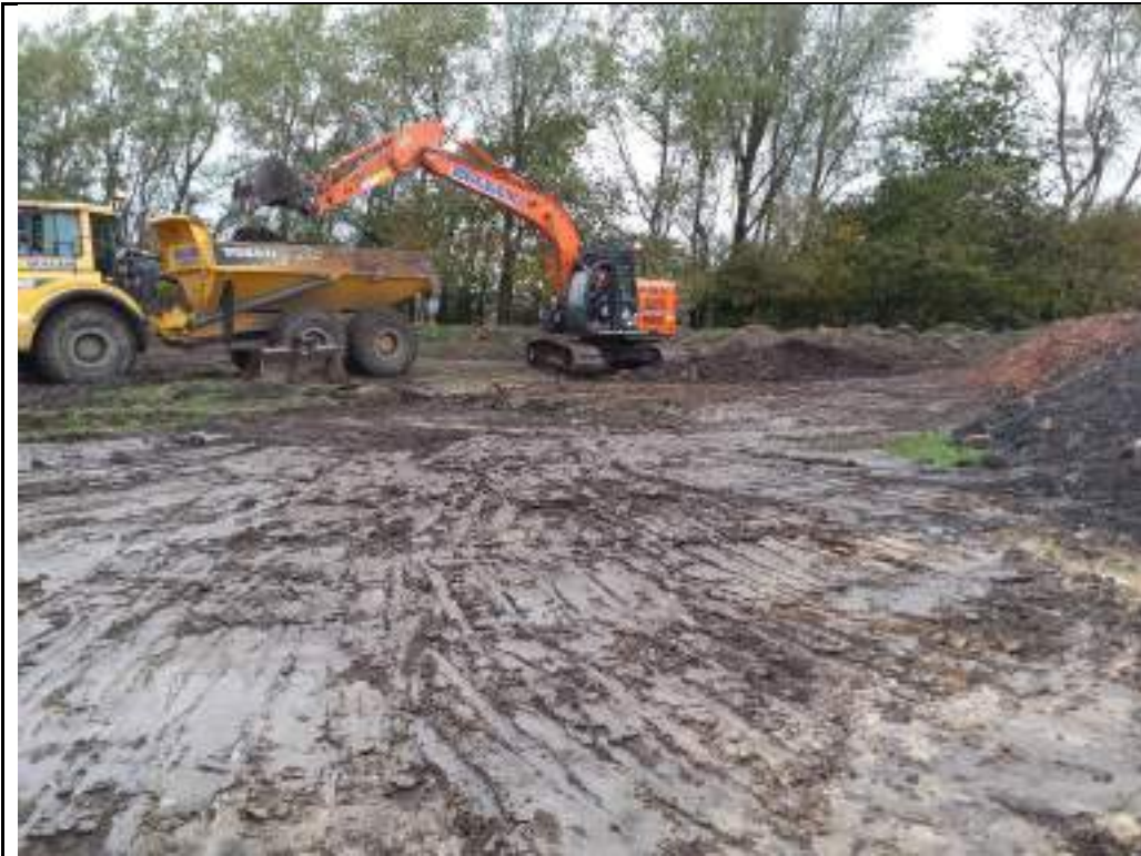
Photograph 17: Transferring stockpile of soft spot material from the north to the northwest.
