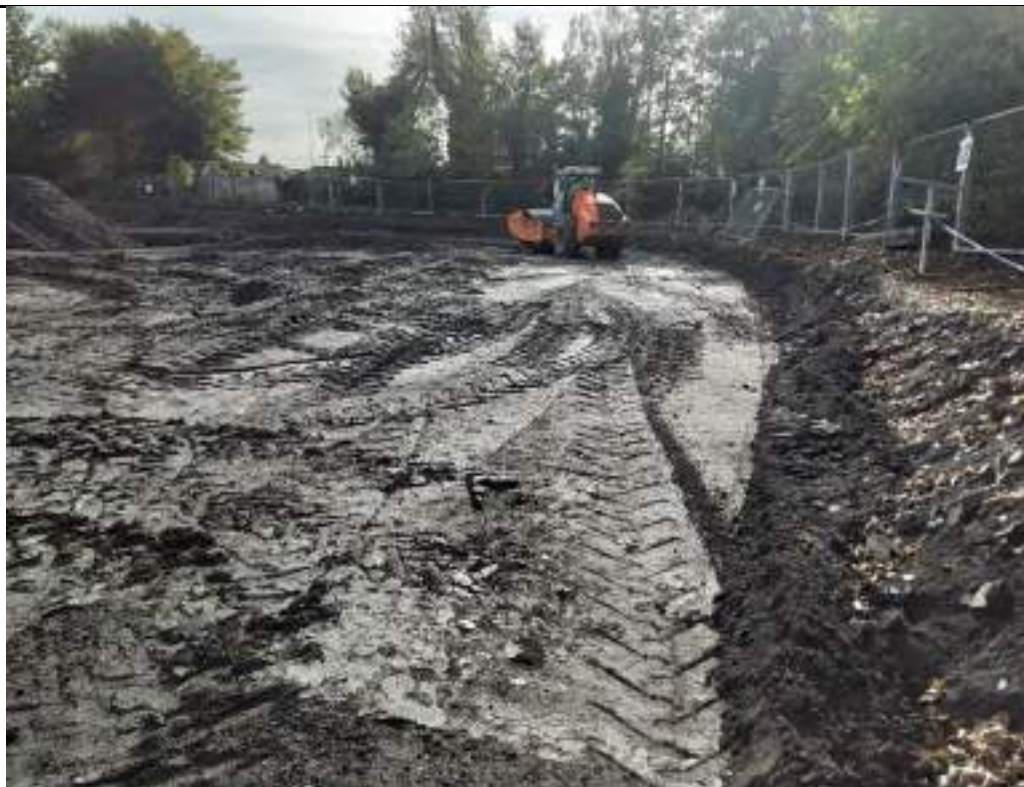
Photograph 16: Proof rolling over fill material in southwestern part of the site.
