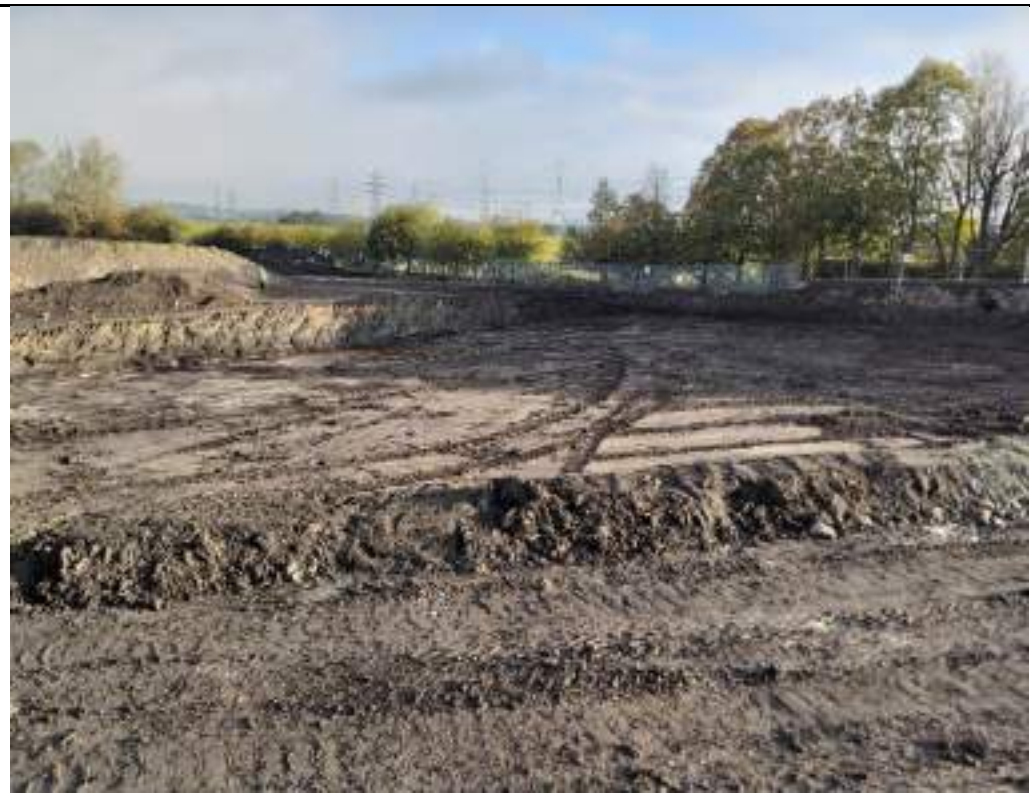
Photograph 10: Surveying of excavations and stockpiles.
