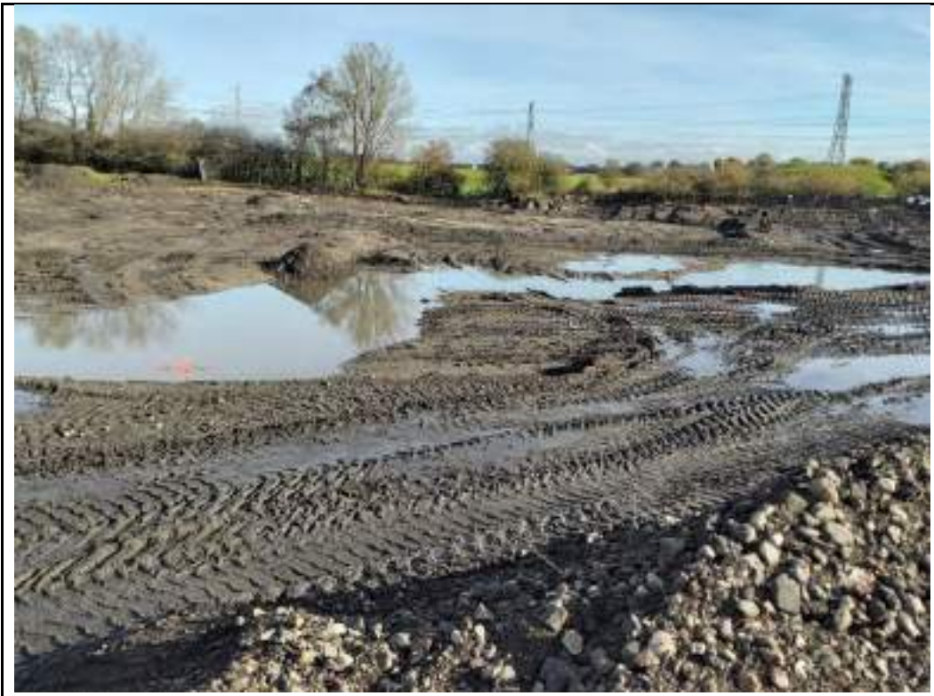
Photograph 14: Standing water in northern part of the site.
