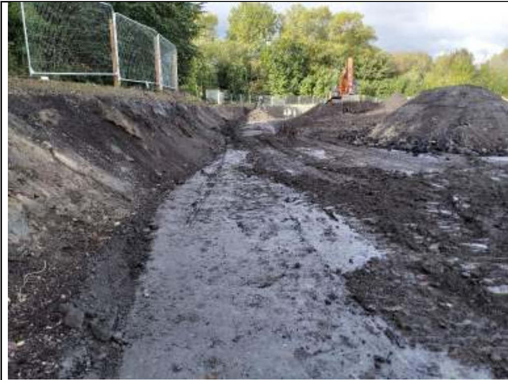
Photograph 17: Southern boundary of the site. Looking towards the west.
