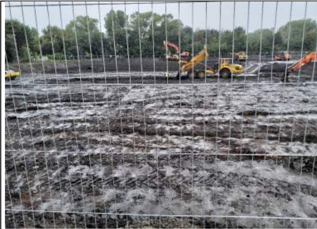
Photograph 17: Backfilling of soft spot excavation using general fill as base material.
