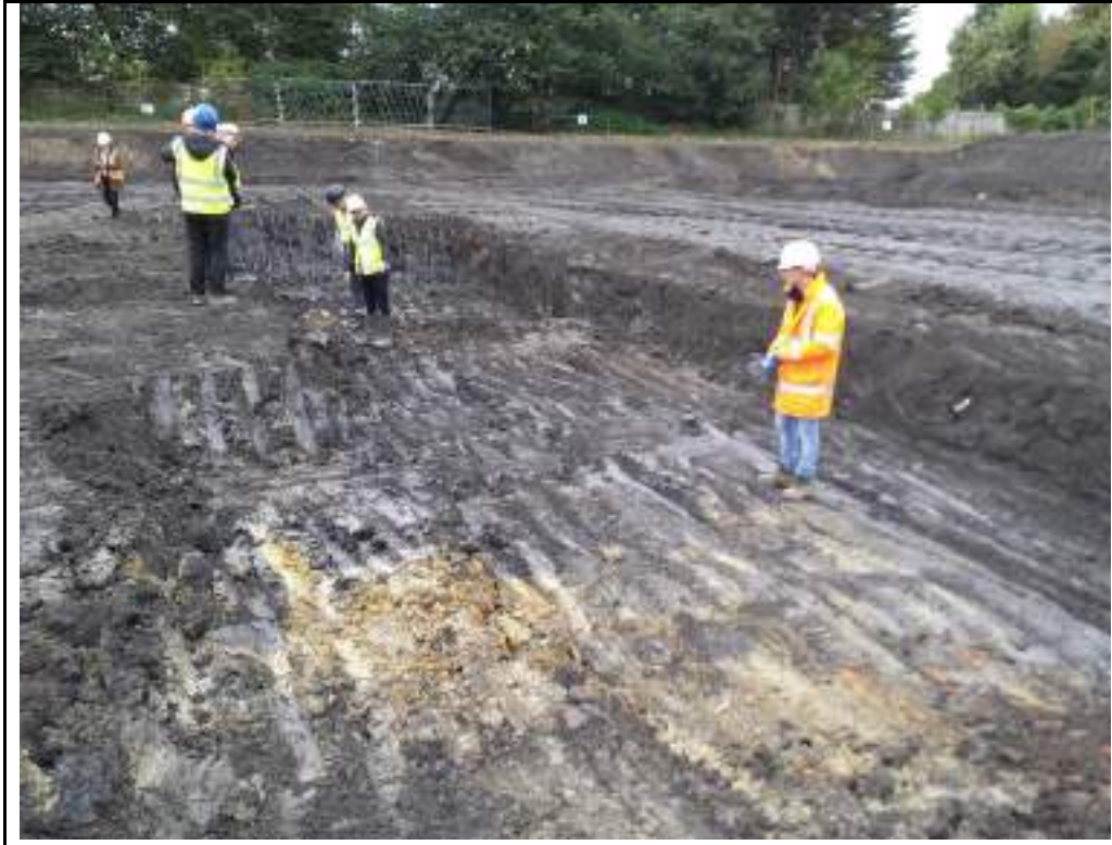
Photograph 9: Soft spot excavation in southern part of the site.
