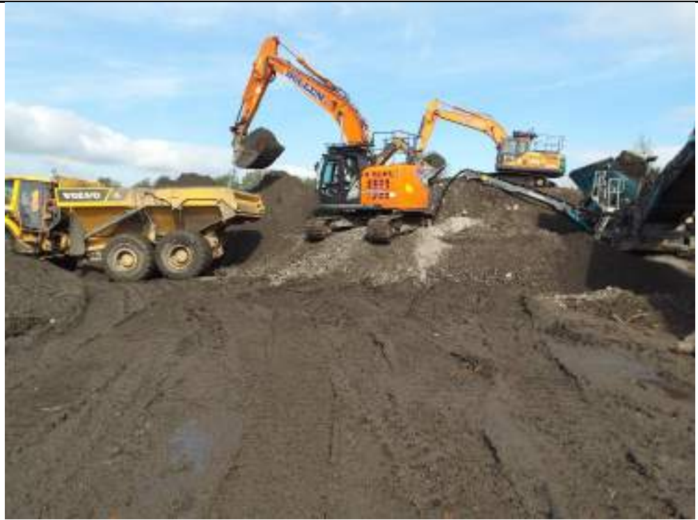
Photograph 6: Loading undersize material from screener to backfill southwest of the site.
