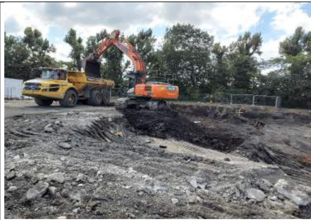
Photograph 2: Excavation of landfill Made Ground in south of the site.
