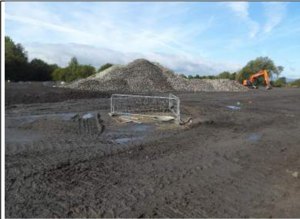
Photograph 27: Stockpile of crushed concrete in northwest of the site.
