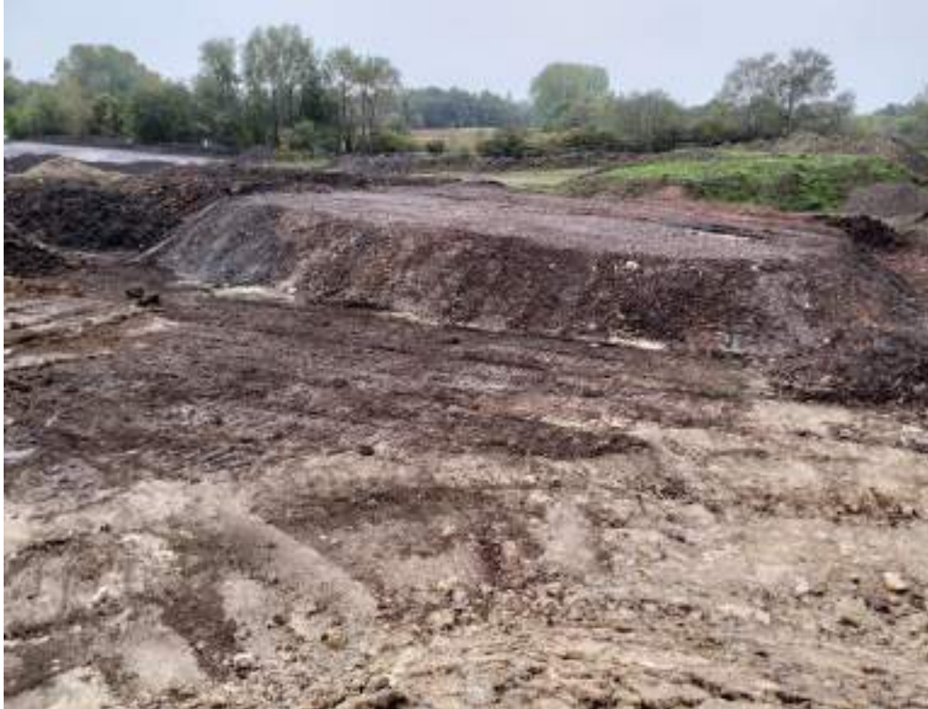
Photograph 16: Topsoil stockpile in northern part of the site.
