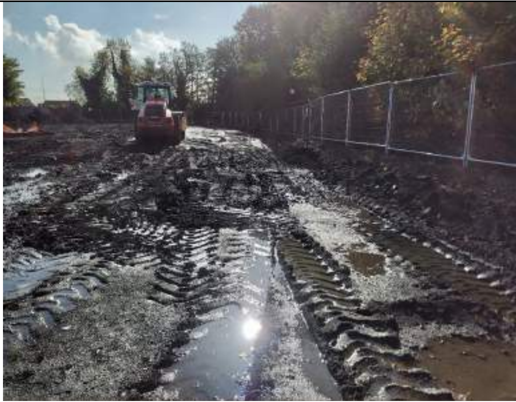
Photograph 21: Proof rolling of fill materials using smooth roller in southwestern part of the site.
