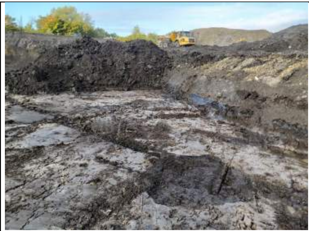
Photograph 4: Discovered peat in eastern part of the site (southern part of the culvert).
