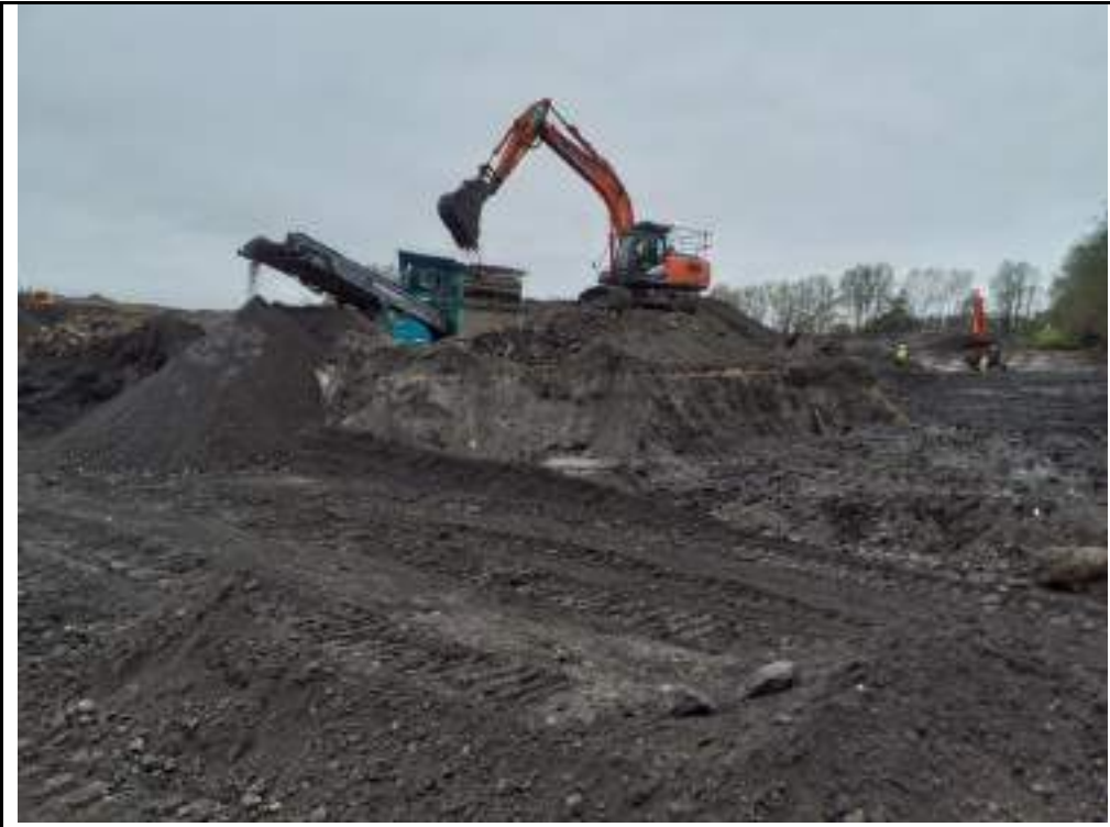
Photograph 3: Screening of stockpiled Made Ground material in northeastern part of the site.
