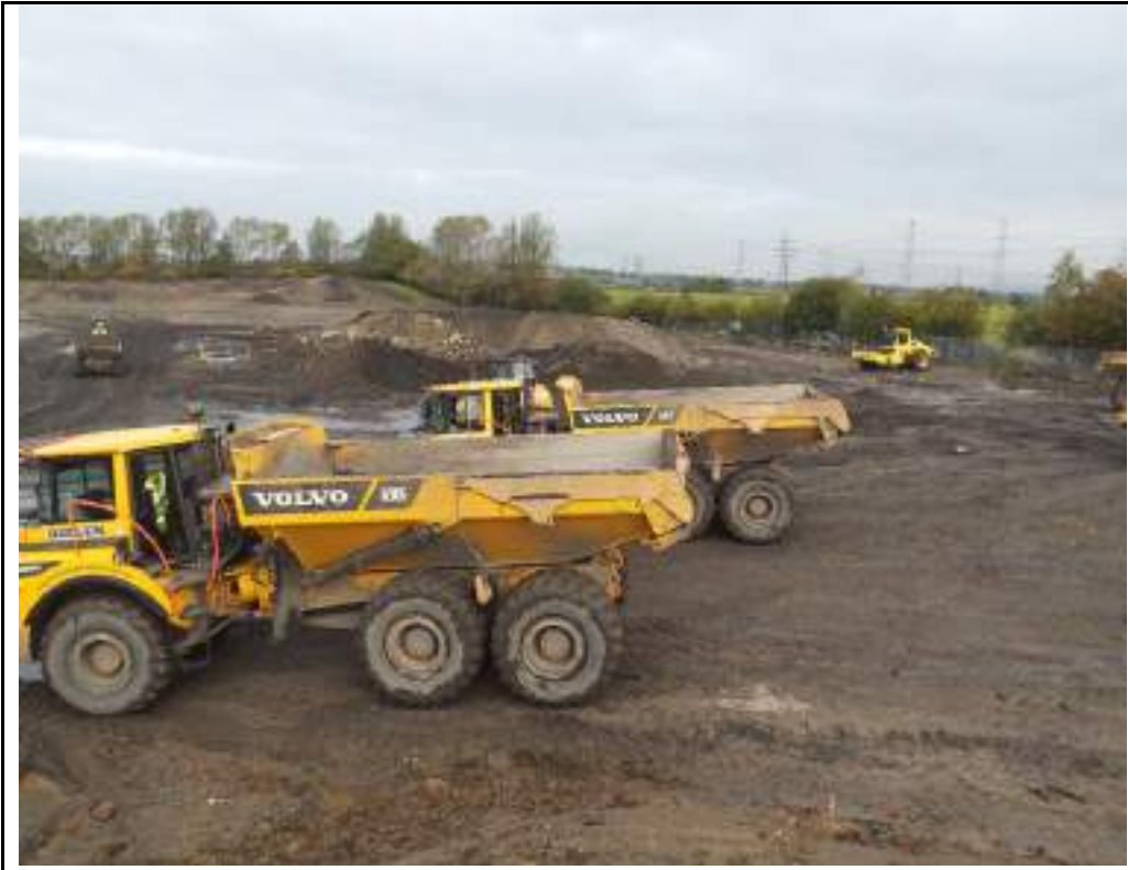
Photograph 9: Overview of northeastern stockpiles.
