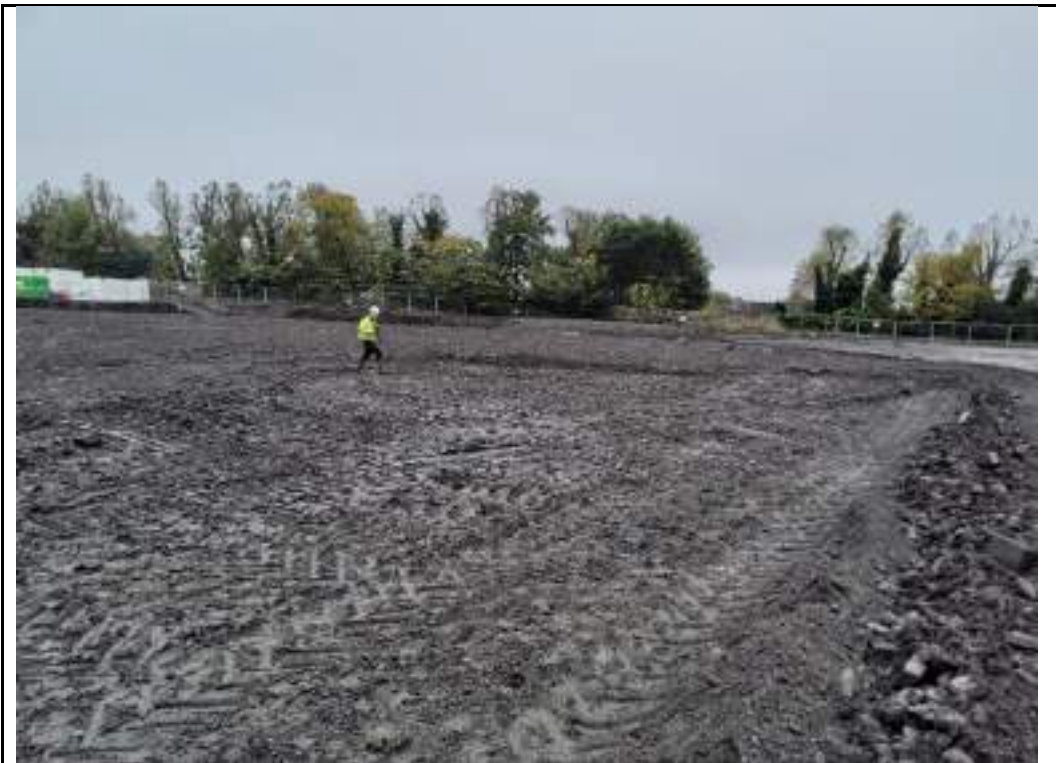
Photograph 10: Surveying of the site.
