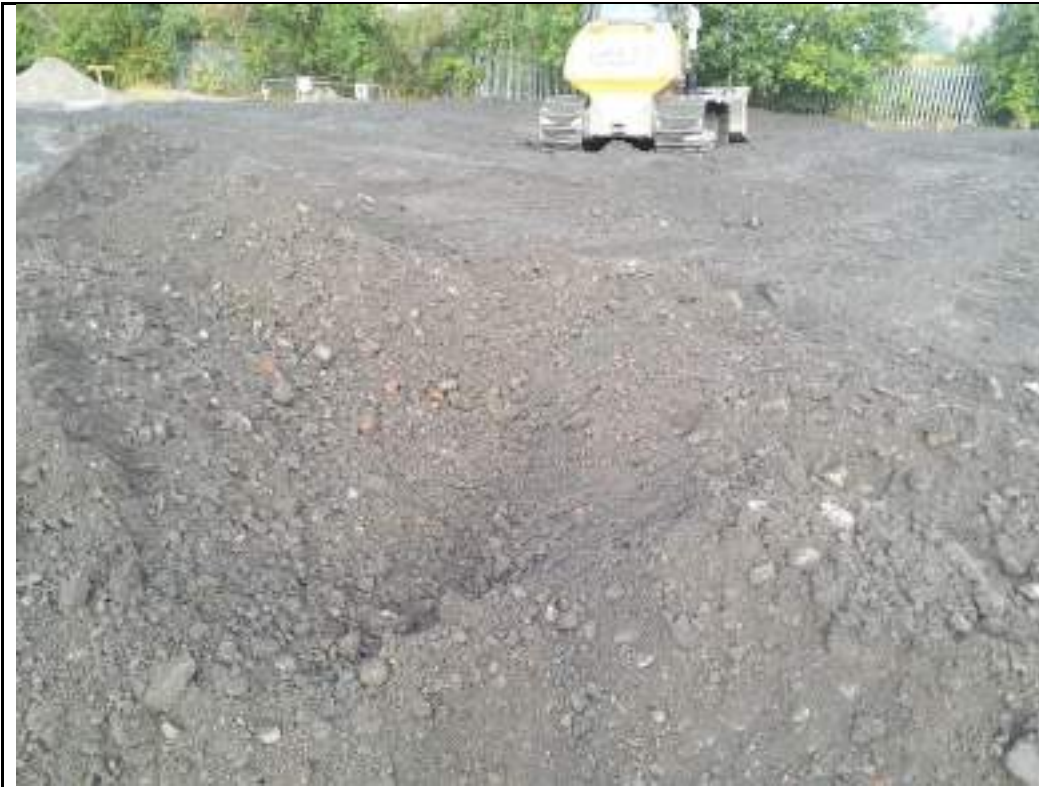
Photograph 125: Fill material in northwest of the site with improved quality.
