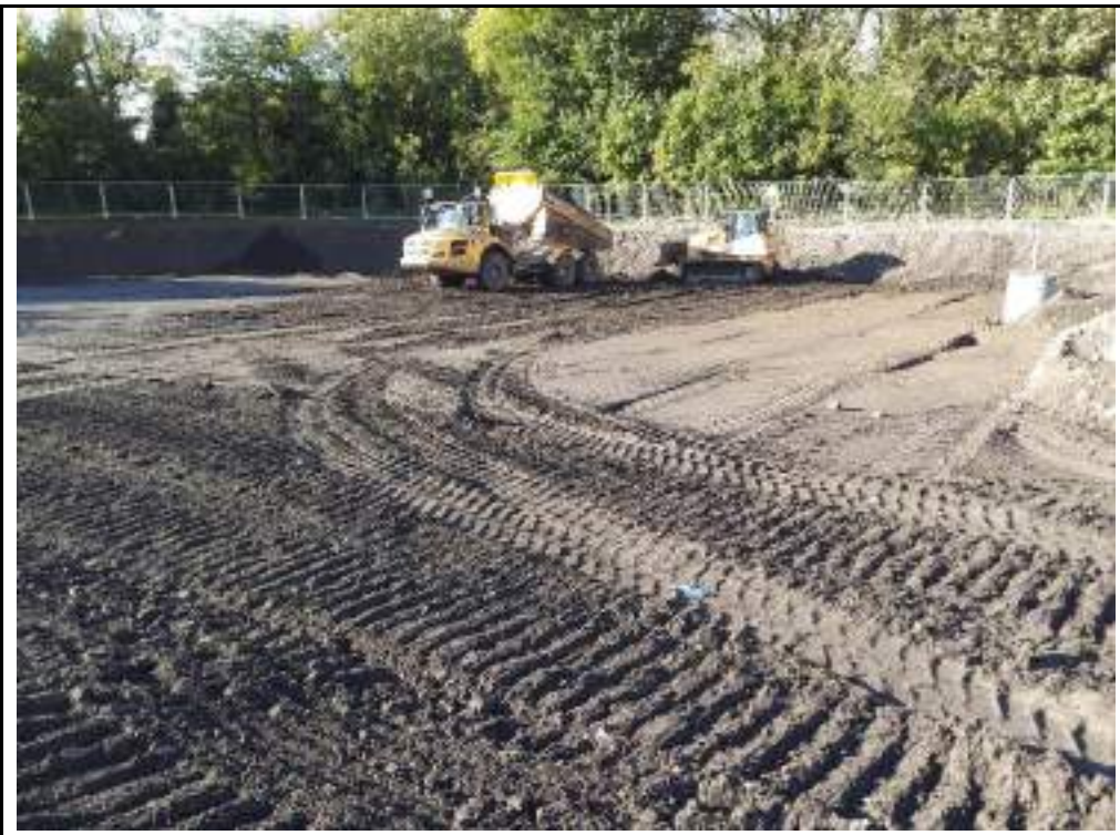
Photograph 4: Backfilling of southwestern part of the site using excavated material from southern part of the site.
