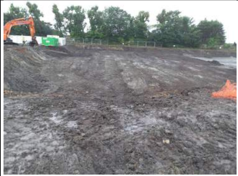
Photograph 3: Battered excavation in southern part of the site.
