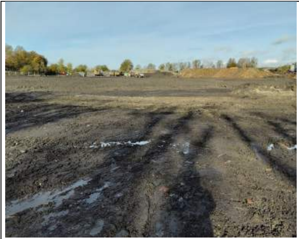
Photograph 10: Overview of backfilled area in southern part of the site. Looking towards the northwest.
