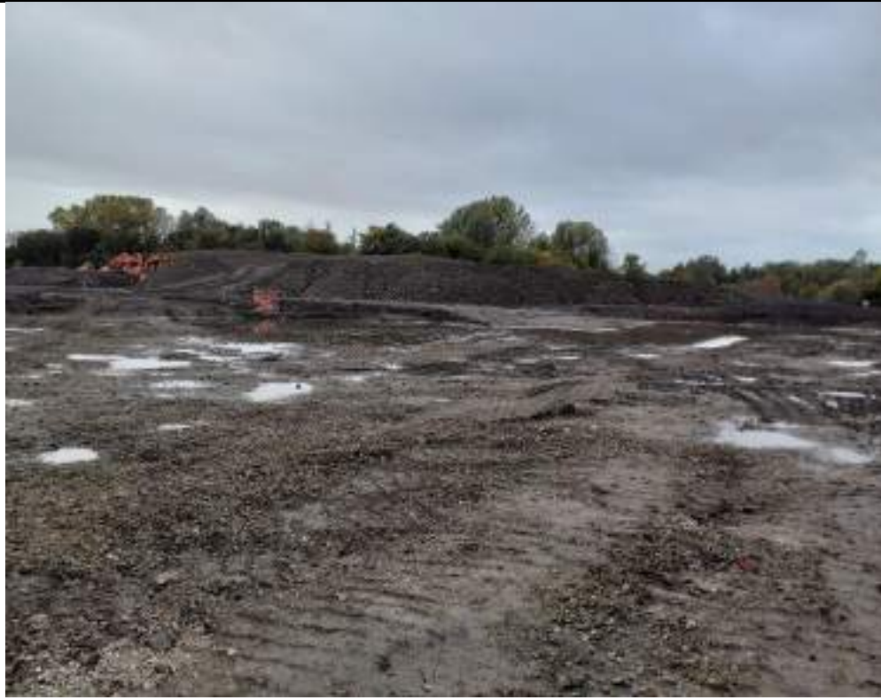
Photograph 7: Stockpile of crushed and granular material in northwestern part of the site.
