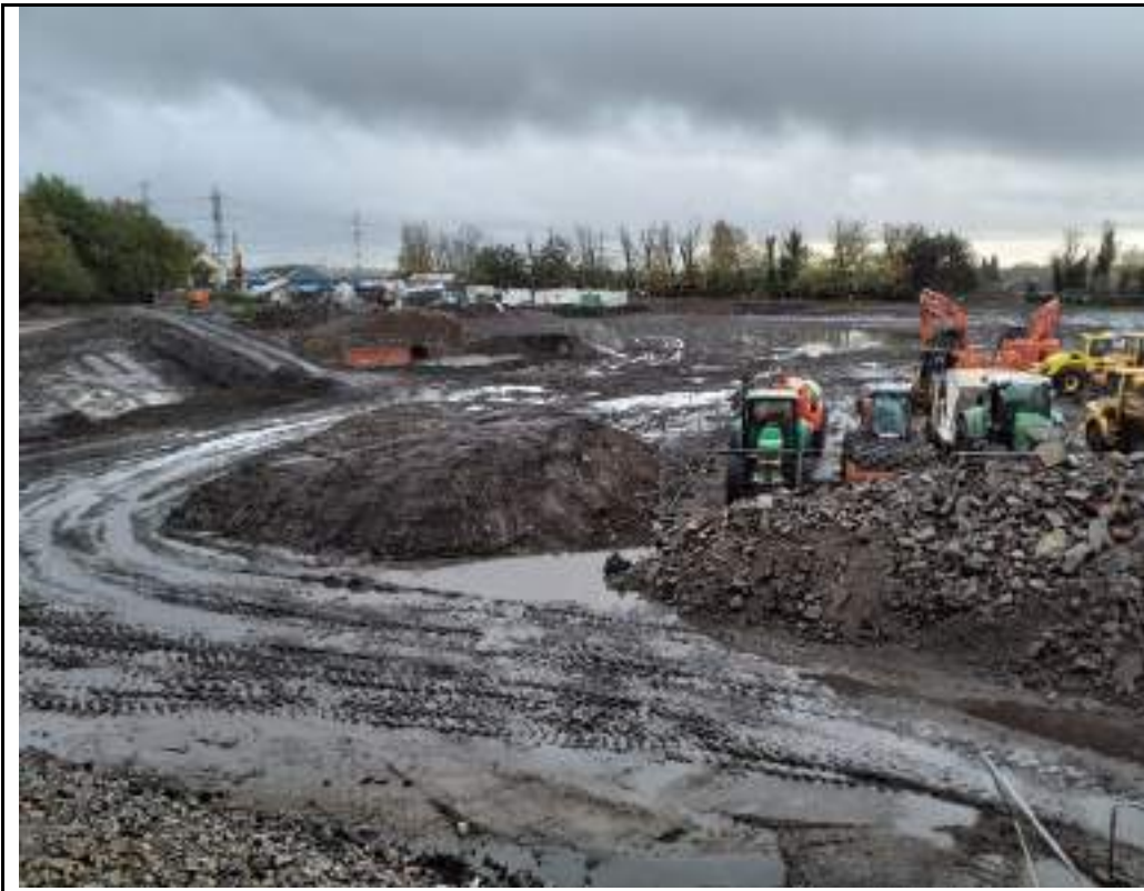
Photograph 11: Overview of the site. Looking towards the south.
