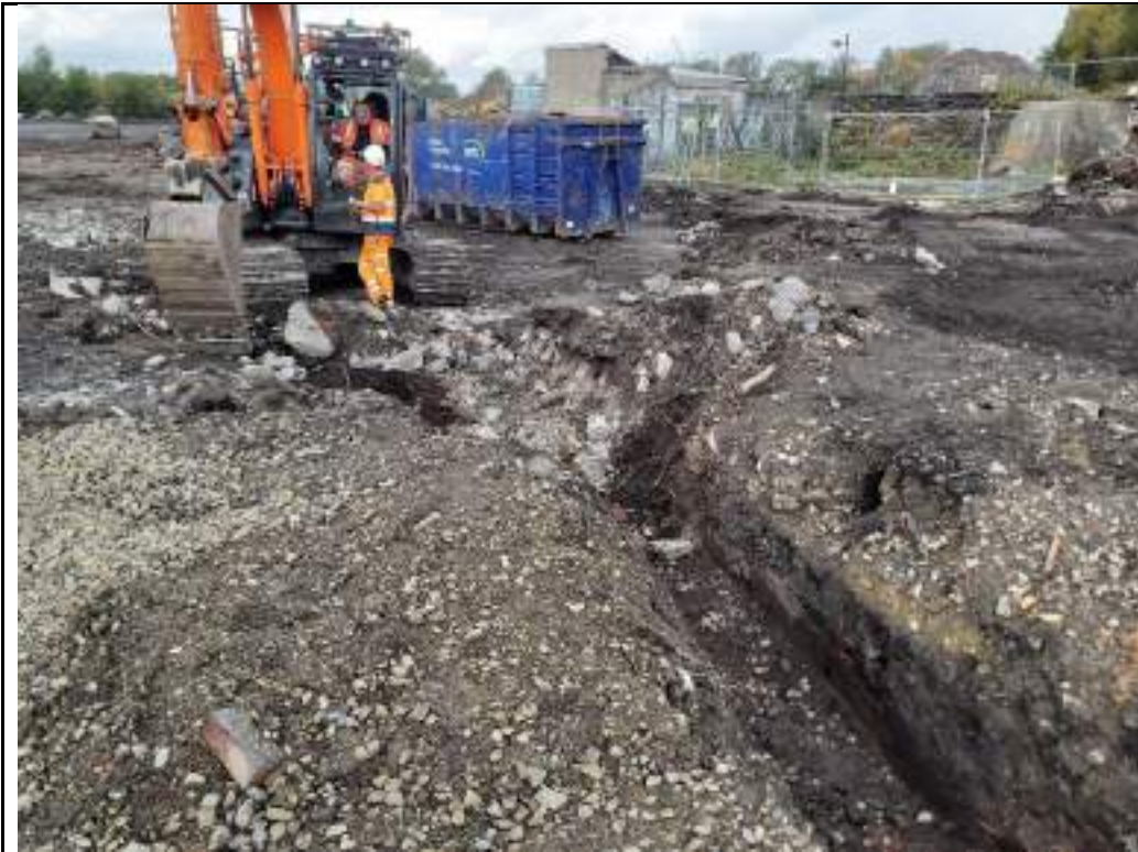
Photograph 147: Excavation for electricity cable in southeastern part of the site.
