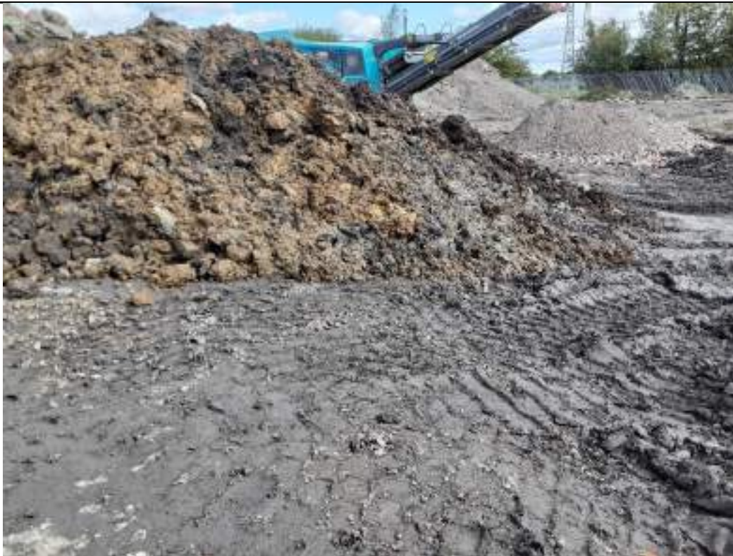
Photograph 24: Stockpiling potentially TPH contaminated material in northeastern part of the site.
