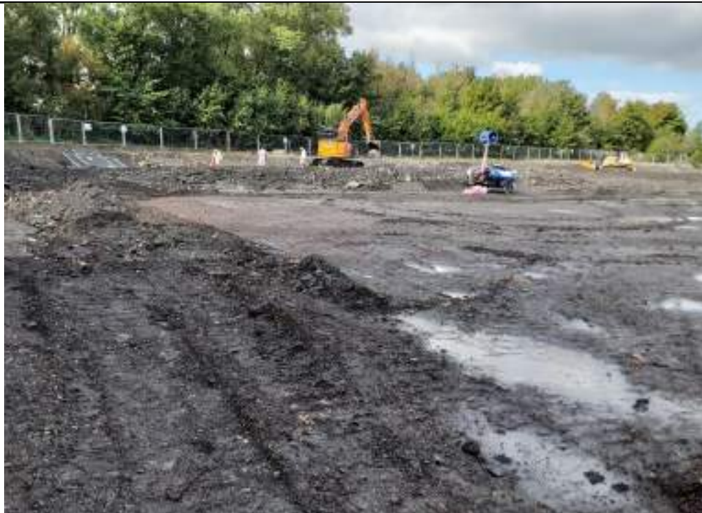
Photograph 20: Handpicking of asbestos from asbestos contaminated stockpile in southwestern part of the site.
