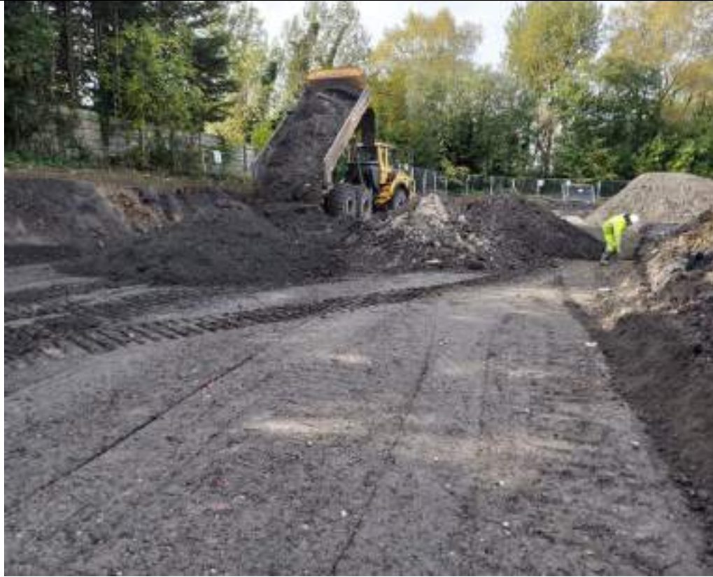
Photograph 17: Backfilling southwestern part of the site using materials from eastern excavation.
