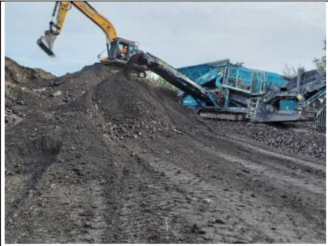
Photograph 9: Screener in northeastern part of the site processing material.
