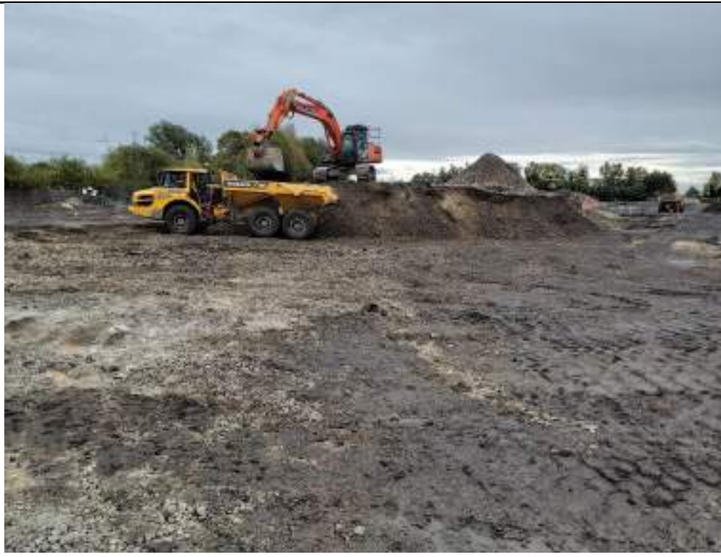
Photograph 6: Transferring granular material from northeastern stockpile to stockpile in northwestern part of the site and backfill southwest of the site.
