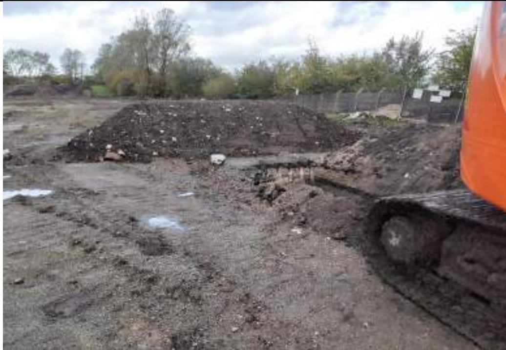
Photograph 24: Trial pit in location of organic Made Ground deposit in northeastern boundary of the site.
