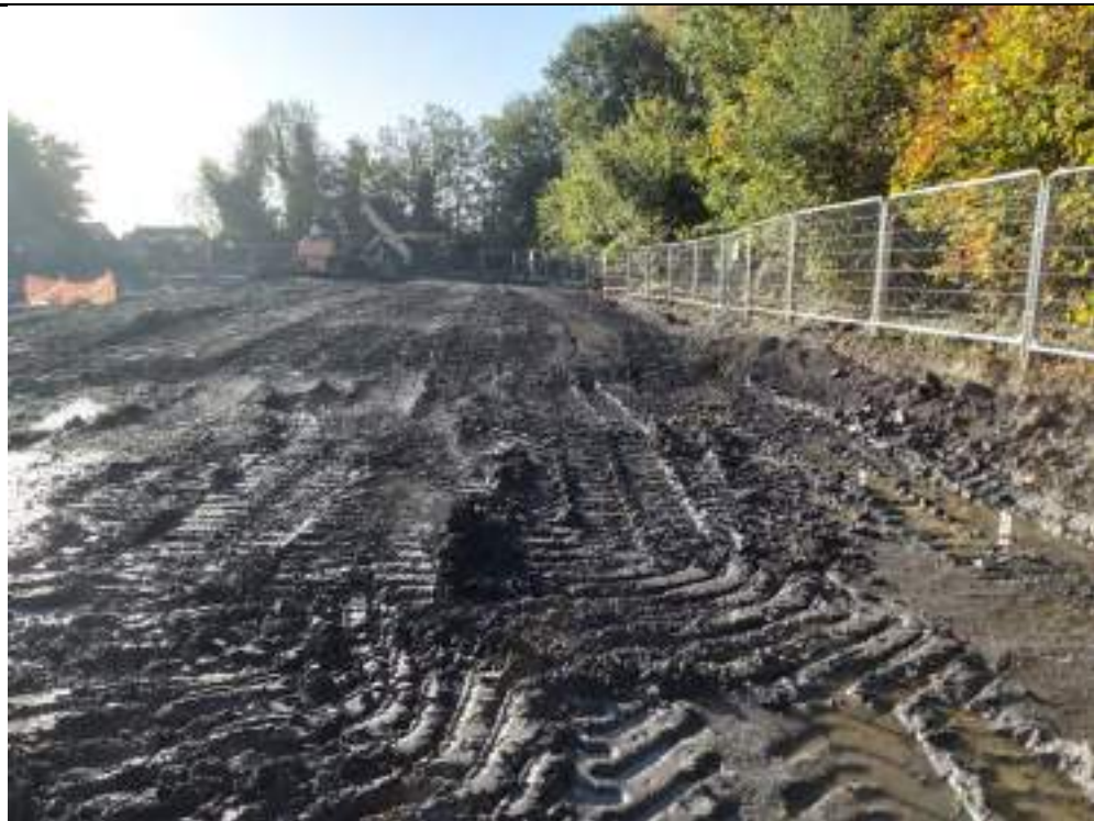
Photograph 6: Backfilling southwestern part of the site using material from eastern excavation
