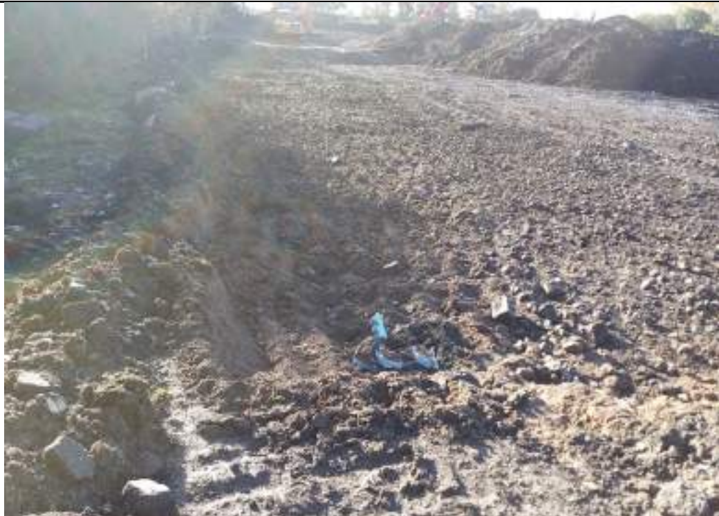
Photograph 18: northeastern boundary of the site. Looking towards the south.
