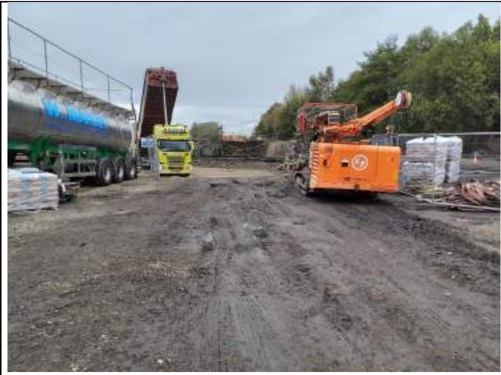
Photograph 3: Shaft grouting platform preparation and grouting rig in eastern part of the site.
