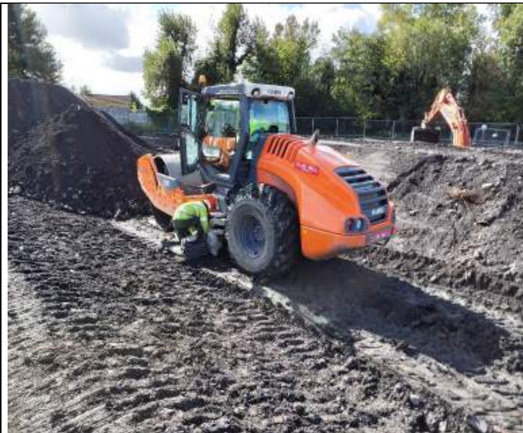
Photograph 12: Plate load testing in southwestern part of the site.
