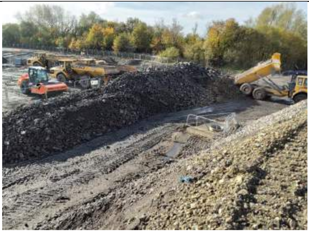
Photograph 6: Stockpiling oversized materials of screener in northwestern stockpile.
