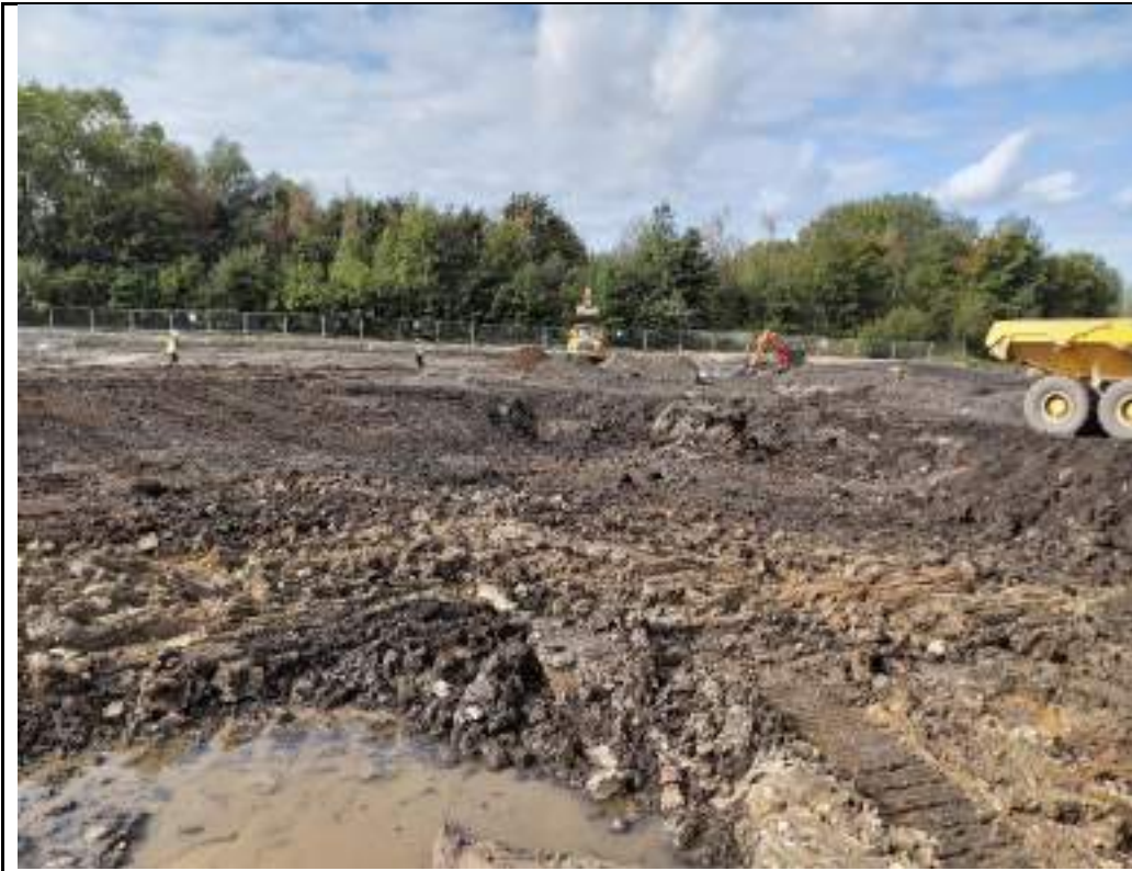
Photograph 27: Loading unsuitable fill from western part of the site to stockpile in northeastern stockpile.
