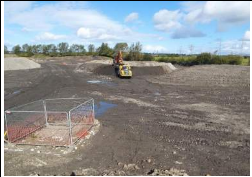
Photograph 9: Transferring material from northeastern stockpile for construction of shaft grouting platform.
