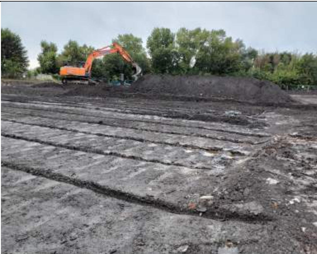
Photograph 22: Excavation of landfill Made Ground in southern part of the site.
