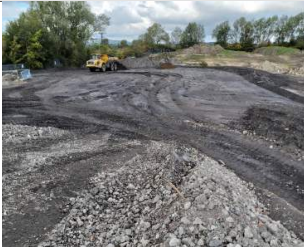
Photograph 24: Stockpiling excavated material from southeastern part of the site in northwest of the site.
