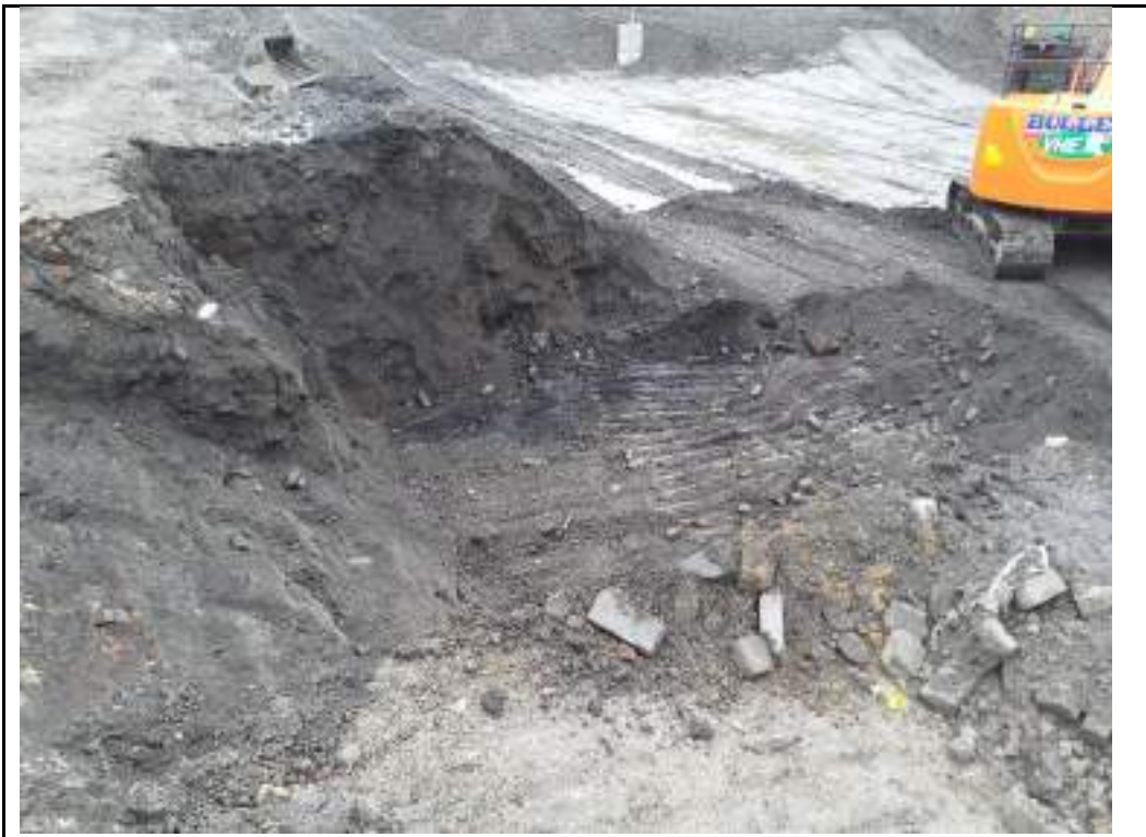
Photograph 10: Excavation of landfill Made Ground to find abstraction well in western part of the site.
