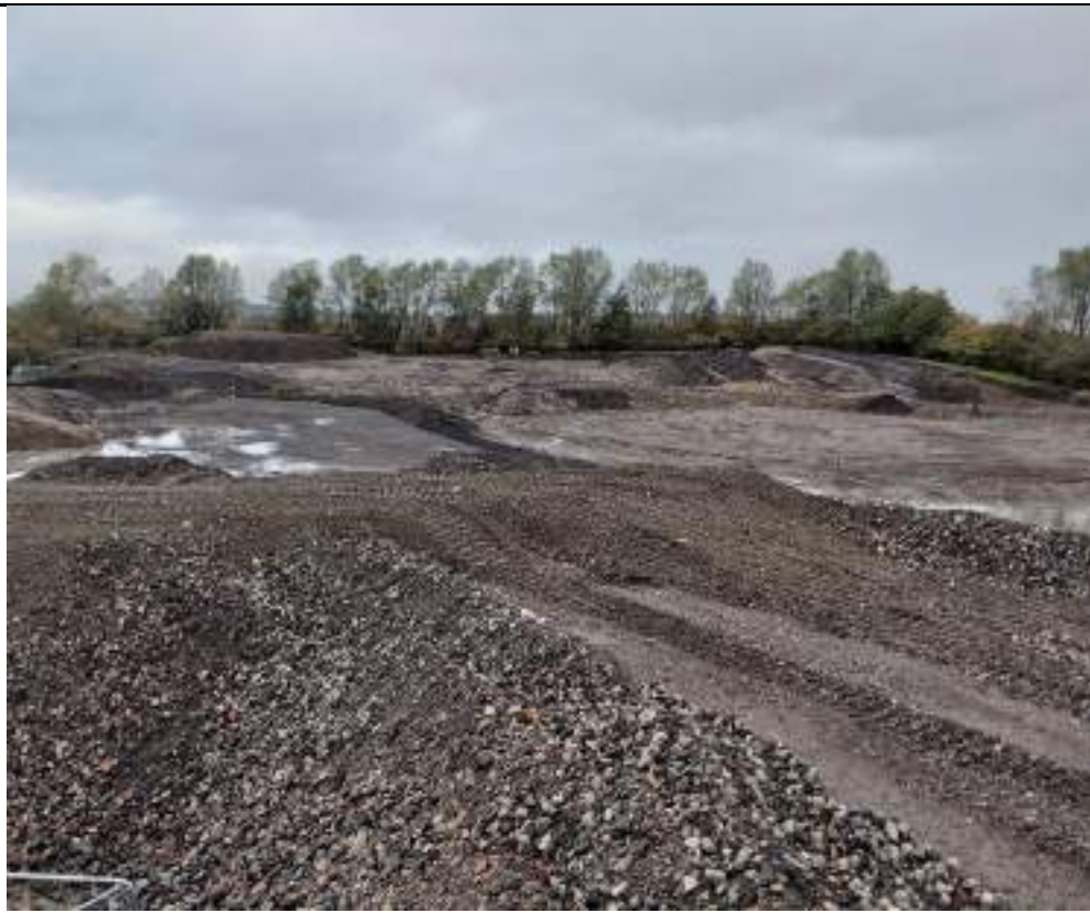
Photograph 8: Overview of northern stockpiles (Topsoil and material from soft spots)
