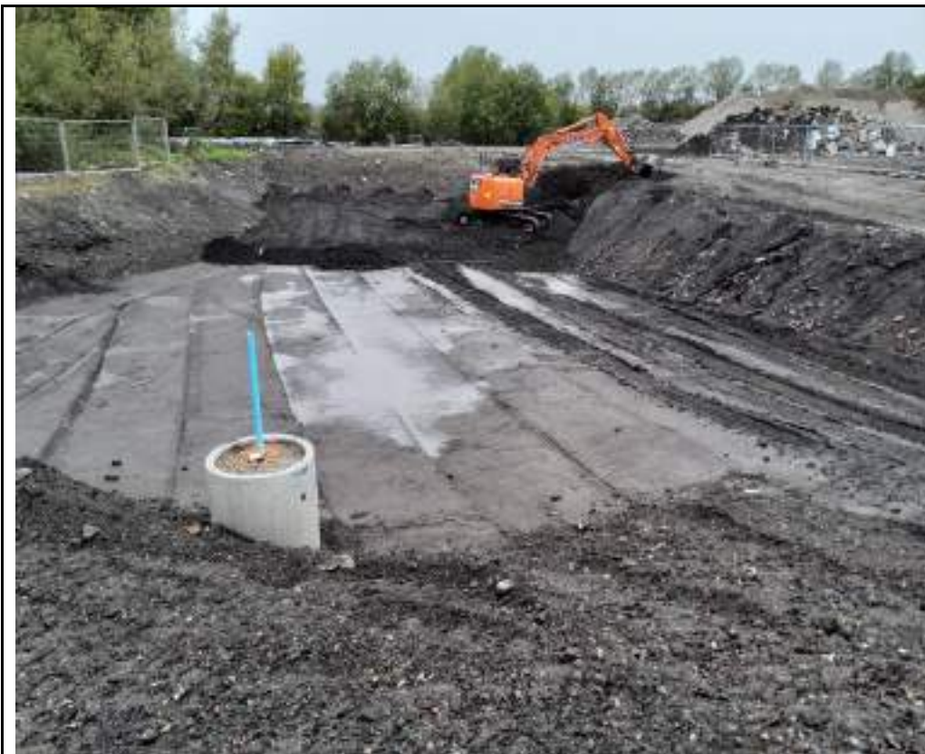
Photograph 12: Backfilling western part of the site using material from excavation in the west.
