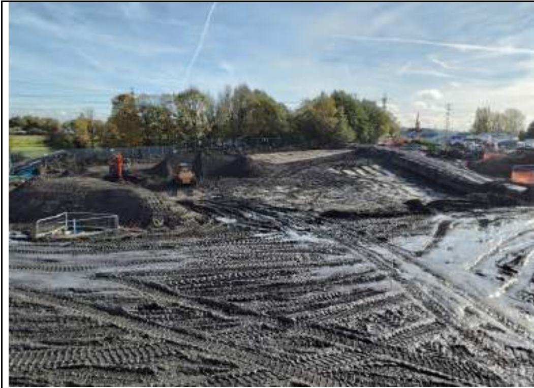
Photograph 17: Placed fill and stockpile of processed materials in eastern part of the site.
