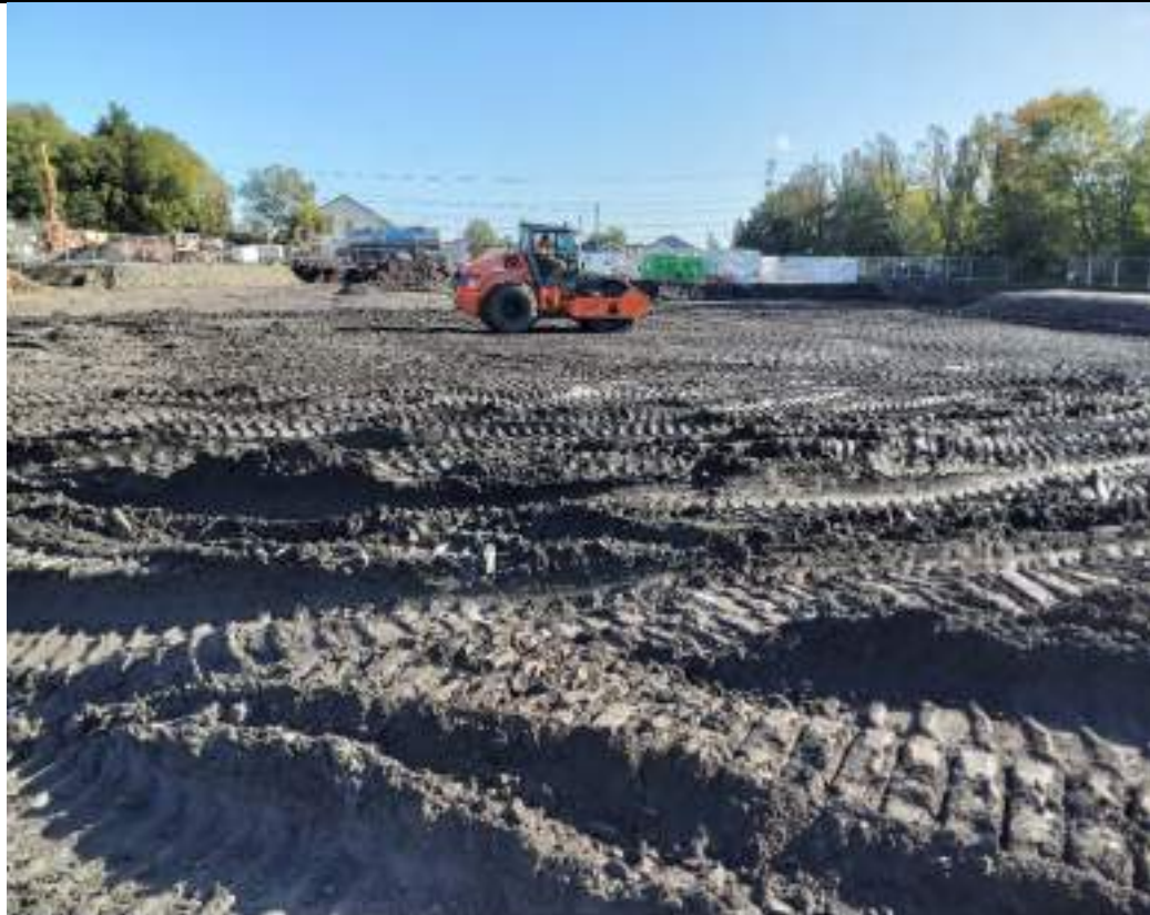
Photograph 23: Proof rolling over fill materials using sheepfoot roller in southern part of the site.
