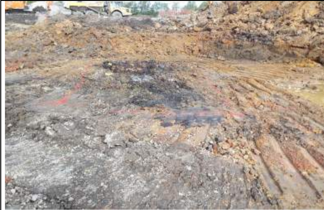
Photograph 21: Potentially TPH contaminated area in southeastern part of the site
