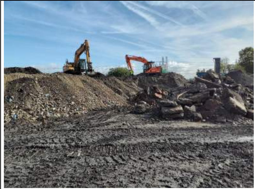
Photograph 113: Surveying of stockpiles in northeastern part of the site.
