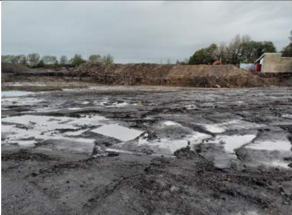
Photograph 18: Stockpile of excavated Glacial Till and standing water in southeast of the site.
