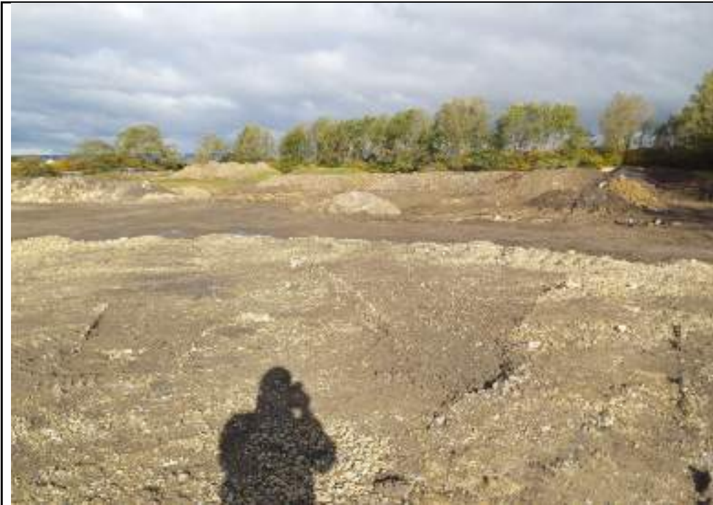
Photograph 15: Stockpile of Topsoil and materials from soft spots excavations in northern part of the site.
