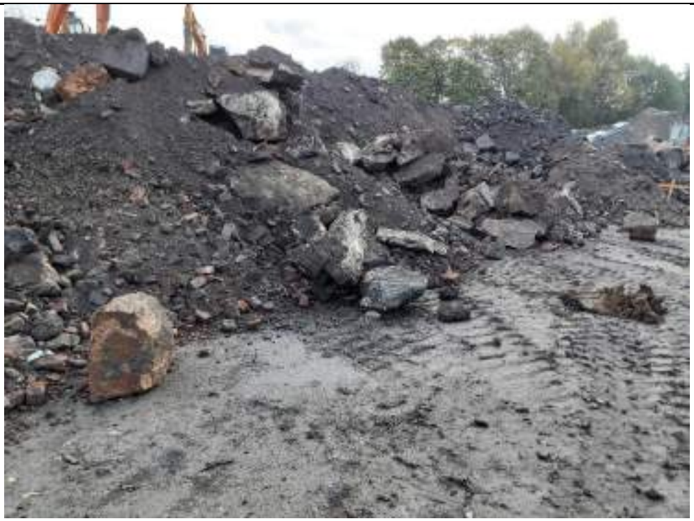
Photograph 6: Oversize and deleterious materials in northeastern stockpile.
