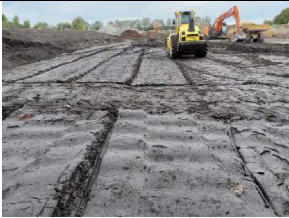
Photograph 5: Compaction of formation by polygonal roller in southern part of the site.
