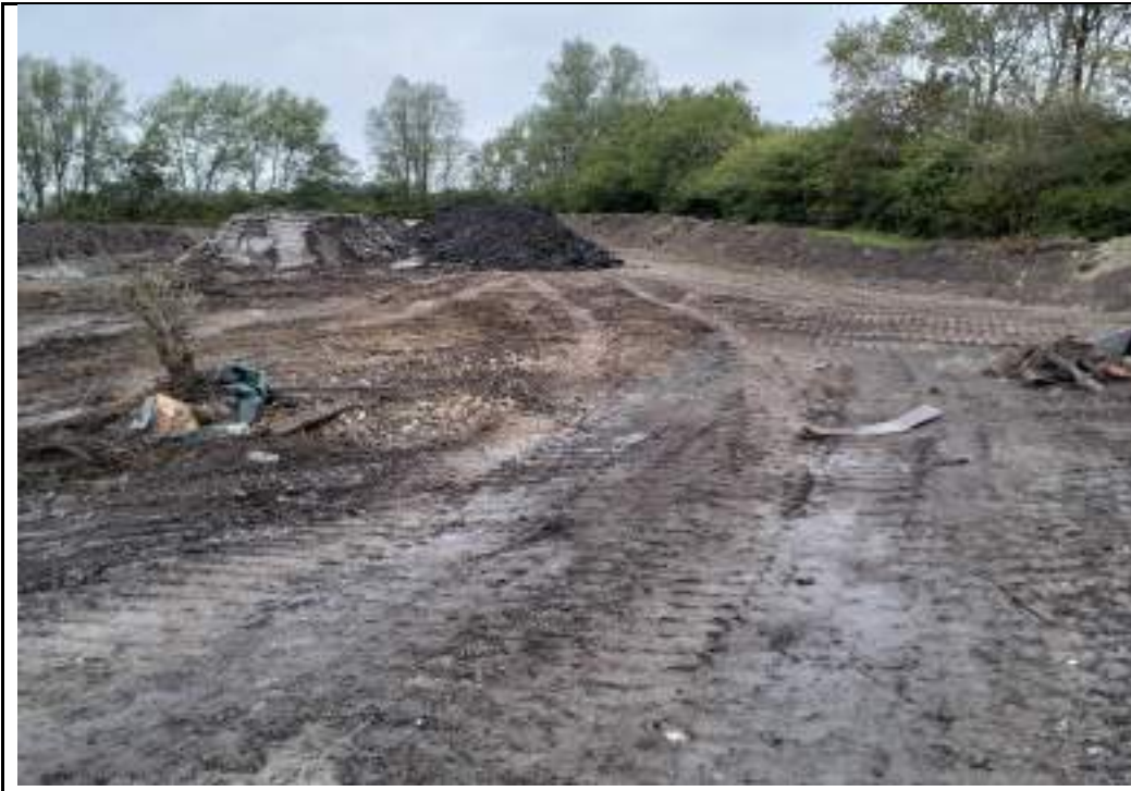
Photograph 15: Stockpile of excavated material from soft spot excavation in northeastern part of the site.
