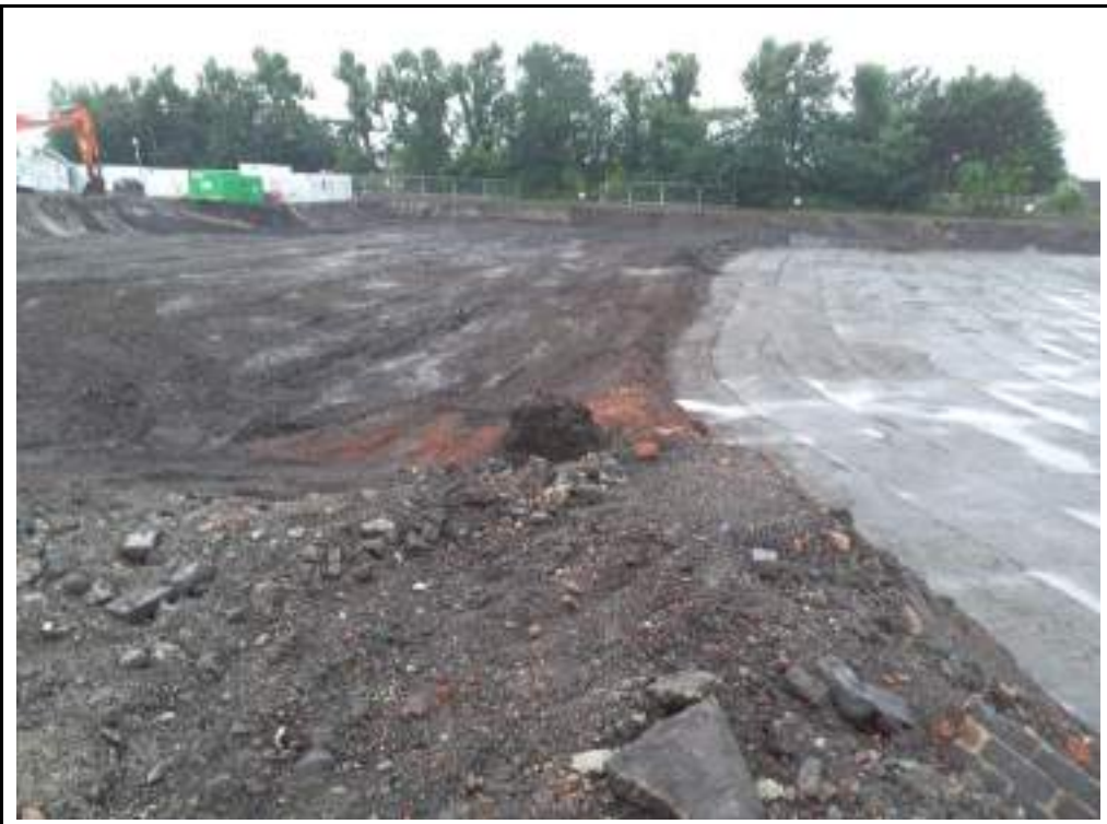
Photograph 4: Boundary between 1.5m cut and 3m cut areas in southern part of the site.
