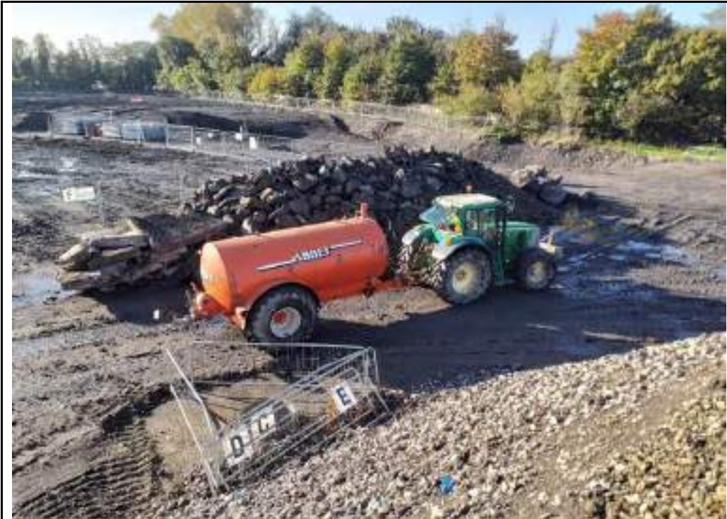
Photograph 11: Oversize and concrete stockpile in northwestern part of the site.
