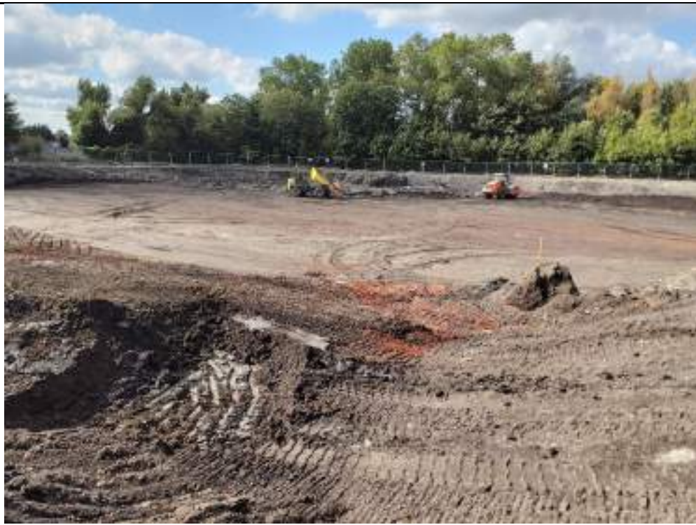
Photograph 6: Proof rolling of fill material in western part of the site.
