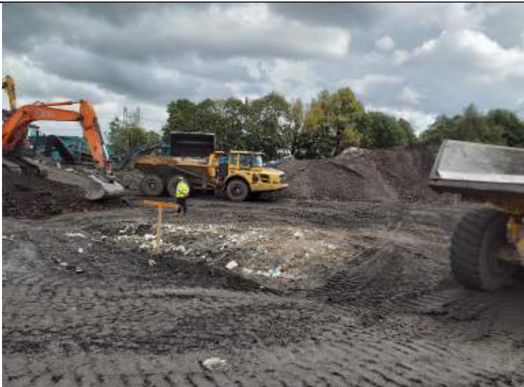
Photograph 20: Loading of fine material (dark ashy) from screener to backfill northwestern part of the site.
