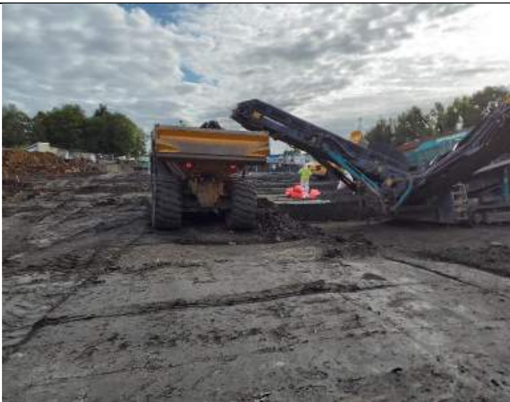
Photograph 158: Separation of oversize material (bricks) from asbestos contaminated stockpile in southwestern part of the site.
