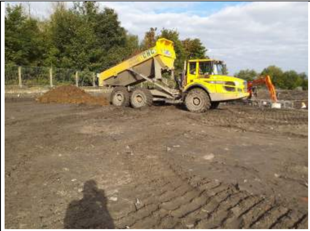
Photograph 3: Backfilling western part of the site with excavated material from southeast of the site.
