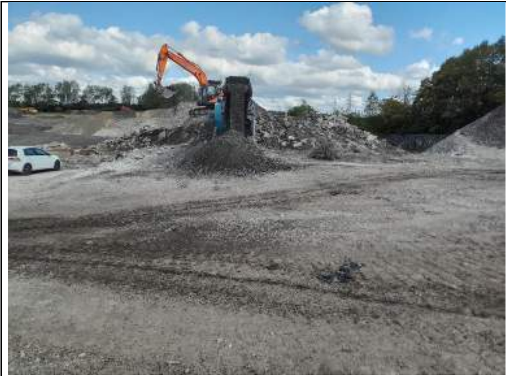
Photograph 91: Crushing concrete and asphalt in eastern part of the site.
