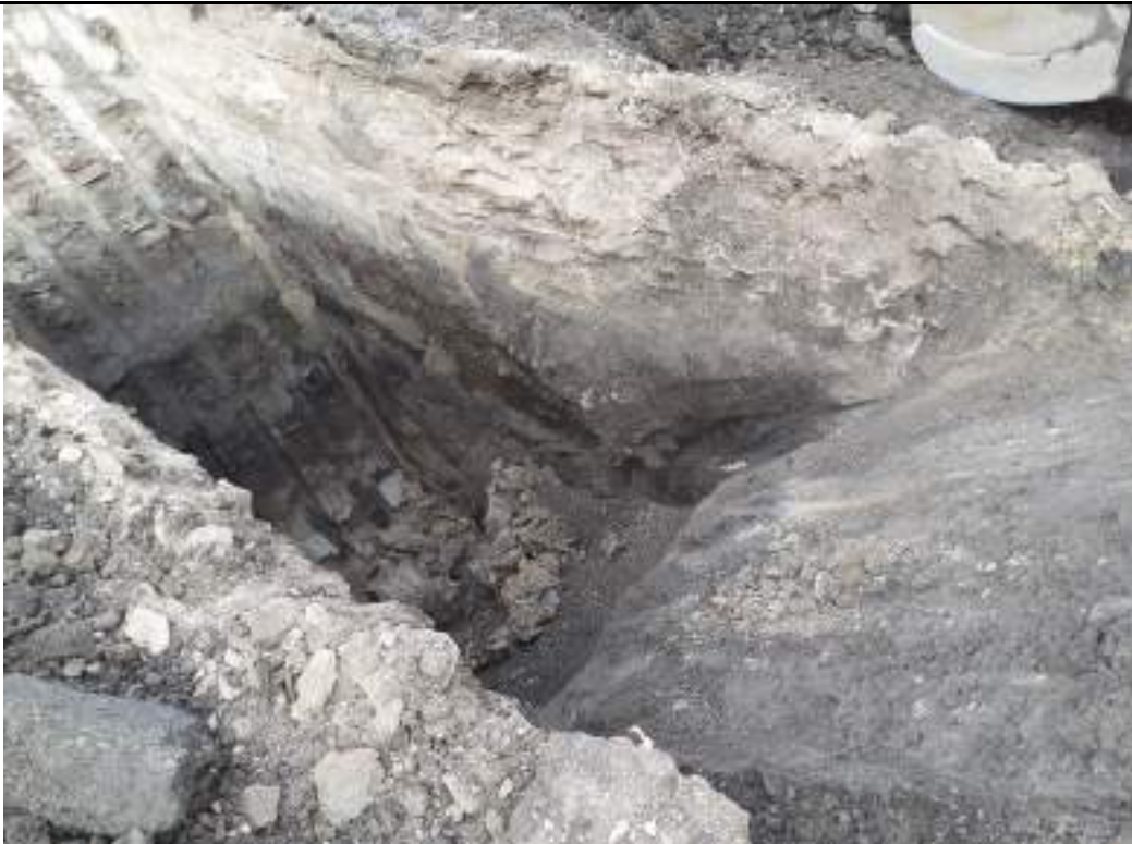
Photograph 20: Trial pit in eastern part of the site.
