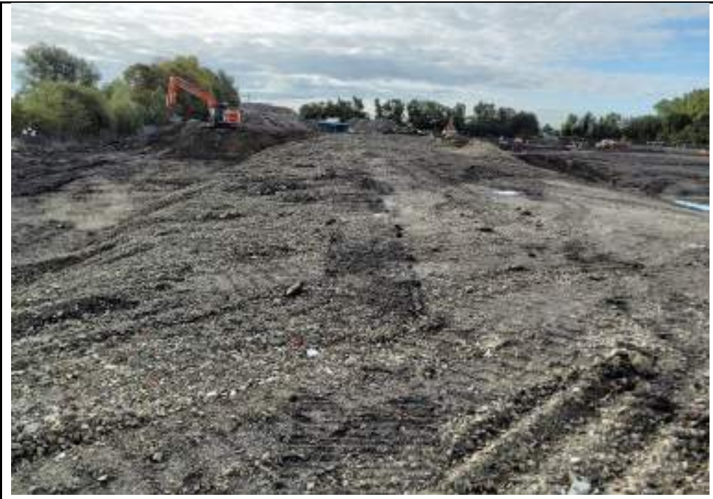
Photograph 1: Overview of the site. Looking towards the south.
