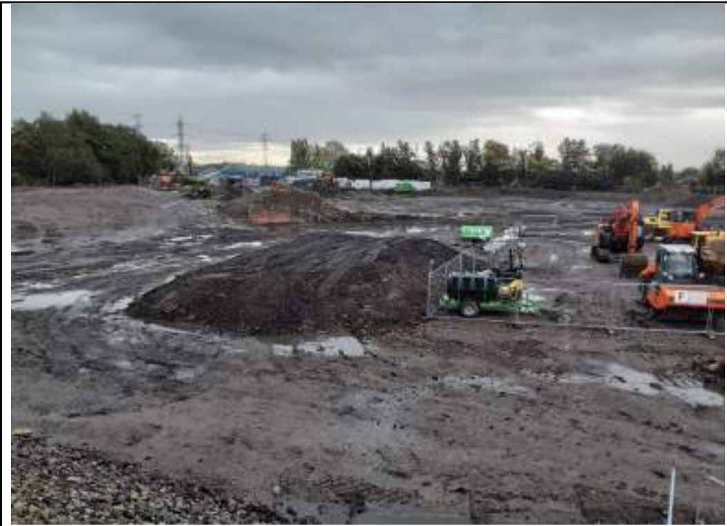
Photograph 1: Overview of the site. Looking towards the south.
