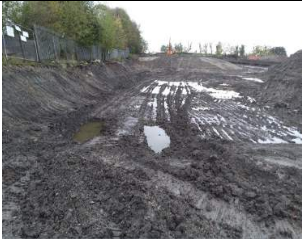
Photograph 7: Northeastern boundary of the site. Looking towards the south.
