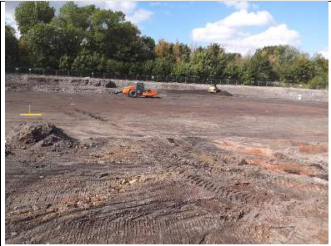
Photograph 9: Proof rolling and backfilling in western part of the site
