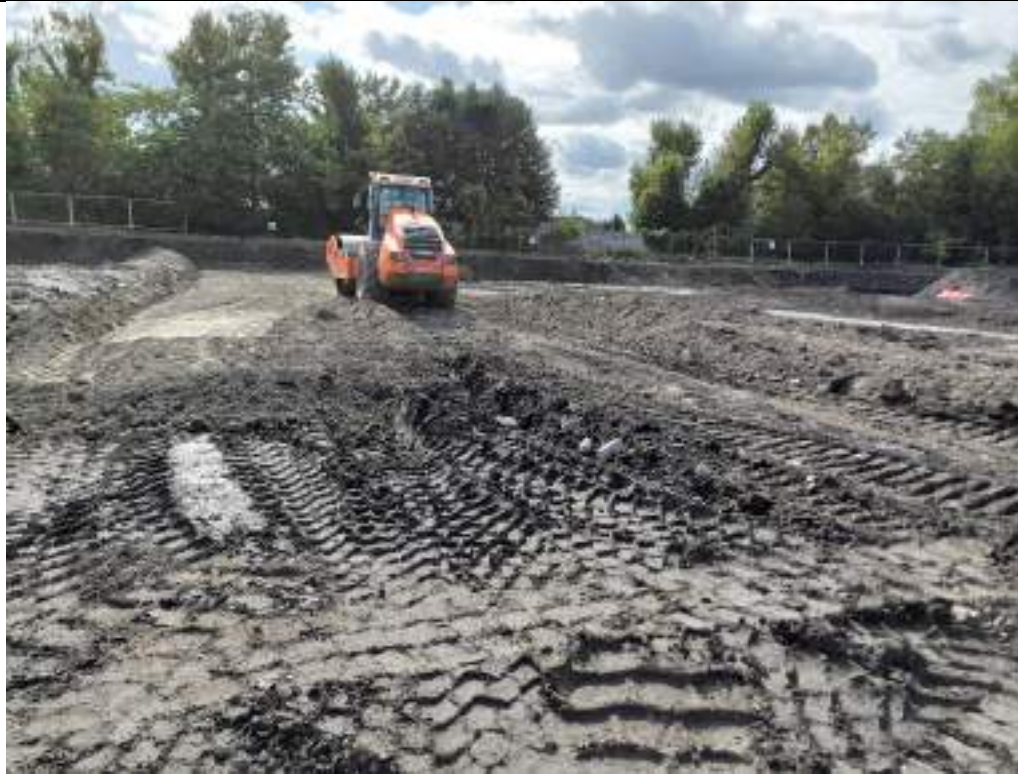
Photograph 31: Proof rolling in southern part of the site.
