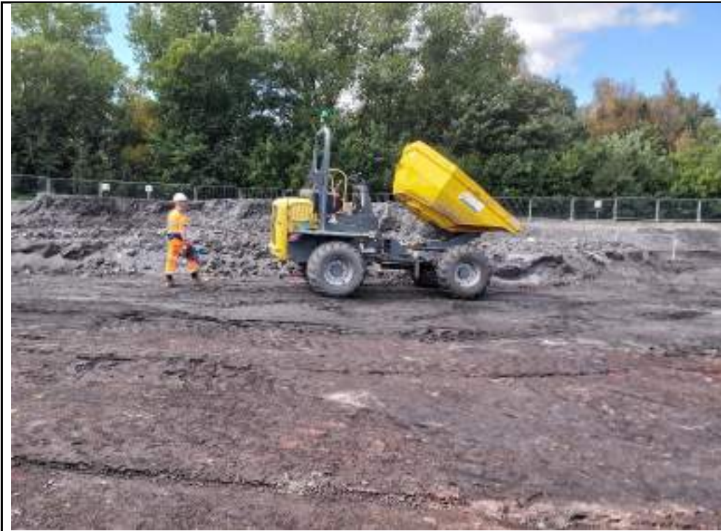
Photograph 125: Hand picking of deleterious material in southwest of the site.
