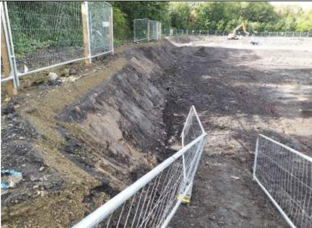
Photograph 22: Southern boundary of the site. Looking towards the west.
