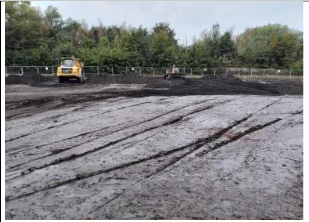
Photograph 11: Backfilling of western part of the site using material from excavation in southwestern part of the site.
