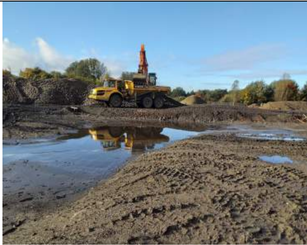
Photograph 8: Transferring crushed material from northwestern stockpile to backfill southeastern part of the site.
