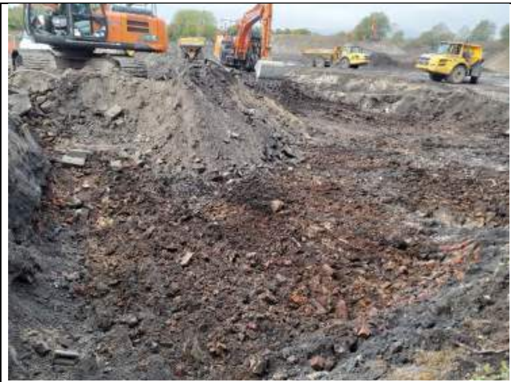
Photograph 4: Excavation of landfill Made Ground in eastern part of the site.
