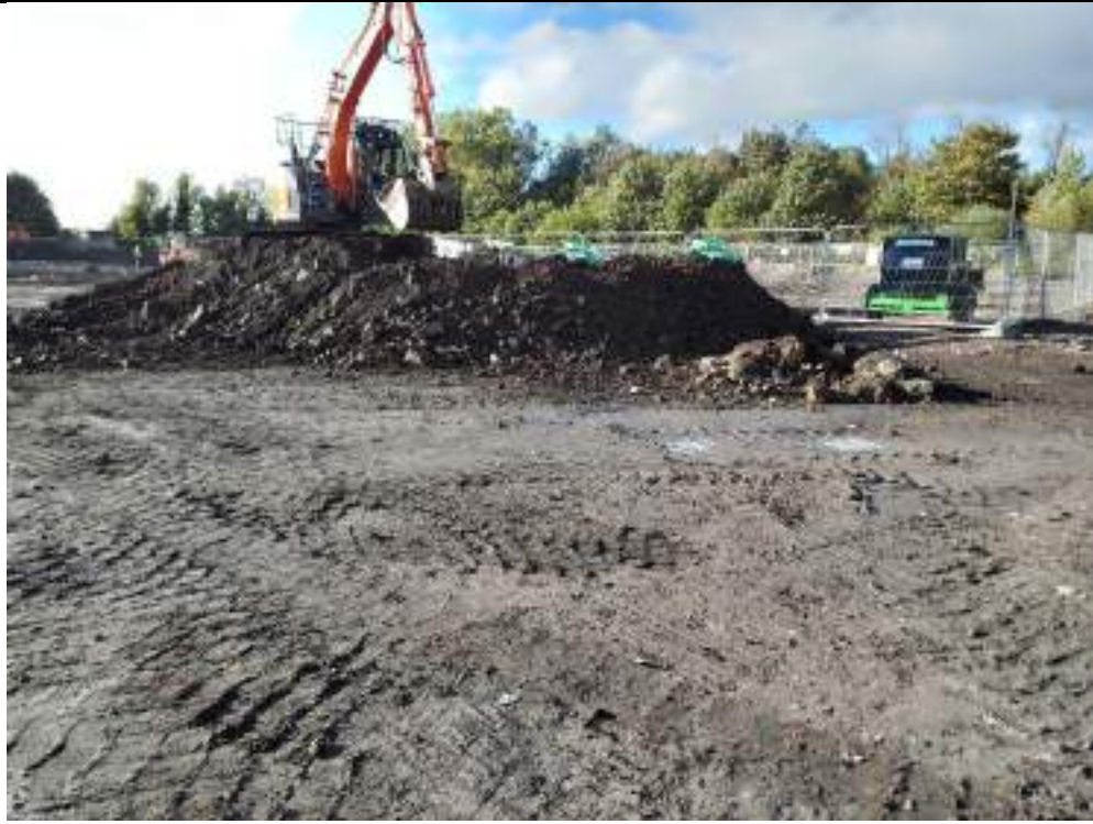
Photograph 7: Removing oversize from excavated material from southeastern part of the site using riddle bucket excavator in northwestern stockpile.
