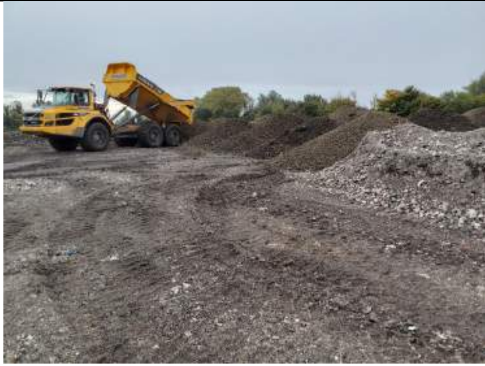
Photograph 7: Stockpiling granular material in northwestern part of the site over crushed material stockpile in northwestern part of the site.
