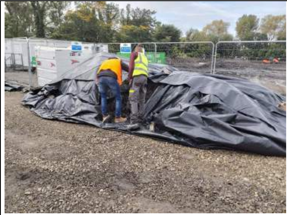
Photograph 3: Sample collection from potentially asbestos contaminated material in car park area.
