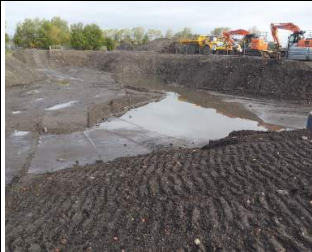
Photograph 17: Standing water in excavation for abstraction well in western part of the site.
