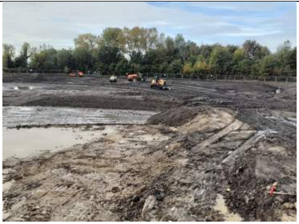
Photograph 6: Temporary Road construction in southern part of the site.
