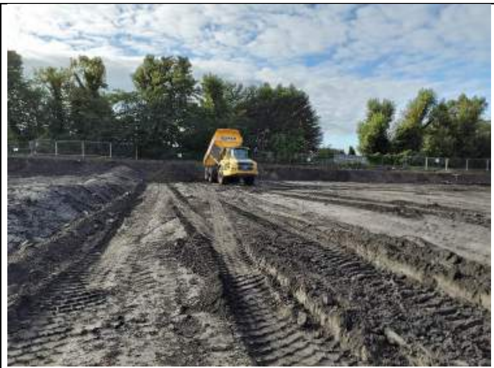
Photograph 4: Backfilling southern part of the site with material from northeastern stockpile.
