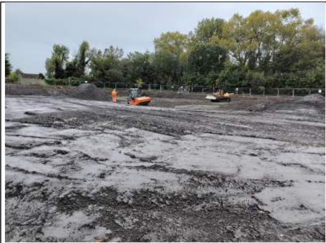
Photograph 14: Proof rolling of granular fill material in southwestern part of the site.
