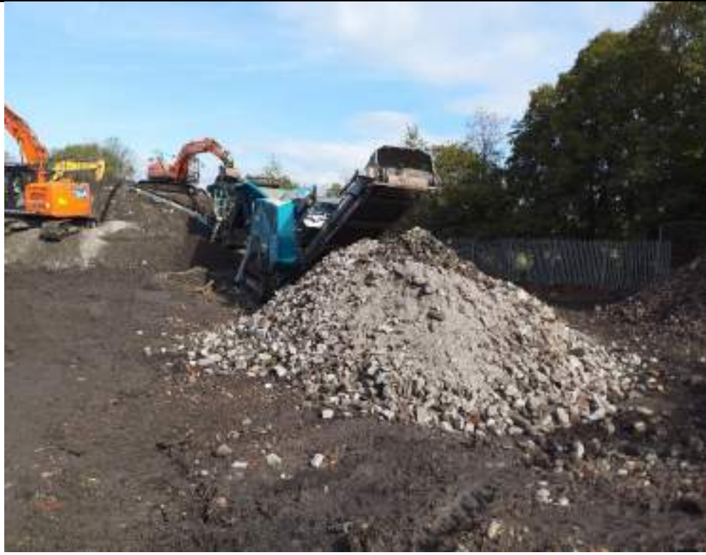
Photograph 7: Crushing oversize material from screener in northeast of the site.
