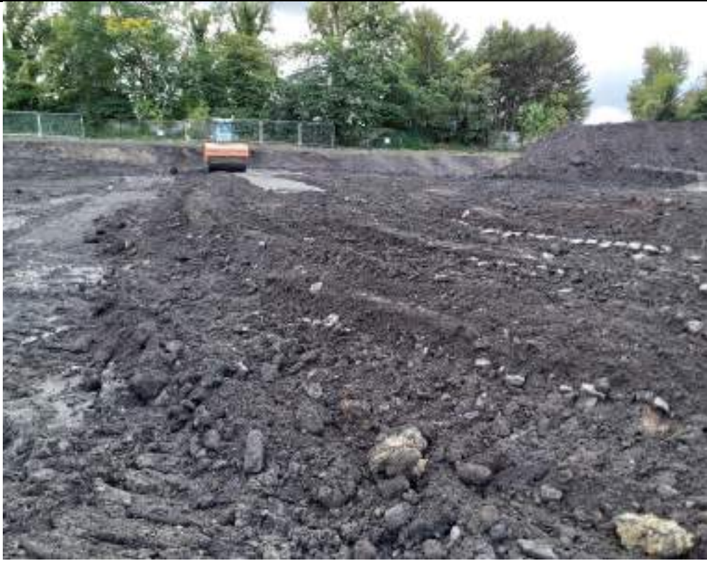
Photograph 19: Proof rolling of fill material in southern part of the site.
