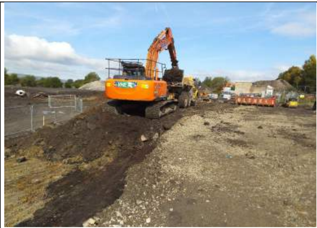
Photograph 2: Excavation of landfill Made Ground in southern part of the site.
