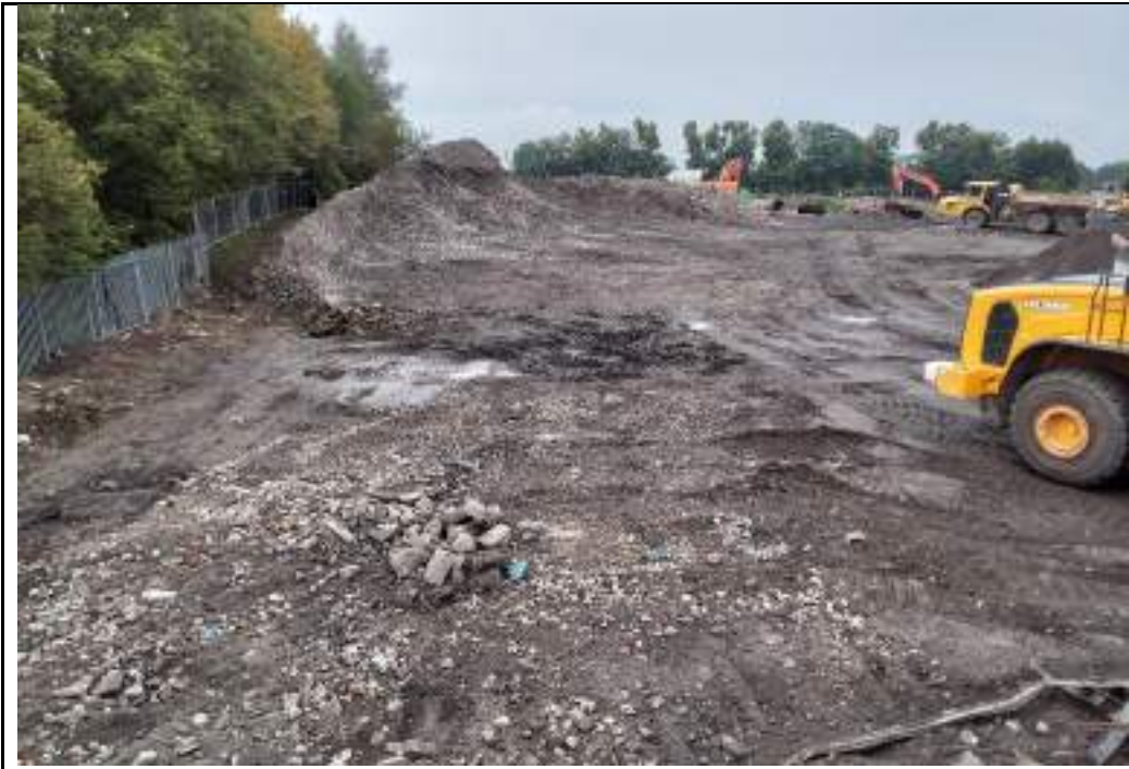
Photograph 147: Stockpile of crushed material in eastern part of the site.
