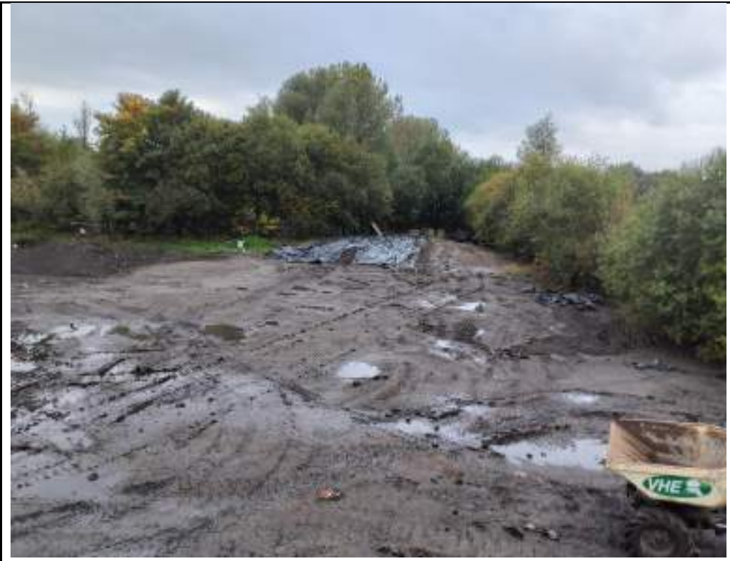
Photograph 9: Stockpile of potentially TPH contaminated material in western boundary of the site.
