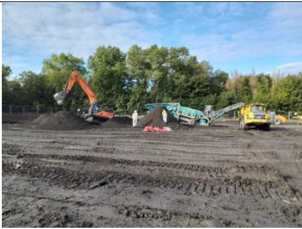
Photograph 6: Screening of asbestos stockpile and hand picking of asbestos in southwestern part of the site.
