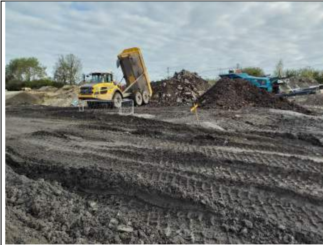
Photograph 125: Stockpiling concrete and oversize material in northeastern part of the site.
