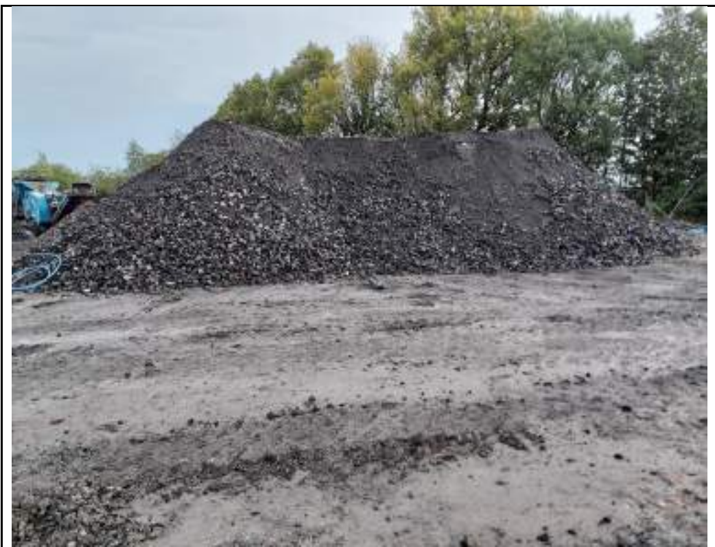
Photograph 110: Stockpile of crushed material from oversize material of the screener in eastern part of the site.
