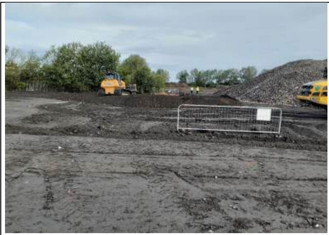
Photograph 14: Backfilling northwest of the site using undersize material from the screener.
