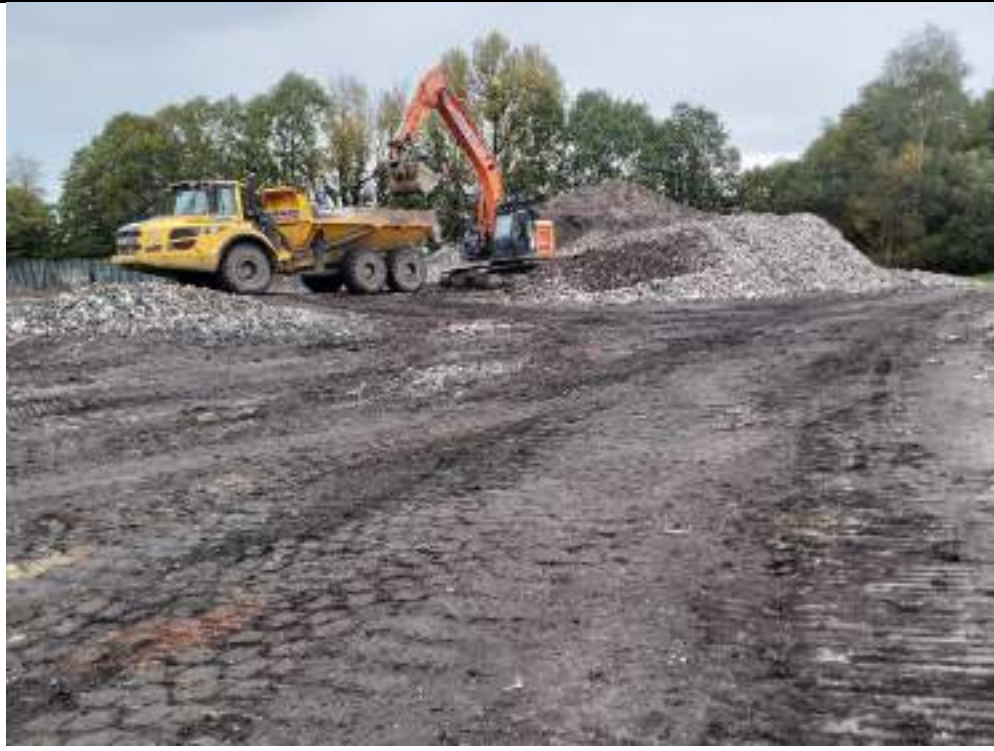
Photograph 5: Transferring crushed material from eastern stockpile to stockpile in northwestern part of the site.
