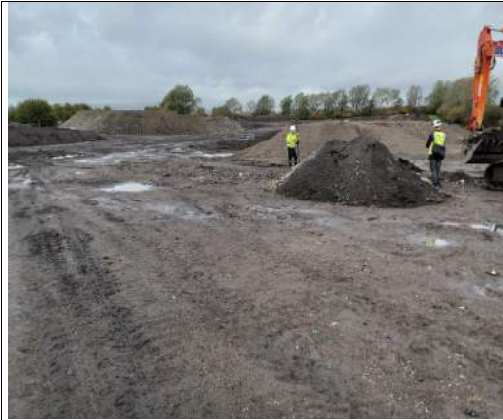
Photograph 19: Excavation of trial pit in eastern part of the site.
