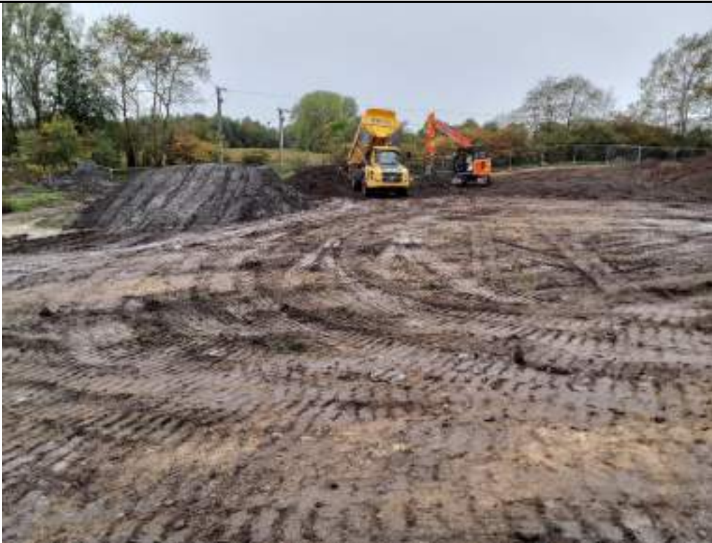
Photograph 18: Stockpiling soft spot material from northern stockpile in northwestern part of the site.
