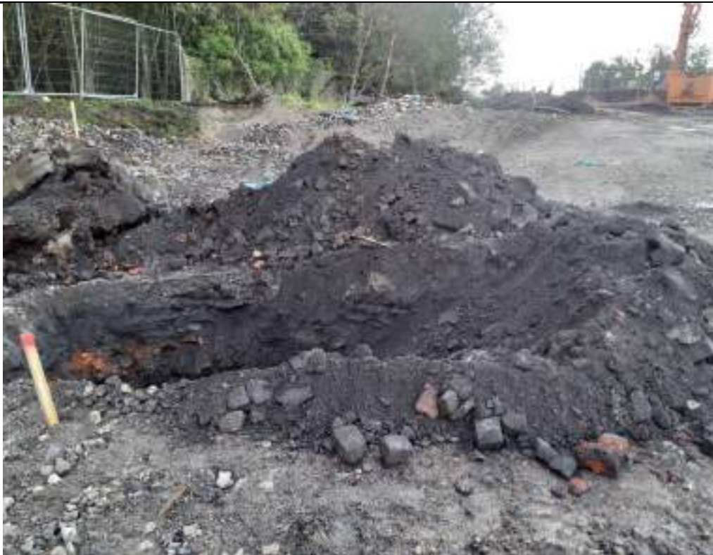
Photograph 24: Trial pit in eastern boundary of the site.
