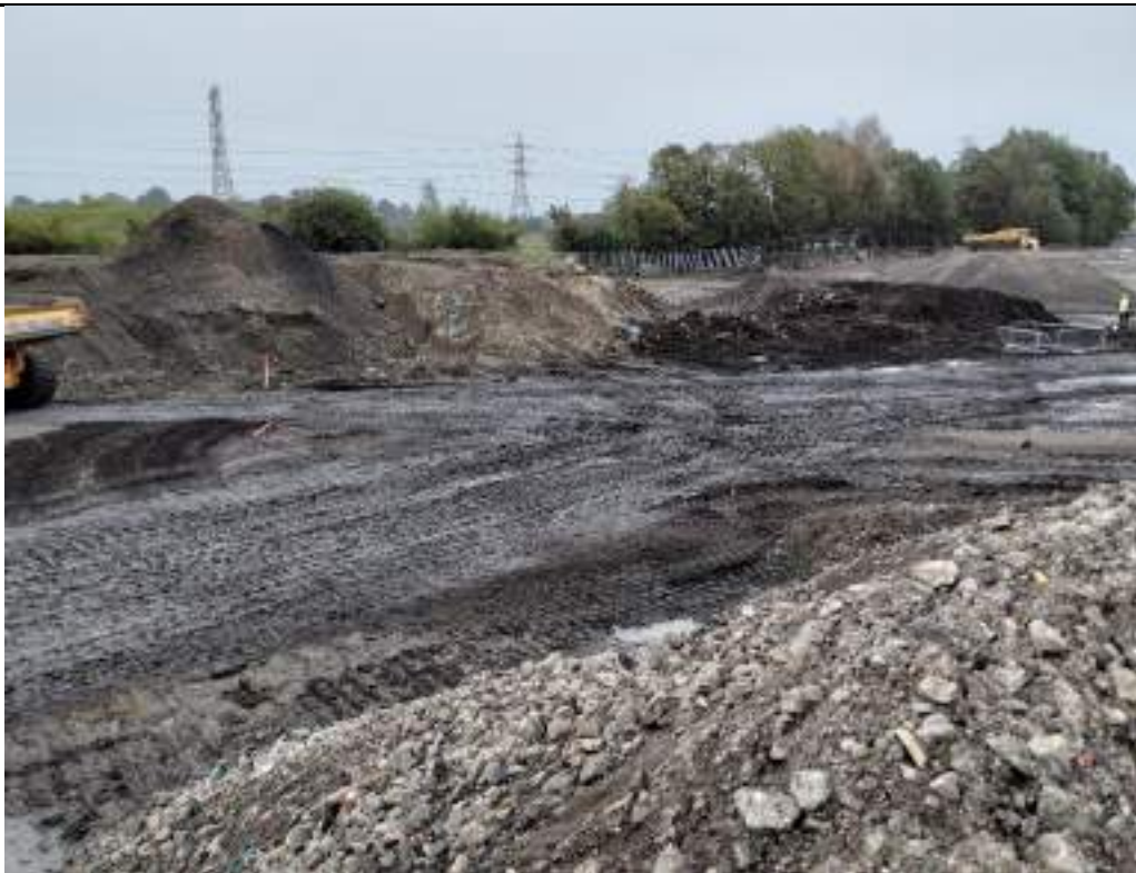
Photograph 16: Stockpiles of processed and excavated material in eastern part of the site.
