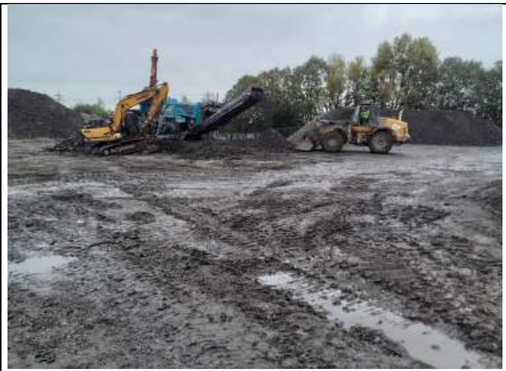
Photograph 6: Crushing concrete and asphalt in eastern part of the site.
