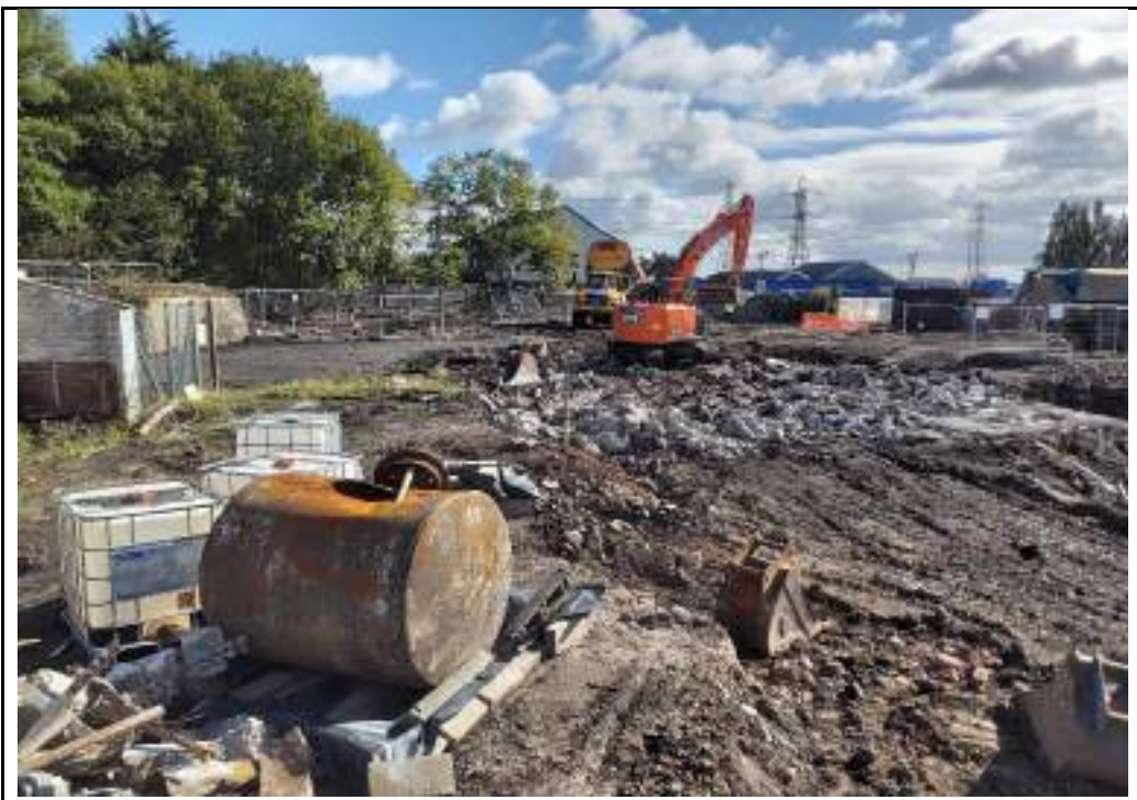
Photograph 10: Unloading material in southeastern part of the site to construct shaft grouting platform.
