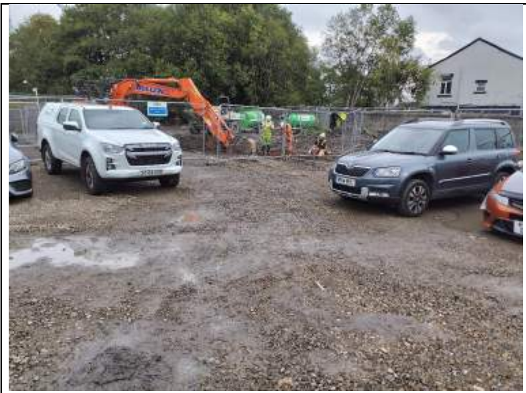
Photograph 2: Excavation for electricity cable in southeastern part of the site.
