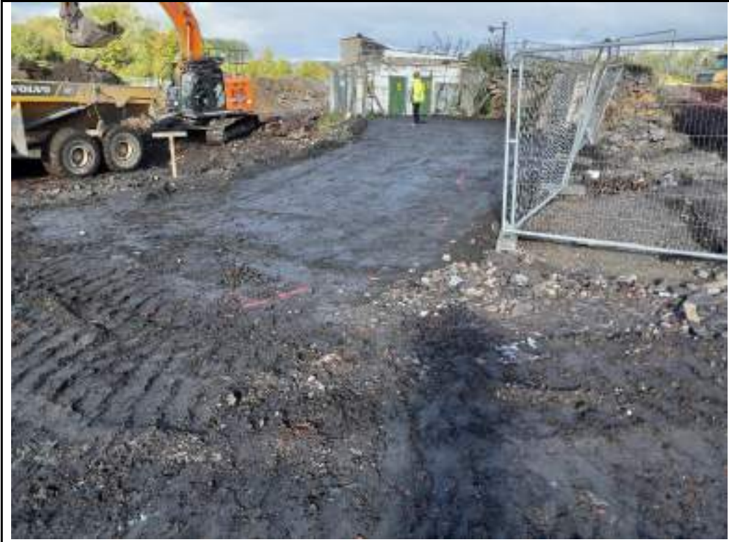
Photograph 93: Constructed platform for mine shaft no.6 grouting operation.
