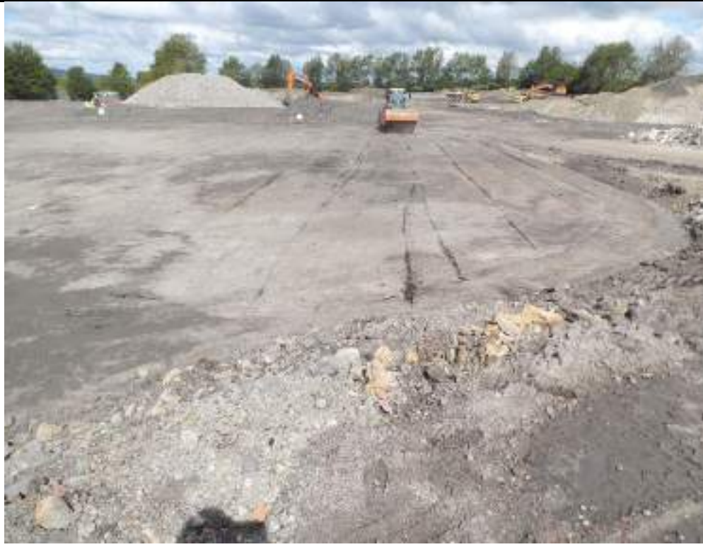
Photograph 7: Proof rolling of fill material in northern part of the culvert.
