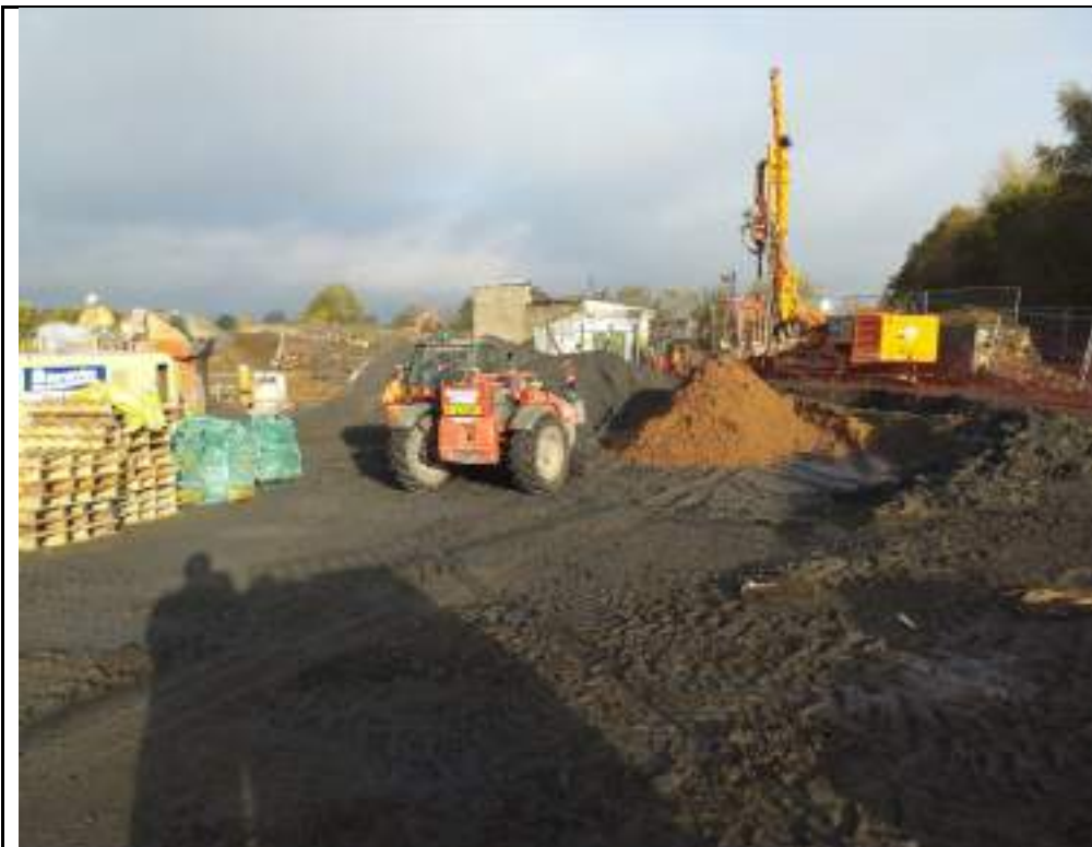
Photograph 2: Grouting shaft no.6 in eastern part of the site.
