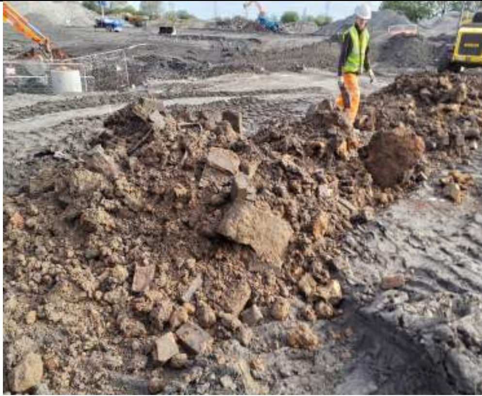
Photograph 8: Hand picking of deleterious material in southern part of the site.
