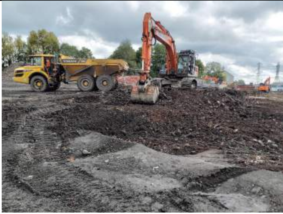
Photograph 7: Removing landfill Made Ground in southeastern part of the site.
