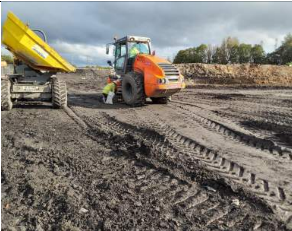
Photograph 16: Plate load testing in southern part of the site.
