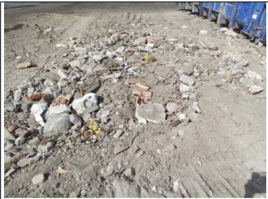
Photograph 10: Deleterious materials in central part of the site.
