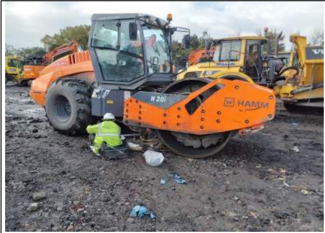
Photograph 23: Plate load testing in truck parking area in northwest of the site.
