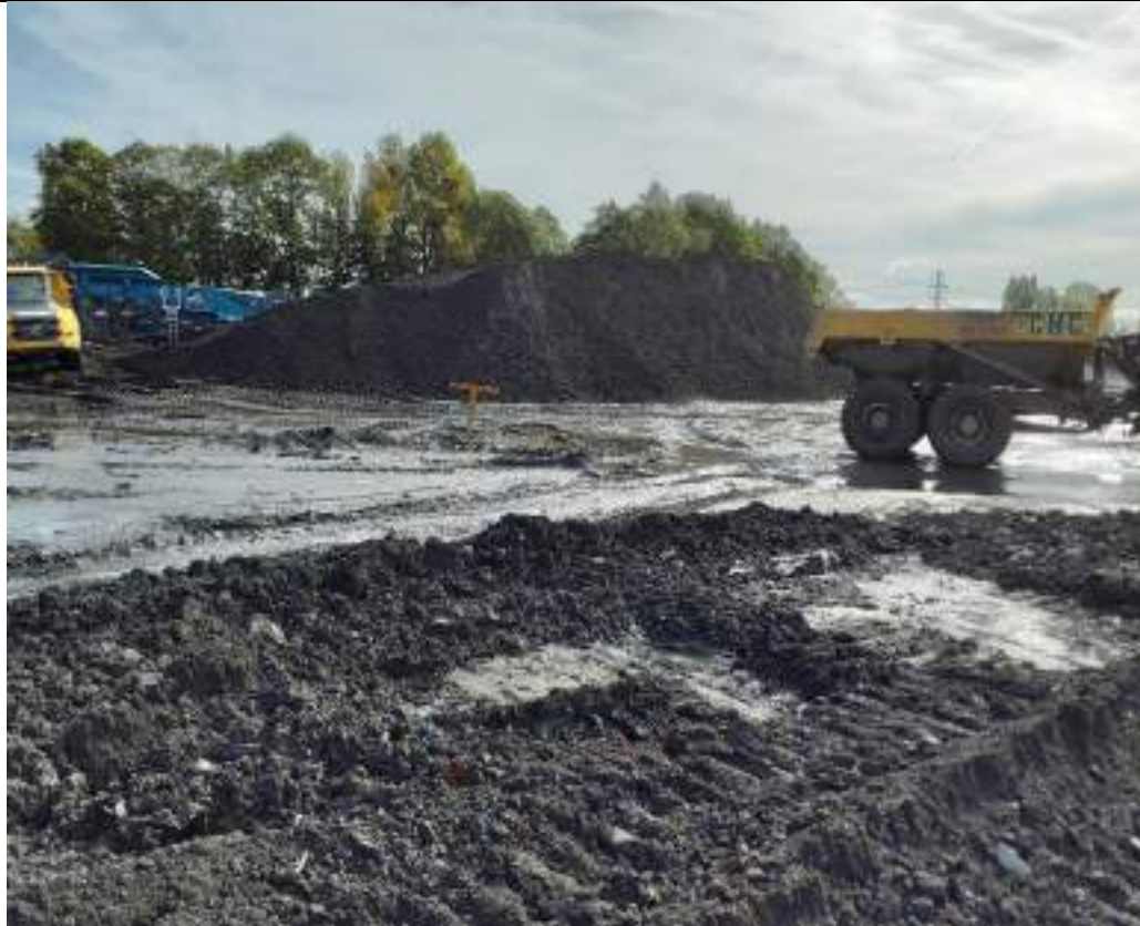
Photograph 25: Stockpile of undersize material from screener in northeast of the site.
