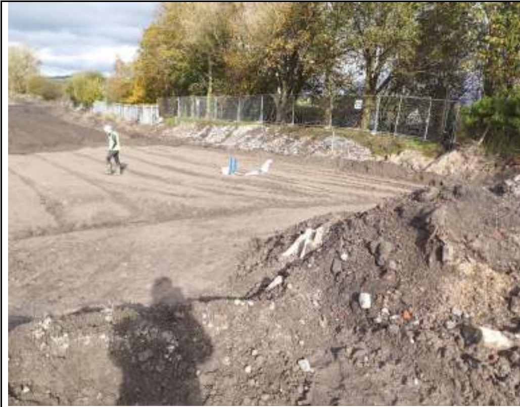
Photograph 23: Sand Replacement Testing in eastern part of the site.
