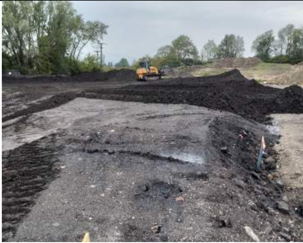
Photograph 7: Backfilling northwestern part of the site.
