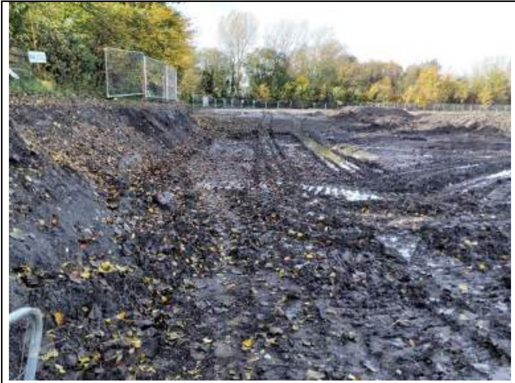
Photograph 9: Southern boundary of the site. Looking towards the west.
