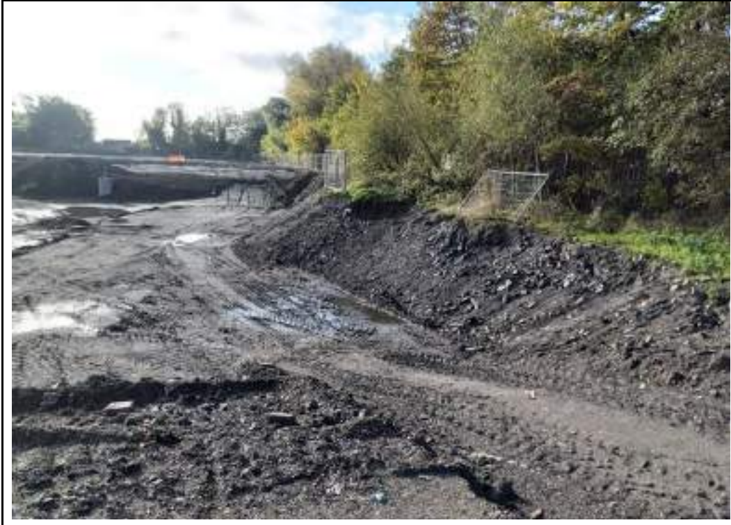
Photograph 93: Western boundary of the site. Looking towards the south.
