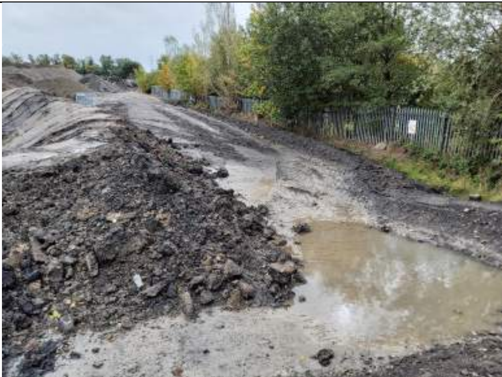
Photograph 24: Northwestern boundary of the site. Looking towards the south.
