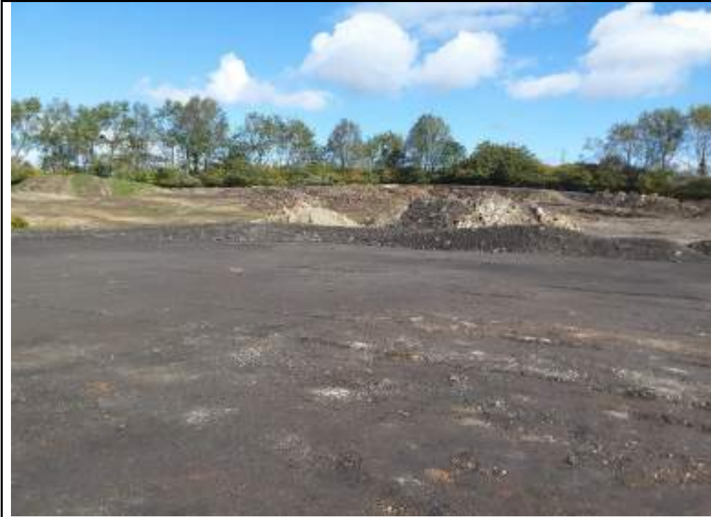
Photograph 17: Topsoil and soft spot materials stockpiles in northern part of the site.
