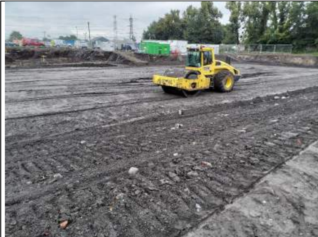
Photograph 21: Compacting formation using polygonal roller in southern part of the site.
