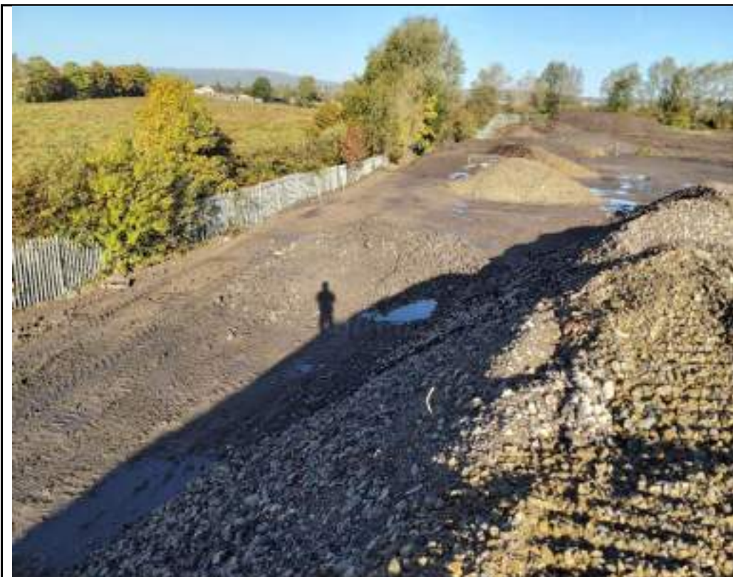
Photograph 12: Stockpiles of bricks, granular and soft spot materials in northwestern part of the site.
