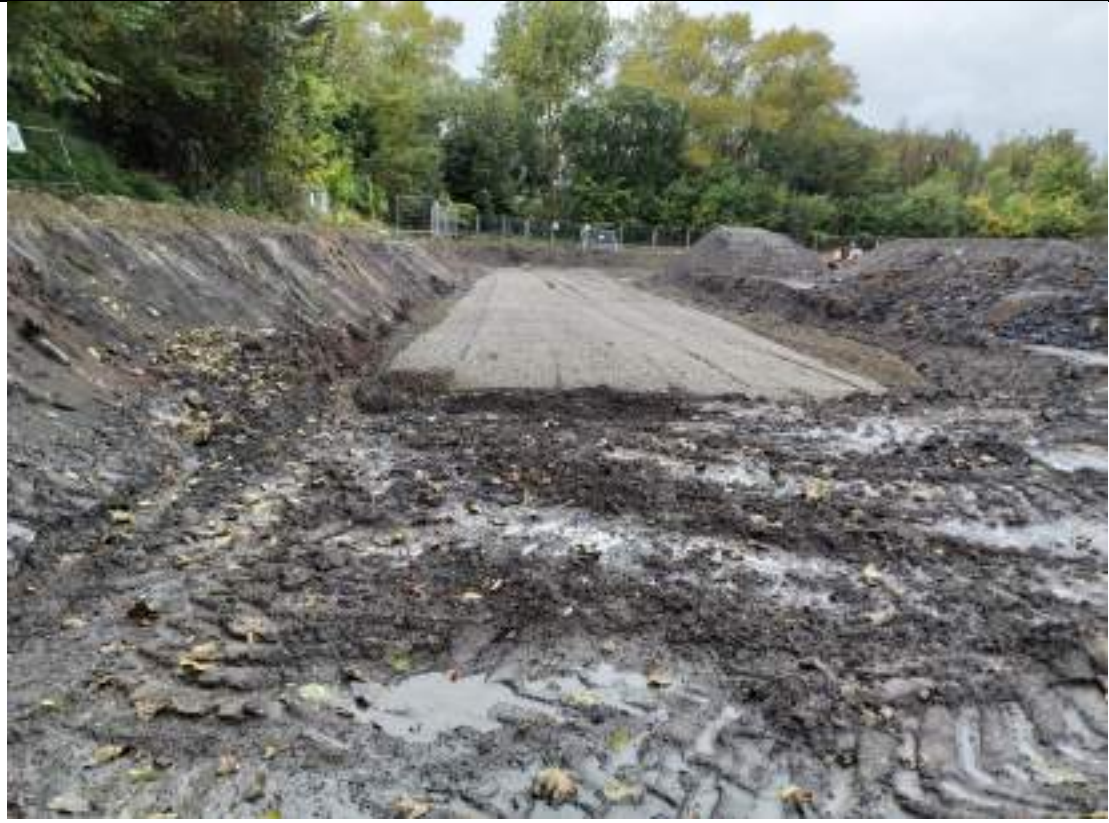
Photograph 21: Southern boundary of the site. Looking towards the west.
