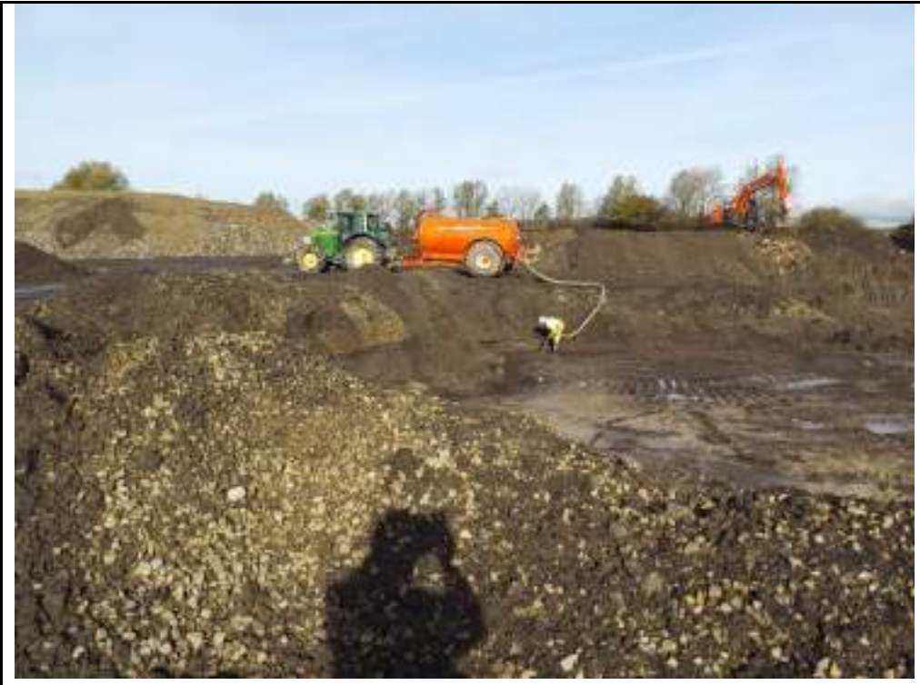
Photograph 3: Dewatering of excavation using tractor mounted pump in northeastern part of the site.
