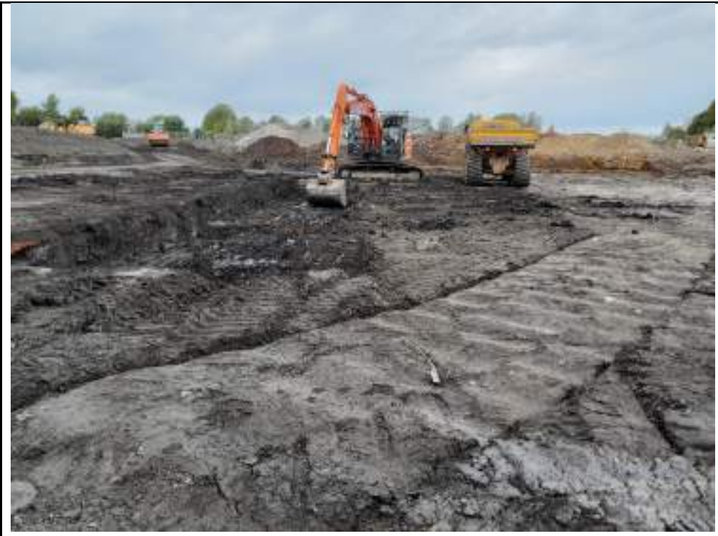
Photograph 3: Excavation of soft spot in southern part of the site.
