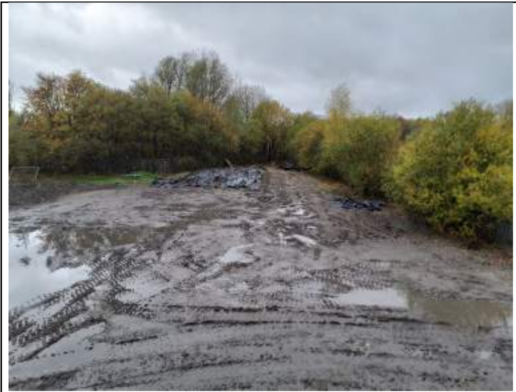
Photograph 10: Stockpile of TPH contaminated materials in western boundary of the site.
