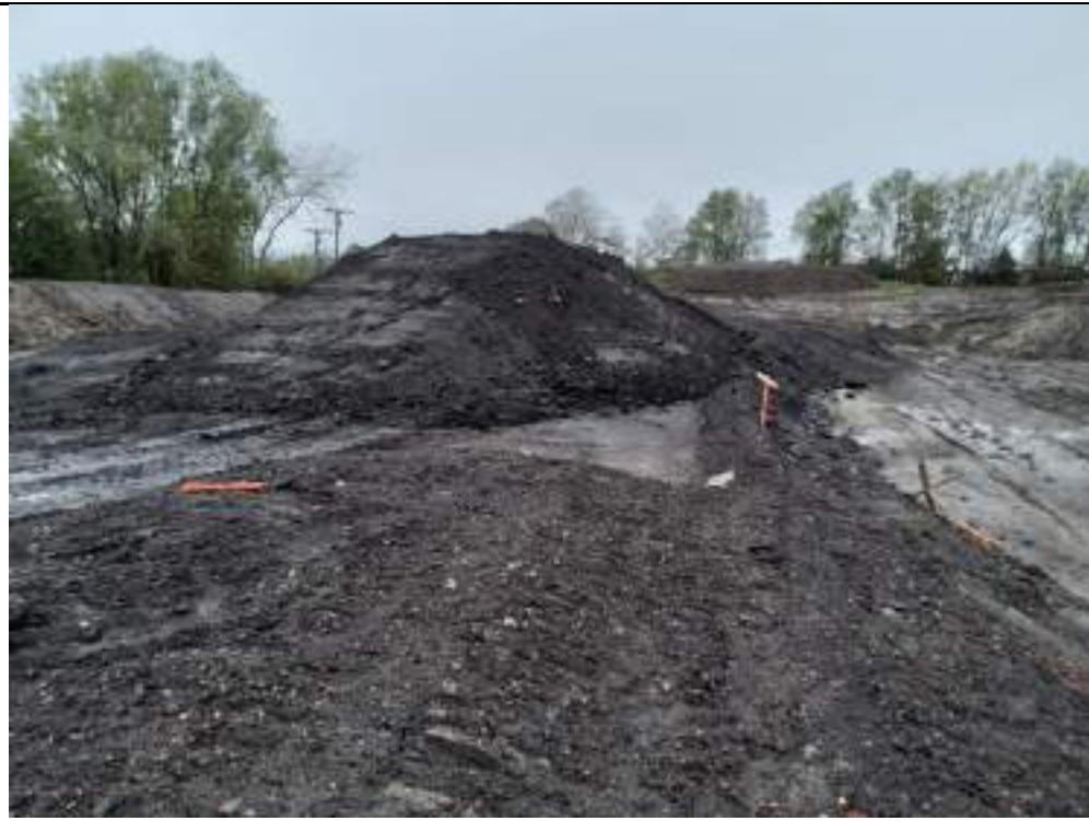
Photograph 6: Excavated peat stockpile in northwestern part of the site.
