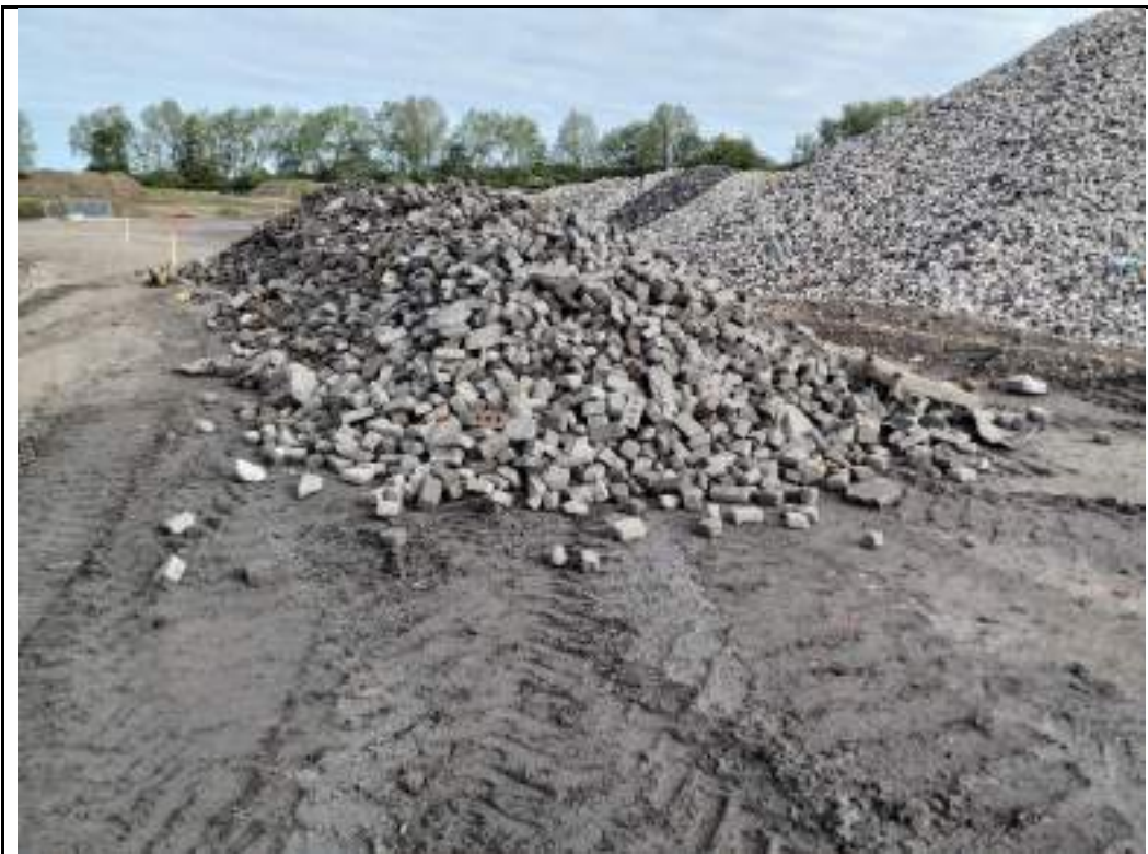
Photograph 14: Deleterious material and bricks stockpile in northwestern part of the site.
