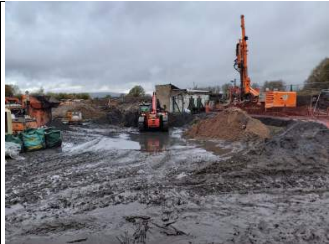
Photograph 2: Grouting shaft no.6 in eastern part of the site.
