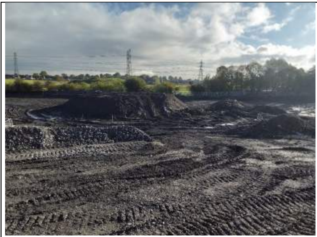
Photograph 14: Stockpiles of excavated materials in the northeastern boundary of the site.
