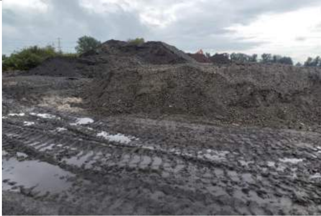
Photograph 53: Stockpiles of granular and landfill Made Ground in northeastern part of the site. Looking towards the east.
