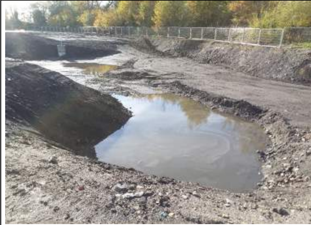
Photograph 11: Standing water in western part of the site.
