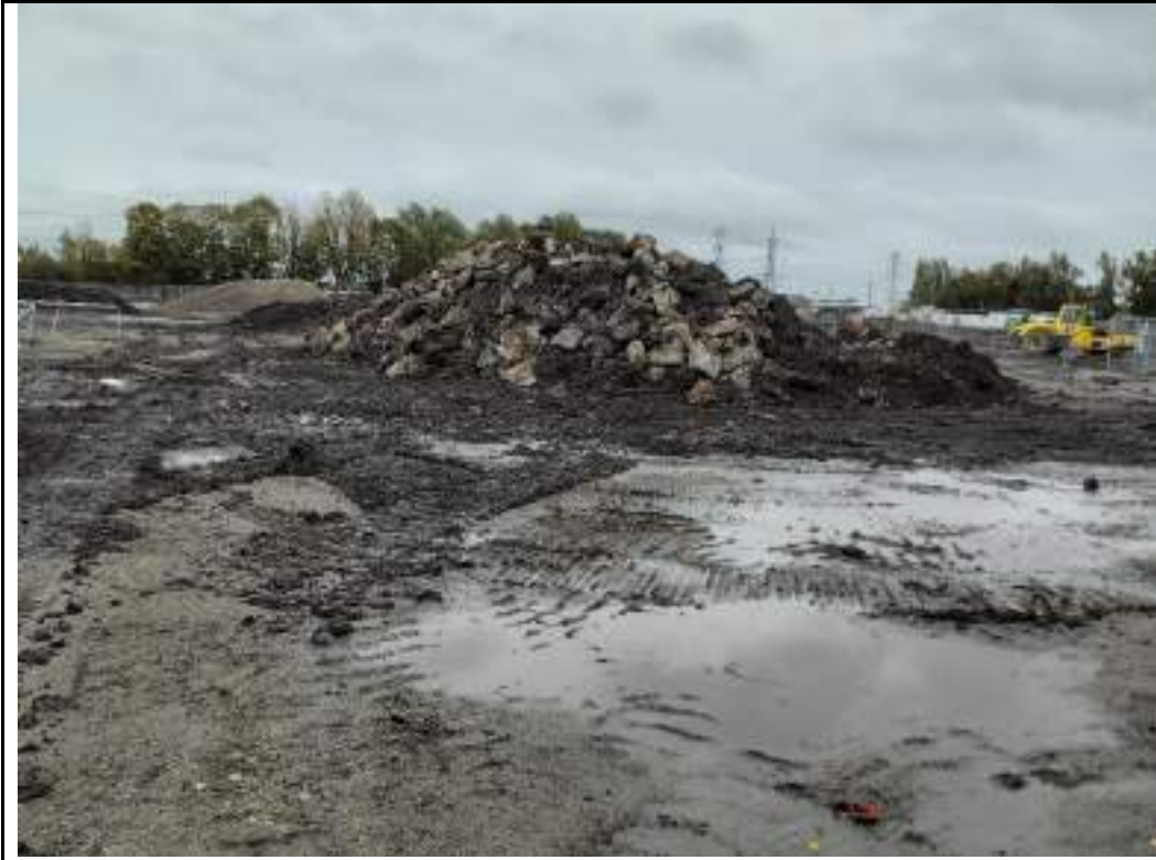
Photograph 23: Stockpile of excavated concrete in central part of the site.
