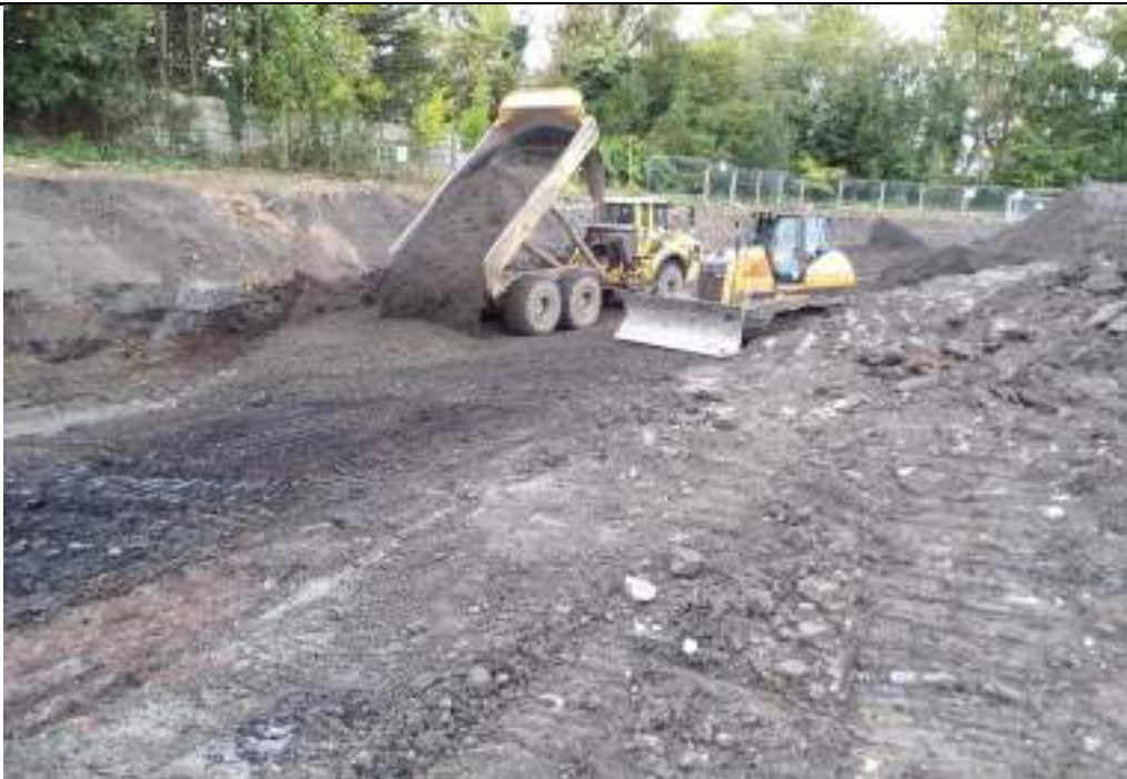
Photograph 22: Backfilling southwestern part of the site using processed material from eastern stockpile.
