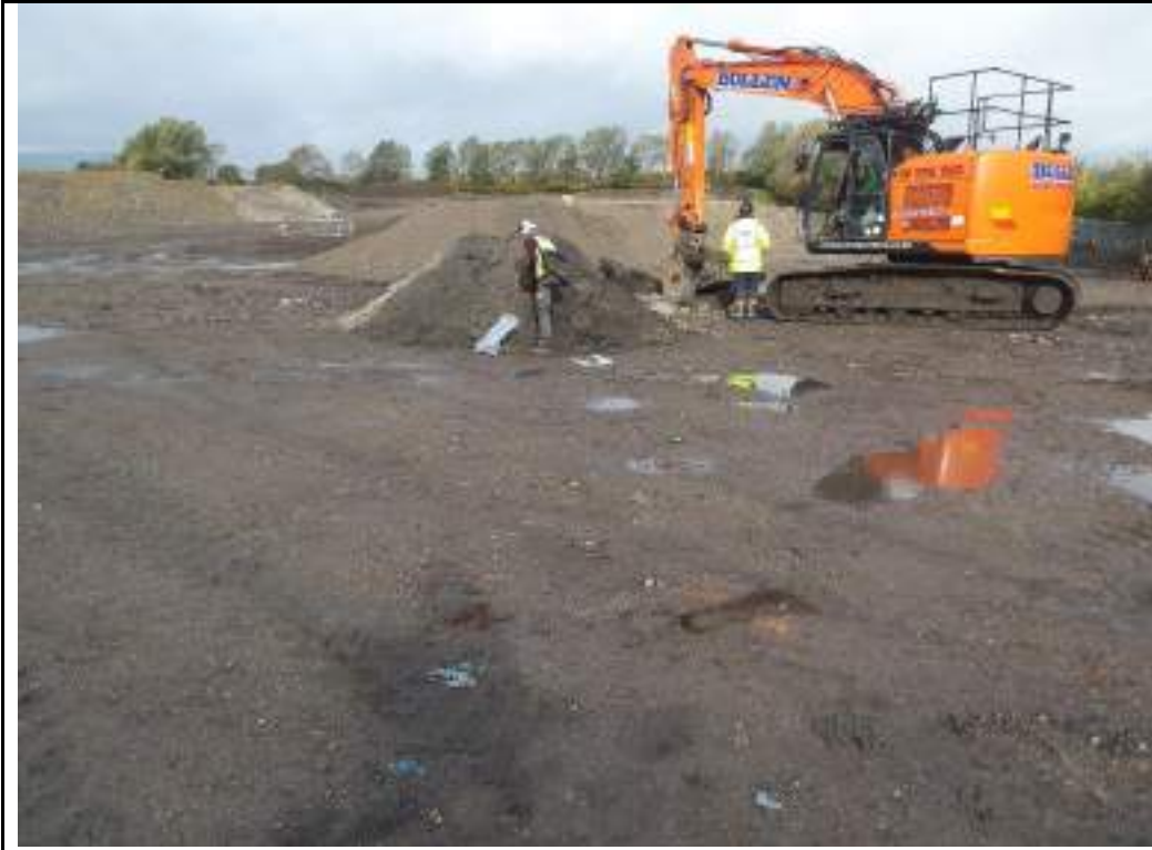
Photograph 21: Sample collection from excavated material from trial pit in eastern part of the site.
