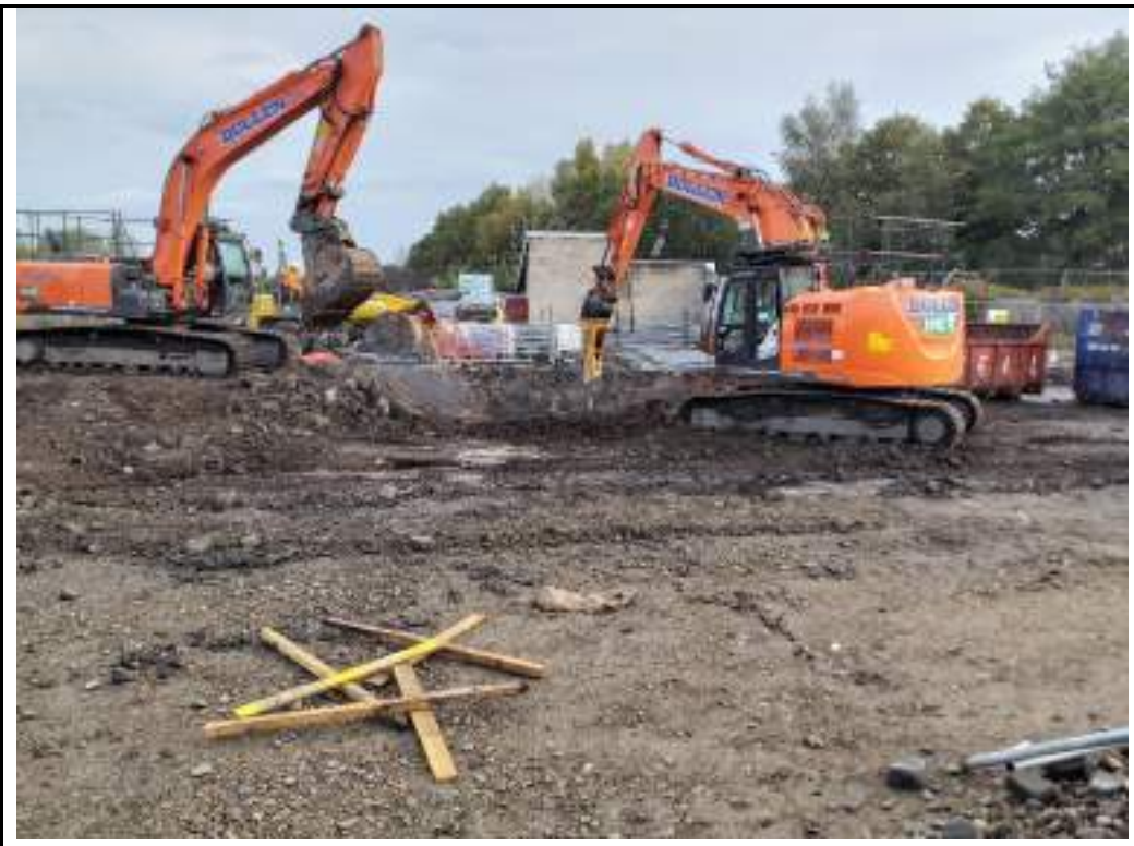
Photograph 2: Excavation of concrete and landfill Made Ground in southeast of the site.
