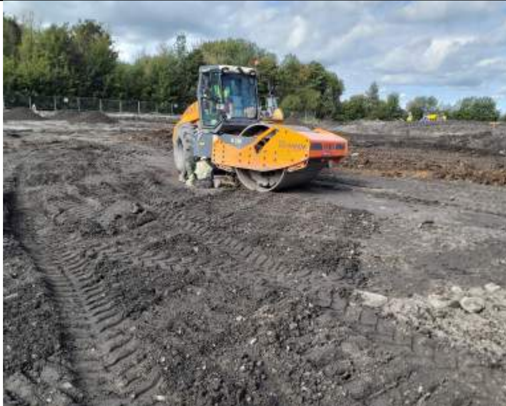
Photograph 32: Plate load testing in southern part of the site.
