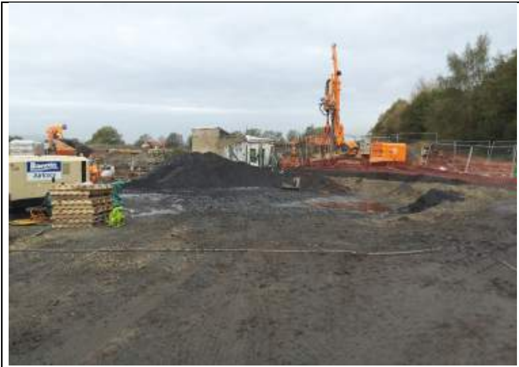
Photograph 2: Grouting shaft no.6 in eastern part of the site.
