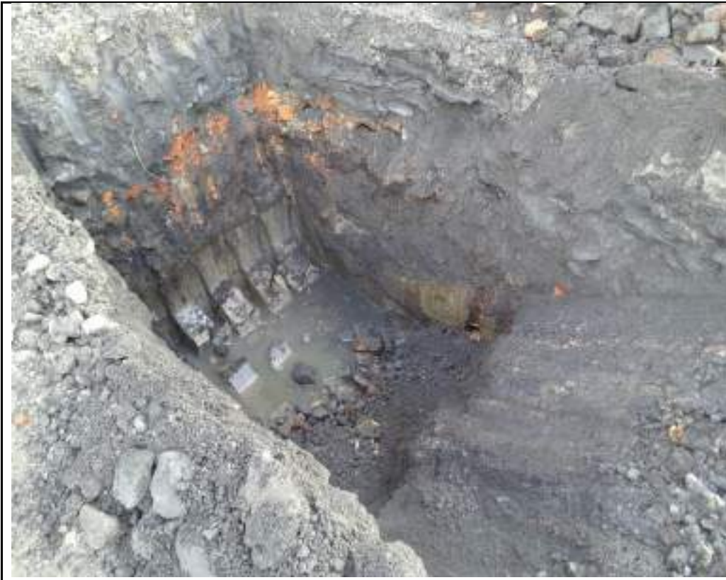
Photograph 23: Trial pit in eastern boundary of the site.
