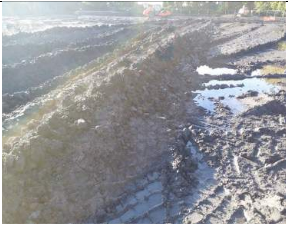
Photograph 8: Constructed temporary road using bricks and general fill to get access to southwestern part of the site.
