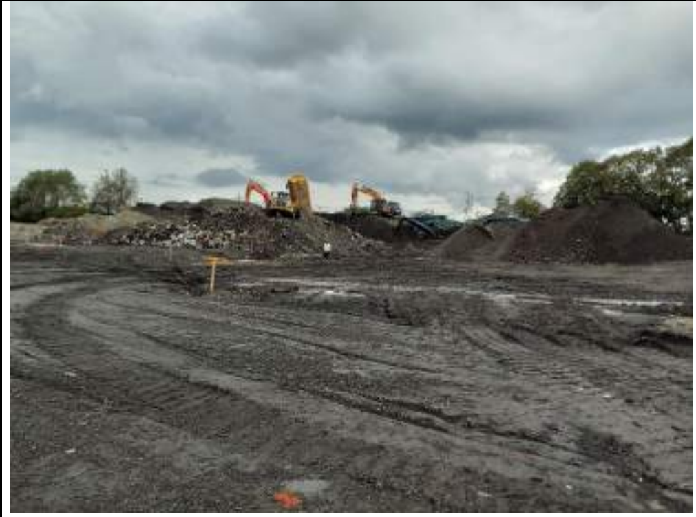
Photograph 3: Unloading excavated material from southeastern part of the site in stockpile in the northeast.
