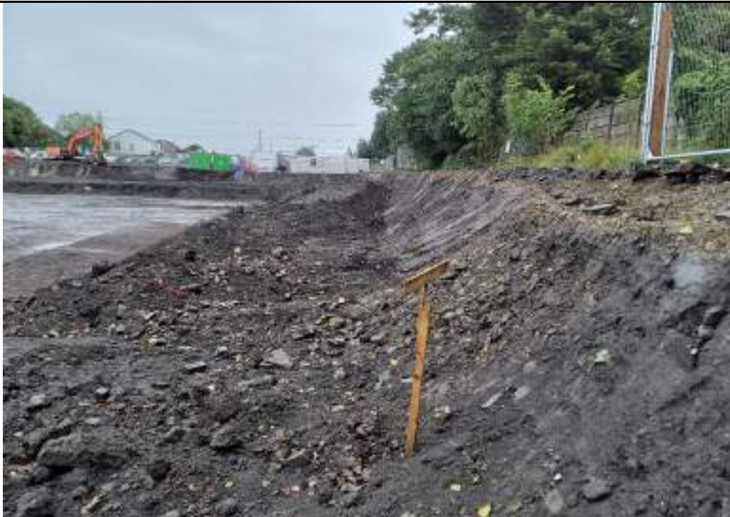
Photograph 8: Southern boundary of the site. Looking towards the east.
