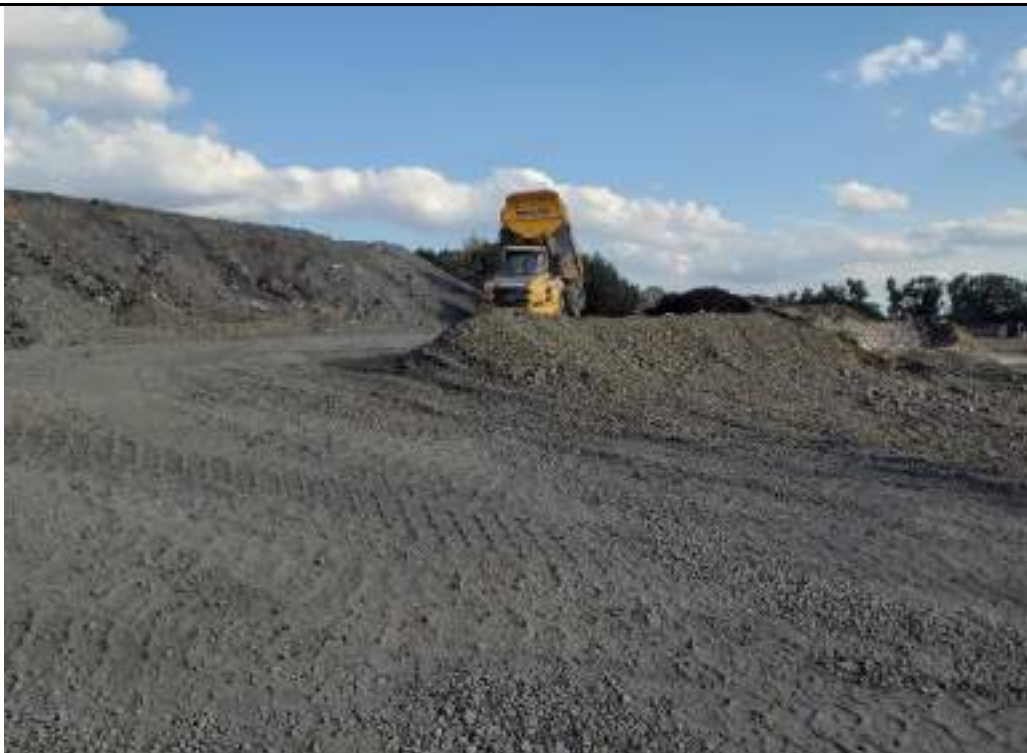
Photograph 20: Stockpiling excavated landfill Made Ground from southern part of the site in stockpile in northeast of the site.
