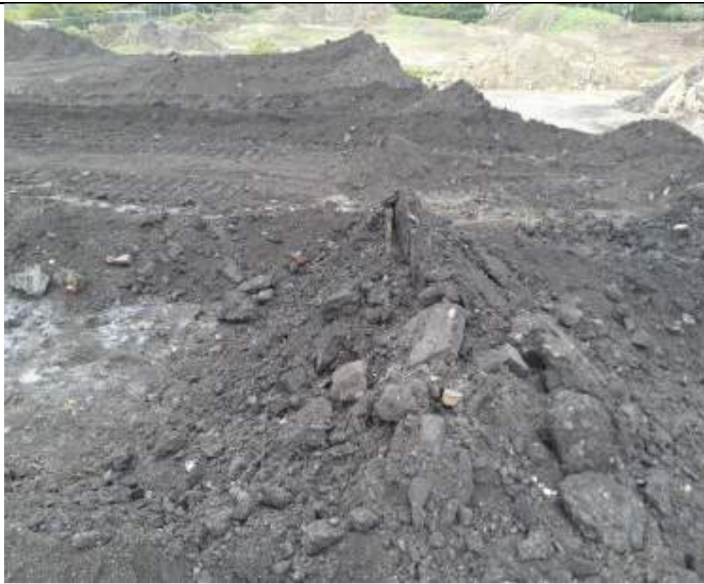
Photograph 8: Oversize in fill material in northwestern part of the site.
