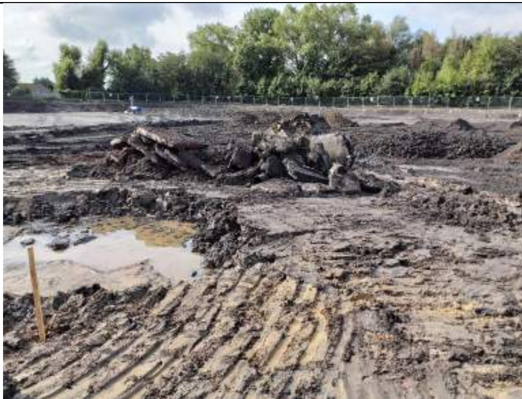
Photograph 158: Stockpile of excavated concrete in southeast of the site.
