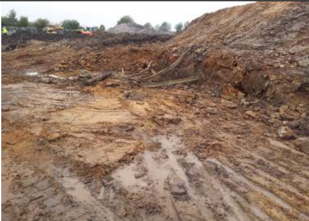
Photograph 20: Deleterious material in excavation in southeastern part of the site.
