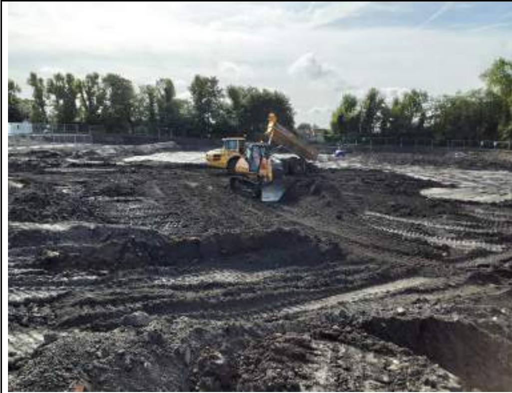
Photograph 125: Backfilling of southern part of the site using undersize material of screener.
