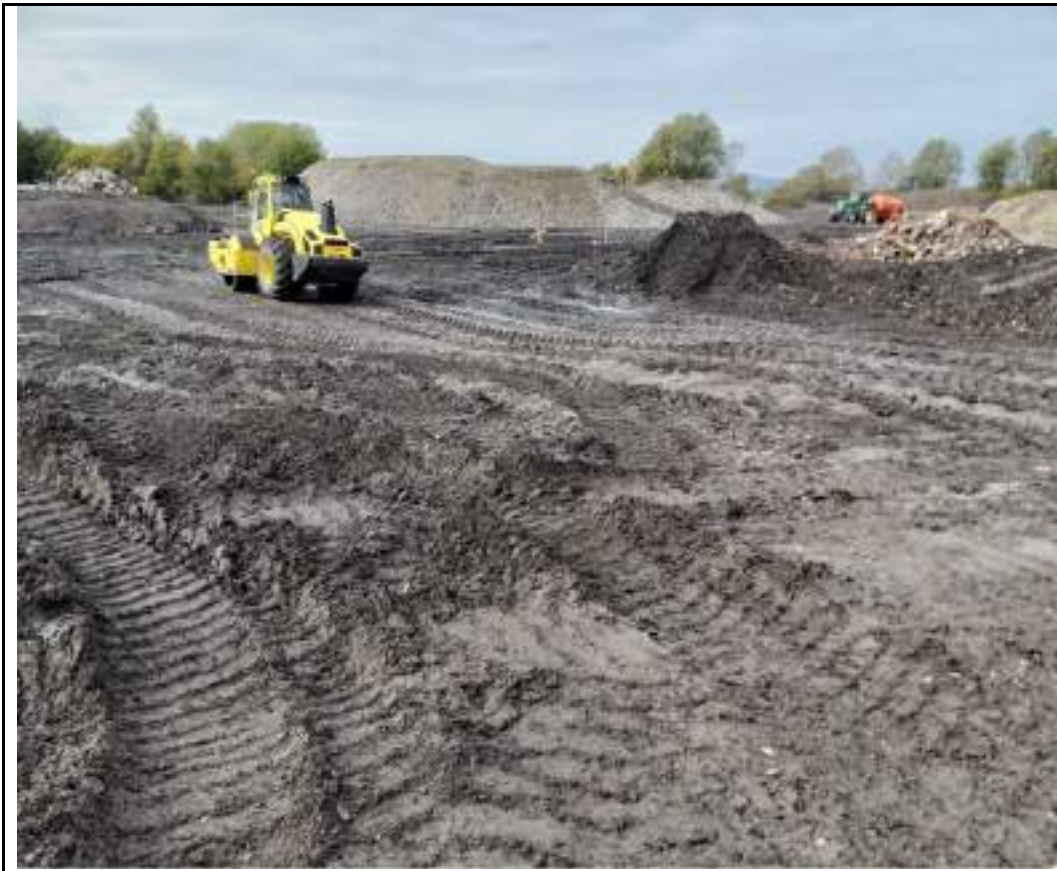
Photograph 19: Dynamic compaction in northeastern part of the site.
