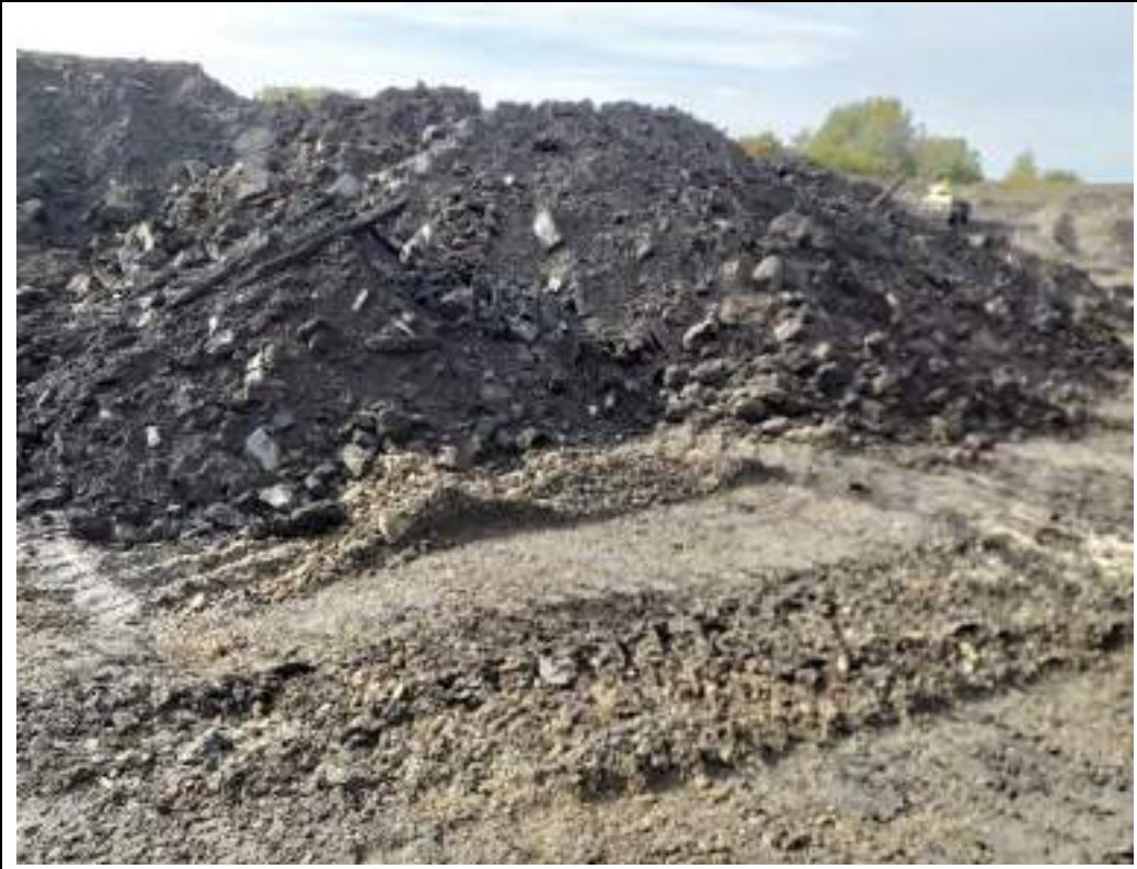
Photograph 11: Oversize and deleterious materials in northwestern part of the site.
