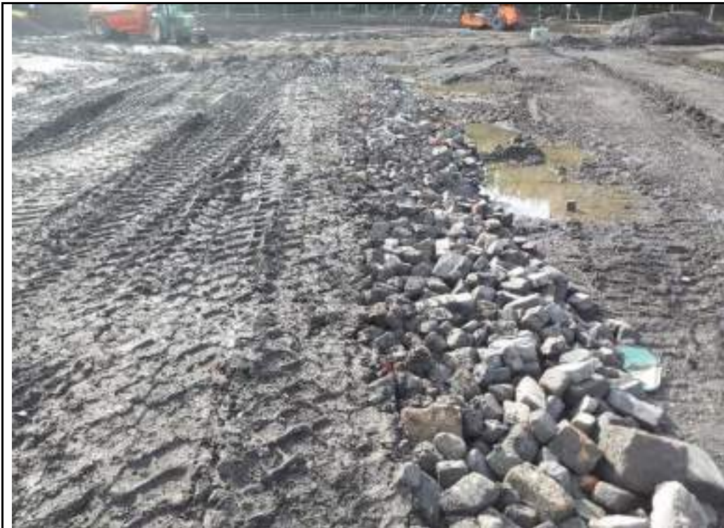
Photograph 15: Temporary Road construction using bricks and general fill materials in southwestern part of the site.
