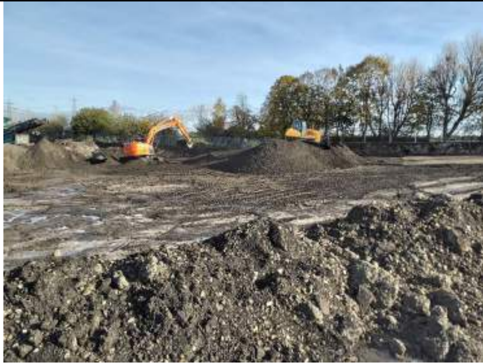
Photograph 5: Stockpiling processed material in northeastern part of the site.
