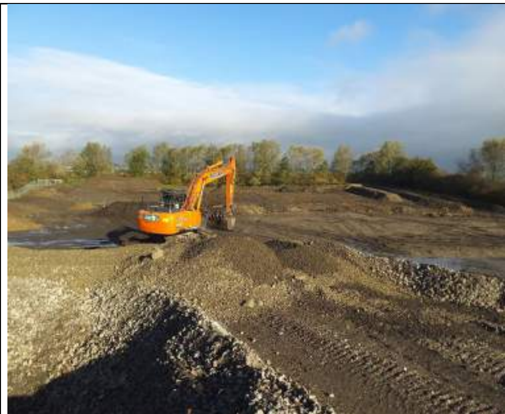
Photograph 12: Overview of stockpiles in northern part of the site.
