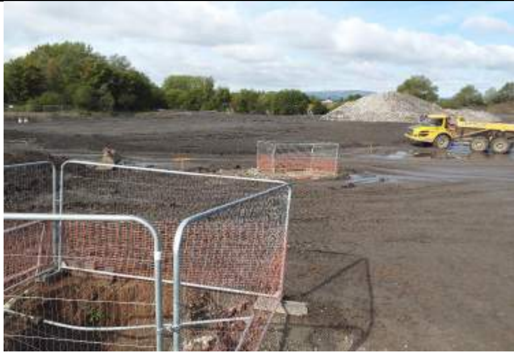
Photograph 5: Final ground level (general fill) in northwest of the site.
