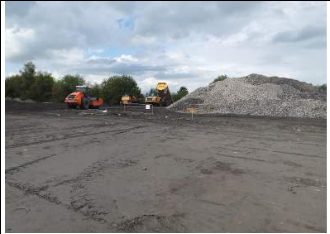
Photograph 169: Backfilling and proof rolling of northwestern part of the site.
