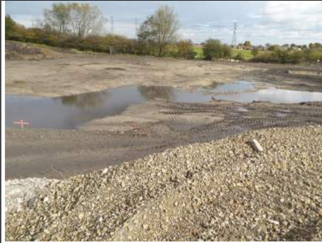
Photograph 21: Standing water in northern part of the site.
