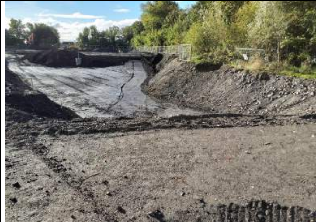
Photograph 11: Western boundary of the site. Looking towards the south.
