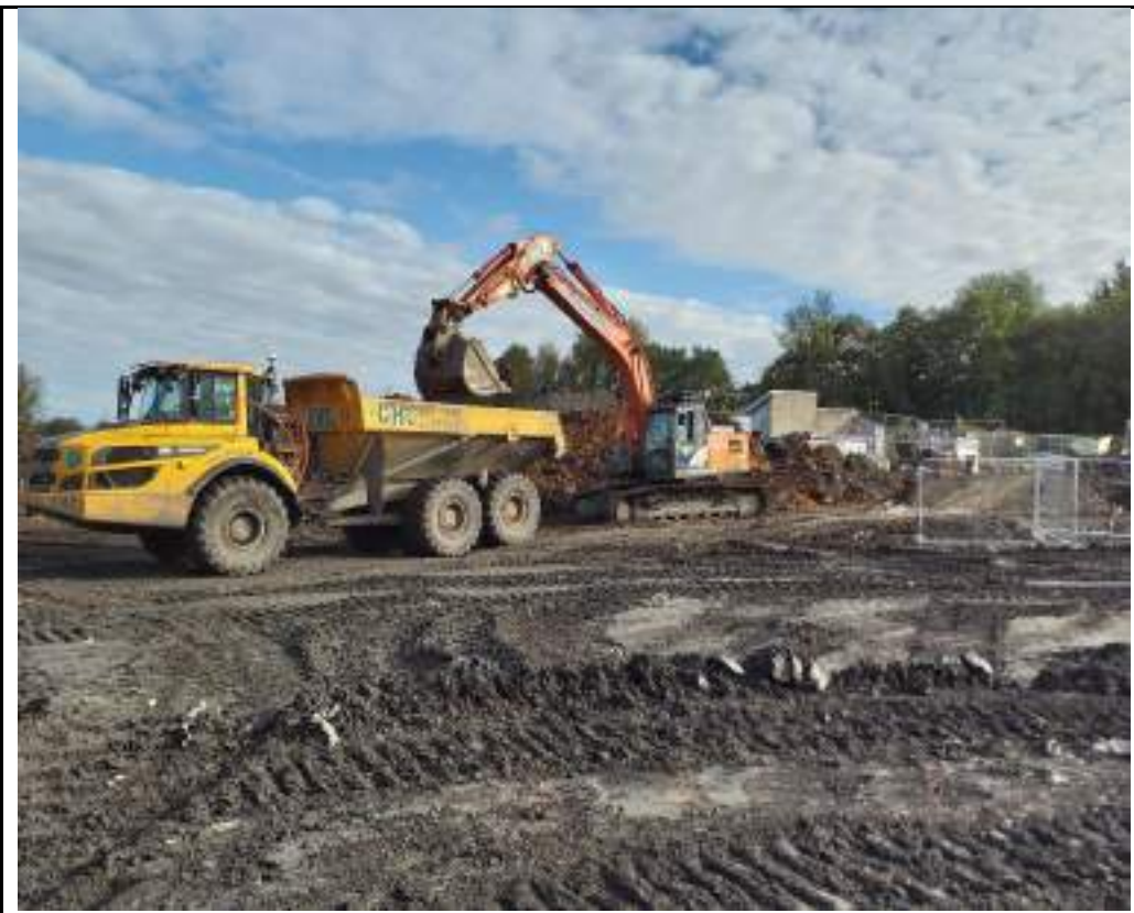
Photograph 2: Excavation of landfill Made Ground in southeastern part of the site.
