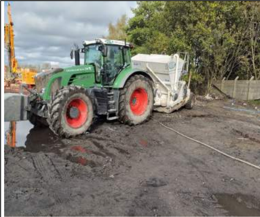
Photograph 21: Lime stabilization tractor in southeastern part of the site.
