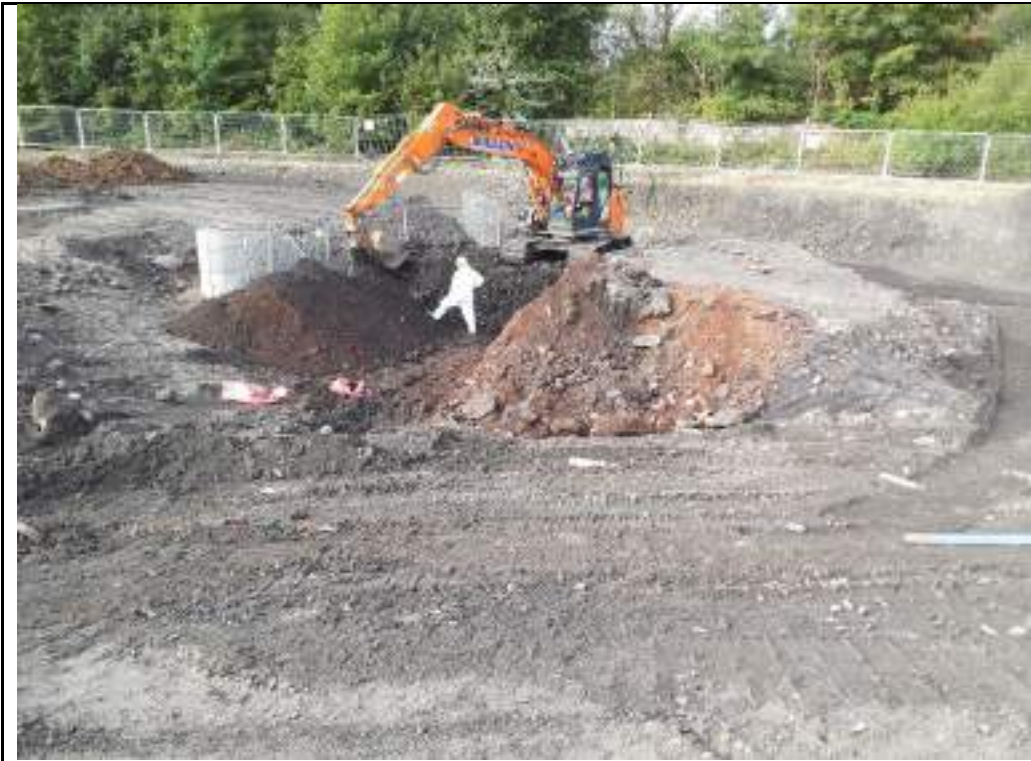
Photograph 91: Screening of the asbestos contaminated stockpile using riddle bucket excavator.
