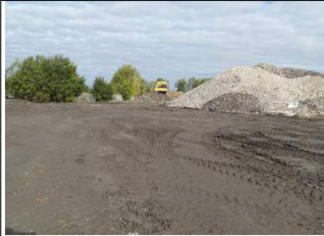
Photograph 169: Unloading bricks in northwest of the site.
