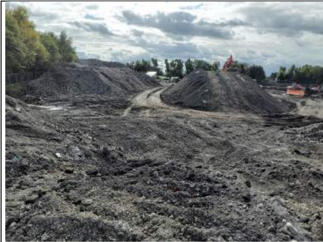
Photograph 29: Stockpiles of crushed materials from crusher and undersize materials from screener in eastern part of the site.
