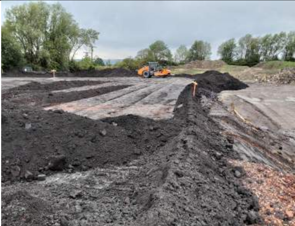
Photograph 24: Proof rolling over fill material in northwestern part of the site.
