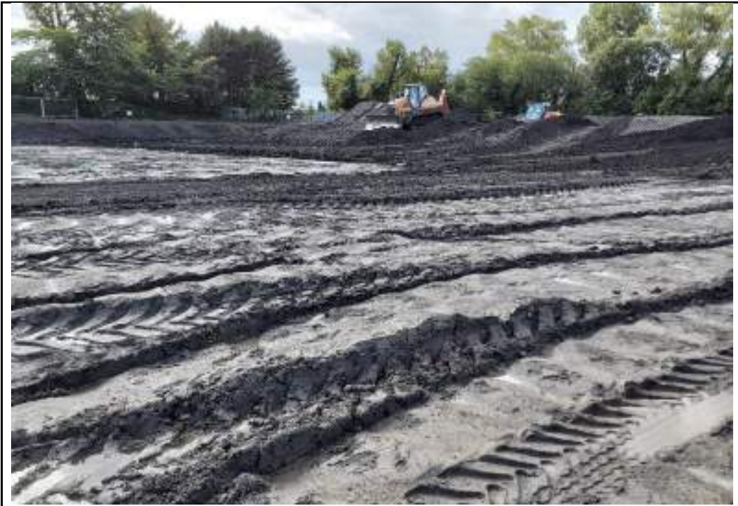
Photograph 21: Dozer pushing fill material to backfill southern part of the site.
