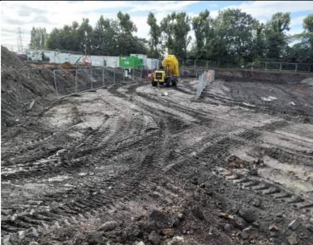
Photograph 20: New parking for VHE's trucks and equipment in southern part of the site.
