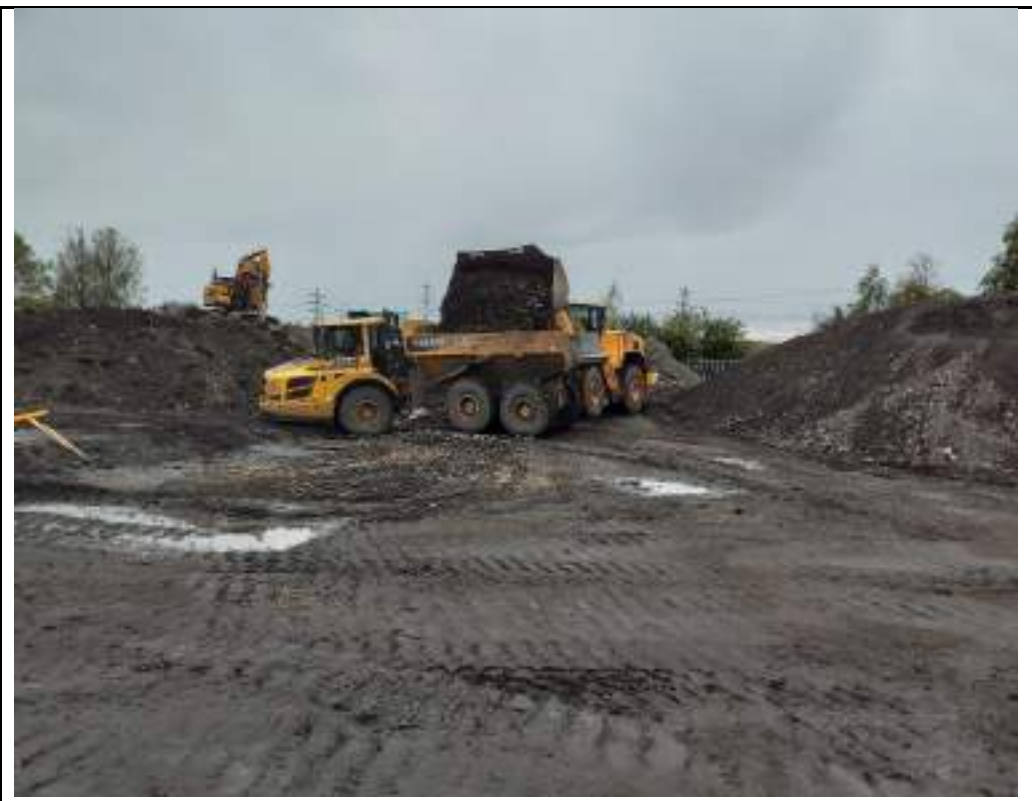
Photograph 10: Loading crushed material in northeastern part of the site.
