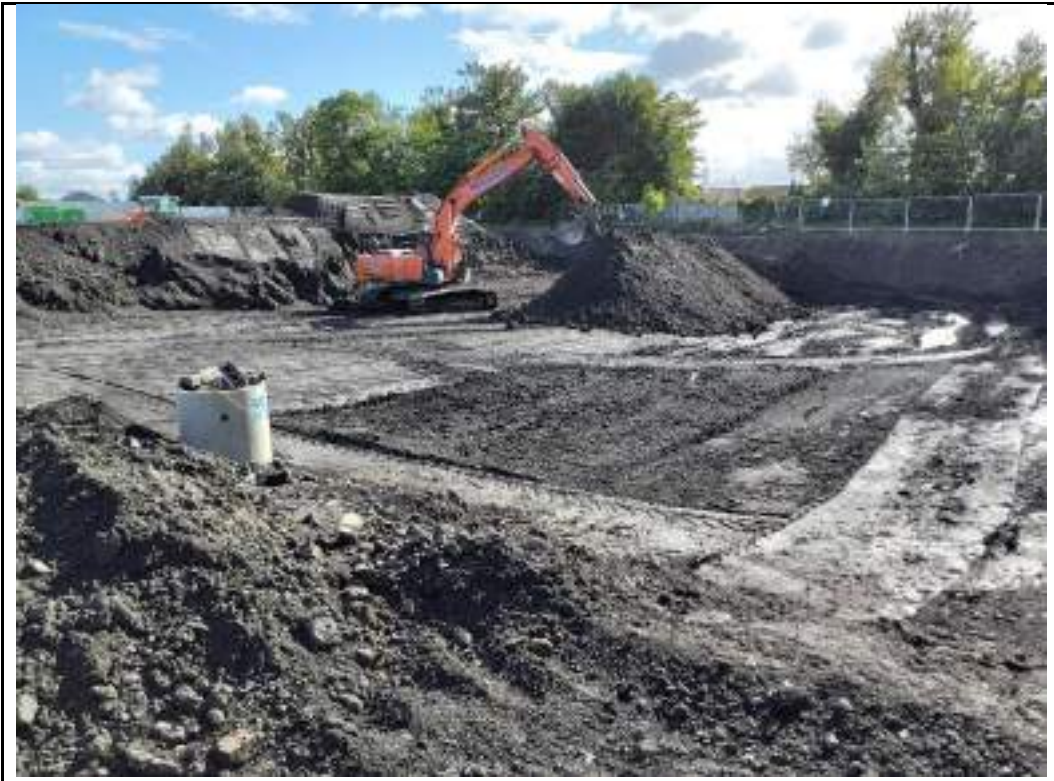
Photograph 93: Excavation of landfill Made Ground in southwestern part of the site.
