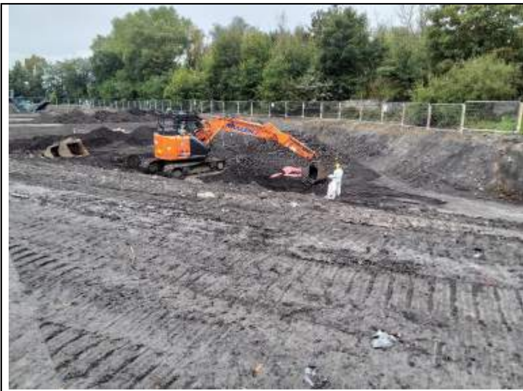
Photograph 110: Hand picking of asbestos in western part of the site.
