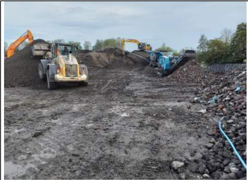
Photograph 91: Screener, crusher and stockpiles in northeastern part of the site.
