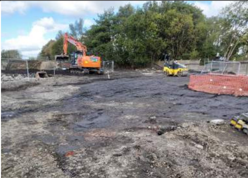
Photograph 22: Construction of shaft grouting platform in southeastern part of the site.
