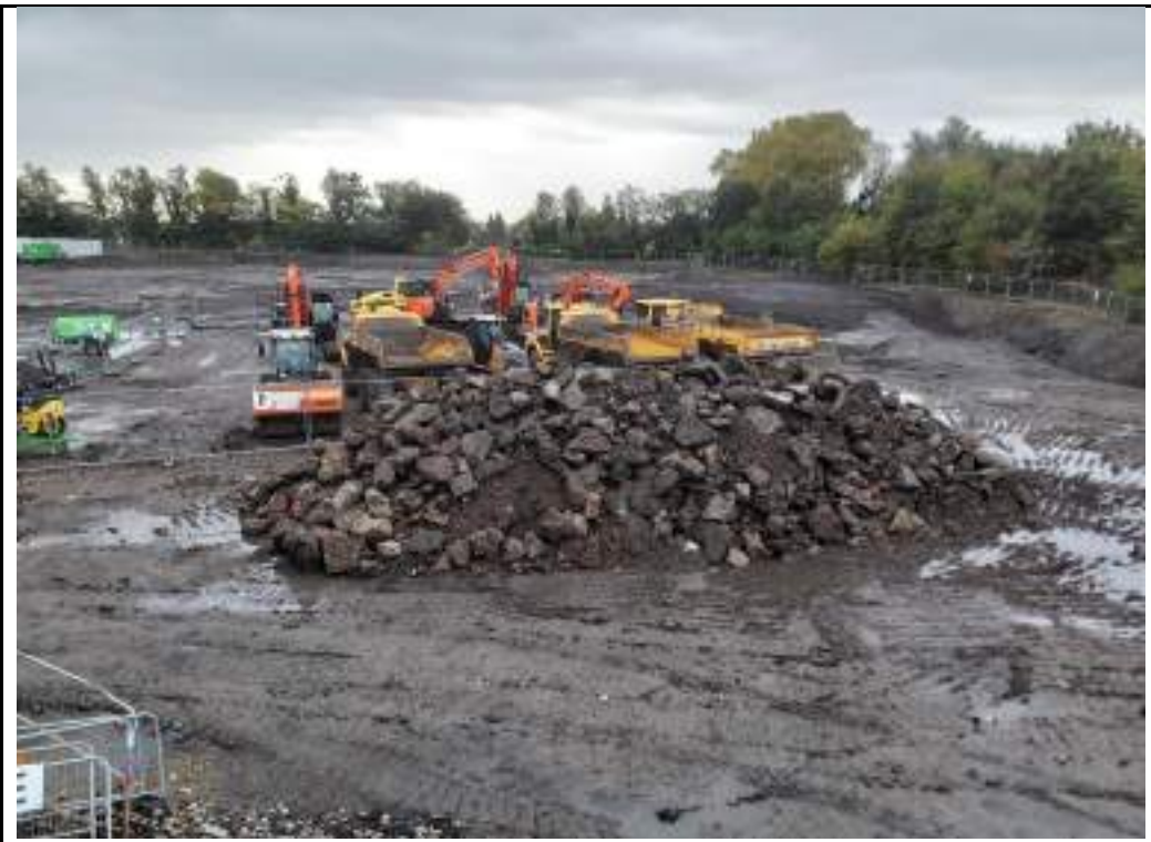
Photograph 10: Stockpile of excavated concrete and oversized material in southern part of truck parking.
