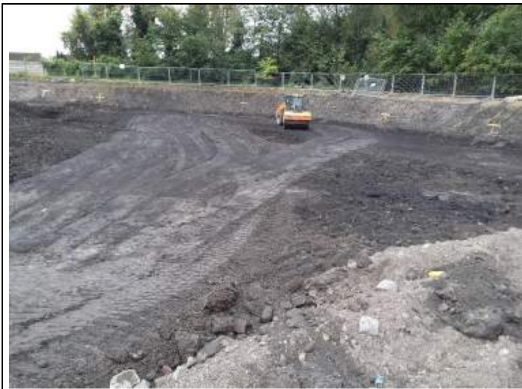
Photograph 10: Proof rolling of fill in southwestern part of the site.
