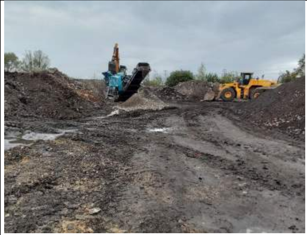
Photograph 9: Crushing oversize material from northeastern stockpile.
