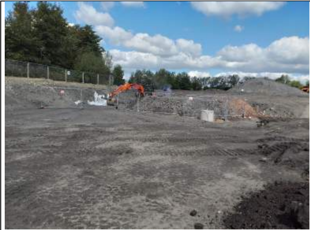
Photograph 113: Hand picking of asbestos in stockpile in western part of the site.
