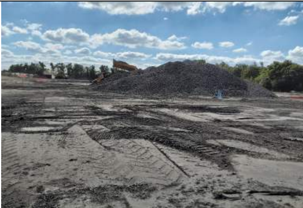
Photograph 20: Stockpiling crushed concrete and asphalt in northwest of the site.
