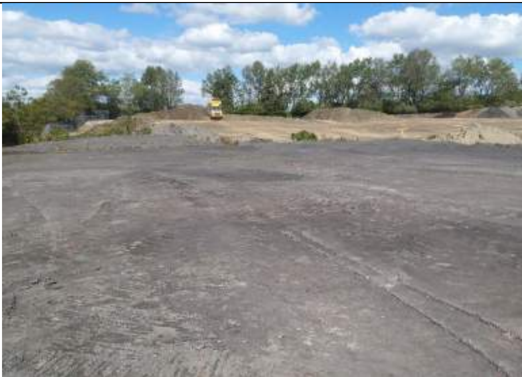
Photograph 20: Stockpiling excavated topsoil from northeastern part of the site in northwest of the site.
