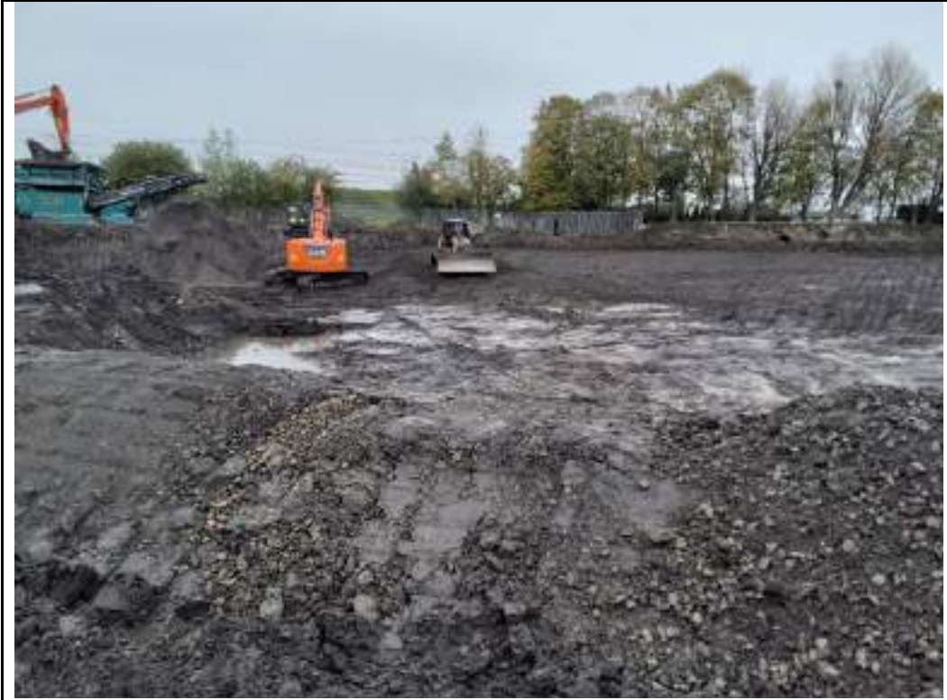
Photograph 93: Backfilling northeastern part of the site using processed material.
