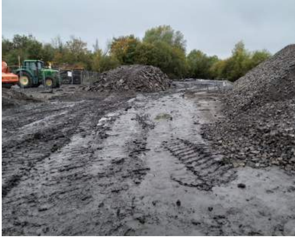
Photograph 17: Stockpile of concrete and oversize materials in northwest of the site.
