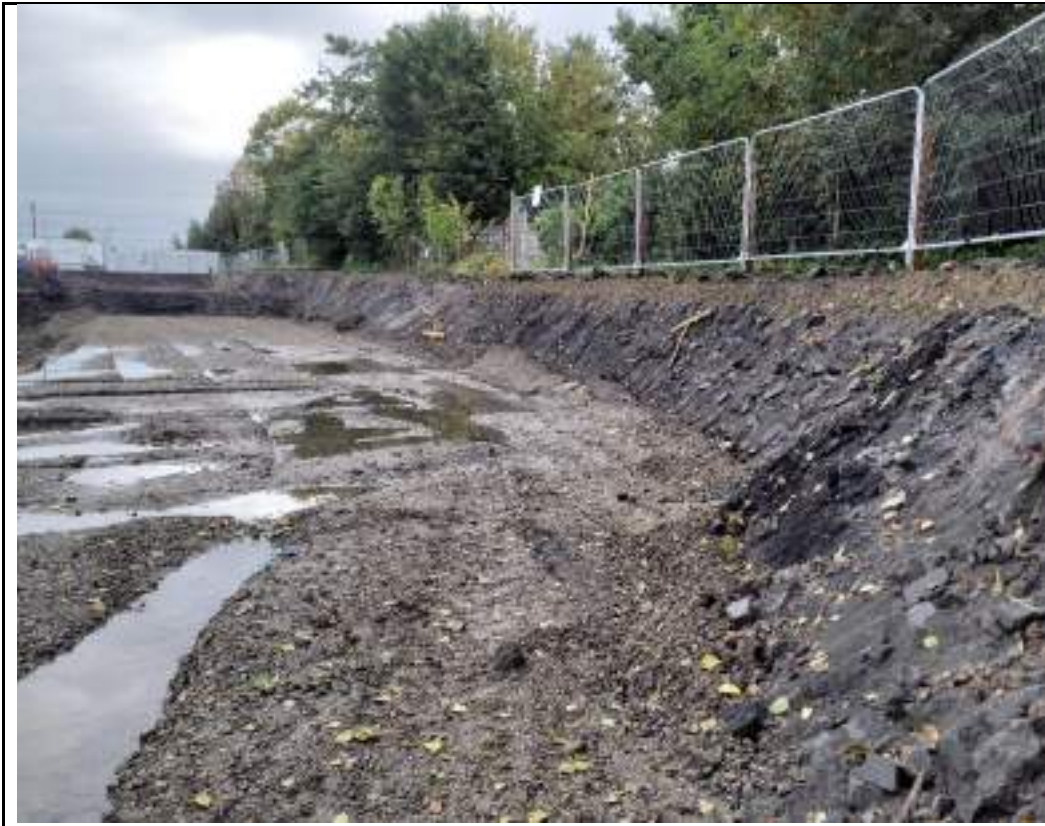
Photograph 15: Southern boundary of the site. Looking towards the east.
