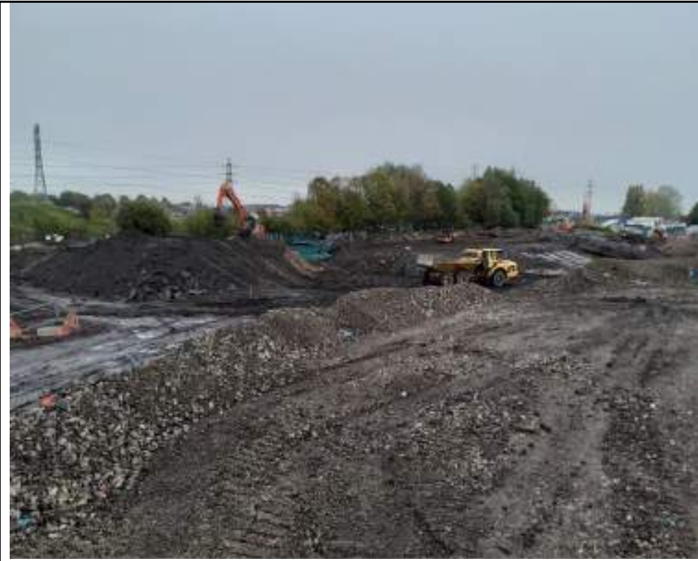
Photograph 1: Overview of the site. Looking towards the south.
