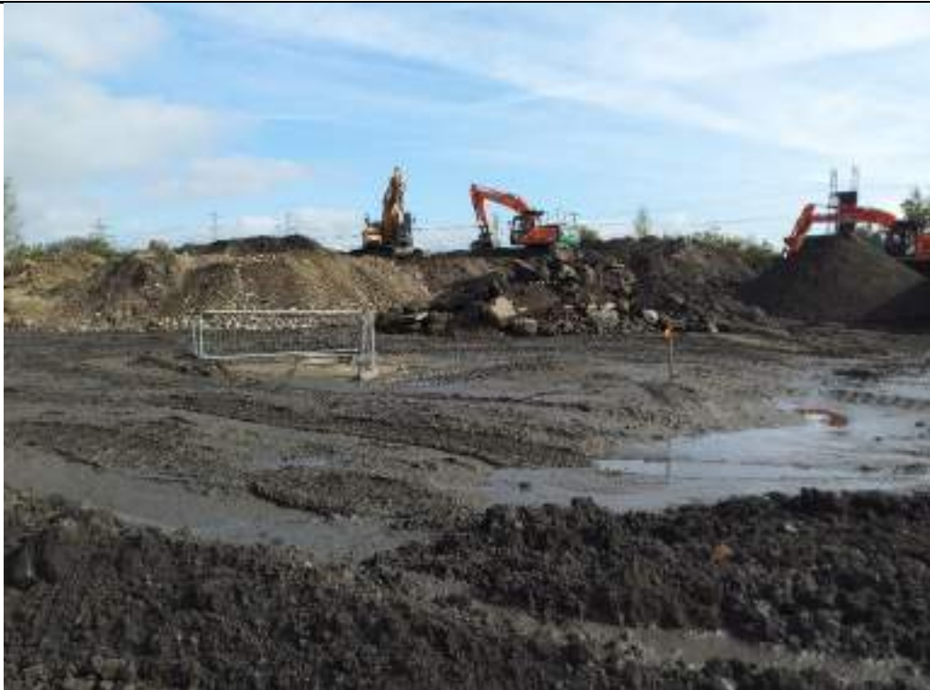
Photograph 24: Overview of stockpiles of excavated material in northeast of the site.
