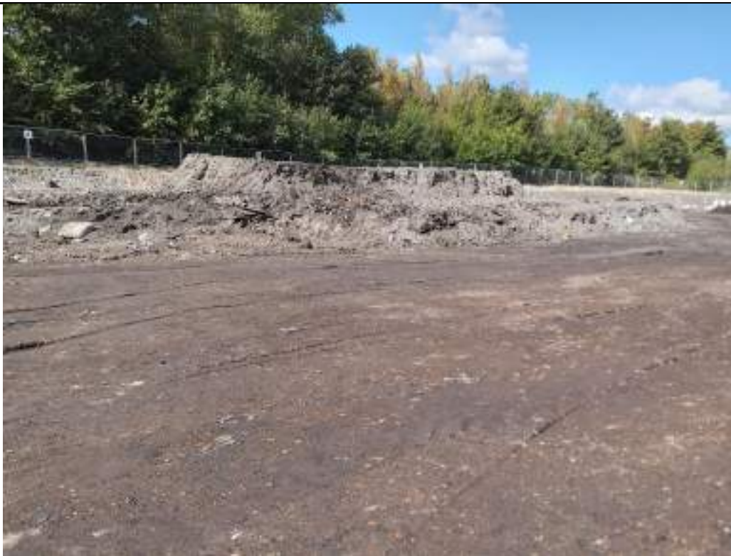
Photograph 158: Asbestos contaminated stockpile after asbestos picking operation in southwest of the site.
