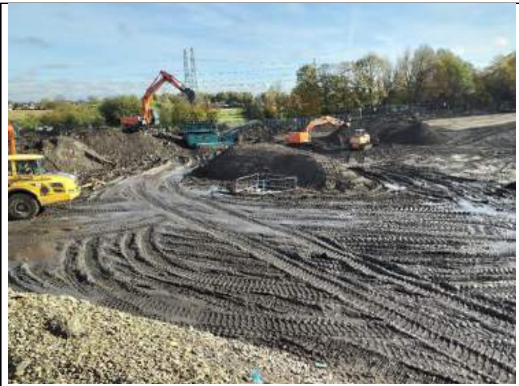
Photograph 4: Processing northeastern stockpile using screener.
