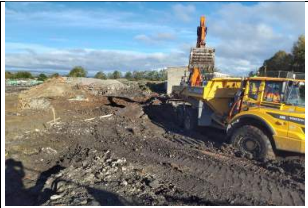
Photograph 2: Excavation of landfill Made Ground and Glacial Till in southeastern part of the site.
