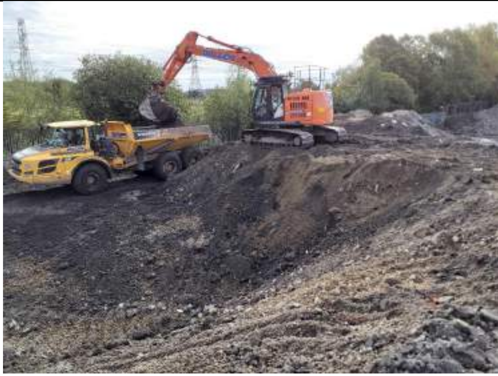
Photograph 5: Transferring material from northeastern stockpile to backfill southern and western part of the site.
