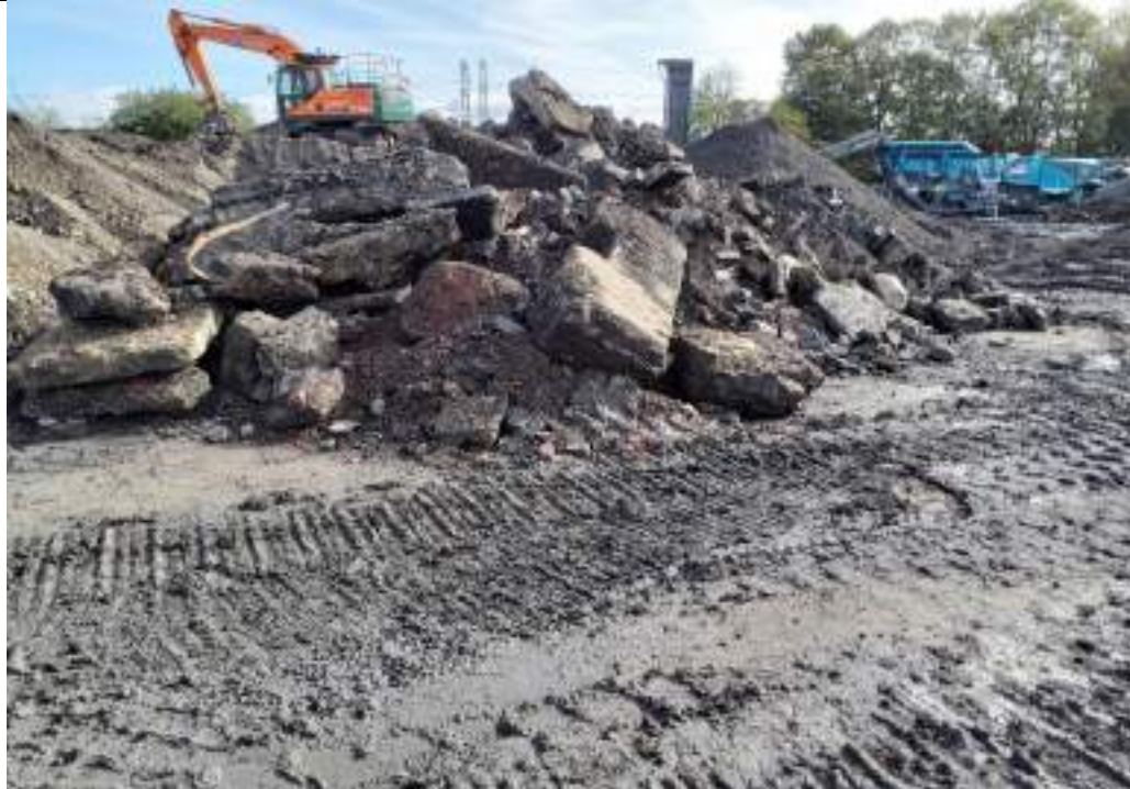
Photograph 26: Stockpile of excavated concrete in northeastern part of the site. Concrete excavated from southeast of the site.
