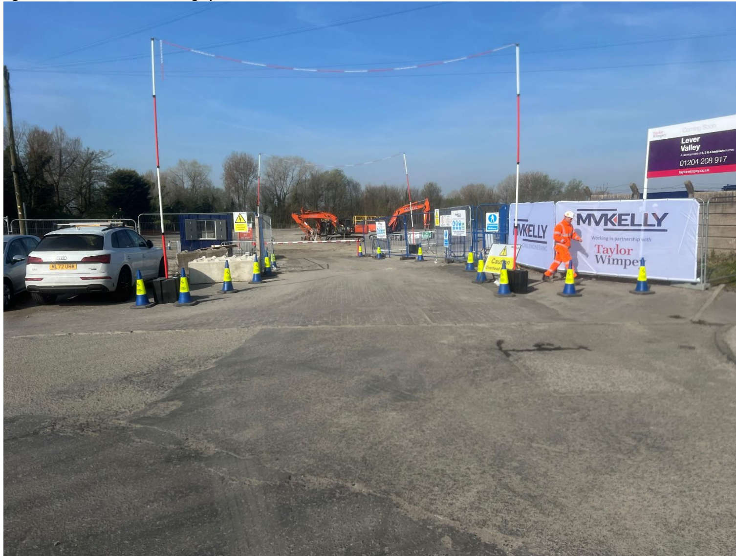
Figure 8: Current Site Access Photograph
