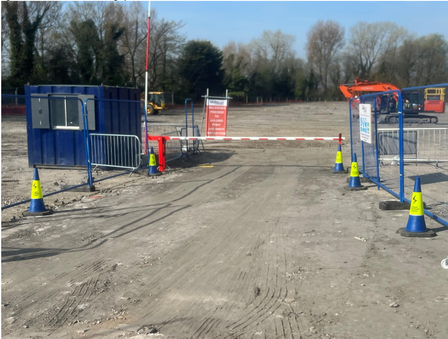
Figure 9: Current Site Access Photograph 2
