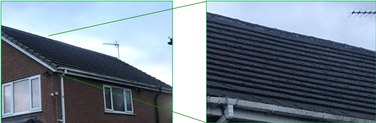
Tight-fitting tiles on the south elevation
