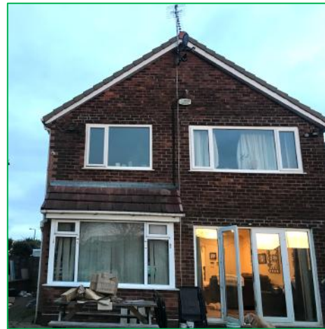
The west elevation of the property
