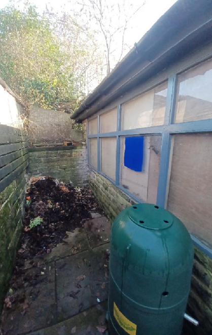
Sides of the garage:
