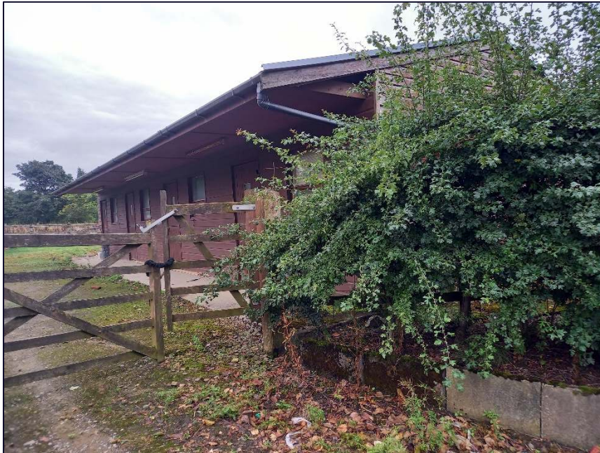
Plate 1: View looking east from Arthur Lane showing the entrance gate and the stable block within the proposed development site boundary
