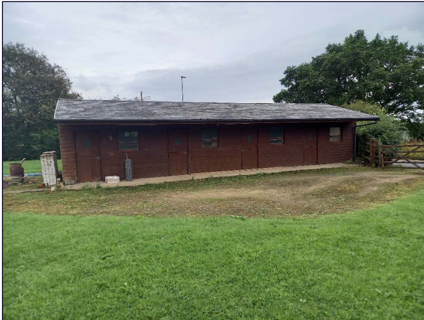
Plate 3: North elevation of the stable block, with Arthur Lane to right of photograph
