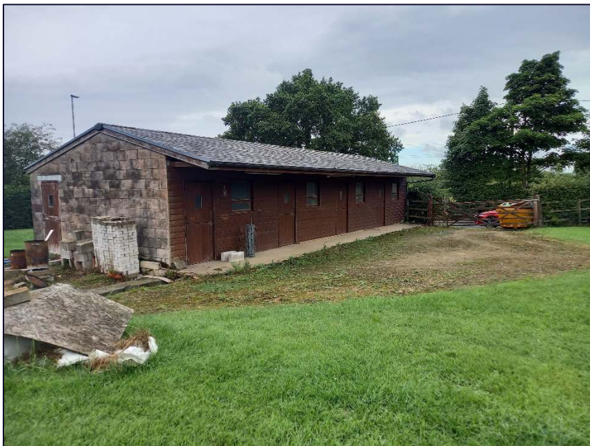
Plate 4: View looking west towards Arthur Lane showing the modern stable block
