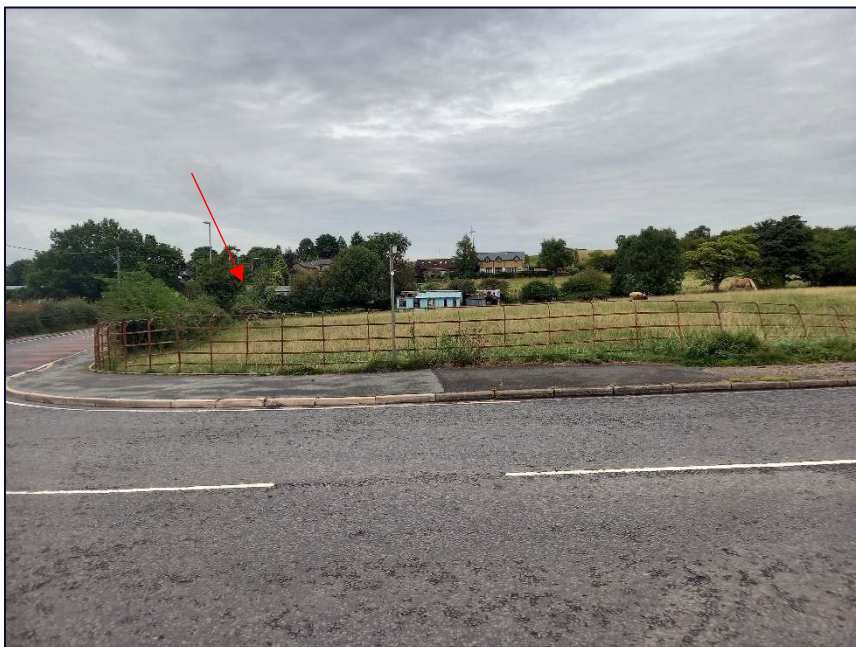
Plate 10: View looking north from the north end of the access track to Dearden Fold Farm. The roof of the stable block within the proposed development site is only just visible among the vegetation (marked with the red arrow)
