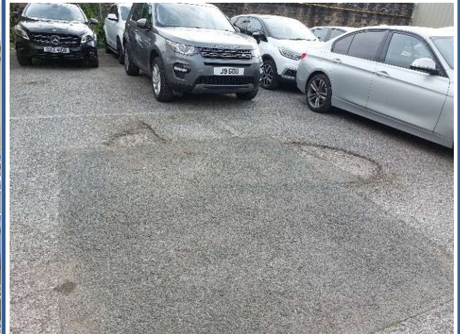
Image 18: Northeastern area of the site, some areas of resurfaced tarmac and new potholes evident. Facing east.
