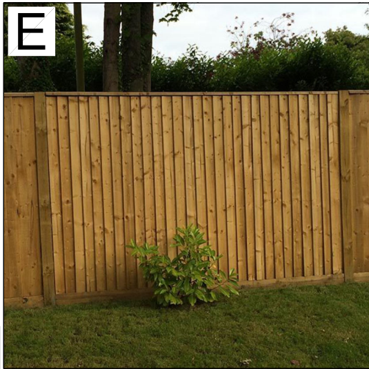
Image E: Closeboard timber fencing
