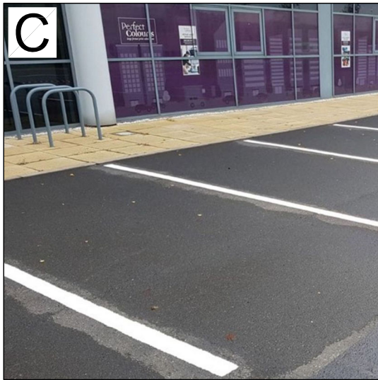
Image C: Tarmac with Resincoat car park line marking paint.
