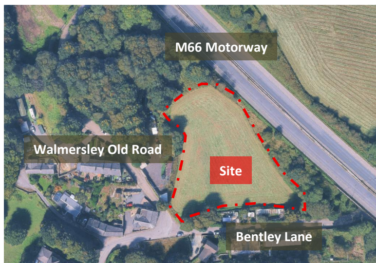
Figure 1.1 Aerial view of site location, image © Google Earth
